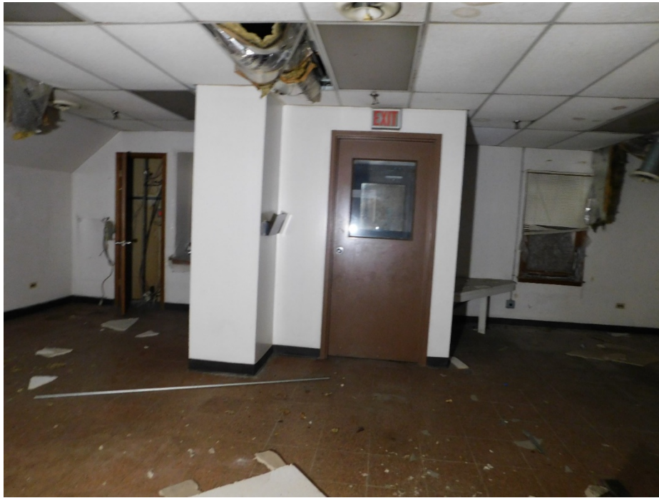
Figure 13: Interior view of second floor door to outside.
