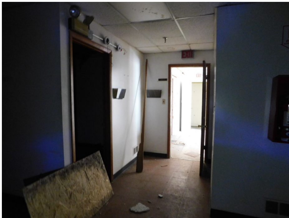
Figure 12: View of second floor hallway.
