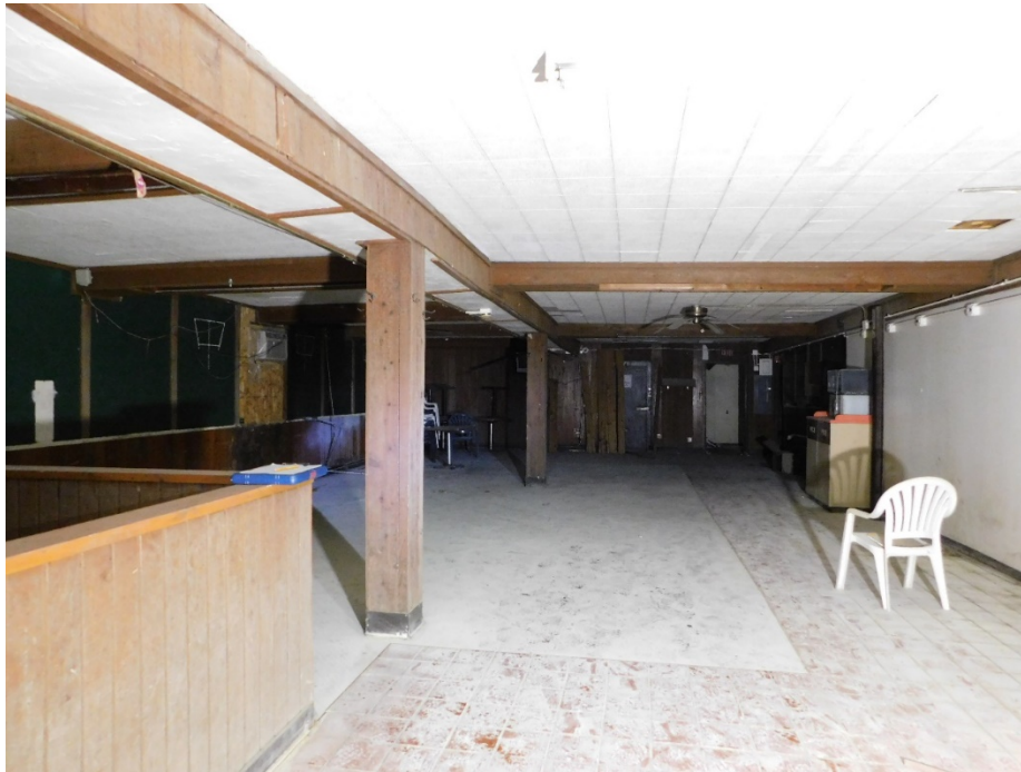
Figure 7: First floor looking west.
