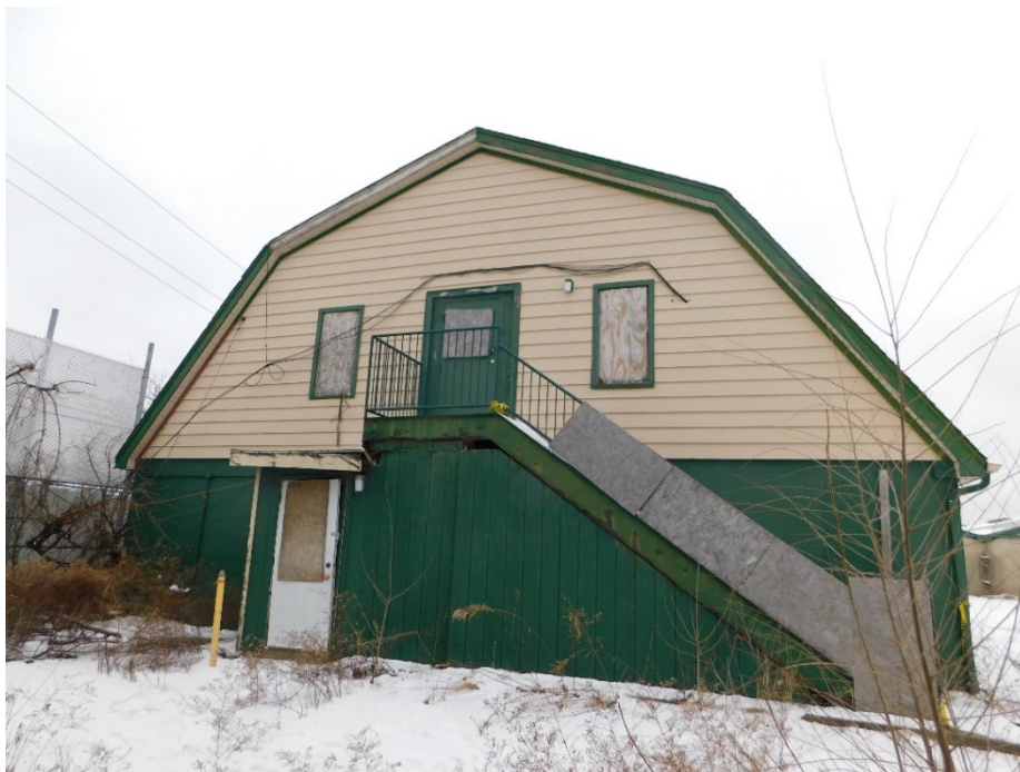
Figure 6: View of east elevation.
