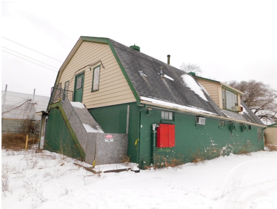
Figure 5: View of east (left) and north elevations.
