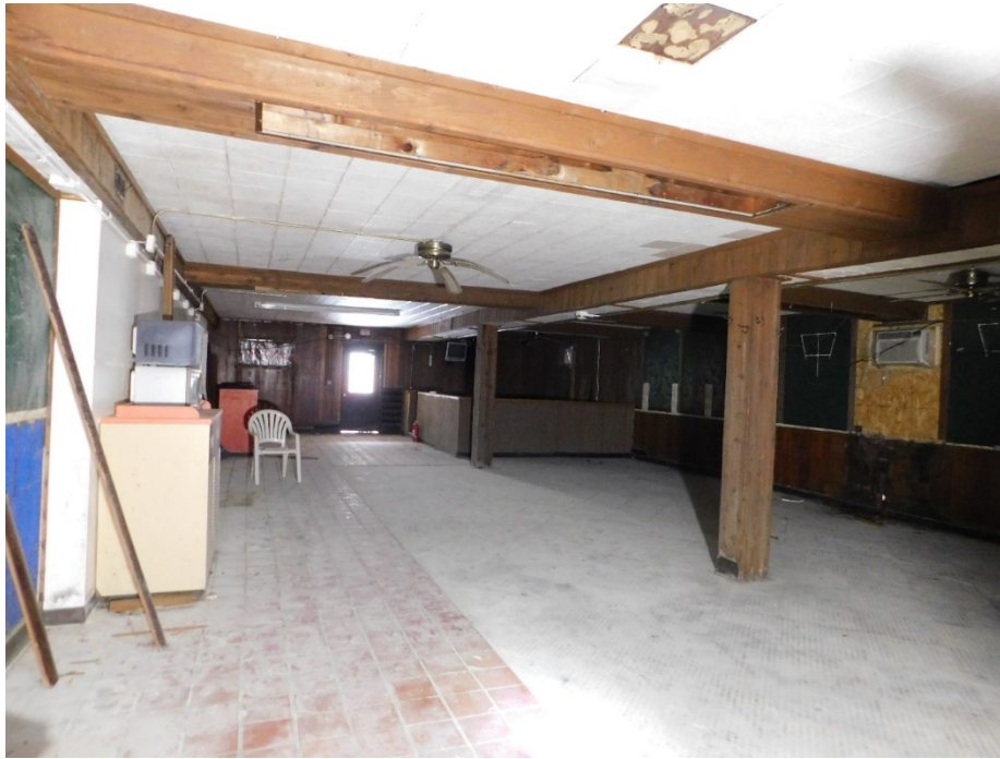
Figure 9: View of first floor looking east.
