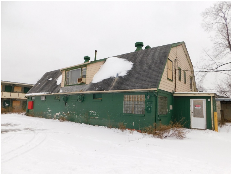
Figure 3: View of north (left) and west elevations.
