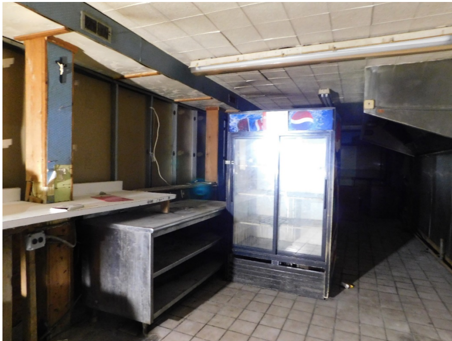
Figure 8: View of first floor kitchen area.
