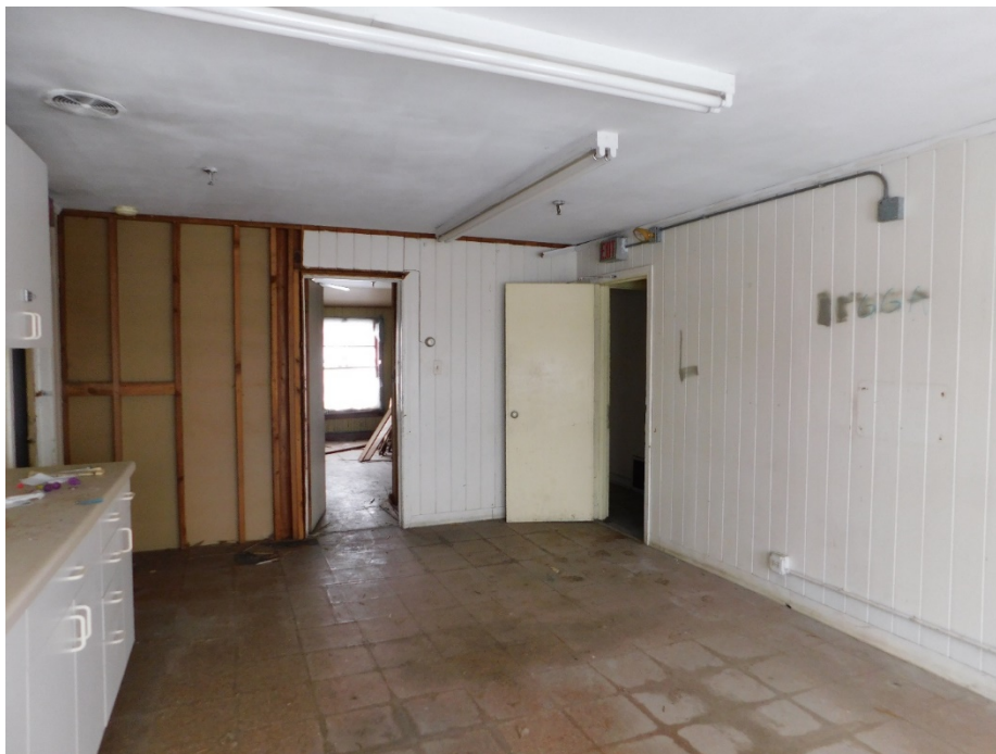
Figure 10: View of former dentist's office on second floor.
