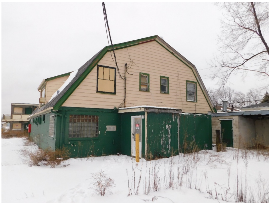
Figure 4: View of west elevation.
