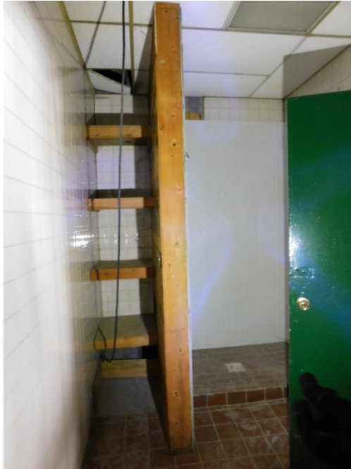
Figure 15: Shower stall off the carpentry room.
