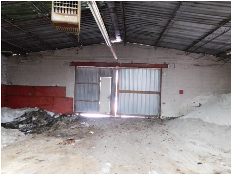
Figure 8: Interior view of side elevation entrance.
