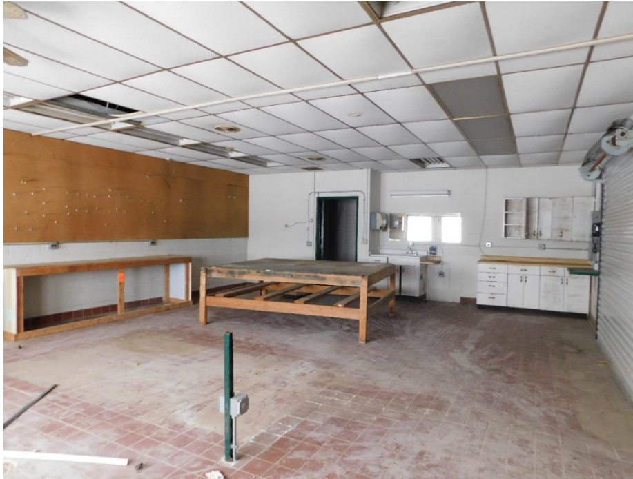
Figure 13: Carpentry room (former sandwich shop/driver locker room).
