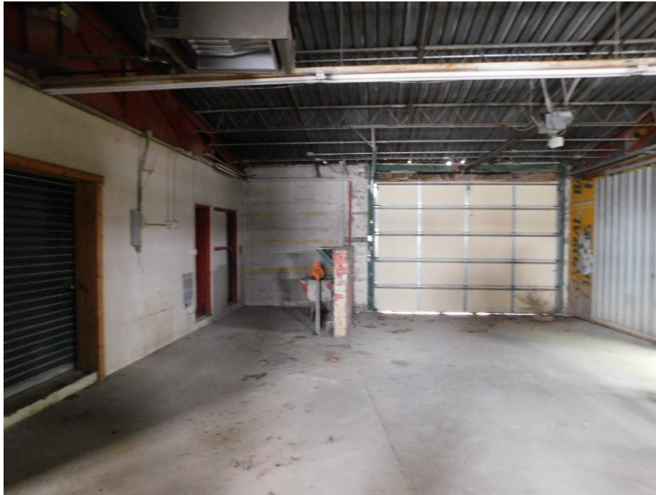
Figure 11: Interior view of rear elevation door.
