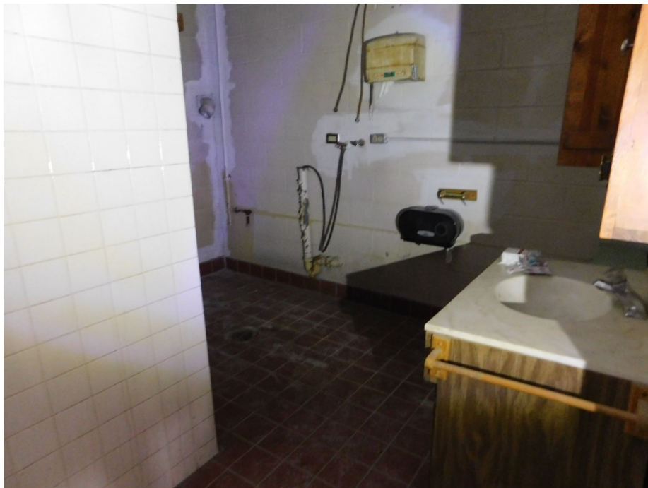
Figure 14: Bathroom off the carpentry room.
