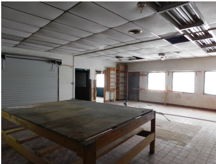
Figure 16: Carpentry room, looking toward office.
