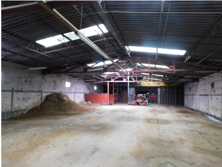
Figure 9: Paddock area looking toward carpentry room.
