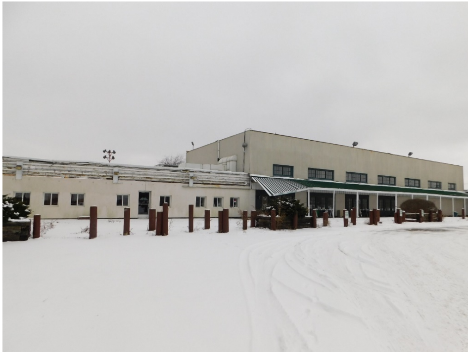
Figure 3: North elevation looking southwest.
