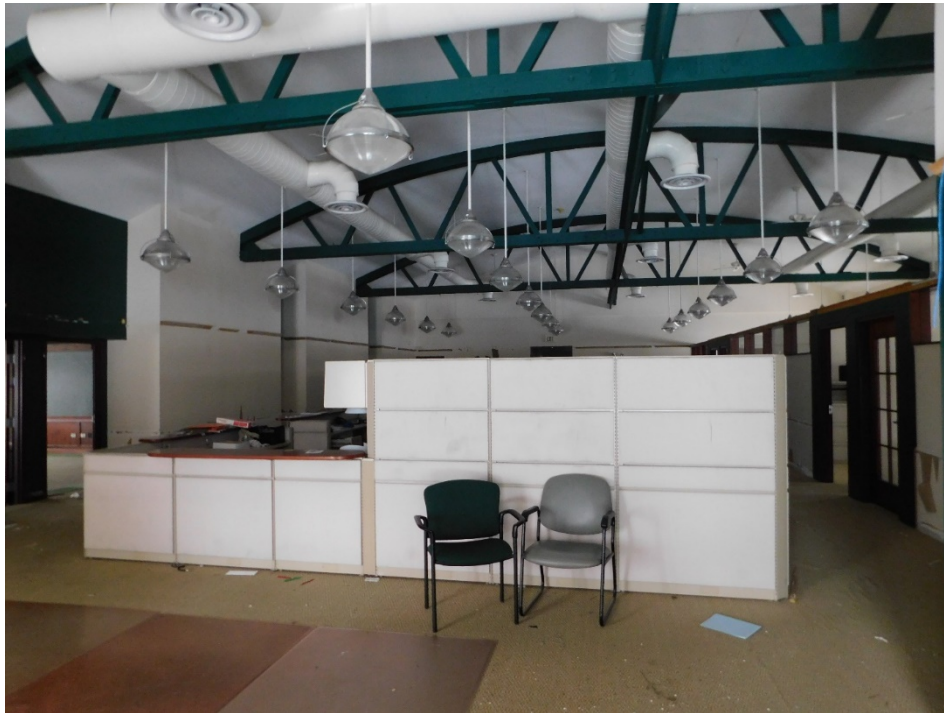
Figure 9: Second floor space with trussed ceiling.
