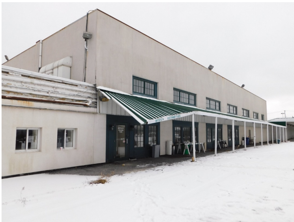
Figure 4: Close-up view of two-story main block's north elevation.
