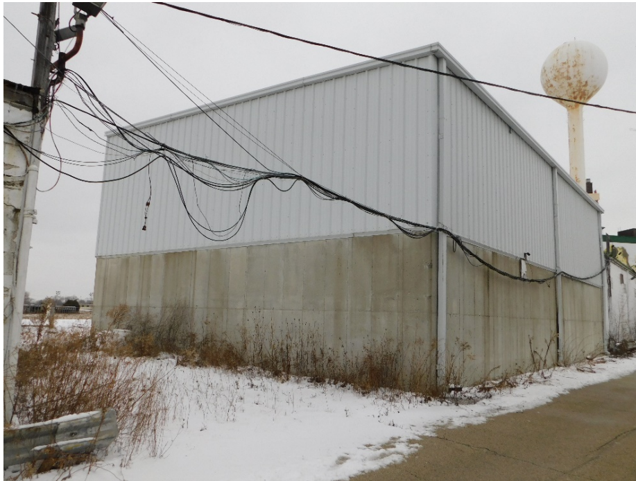
Figure 5: View of the site and rear elevations, looking northwest.
