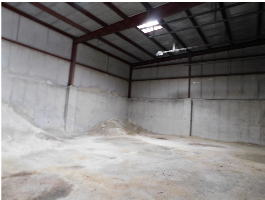
Figure 6: Interior of Materials Storage Building.
