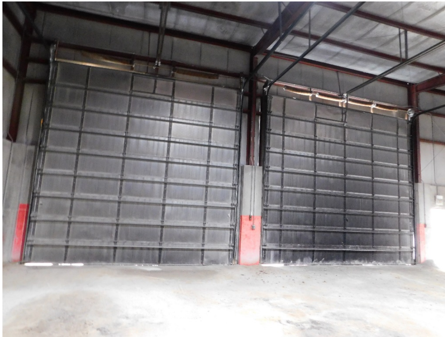
Figure 7: Interior view of overhead doors.
