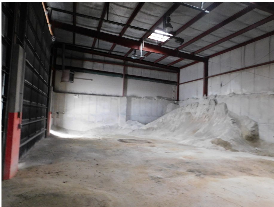
Figure 8: Interior view of Materials Storage Building.
