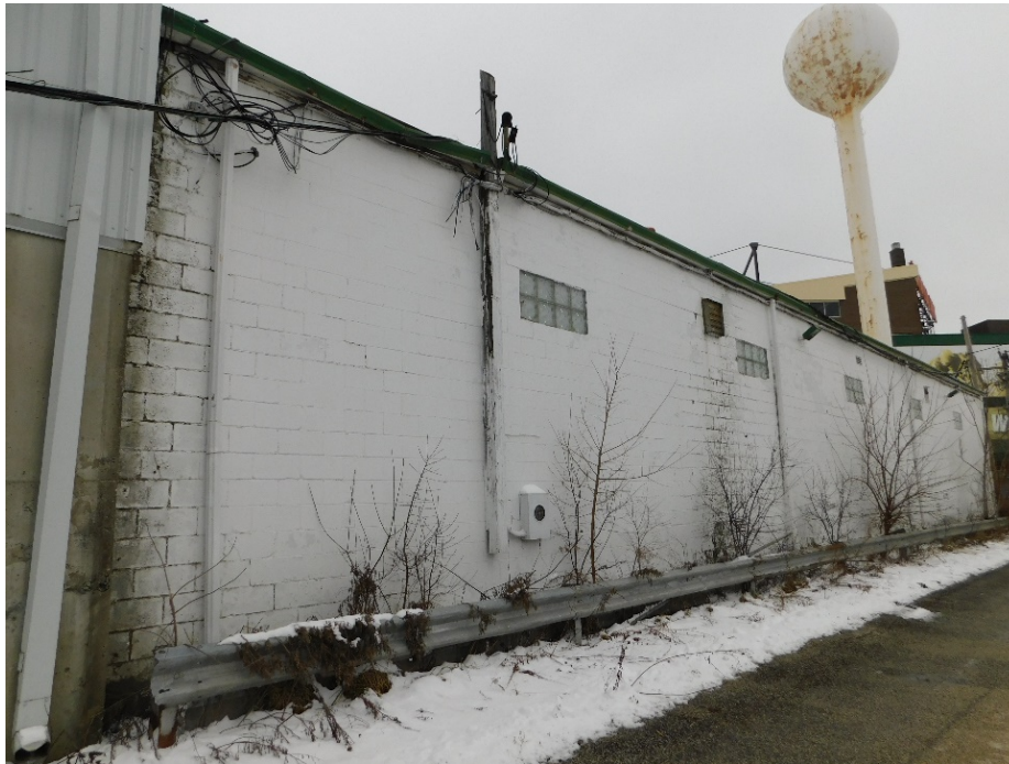
Figure 7: View of rear elevation looking northwest.
