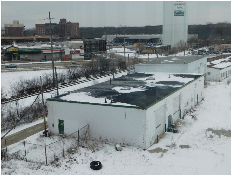
Figure 3: View of building from upper level Grandstand seating.
