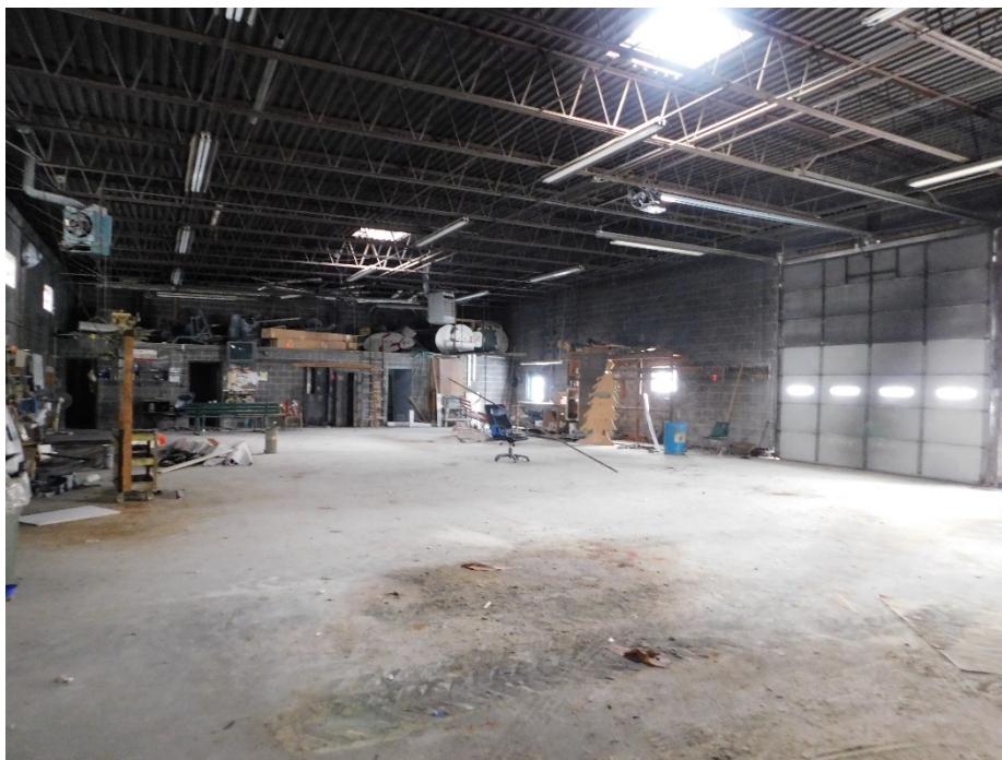
Figure 8: Primary equipment storage space.
