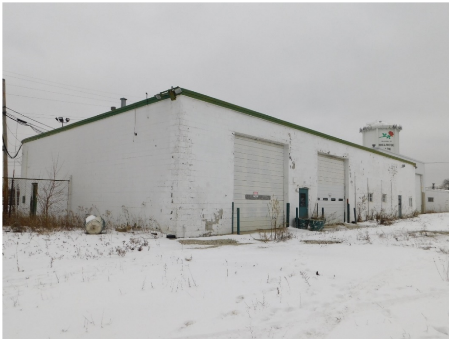
Figure 4: View of front and side elevations looking east.
