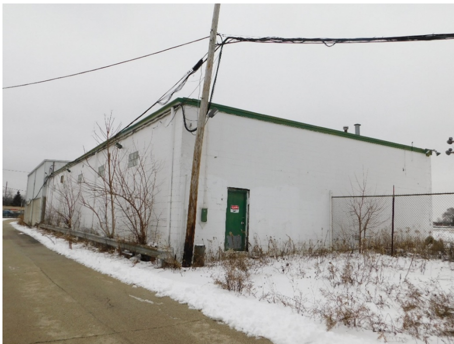
Figure 6: View of rear and side elevations, looking southeast.
