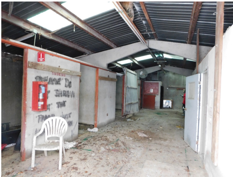
Figure 6: Barn interior, view looking southeast.
