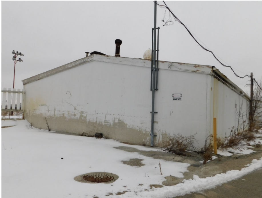
Figure 5: South and east elevations of barn.
