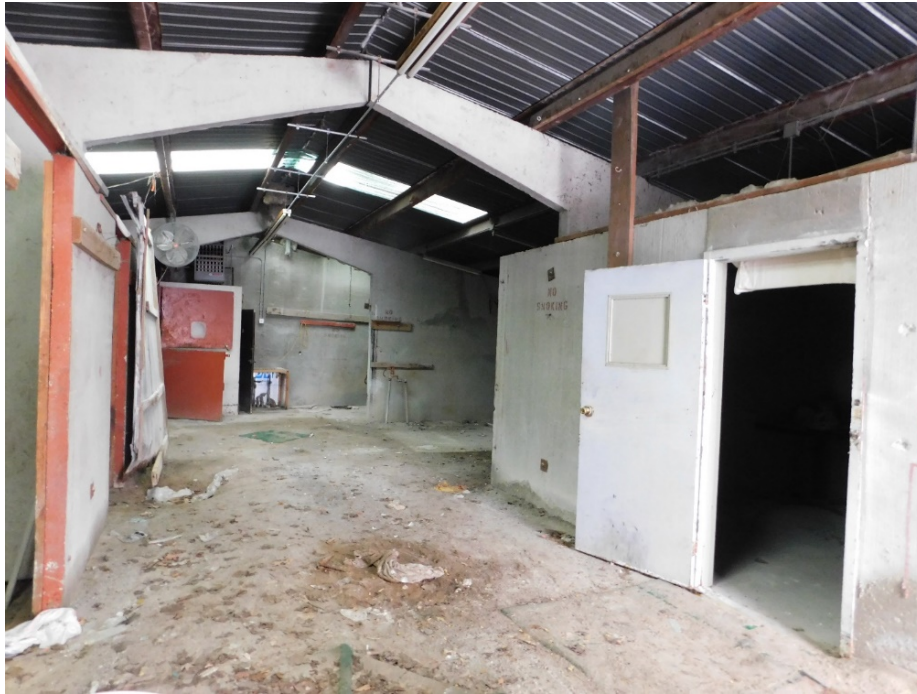
Figure 7: Barn interior showing door to offices in northwest corner.
