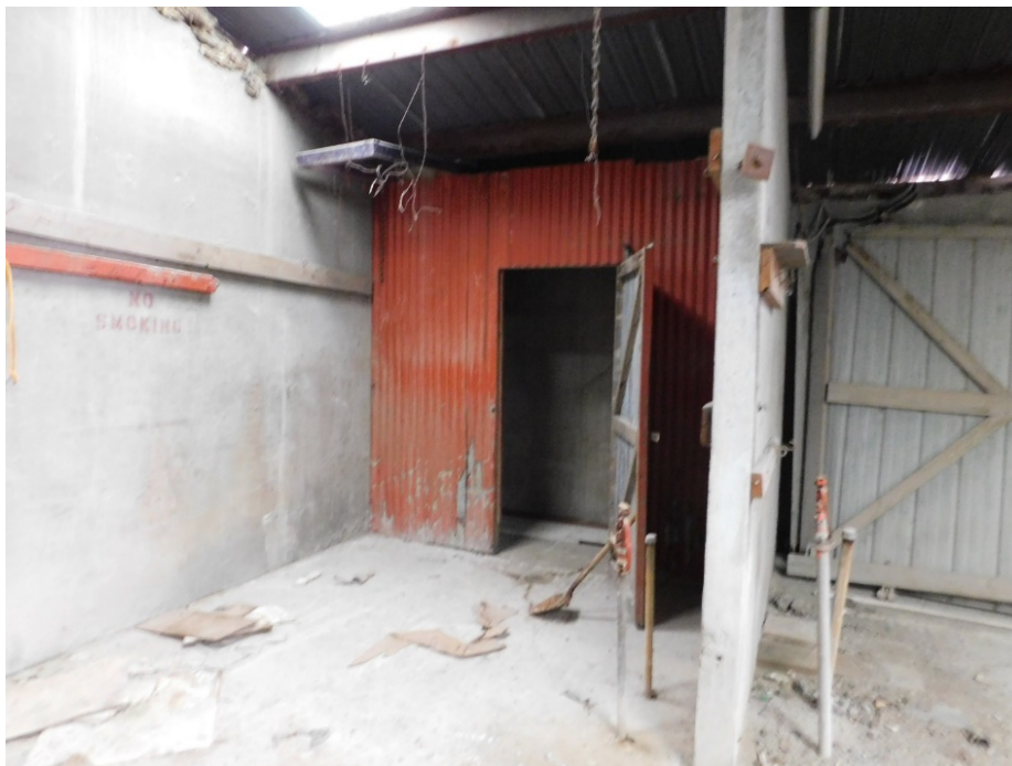
Figure 10: Storage area at southwest corner of barn.
