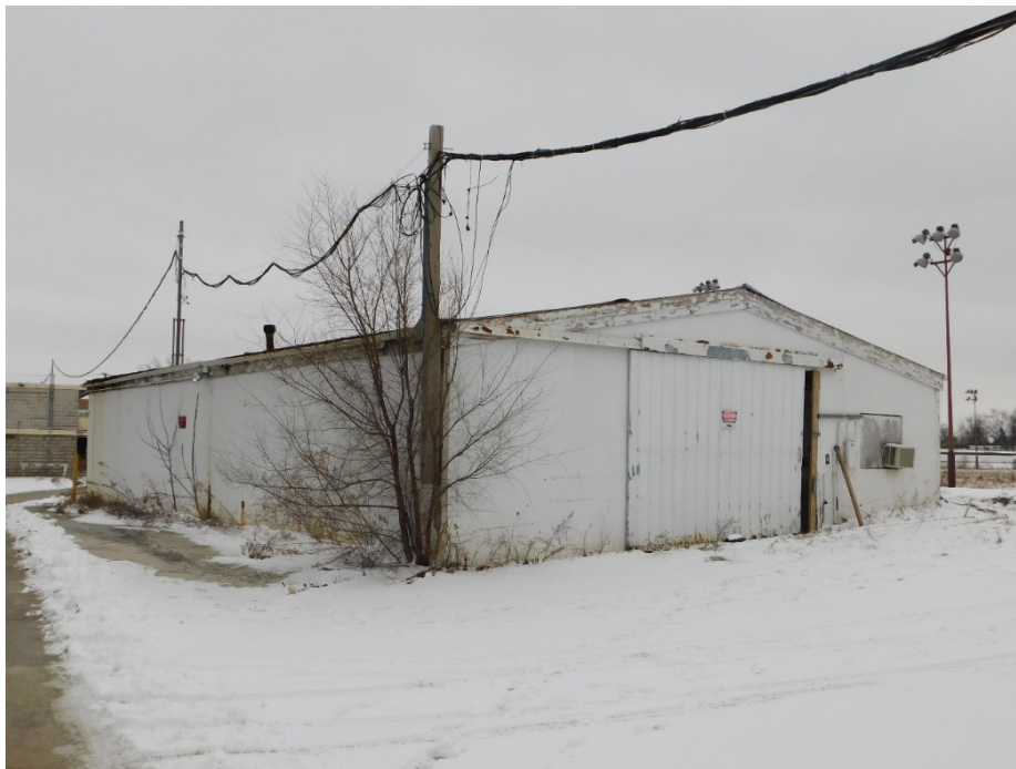
Figure 4: Main entrance on north elevation, looking southwest.
