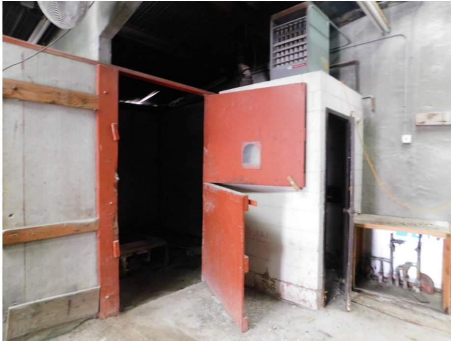
Figure 9: View of split door to horse stall and concrete block toilet stall.
