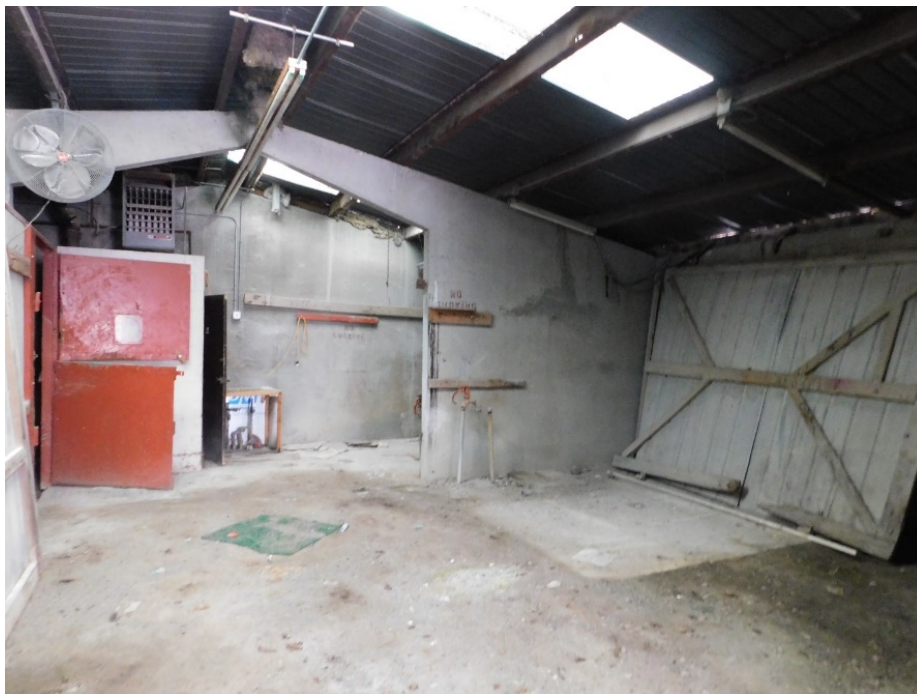
Figure 8: Barn interior, view looking southwest.
