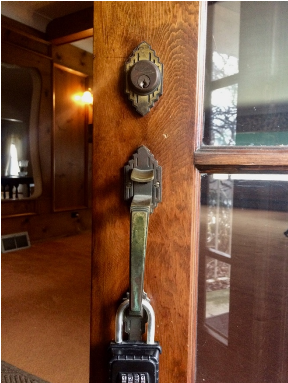
Hardware on 1953 north entrance door
