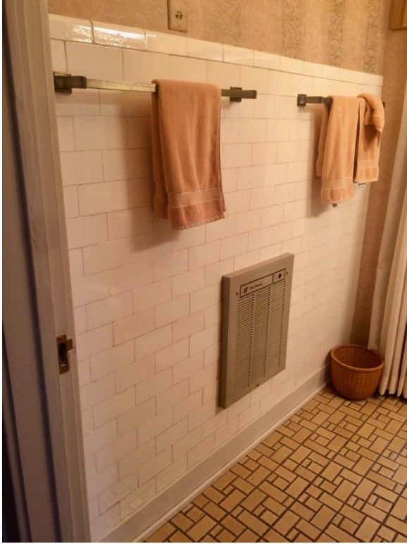
Original 1926 wall tile in bathroom
