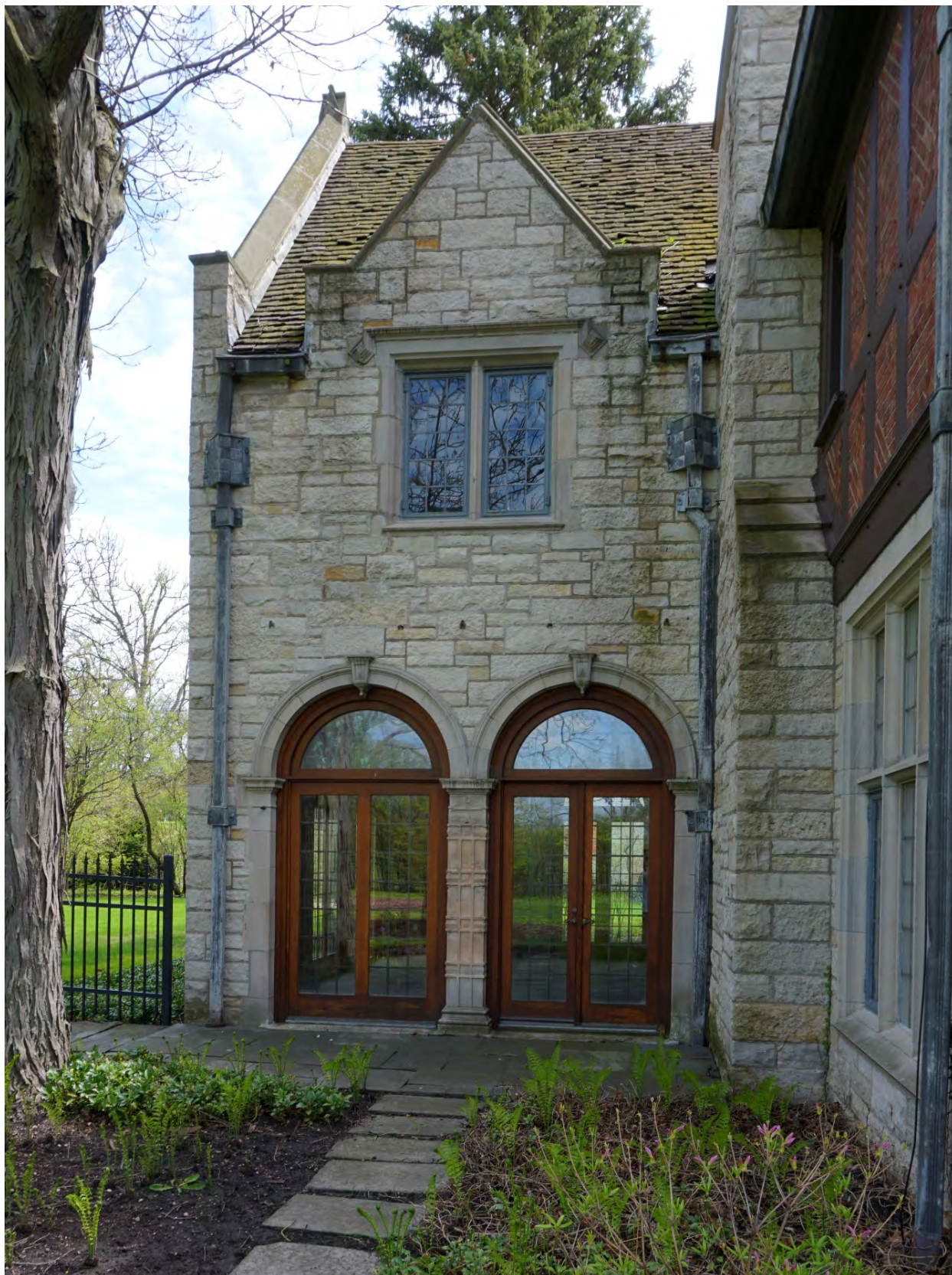
Photograph 13: Detail view of the west façade at the northwest corner looking east.
