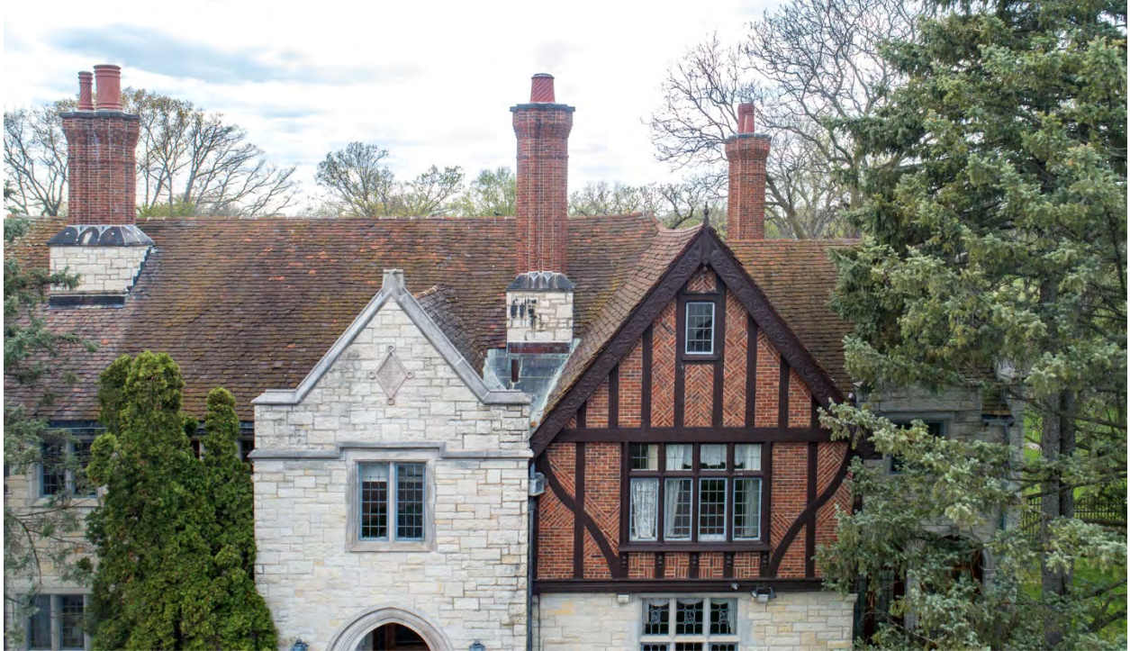
Photograph 4: Aerial detail view of the original roofline and details at the north end of the front (east) façade of the original residence, looking west.
