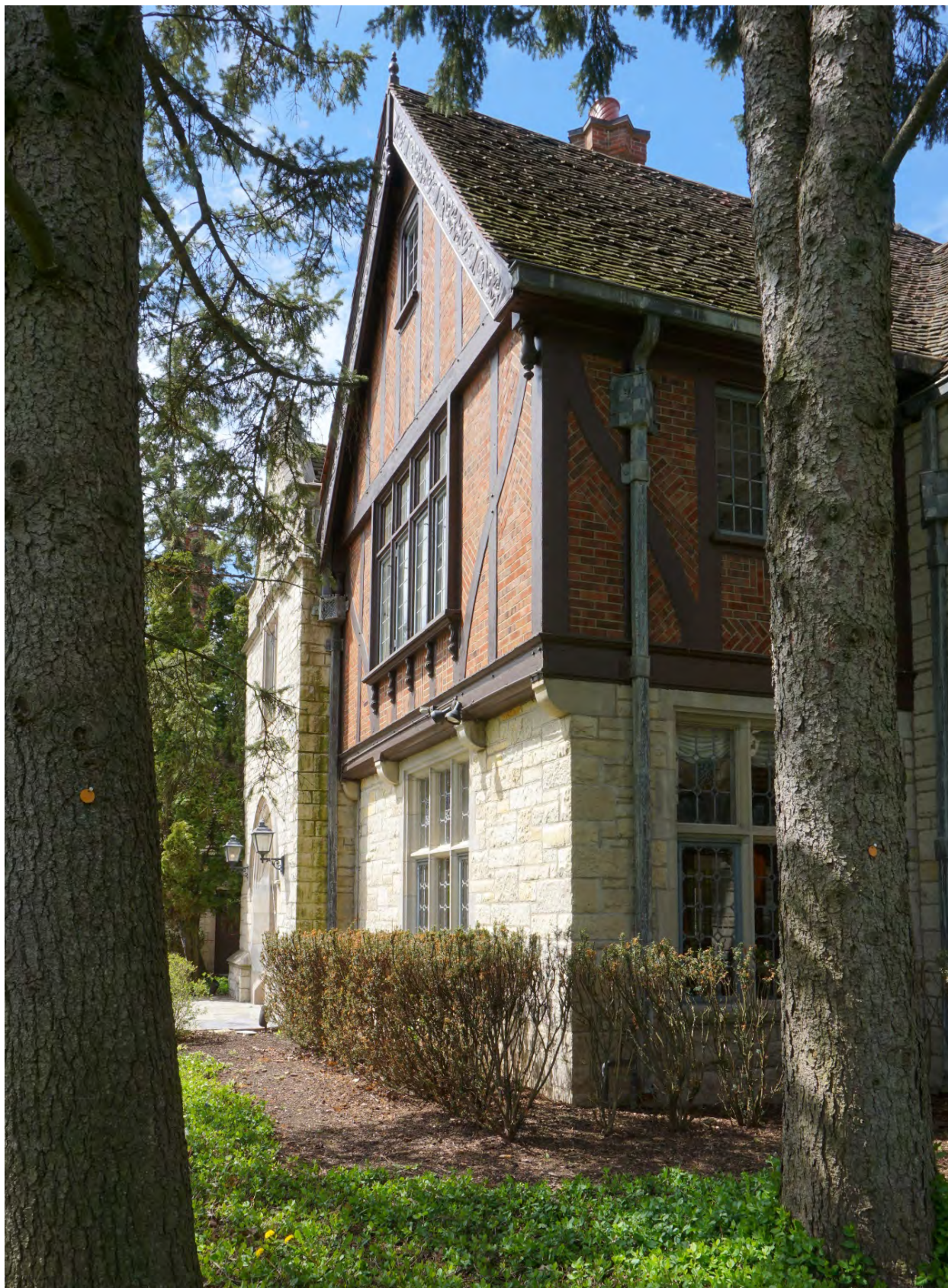
Photograph 10: Detail view of the north end of the front (east) façade looking southwest.
