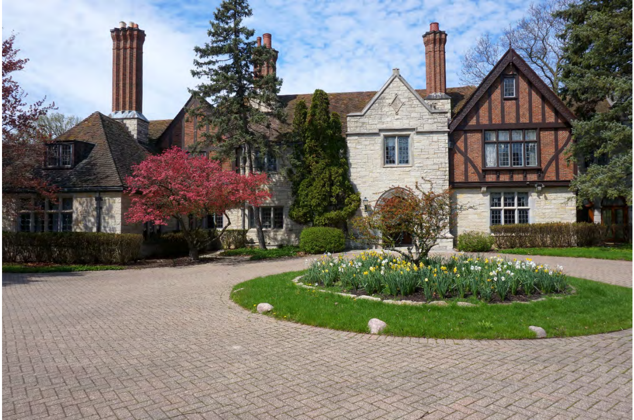
Photograph 2: View of the front (east) façade looking west.
