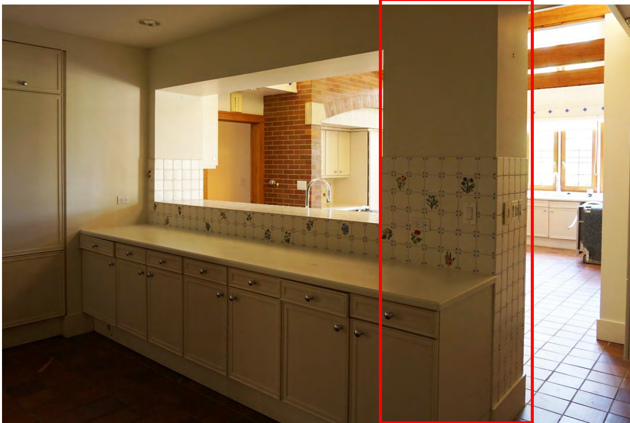
Photograph 50: View of the east end of the non-historic kitchen (remodeled c. 1990) located in the original residence. The footprint of the original residence returned east from the southwest corner. The thick wall denoted by the red bounding box is an original exterior wall that has been enclosed.
