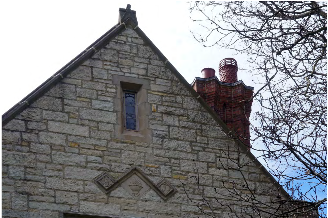
Photograph 11: Detail view of the limestone parapet at the north façade.
