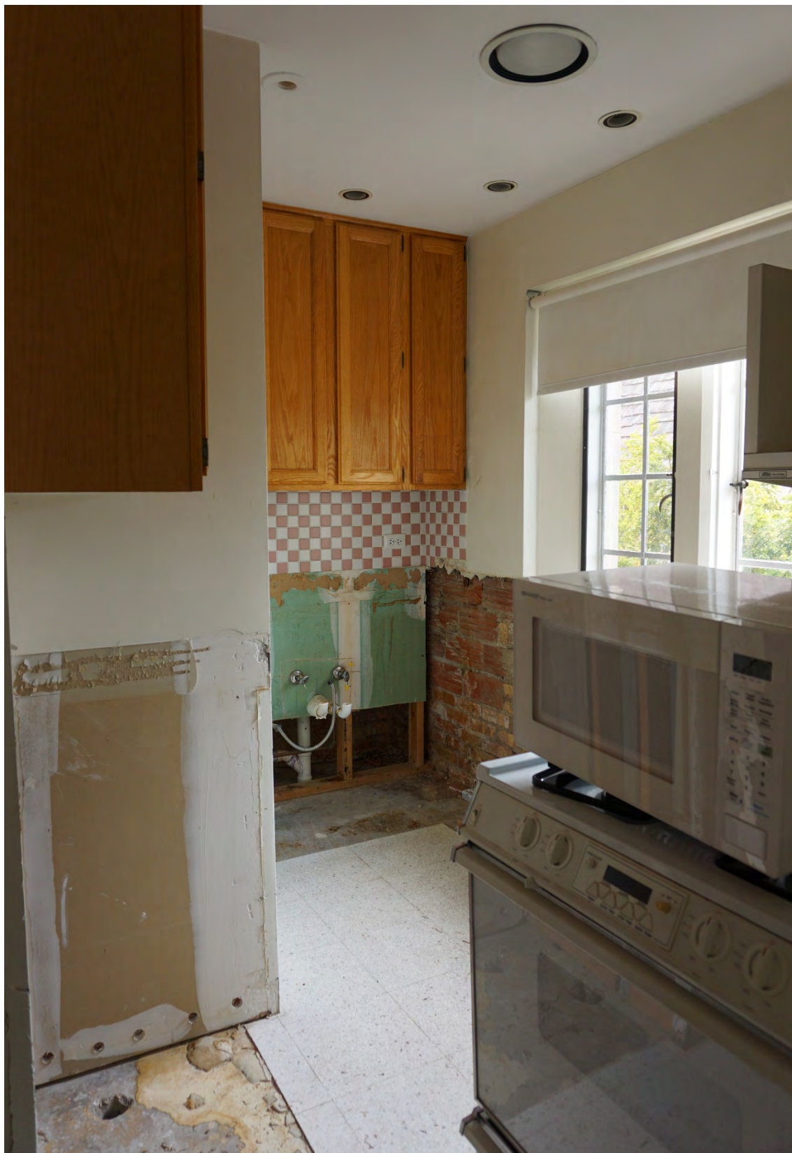
Photograph 70: View of the kitchen in the northwest corner of the second floor plan of the original coach house.
