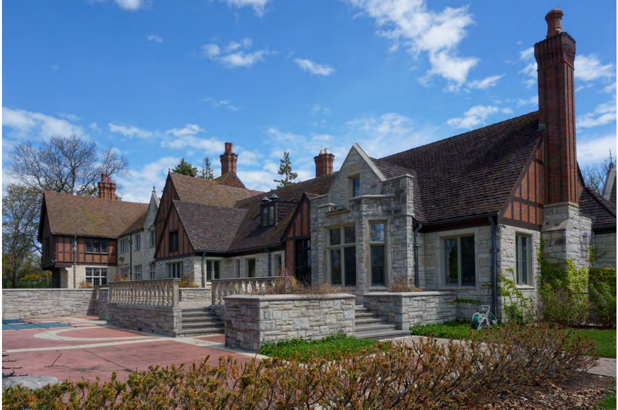
Photograph 21: Overall view of the south end of the rear (west) façade looking northeast.
