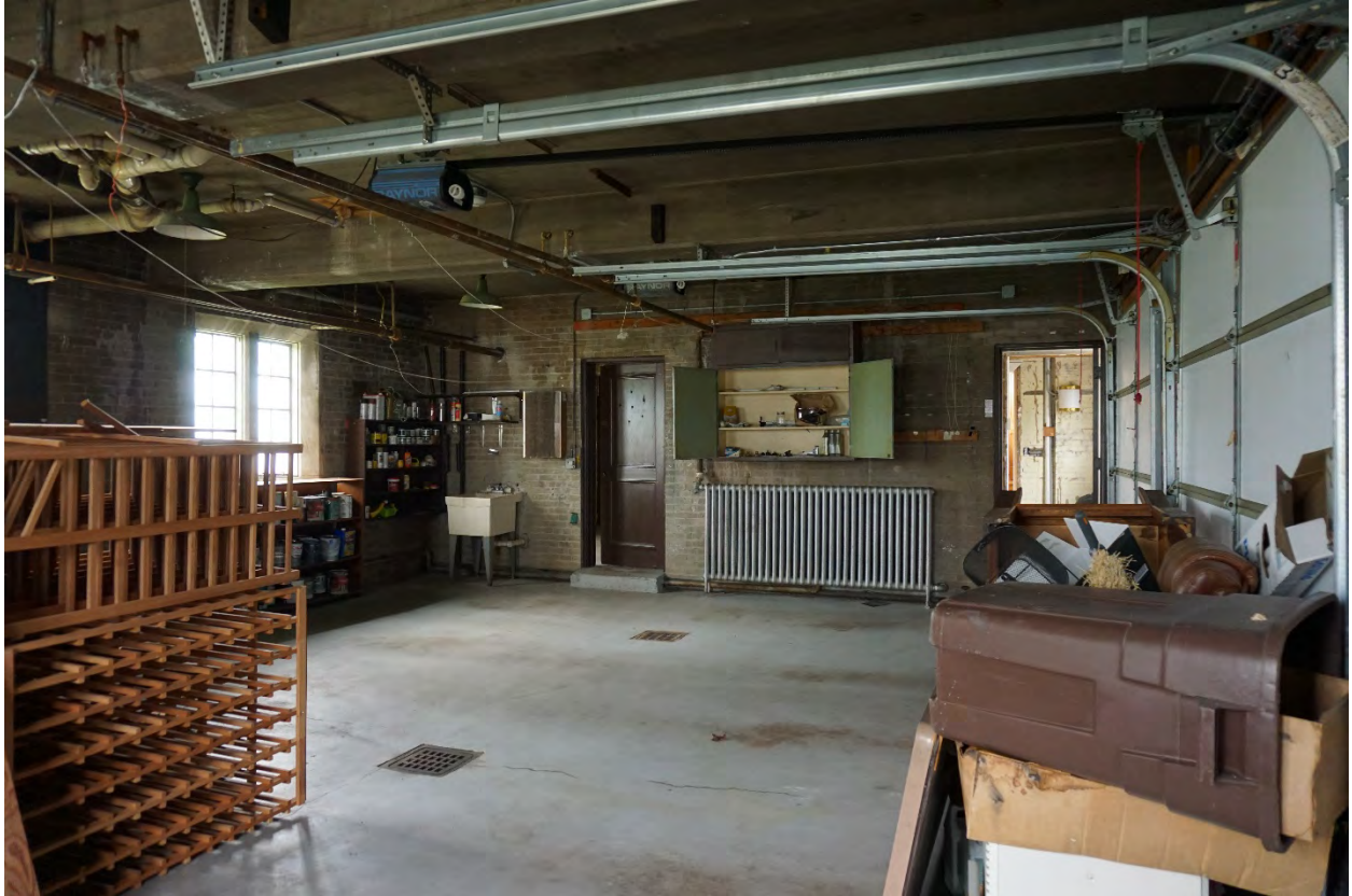
Photograph 68: View of the primary garage space at the east end of the original coach house looking west from the northeast corner of the space.
