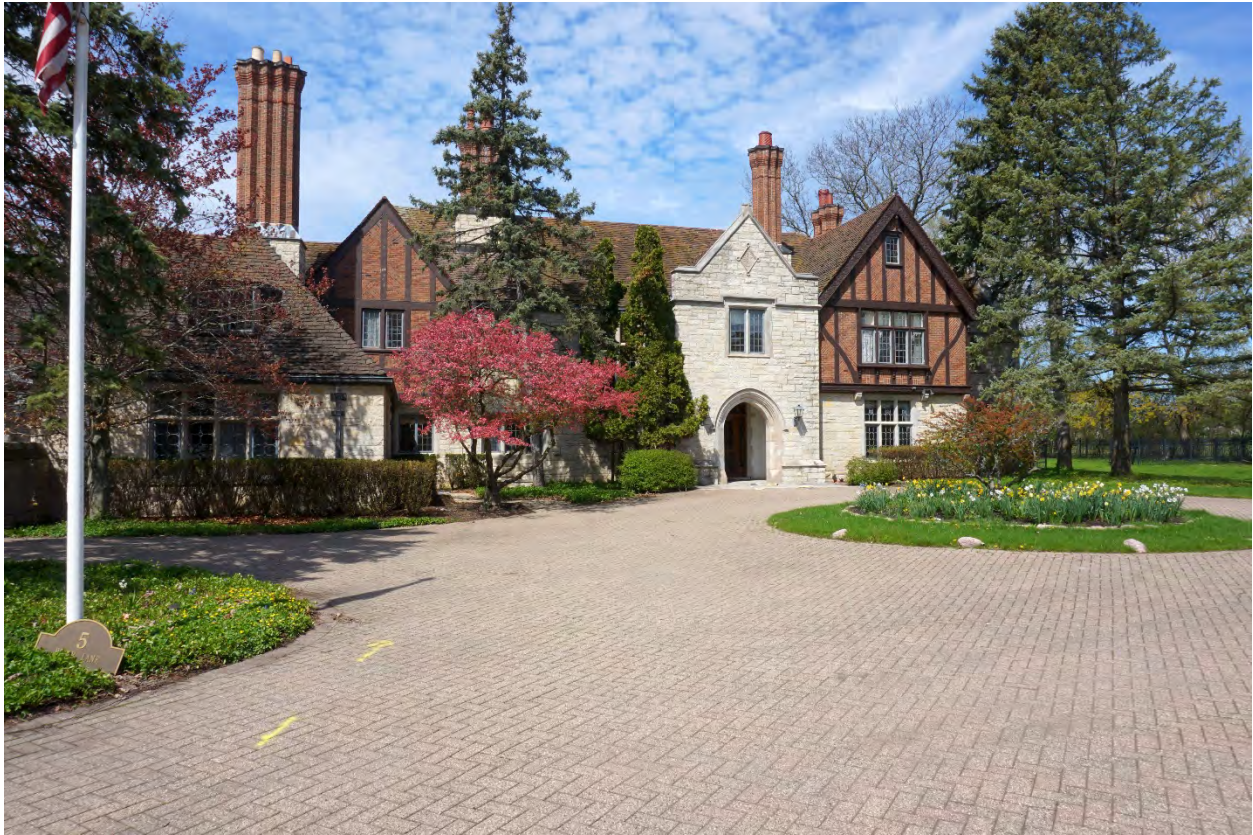
Photograph 1: View of the front (east) façade looking northwest.
