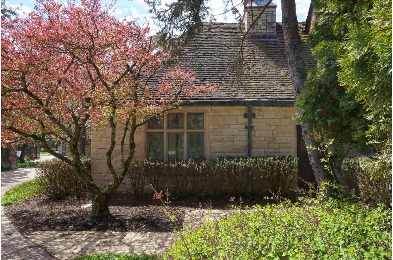
Photograph 31: View of the north façade at the south end of the original residence looking south.
