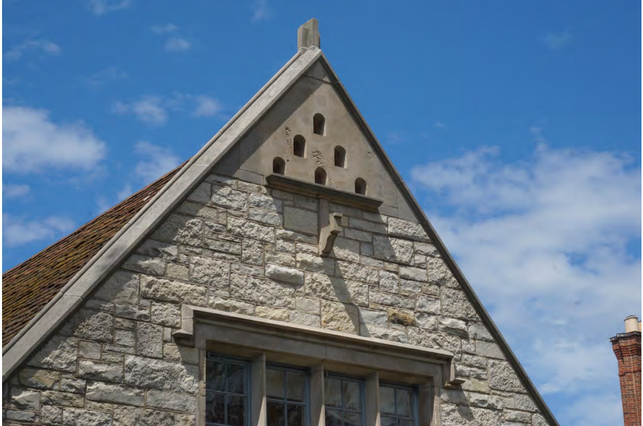
Photograph 25: Detail view of the limestone details at the east façade of the original coach house.
