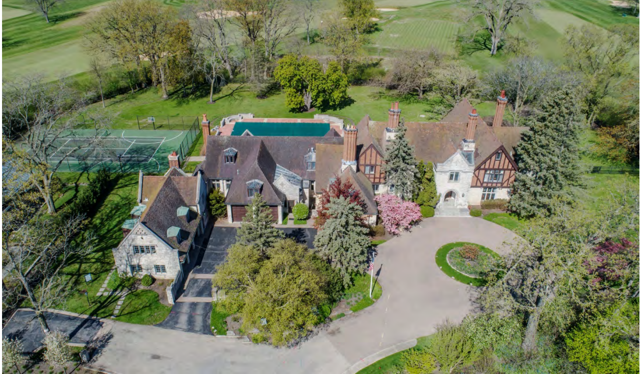
Photograph 2: Aerial perspective view of the site, with the original residence (right), addition (center), and original coach house (left) visible, looking west.
