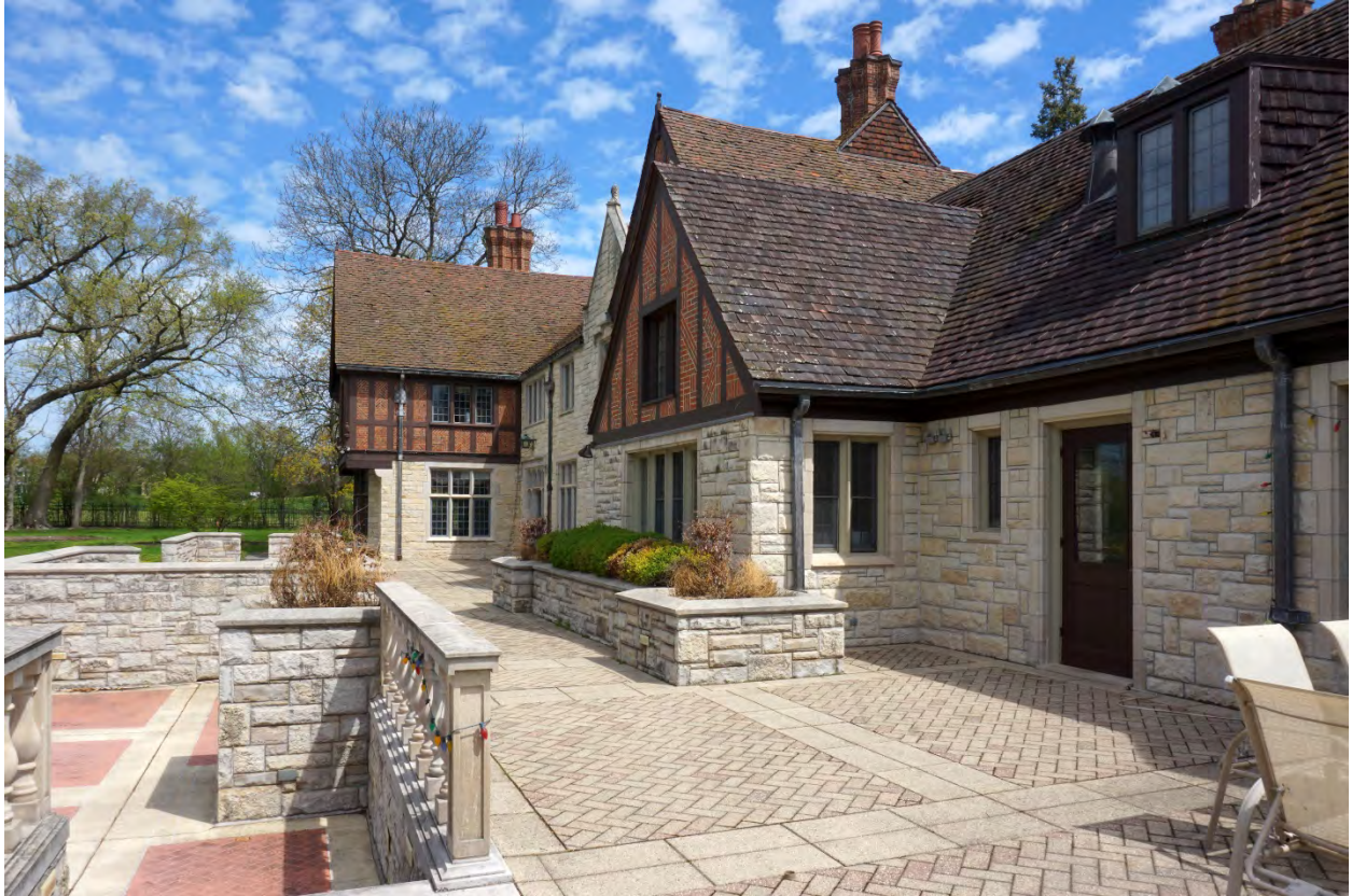
Photograph 17: Detail view of the mid-section of the rear (west) façade, where the original residence and addition meet, looking northeast.
