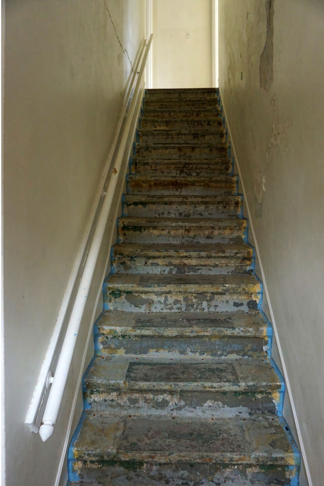
Photograph 66: View of the staircase in the original coach house.
