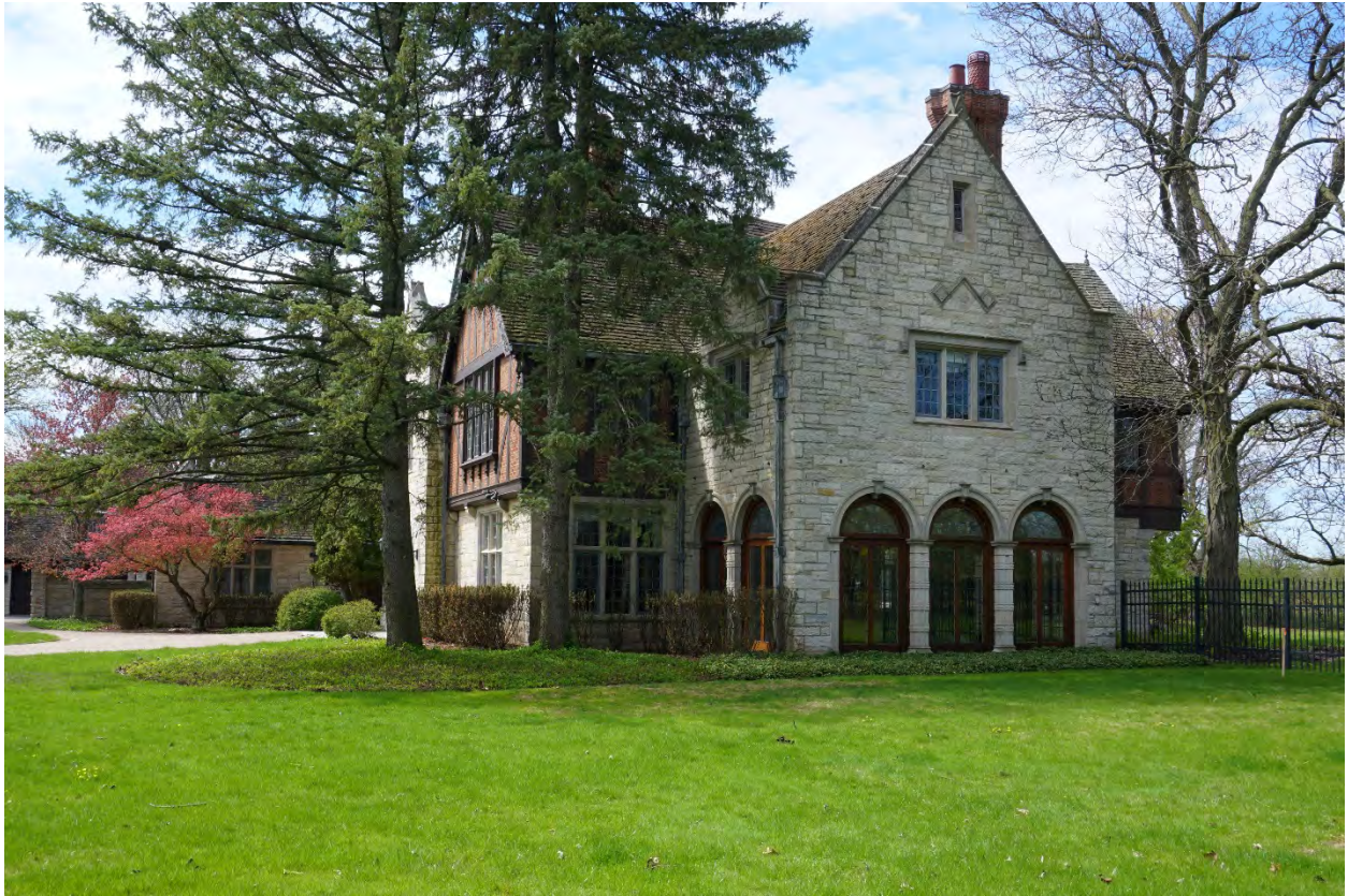
Photograph 8: View of the north façade looking southwest.
