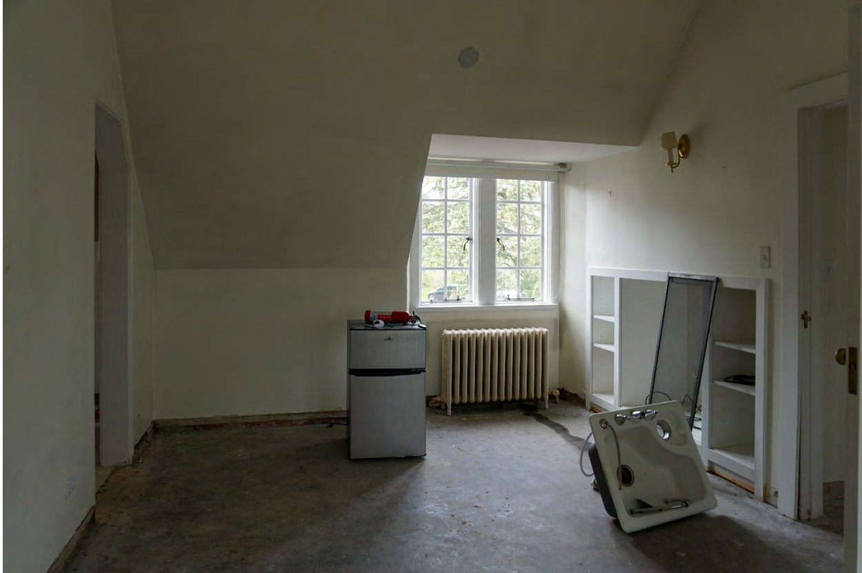
Photograph 69: View of the living room at the center of the second floor plan of the original coach house.
