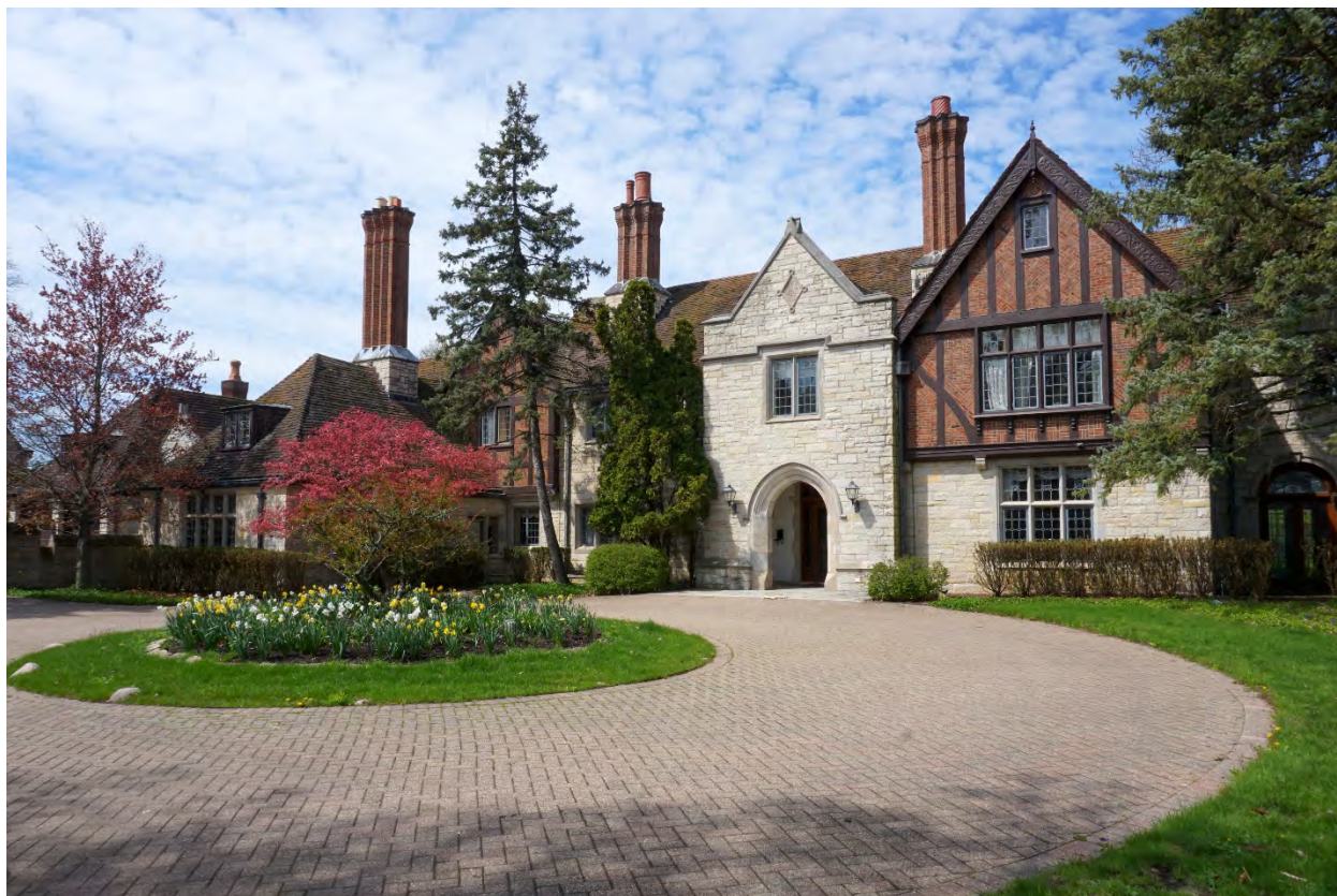
Photograph 4: View of the front (east) façade looking southwest.
