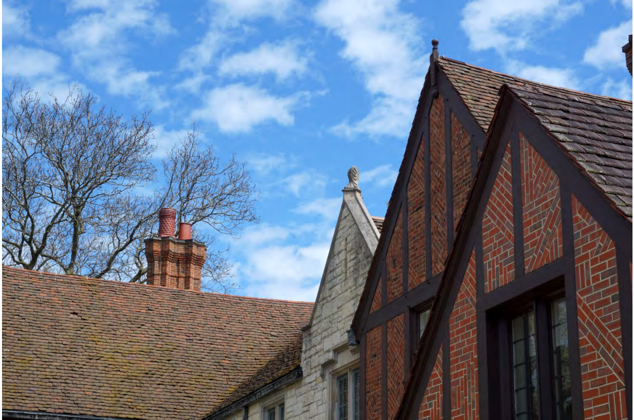
Photograph 16: Detail view of the parapet details at the north end of the rear (west) façade.
