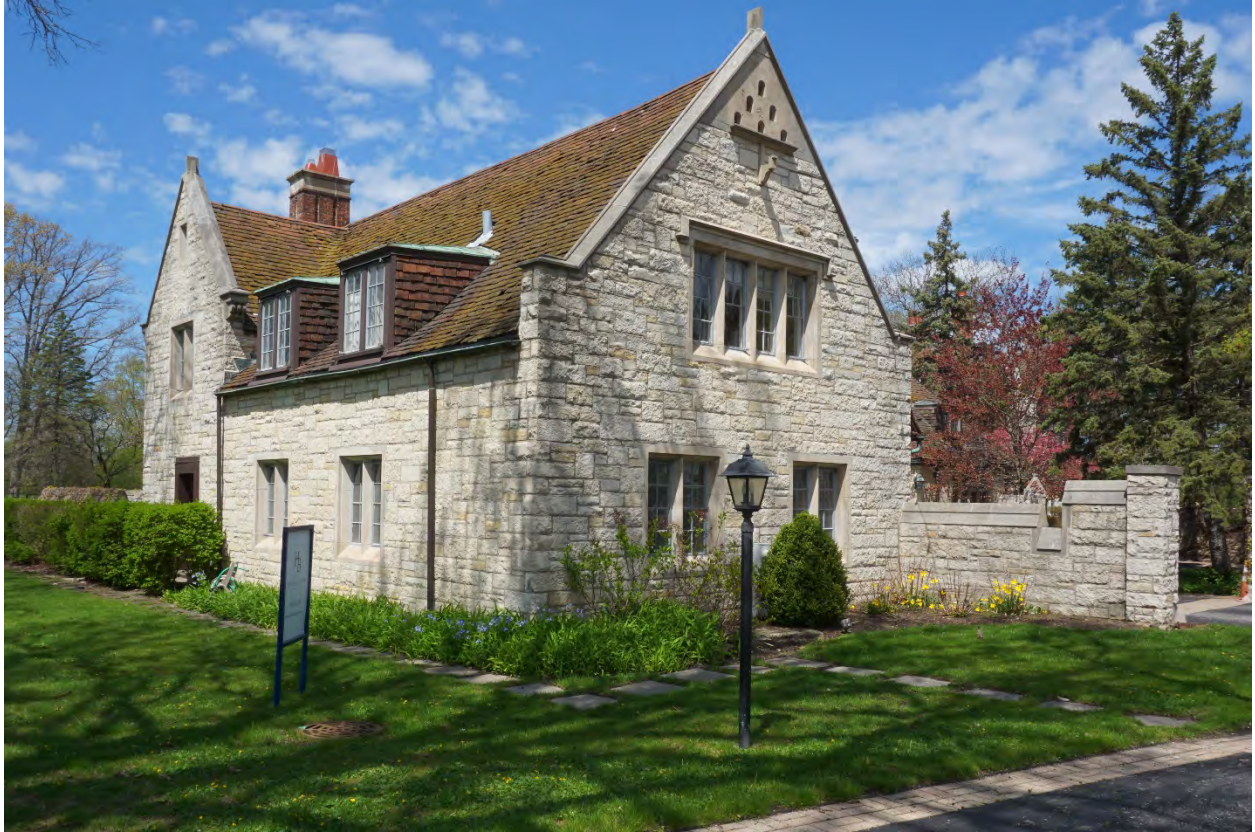
Photograph 24: View of the south and east façades of the original coach house looking northwest.
