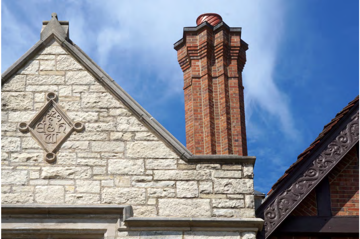
Photograph 5: Detail of the limestone parapet above the front (east) entrance.
