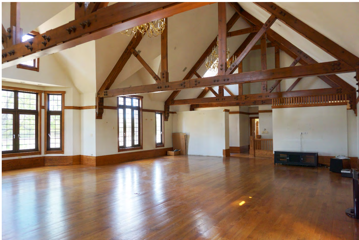
Photograph 54: View of the family room at the south end of the addition looking northwest from the southeast corner of the space.
