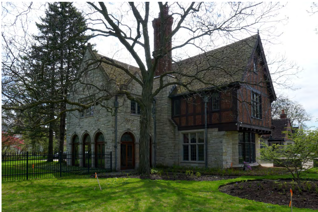
Photograph 12: View of the northwest façade looking southeast.
