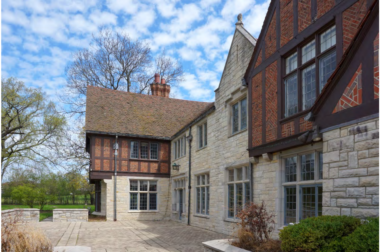
Photograph 15: Detail view of the rear (west) façade of the original residence looking northeast.
