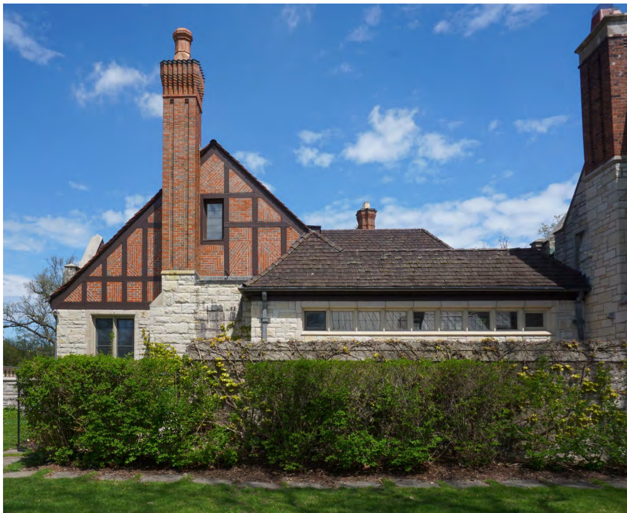
Photograph 22: Overall view of the south façade of the addition and connecting hyphen to the original coach house looking north.
