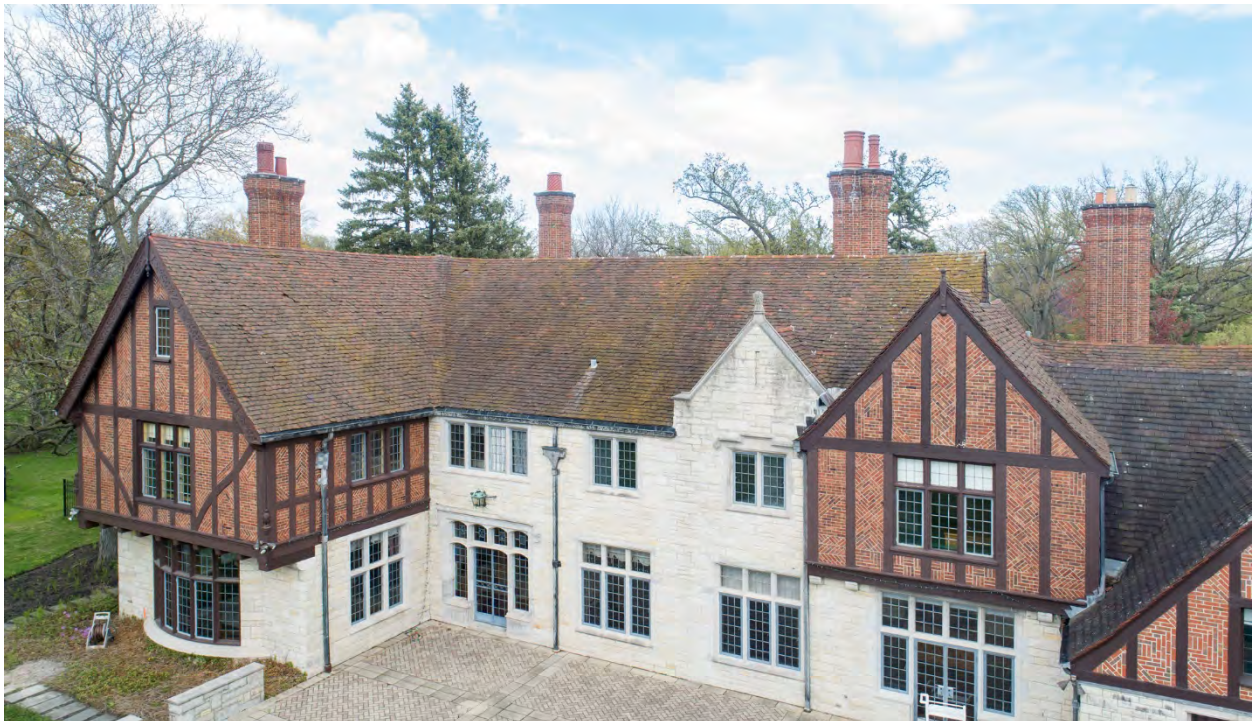
Photograph 5: Aerial detail view of the original roofline and details at the north end of the rear (west) façade of the original residence, looking northeast.
