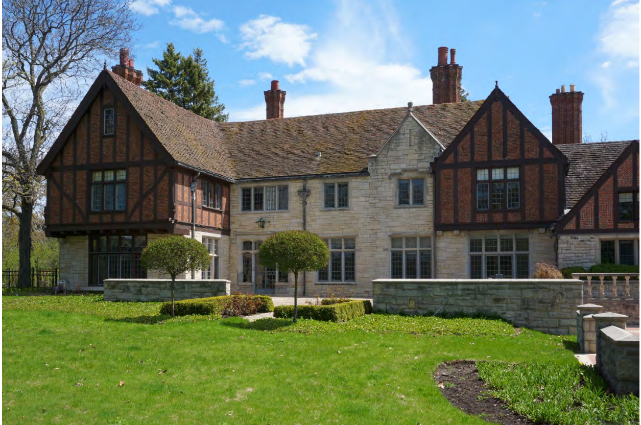
Photographs 19: Overall view of the rear (west) façade of the original residence looking east.
