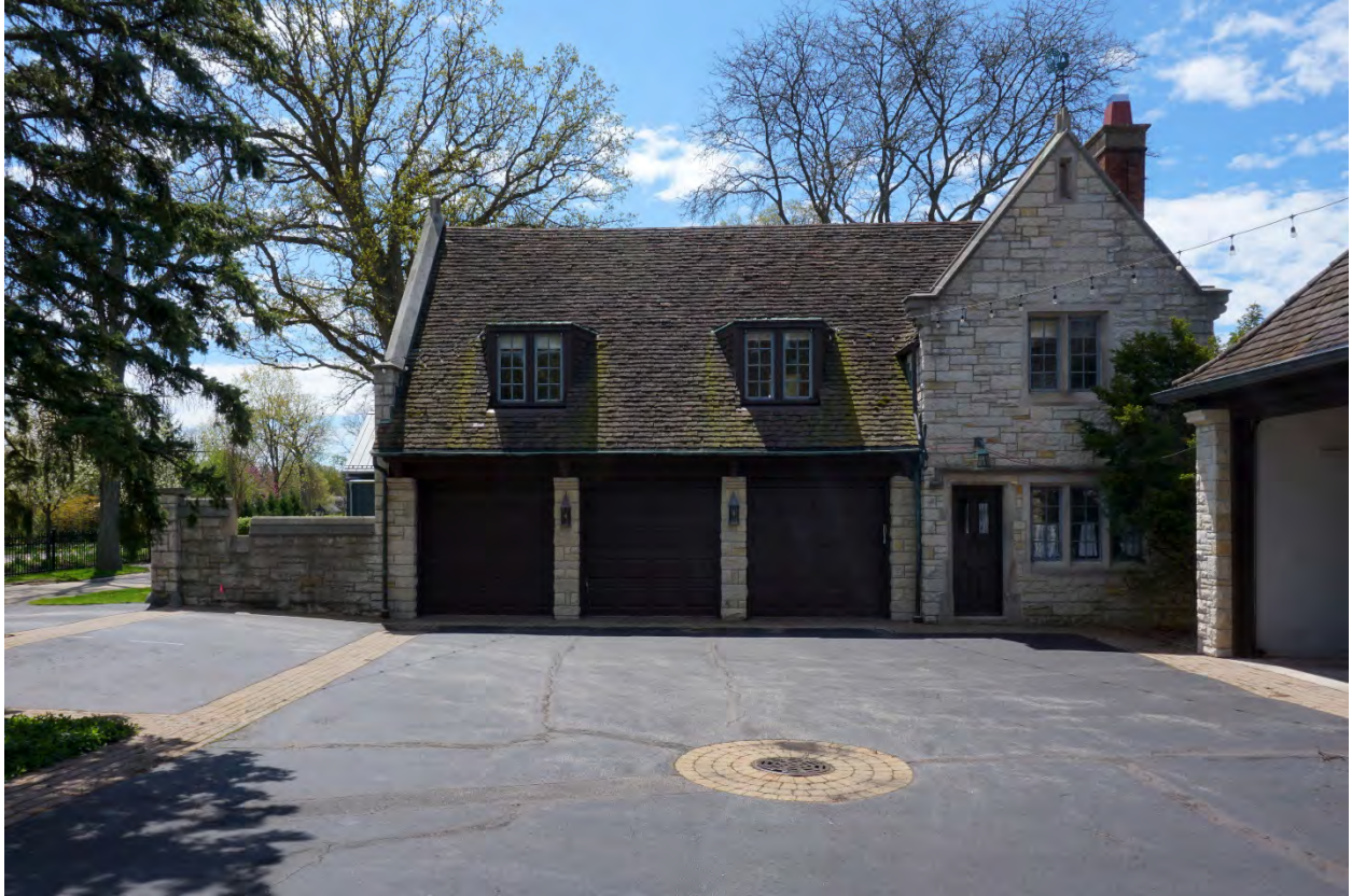
Photograph 27: View of the north façade of the original coach house looking south.
