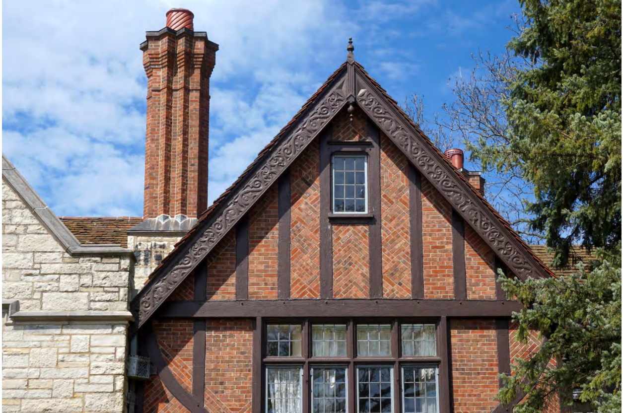
Photograph 6: Detail view of the brick detailing and carved bargeboard at the north end of the front (east) façade.
