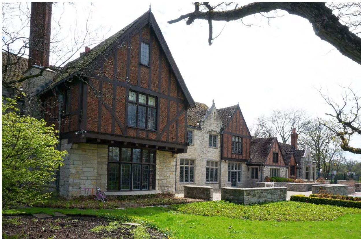
Photograph 14: Overall view of the rear (west) façade looking southeast.
