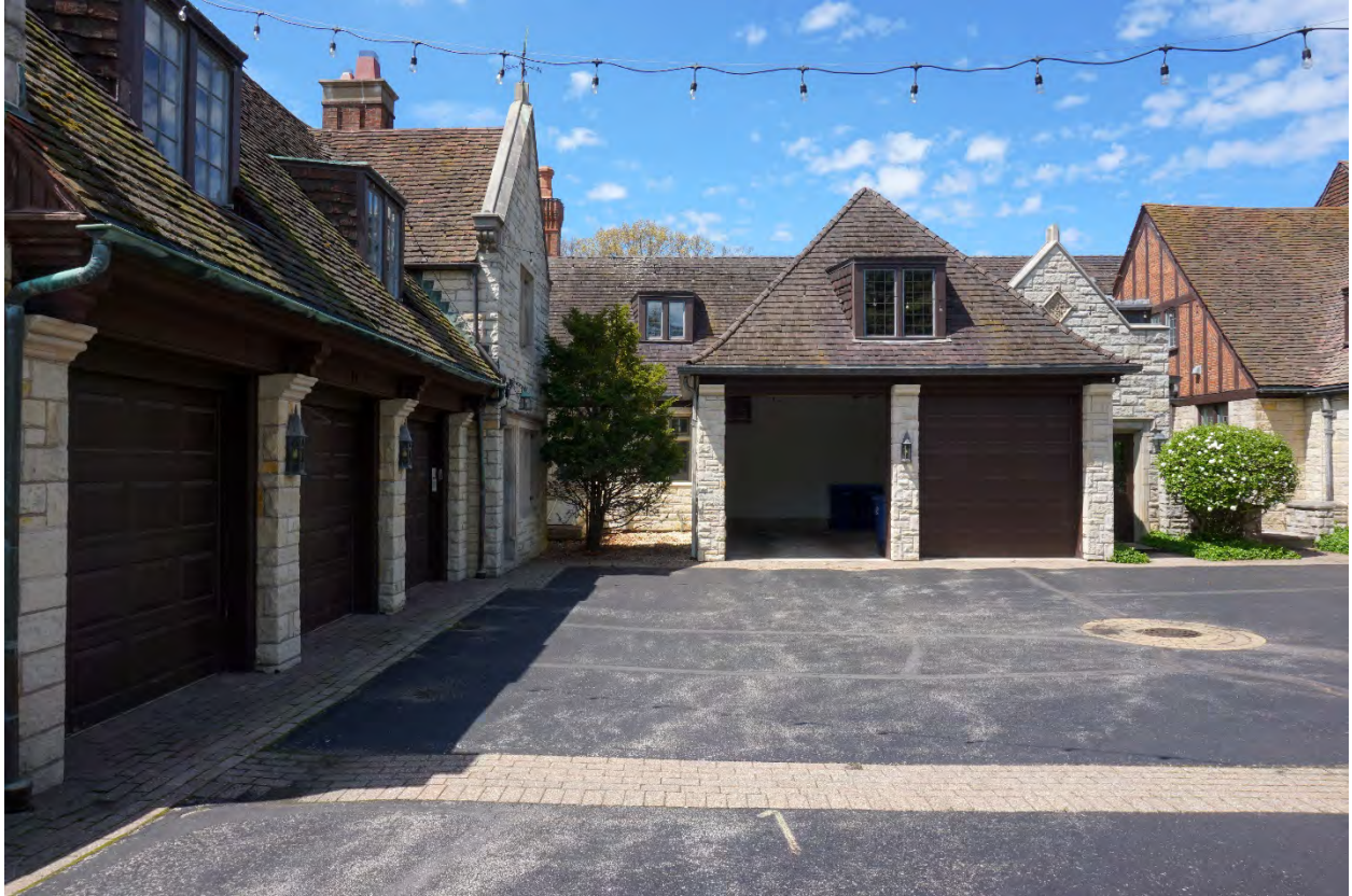
Photograph 28: View of the east façade of the addition (right) and the north façade of the original coach house (left) looking west.
