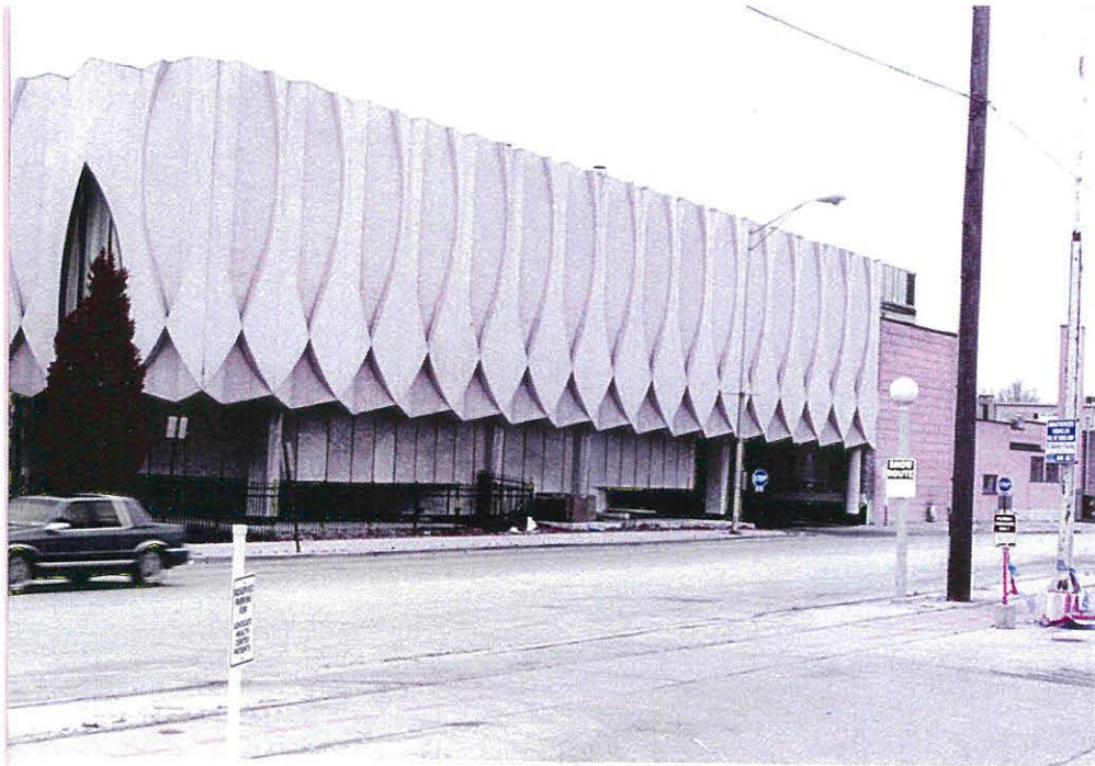
Figure 18. Sky Room addition (Structure B) concrete and gravel panels. The view is to the south.
