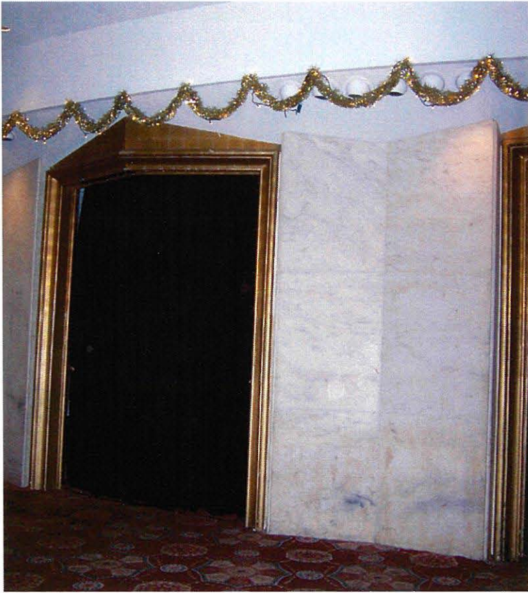
Figure 12. Marble panels of interior walls.
