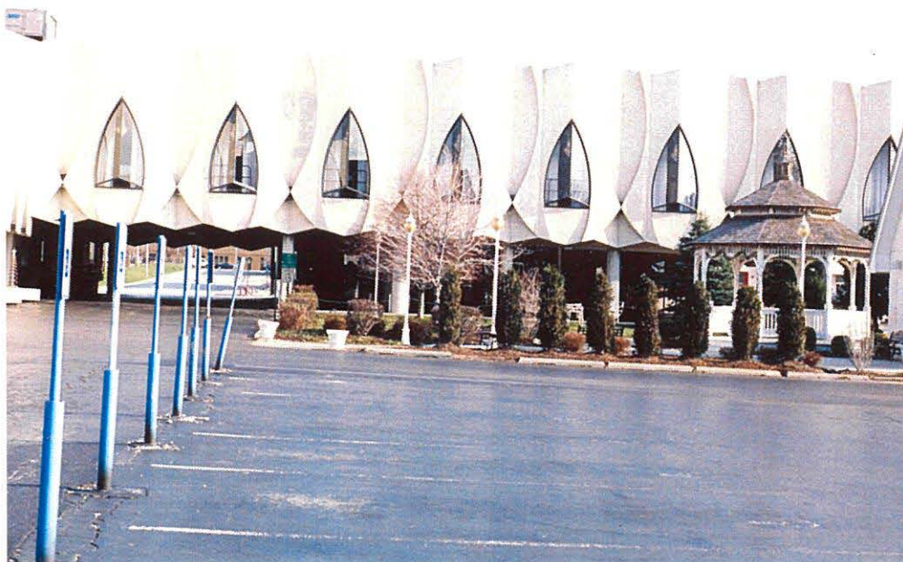
Figure 19. Covered drive. The view is to the east.
