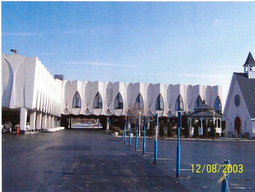
Figure 7. The Drury Lane Sky Room addition (Structure B). The view is to the east.
