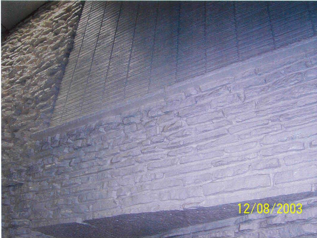
Figure 14. Tabular limestone walls.
