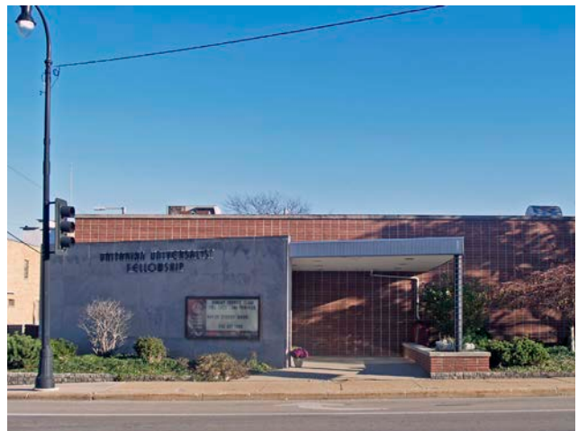
Mid-Century Vernacular/Mid-Century Modern examples: 317 East Locust Street (above); 158 North Fourth Street (below)
