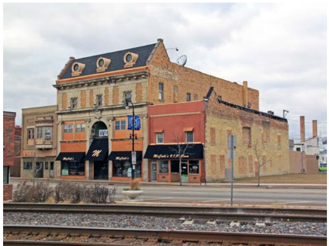
Classical Revival/Beaux Arts examples: 164 East Lincoln Highway (above); 323 East Lincoln Highway (below)
