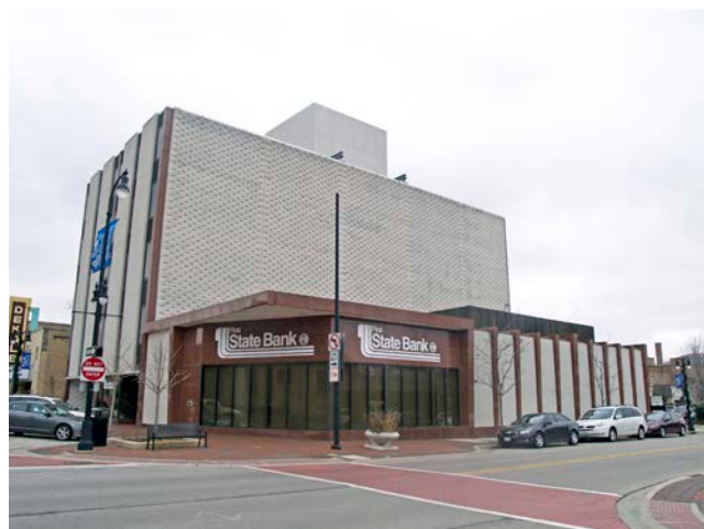
International Style examples: 126 Oak Street (above); 155 North Third Street (below)
