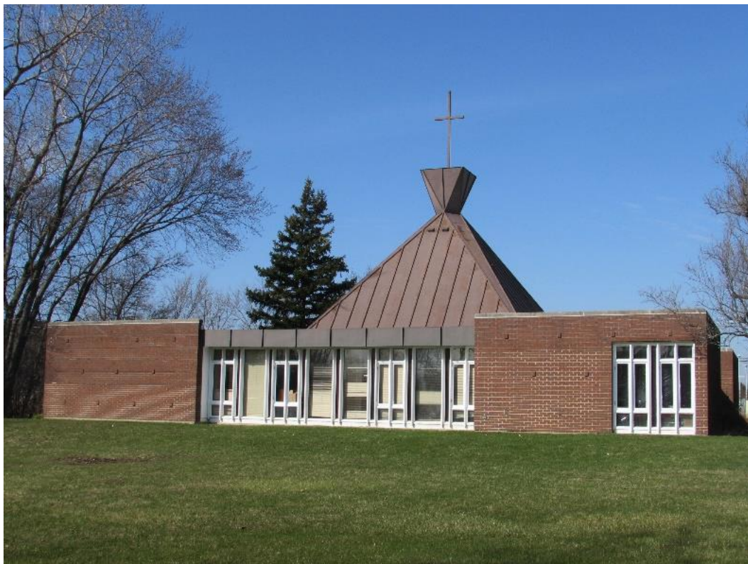
East elevation, looking southwest
