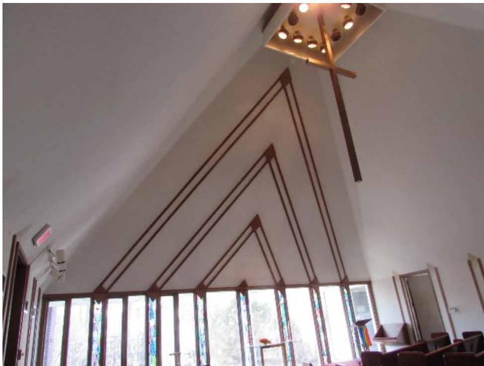
Nave looking southwest with ceiling cross
