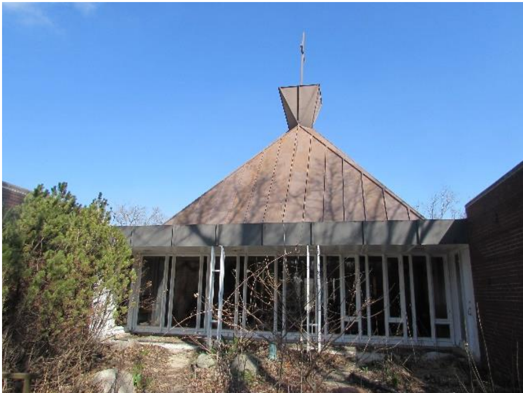
Rear (south) elevation, looking northwest
