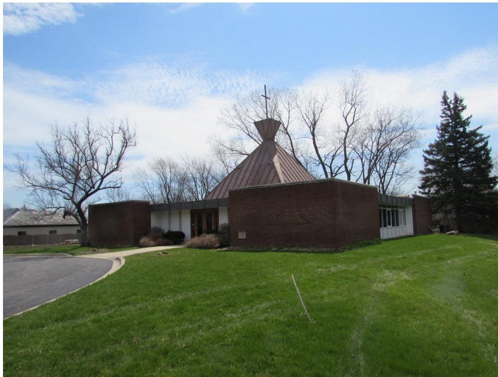
Front (north) and west elevation looking southeast
