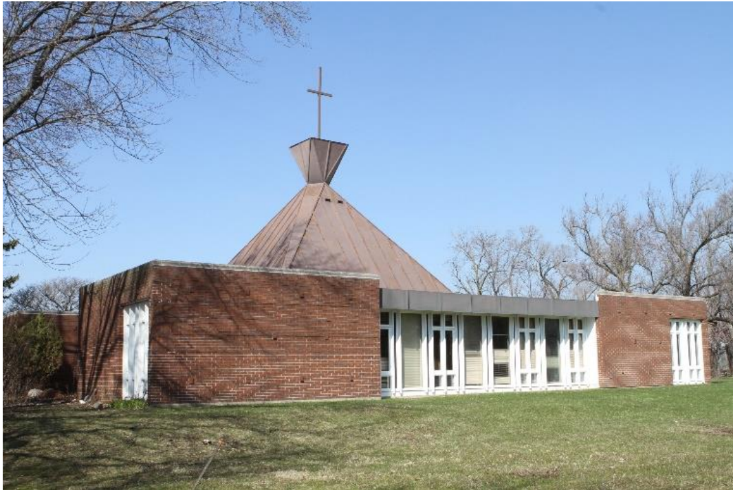
East elevation, looking northwest
