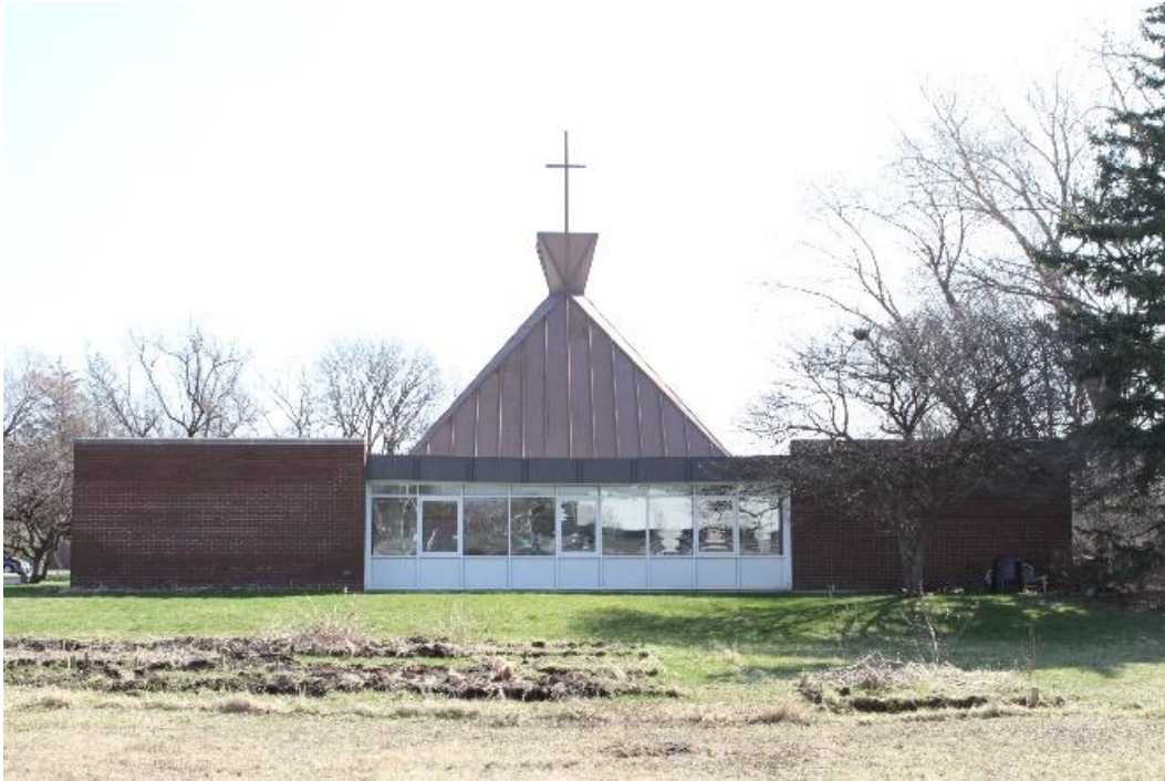
West elevation, looking east
