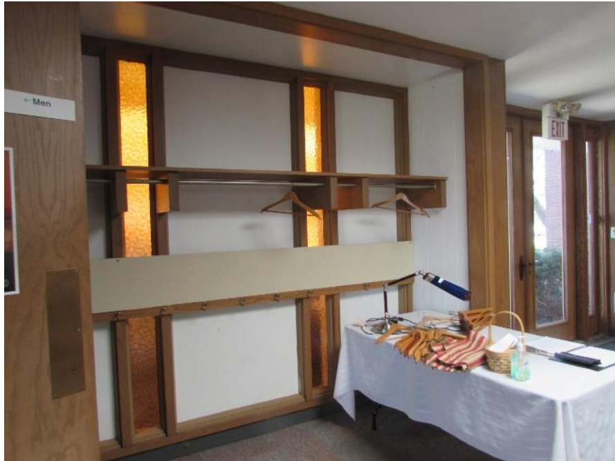
Narthex looking northeast showing original frosted glass windows.
