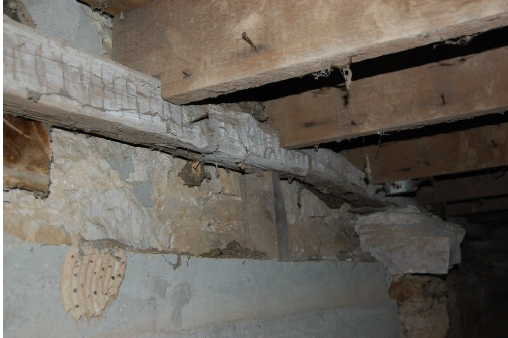
Figure 106. View of the sill plate on the east side of Room 001. The plate is hand-hewn oak and has mortises on its lower side, which suggests that it is reused stock salvaged from an unknown location. The existing joists are pine and were installed as part of the late-nineteenth-century rebuilding of the rear wing on the original house.
