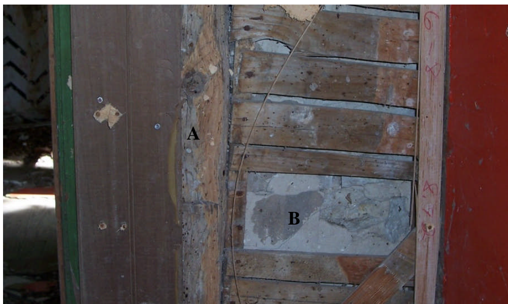
Figure 66. Detail of the southwest corner of Room 102C showing the junction of between the original rear wing and stone addition. “A” indicates the original southwest corner post of the rear wing. “B” marks the north end of the west wall of the stone addition, which originally extended just past the wall plain of the original frame wing and was plastered over. Late in the nineteenth century, the west wall of the frame wing was pushed outward to be even with the stone addition, and the formerly exposed end of stone wall was covered over with lath shown.
