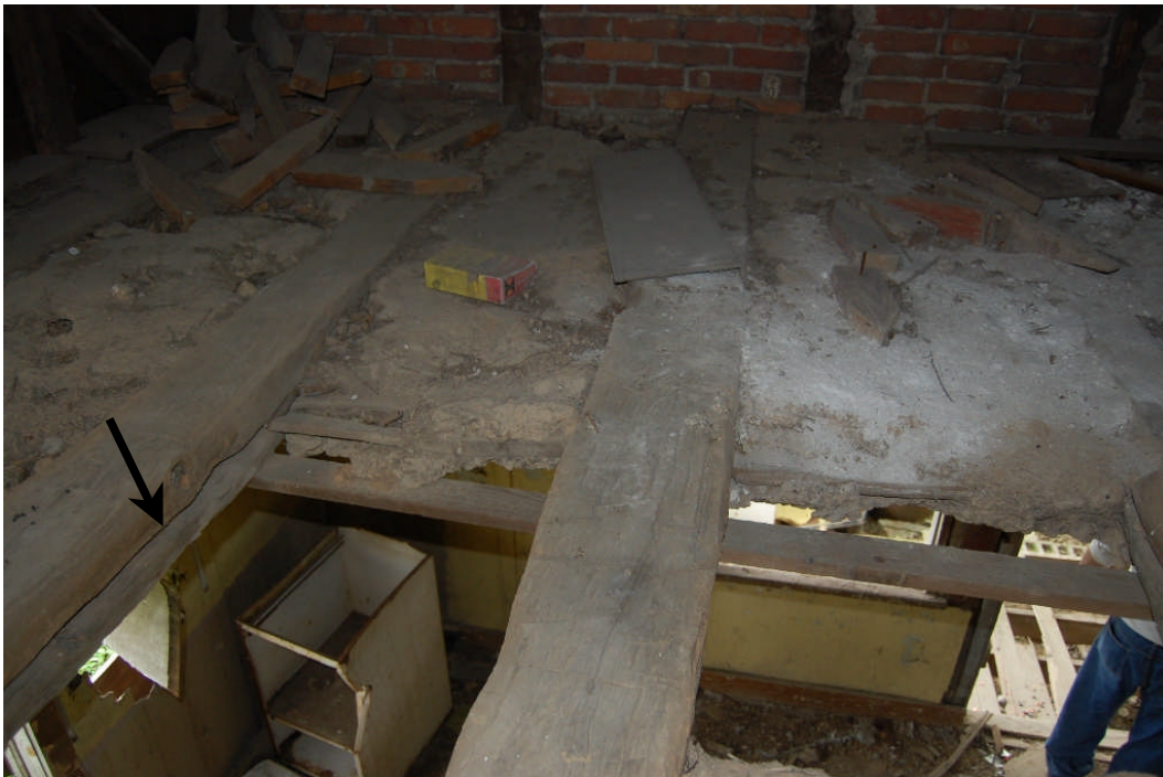
Figure 78. Detail of the floor joists in Room 200. Note mitered channel on side of joists into which the straw-and-clay batts were inserted.
