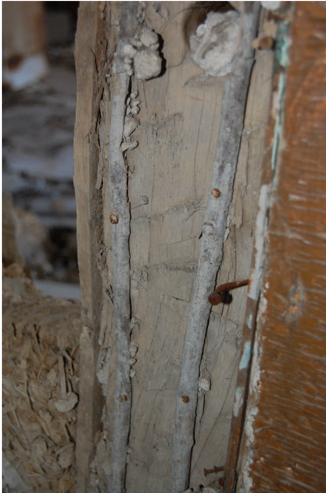
Figure 58. (LEFT) Detail of a hand-hewn post in the common partition wall between Rooms 100 and 101. Twigs have been nailed to surface of the post to provide a surface to which the mud plaster could adhere to. (RIGHT) View of the south wall in Room 101 showing the brick nogging used between the posts and posts on this wall. Brick nogging also was used on the other exterior walls of the original house, as well as in the partition wall between the front two rooms (100 and 101) and rear room (102).
