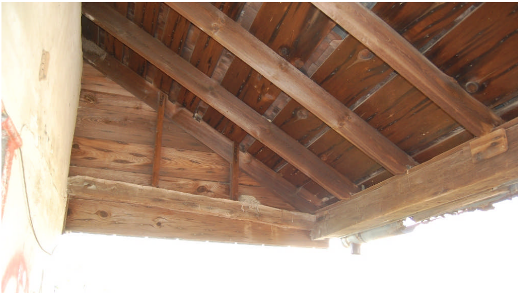
Figure 41. View of the roof framing on the north end of the house porch. The rafter plate is hand-hewn oak, as is the beam on the gable end. The rafters are sawn and were installed when the roof was replaced in the late nineteenth century.
