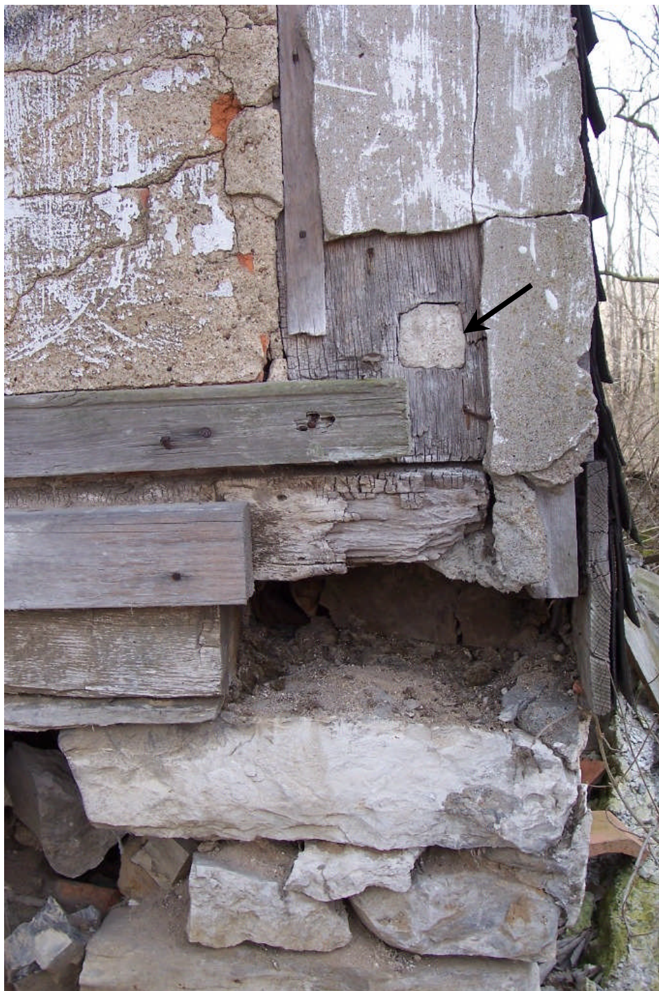
Figure 37. In contrast to the sill on the opposite end of the porch, the north porch sill was half-lapped around the eastern sill plate of the house. The porch here has fallen away from the house, but its location is marked by the void shown above. This image also shows the location of a long-removed porch rail (note arrow).
