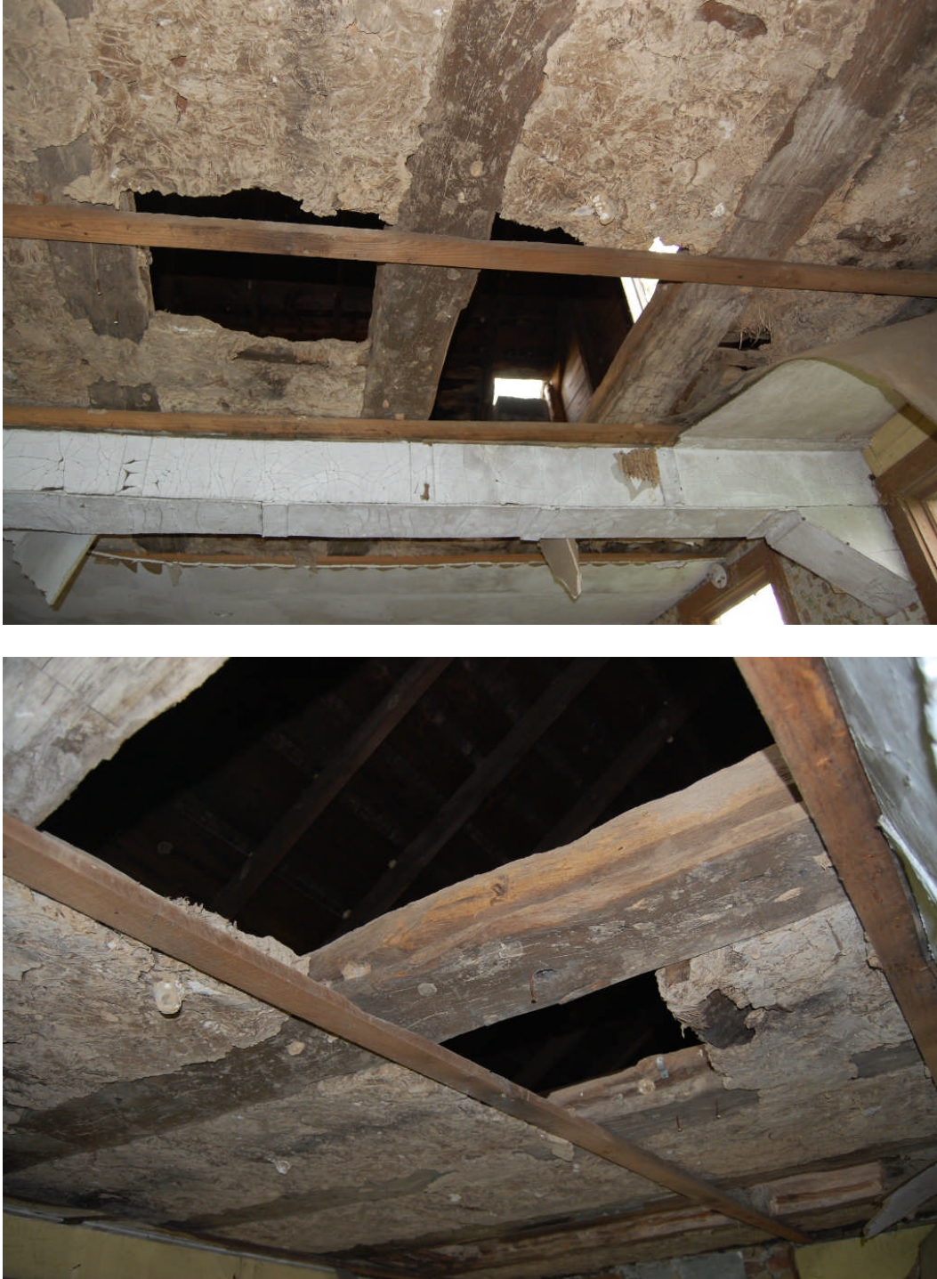
Figure 50. Details of the ceiling framing in Room 100. The ceiling is framed with widely spaced, hand-hewn oak joists that have been mitered to accommodate batts of insulation composed of a straw and mud mixture wrapped around rived oak planks/lath. This method of insulation is referred to by some sources as “Dutch biscuit.” After the batts were installed, the entire ceiling was then coated over and leveled off with a mud-based plaster and painted.
