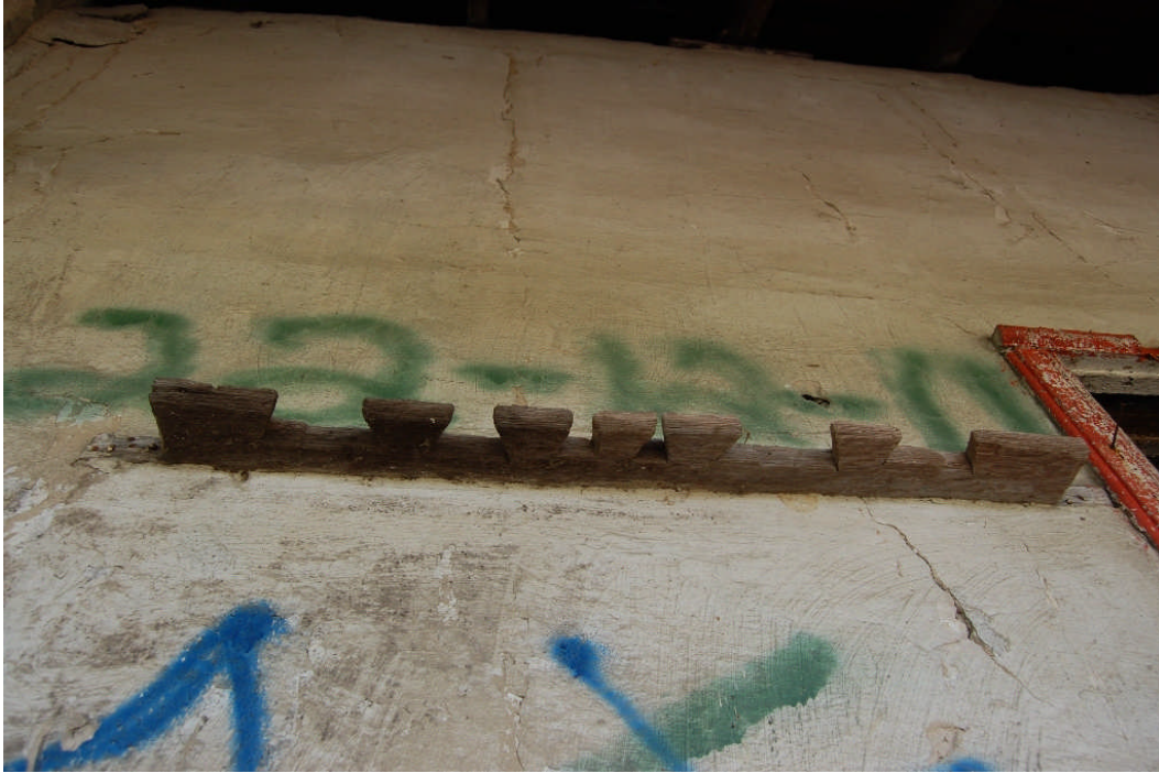
Figure 40. Incised into the north wall of the original house is a plank that has variably sized notches. This served as a rack for holding different tools, such as brooms. The tool rack appears to be original to the house, or at least was installed very early in the dwelling's history.
