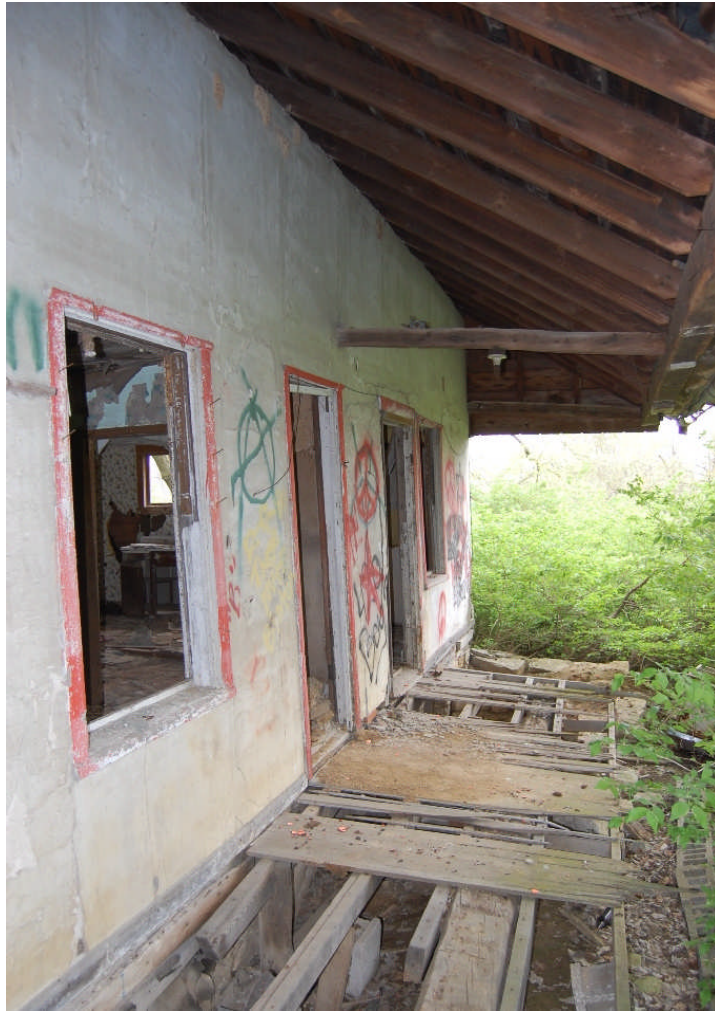
Figure 35. (LEFT) View of the front porch on the east side of the original house. The wood deck has been replaced at least once in the house's history and that which remains is badly deteriorated. (RIGHT) Detail of the south end of the original porch at its juncture with the stone addition. The southeast corner post of the original house is partially exposed, and there is evidence of a porch rail having been mortised into it at one time (marked with arrow). The hand-hewn oak sill of the original porch has been sawn off.
