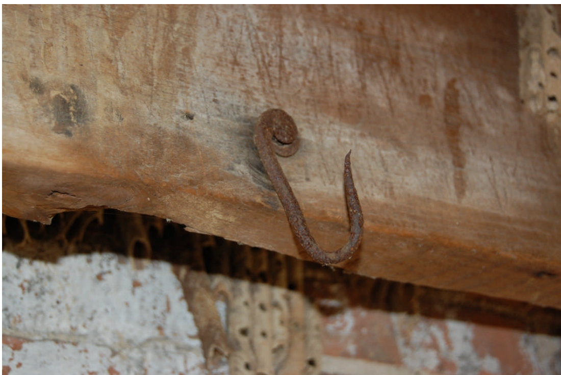
Figure 120. Details of the hooks and nails from which meat was hung in the smokehouse.
