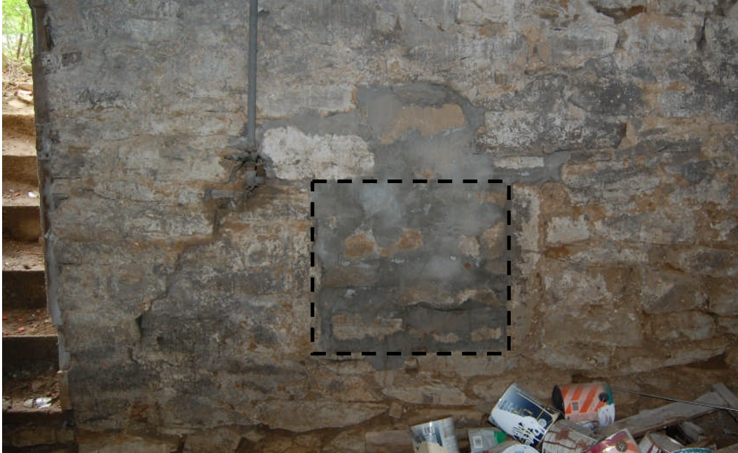
Figure 98. View of an infilled wall niche on the east side of Room 000. The dashed line delineates the outline of the niche.
