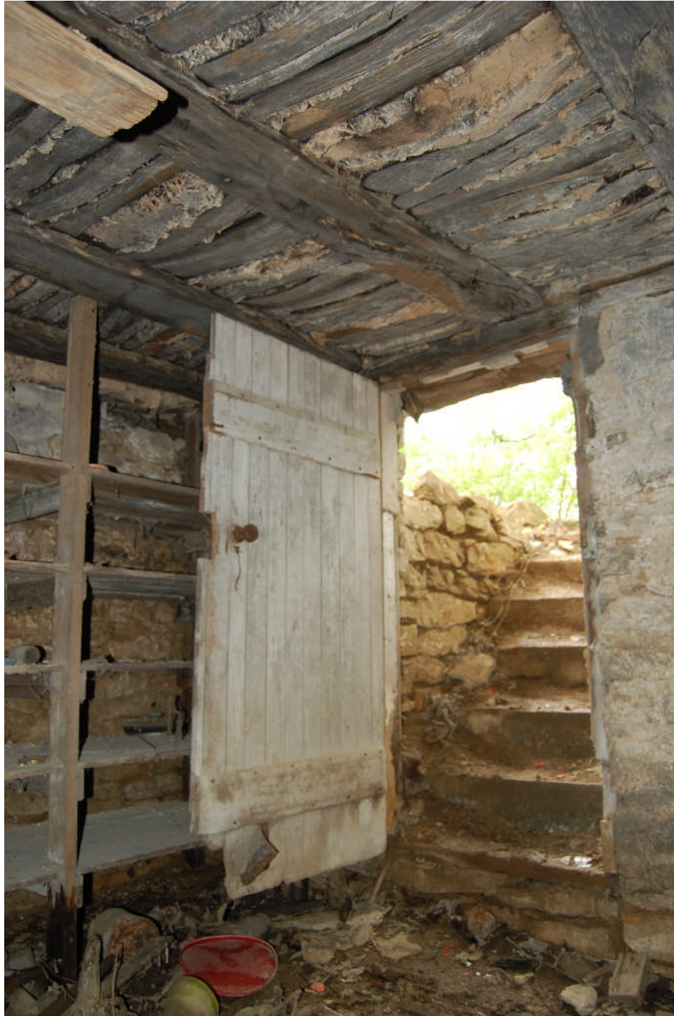
Figure 94. View of the entrance door from the original cellar (Room 000). The ceiling joists are similar to those used on the floor above and employed a similar method of “Dutch biscuit” insulation.
