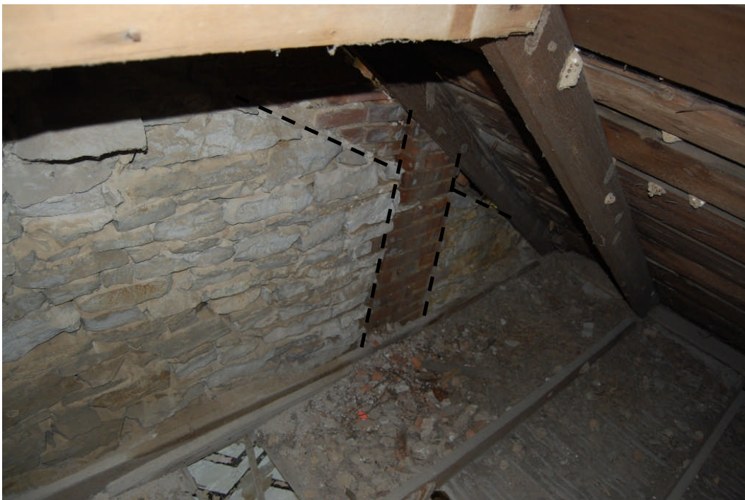
Figure 91. Inside of the south-gable-end wall of the stone addition in attic “dead space” above Room 104. Dashed lines indicate the location of a brick chimney integrated within the stone wall, and also the original roof line.
