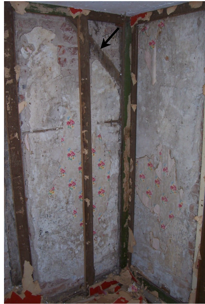
Figure 65. (LEFT) View of a remnant of the original rafter plate from the rear wing of the original house (marked with arrow). This plate was sawn off when the west wall of the wing was pushed outward late in the nineteenth century. The plate and post below it are hand-hewn oak. (RIGHT) View of the southeast corner of Room 102C showing original wall finishes. The walls shown have brick noggin between the framing and are plastered. Note the diagonal bracing.
