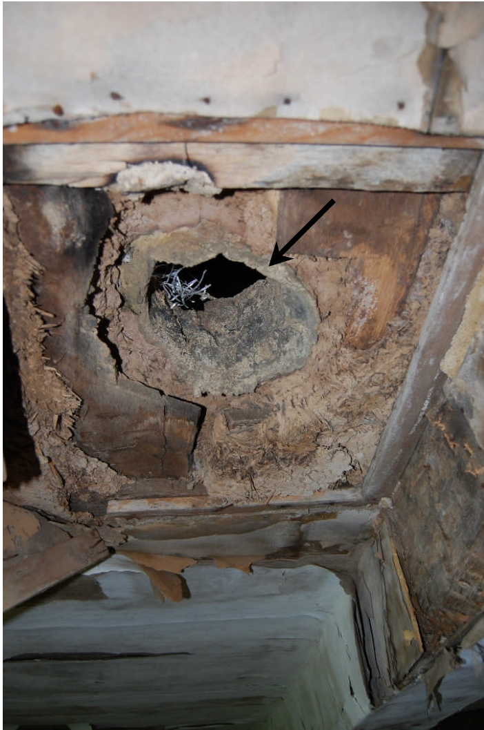
Figure 59. (LEFT) Opening for a stovepipe in the ceiling of Room 101. There is no evidence of a masonry chimney ever being present in this room. (RIGHT) Surviving section of wallpaper on the south side of Room 101. There is evidence of several generations of wallpaper on the walls and ceiling.
