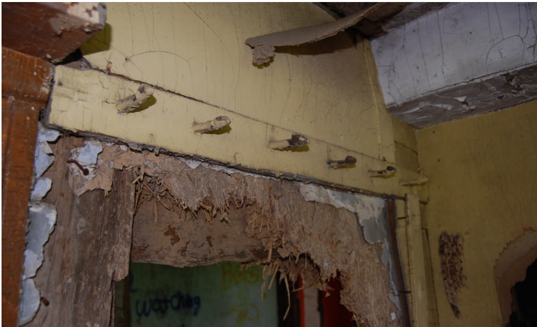
Figure 45. Close-up of the preview figure showing the hat/clothing rack in more detail. The hooks are carved wood. This image also illustrates the character of the partition wall between Rooms 100 and 101, which was enclosed with a straw-mud mixture applied over wide, rived, oak lath.
