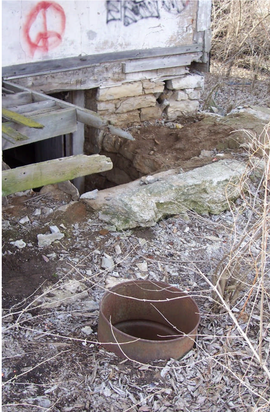
Figure 124. The farmstead also had an outdoor drinking fountain in its front yard during the middle twentieth century. The supply pipe for the drinking fountain ran up through the steel drum shown in the image above.
