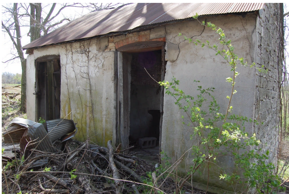
Figure 113. East elevation of the summer kitchen, which faces towards the house. The door at left opens into the smokehouse, while that at right accesses the washroom, which is the larger of the two rooms. The debris piled in between the doorways obscures the opening to a brick-lined cistern.
