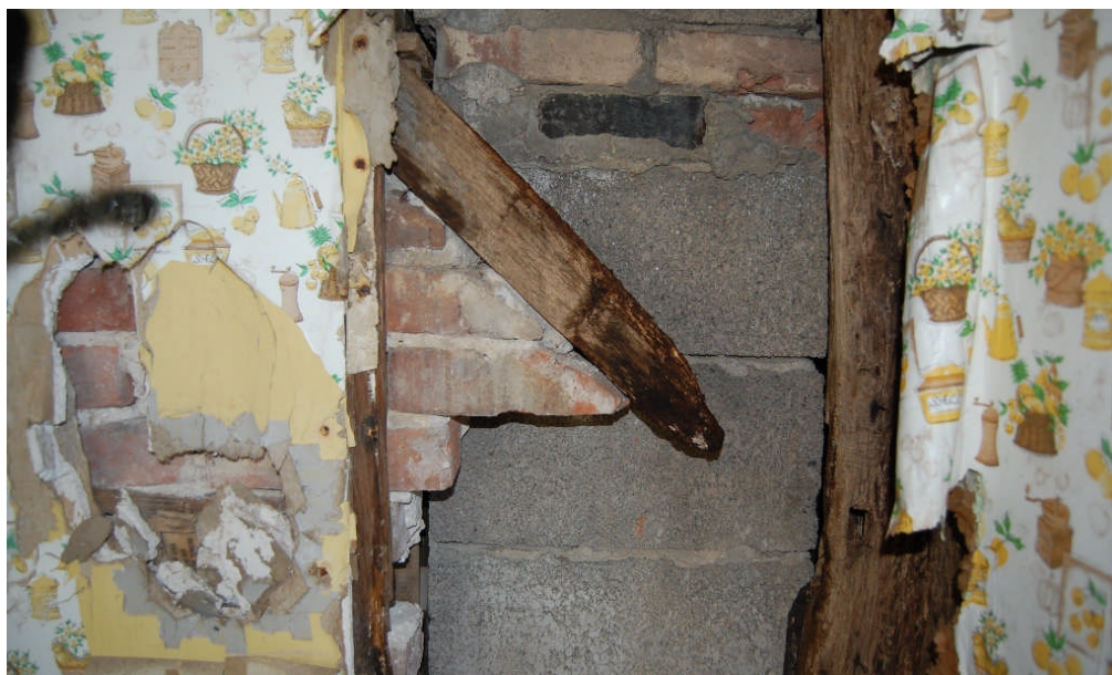
Figure 53. Deteriorated diagonal corner bracing in the northwest corner of Room 100, adjacent to the concrete-block. The deterioration appears have been caused by water leaking down through the chimney opening. Note the manner in which the brick nogging has been cut to fit the framing.
