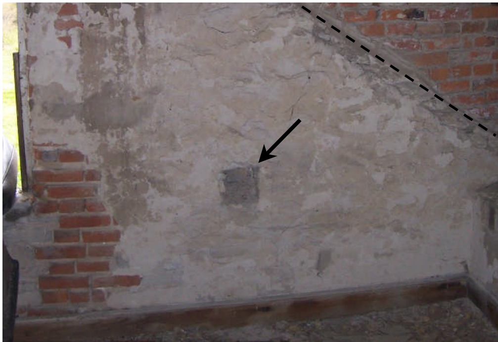
Figure 89. View of one of two niches or (more likely) infilled vents in the south gable-end wall of Room 202. The brickwork to the left of the niche or vent is associated with a chimney. The dashed line again illustrates the original roof line for the stone addition.
