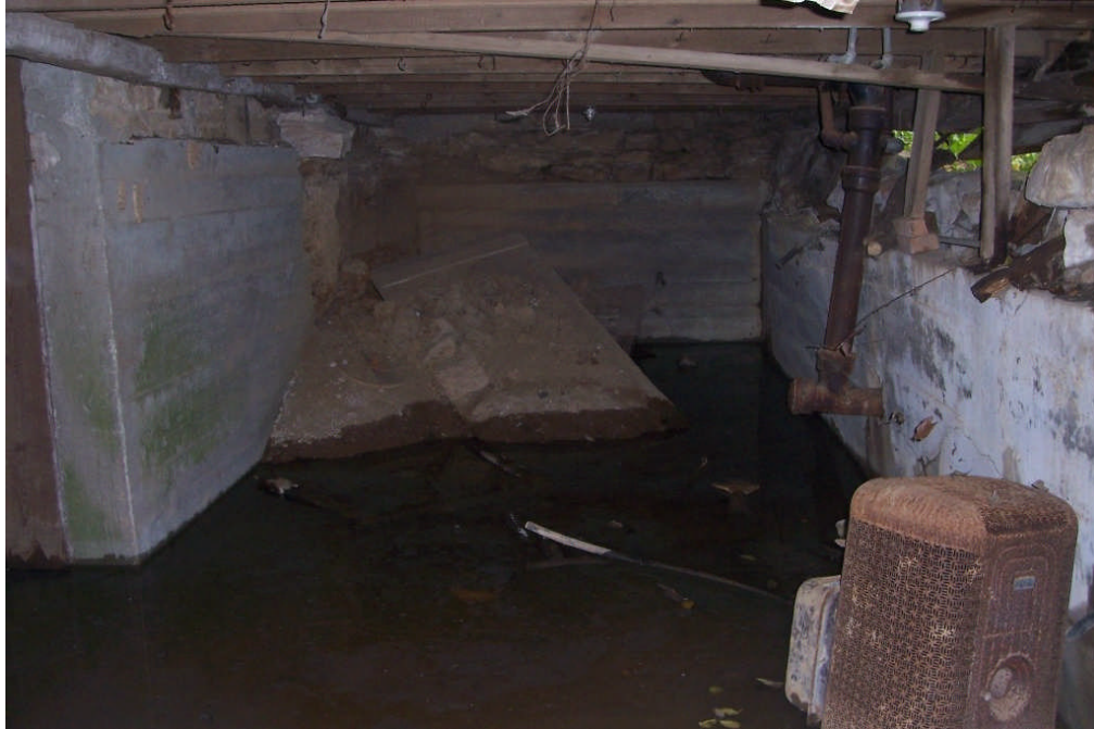
Figure 104. Interior view of Room 001, the “new” basement excavated in the 1940s, looking south. The room has concrete walls/foundations, a section of which have collapsed, as seen in this view. Note oil heating stove at lower right.
