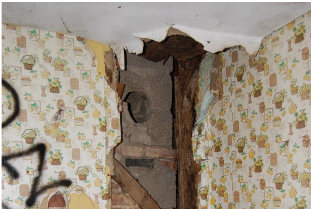
Figure 52. A concrete-block chimney is located along the common partition wall between Rooms 100 and 102A. This chimney has a flue vent facing into Room 100 (as shown above). The current stack appears to have replaced an early brick chimney, the base of which is still present in the basement.
