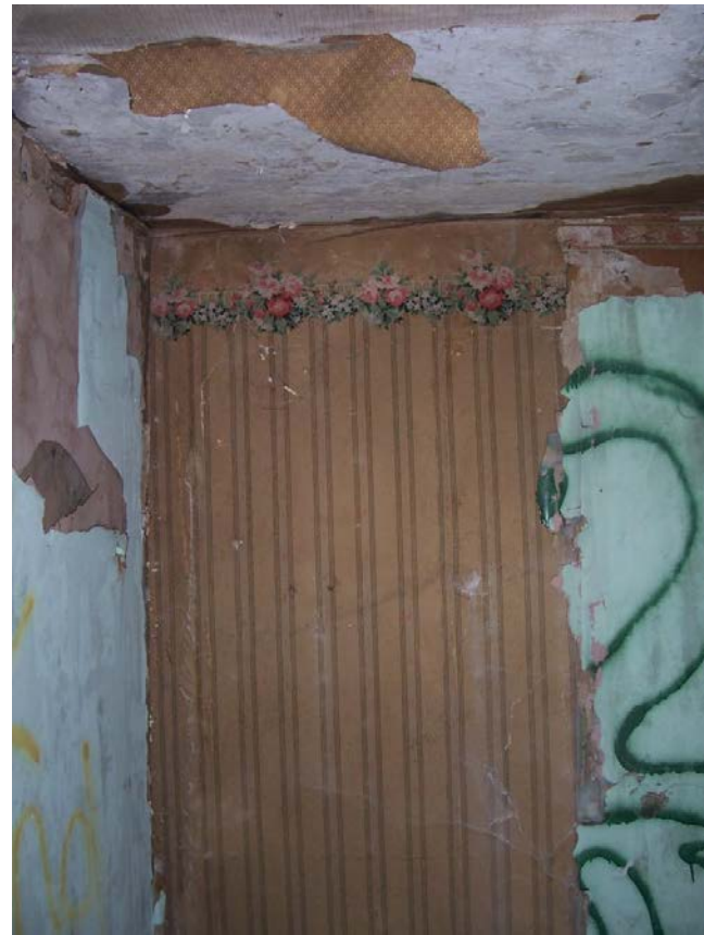
Figure 59. (LEFT) Opening for a stovepipe in the ceiling of Room 101. There is no evidence of a masonry chimney ever being present in this room. (RIGHT) Surviving section of wallpaper on the south side of Room 101. There is evidence of several generations of wallpaper on the walls and ceiling.
