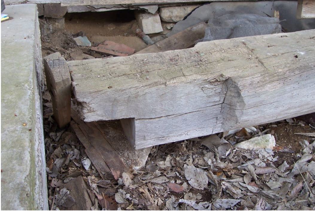
Figure 38. View of the south end of the center beam on the front porch of the original house showing method of notching used around to fit the beam around the sill.
