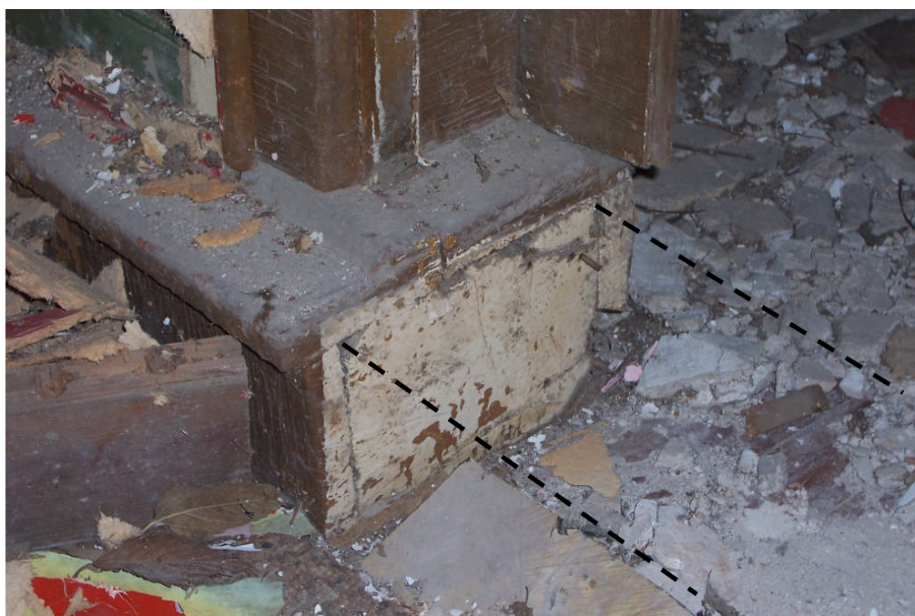
Figure 64. Close-up of the base of the doorway shown in the previous figure, between Rooms 102C and 104. The original sill plate was sawn off to install this opening, and the remaining sill was boxed in with trim. The dashed lines indicate continuation of the sill plate.
