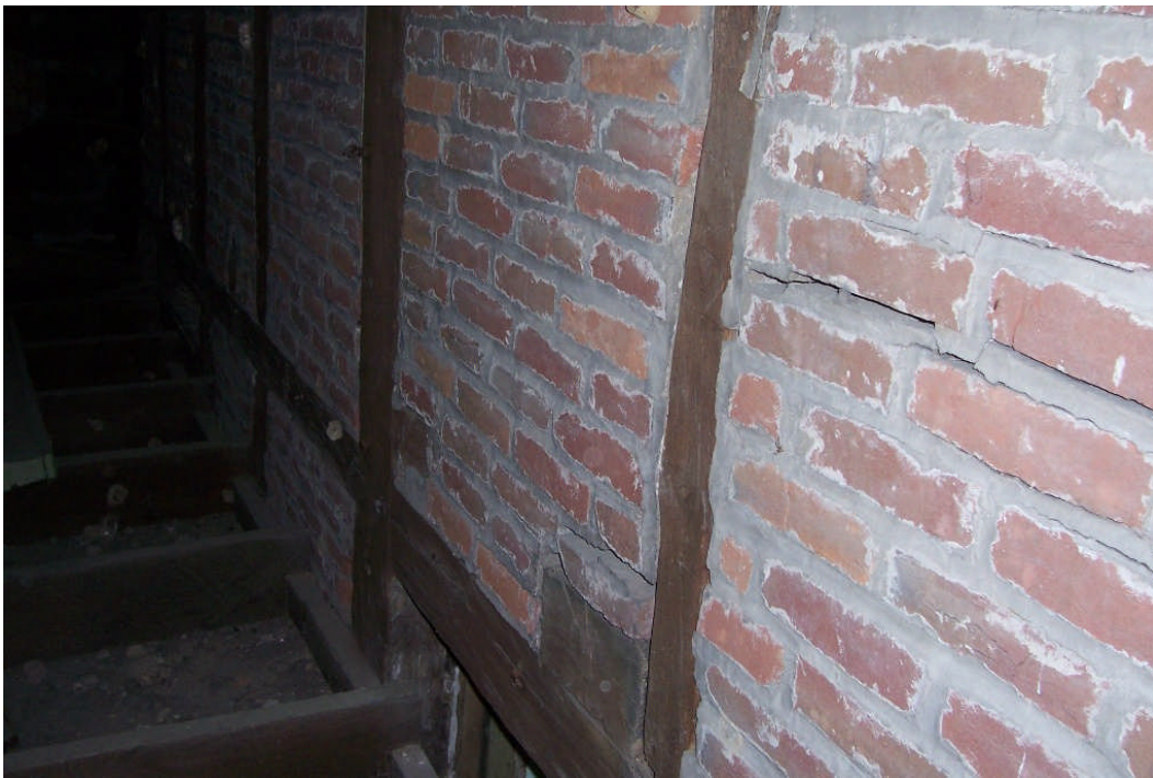
Figure 82. Two views of the rear (or west) side of the wall of Rooms 200 and 201. Unlike the front elevation of the house, the brick nogging here shows no evidence of ever having been plastered over. The mortar joints also are in exceptionally good condition. These facts support the impression that the original house always had a rear wing. These images also illustrate the manner of framing employed in the original house, with the posts being mortised—and slightly inset—into a girt, which serves a ceiling plate on which the joists rest directly on top of (as opposed to being notched into or around).
