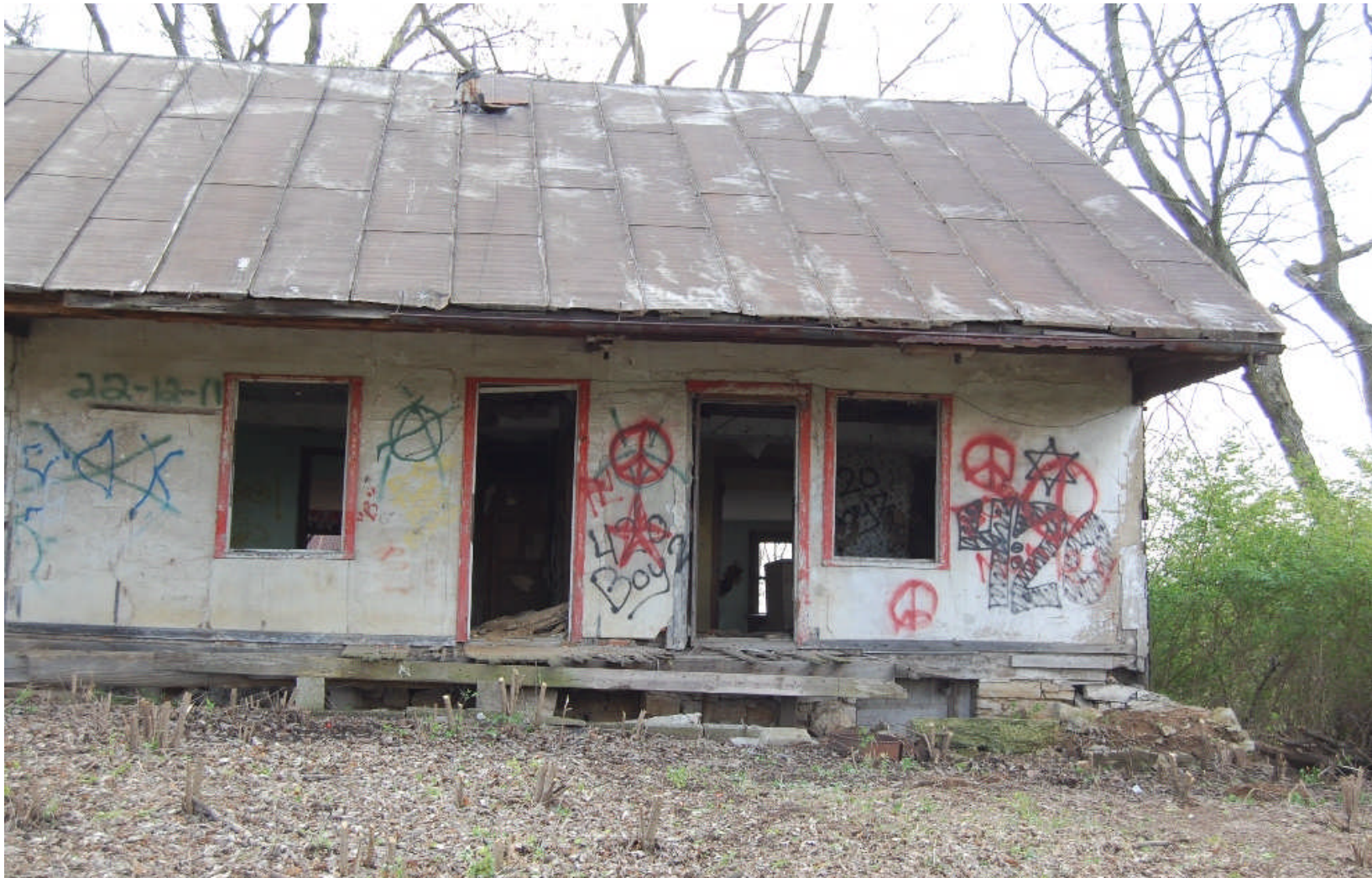
Figure 32. Front (east) elevation of the house, showing original section. Note the paired doorways accessing the two front rooms of the original house. Also of note is plastered façade, which is protected from elements within the deep porch. The plaster finish covers a half-timber frame with brick nogging.
