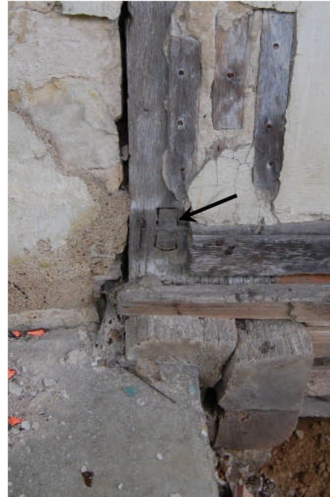
Figure 35. (LEFT) View of the front porch on the east side of the original house. The wood deck has been replaced at least once in the house's history and that which remains is badly deteriorated. (RIGHT) Detail of the south end of the original porch at its juncture with the stone addition. The southeast corner post of the original house is partially exposed, and there is evidence of a porch rail having been mortised into it at one time (marked with arrow). The hand-hewn oak sill of the original porch has been sawn off.
