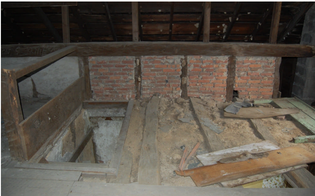
Figure 76. Room 200, looking north. The walls and floor in this room were never finished, which suggests that it was not intended to have regular use. Note the exposed floor joists, posts, and brick nogging. The stairway accessing the attic from Room 100 appears at lower left.
