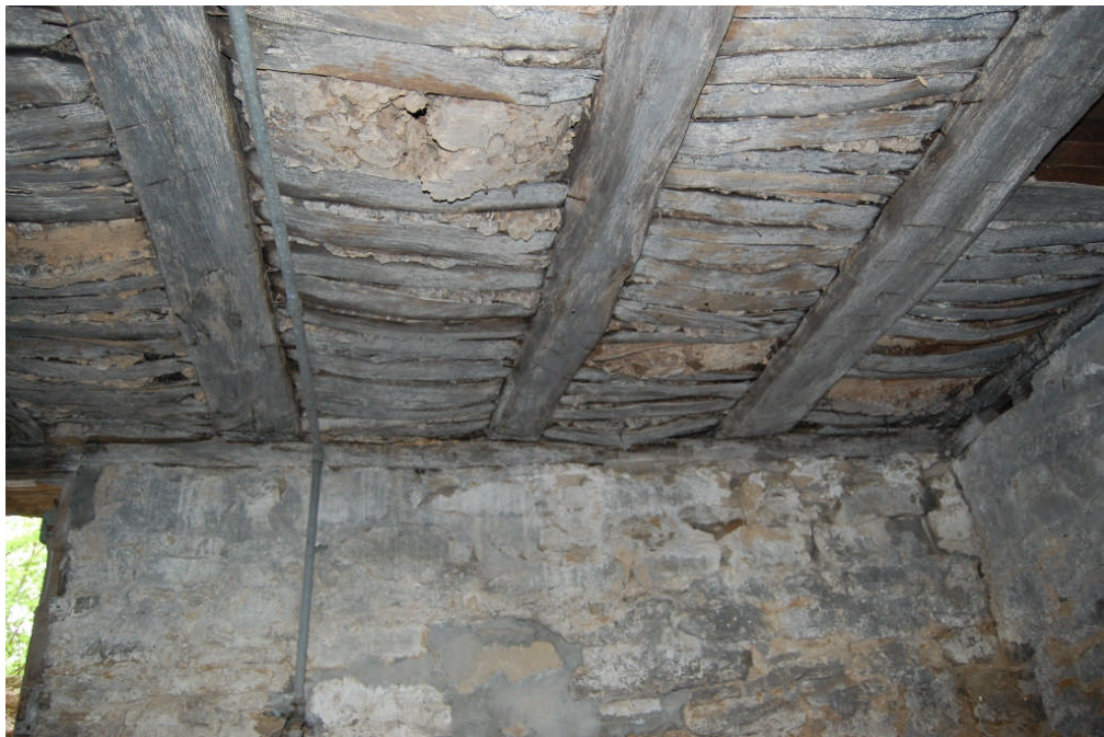
Figure 101. Like the ceilings in Rooms 100 and 101, that in Room 000 is insulated with clay and straw. However, the straw-and-clay mixture was not rolled around the rived oak planks/lath to form a batt, but rather was deposited in a distinct layer on top of latter and then covered over with tongue-and-groove flooring.
