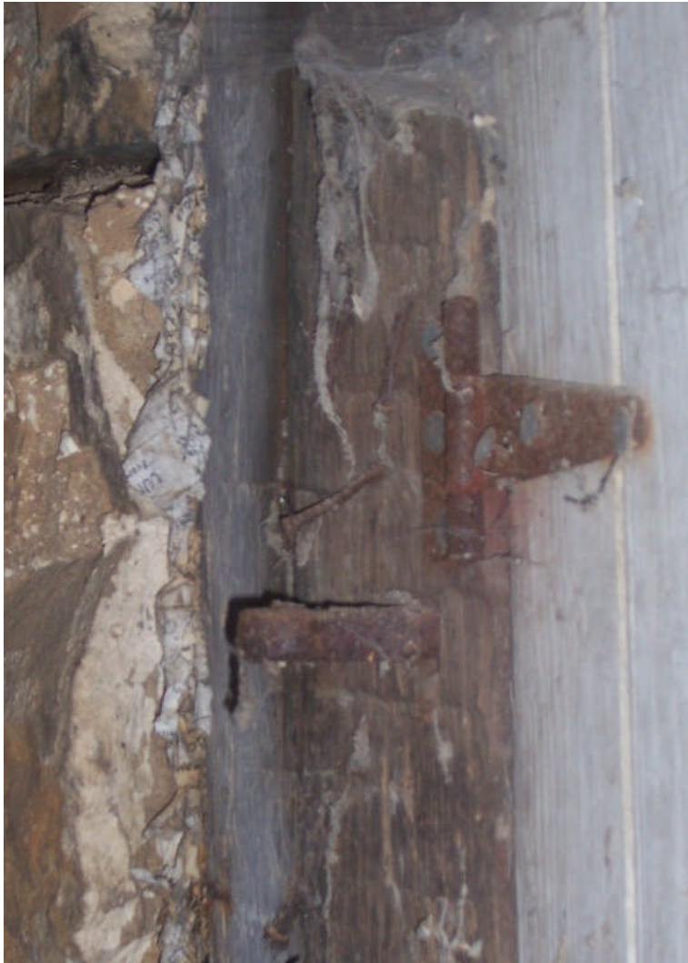
Figure 97. (LEFT) The original cellar entrance door appears to have been hung from hand-forged pintle, one of which is shown here. The existing door is hung with strap hinges. (RIGHT) View of a wall niche on the south side of Room 000. This is one of three once present in the cellar. Such niches have been documented at several other German farmstead in southwest Illinois.
