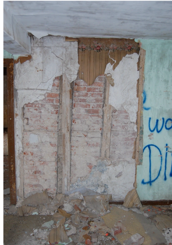
Figure 58. (LEFT) Detail of a hand-hewn post in the common partition wall between Rooms 100 and 101. Twigs have been nailed to surface of the post to provide a surface to which the mud plaster could adhere to. (RIGHT) View of the south wall in Room 101 showing the brick nogging used between the posts and posts on this wall. Brick nogging also was used on the other exterior walls of the original house, as well as in the partition wall between the front two rooms (100 and 101) and rear room (102).
