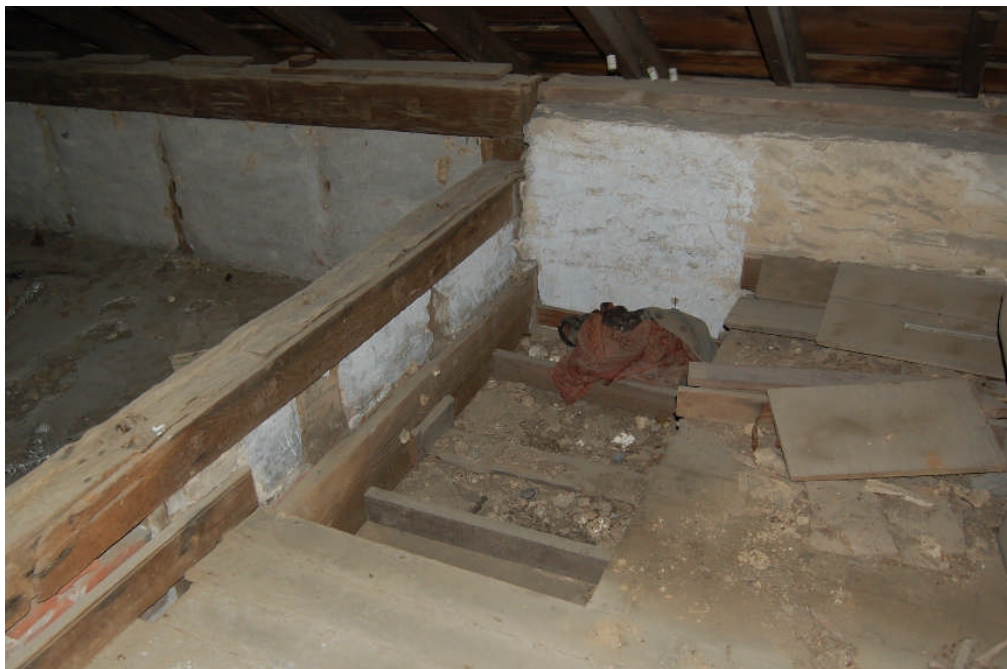
Figure 85. Infilled stair opening in the northeast corner of Room 202. The stairway once located here allowed access to the attic from Room 103 below.
