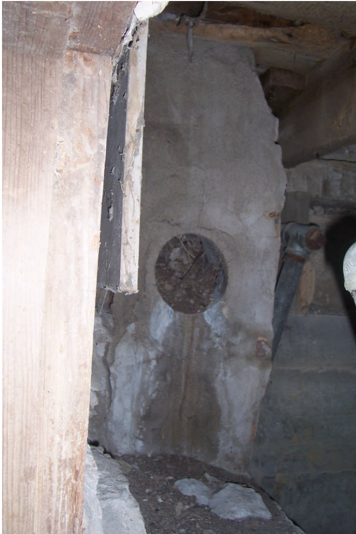
Figure 108. Two views of the brick chimney located in the northeast corner of Room 001. This is connected to the concrete-block chimney that presently rises through Room 101A—thereby suggesting that the latter is a replacement of an earlier brick stack. A stove vent is present in the north side of the chimney.
