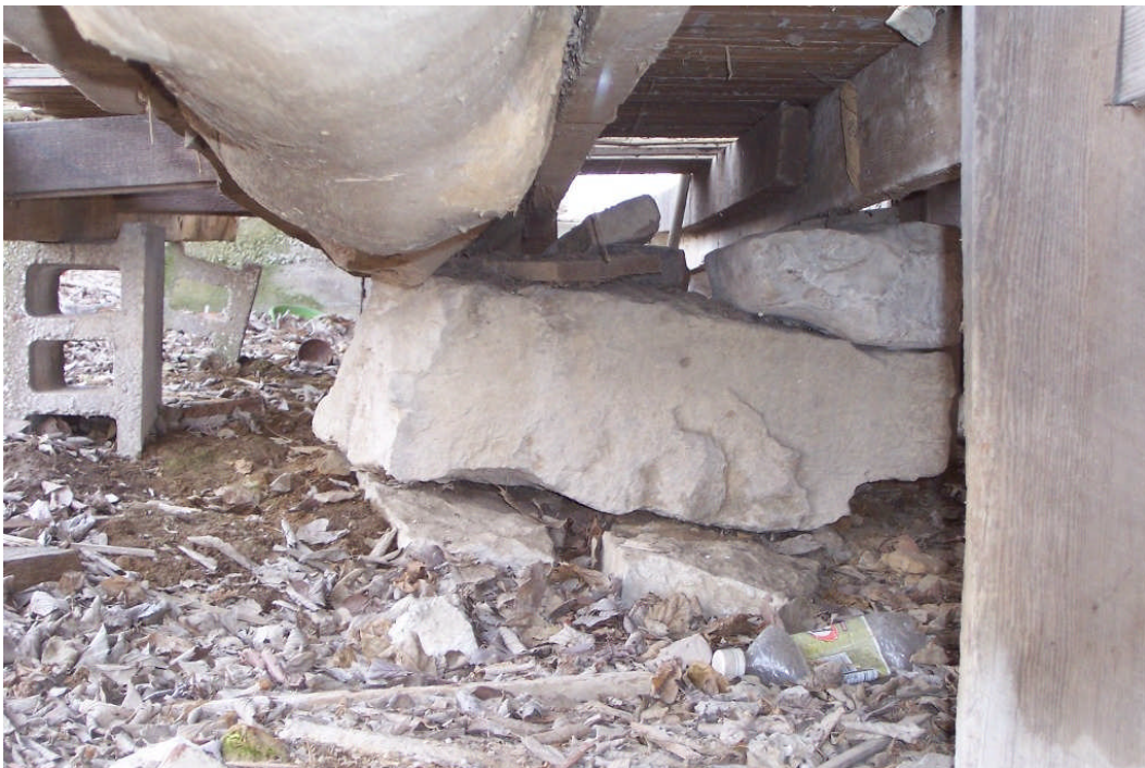
Figure 39. The center beam of the original porch was supported by a stone pier in the middle of its span, as shown above.
