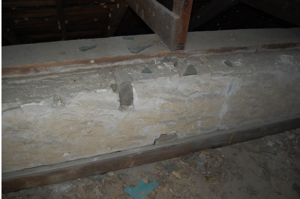
Figure 88. Knee wall on west side of Room 202 showing original rafter plate (A) and associated nailer block (B) integrated within the stonewall. Similar nailer blocks were used for the baseboard below.
