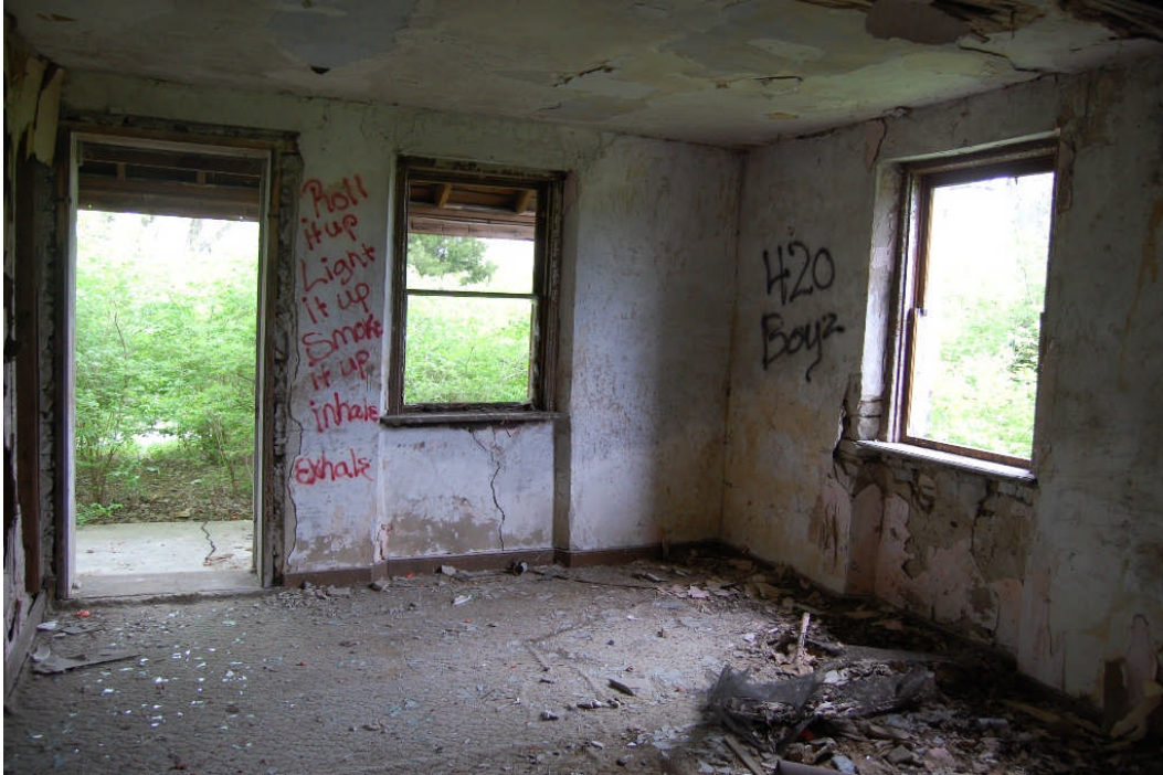
Figure 68. Interior view of Room 103, the front (or east) room of the stone addition, looking into the southeast corner. Note the manner in which the walls are recessed below the window openings.
