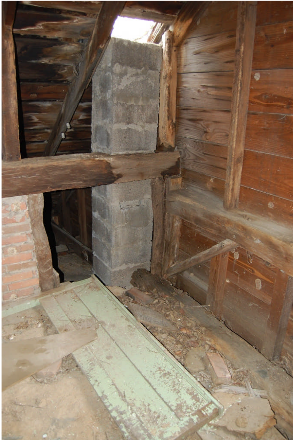
Figure 79. Northwest corner of Room 200, showing the top of the concrete-block chimney. The chimney no longer extends through the roof, but the roof opening was never closed off. This has caused some water damage to the framing adjacent to the chimney.
