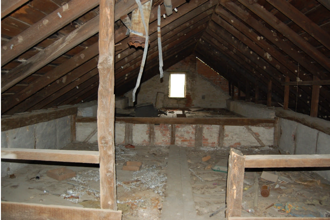
Figure 80. View of Room 201 looking south. In contrast to Room 200, the walls in this area have been plastered and the floor has as well. The wall in the foreground—which separates Rooms 200 and 201—is of horizontal plank construction but has been partially demolished. A section of stovepipe from Room 102 also is shown passing through the roof.
