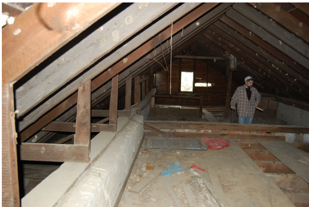
Figure 87. View of west side of Room 202 showing the studs and collar beams added to support the rafters for the late-nineteenth-century replacement roof.
