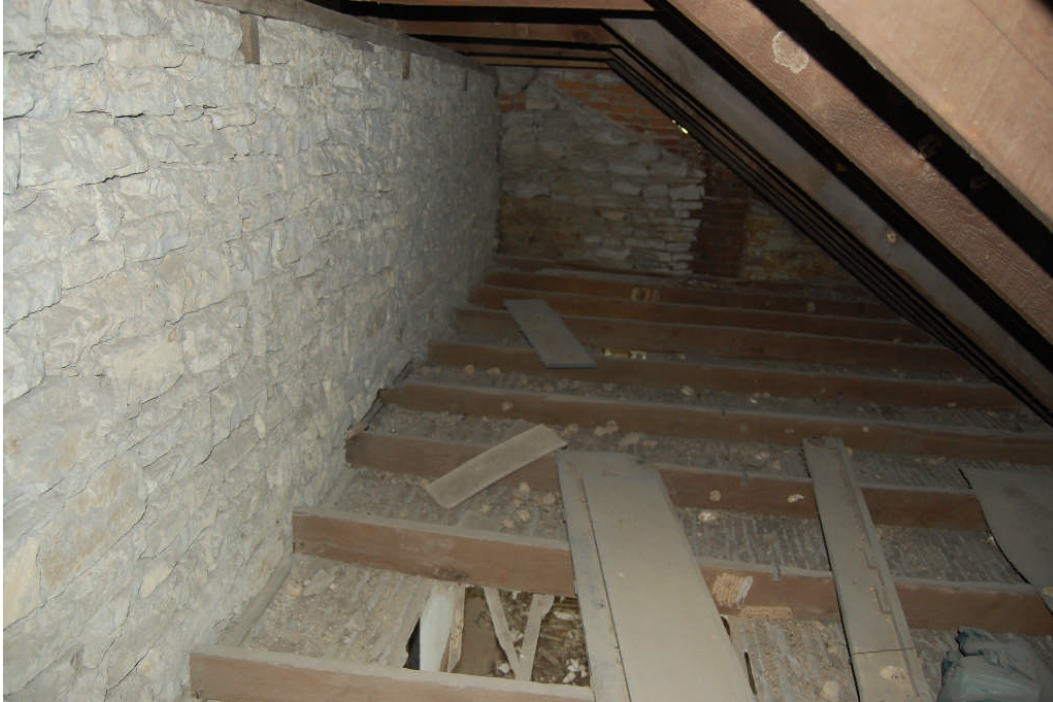
Figure 90. View of the attic “dead space” above Room 104. The stonework here was never exposed and hence no need to be plastered.
