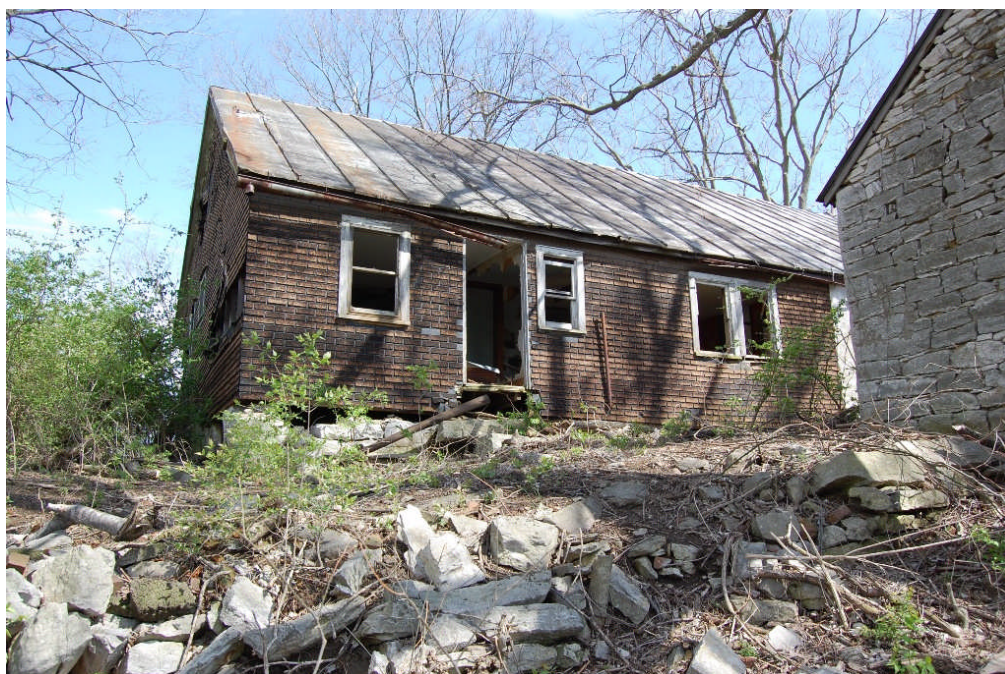
Figure 25. View of the northern end of the west elevation of the house. This wall was rebuilt in the late nineteenth century and remodeled once again the middle twentieth century.
