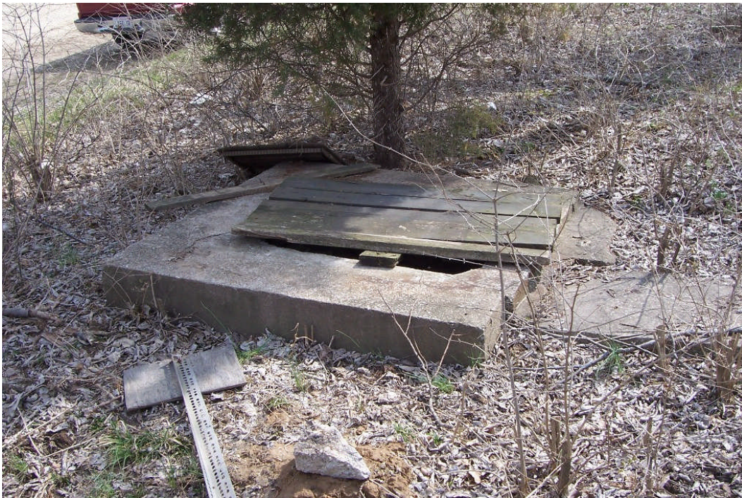
Figure 121. Two views illustrating the location and surface character of the early well shaft at the farmstead. The well is located in the front (east) yard of the house and is connected to the southern front porch by a concrete sidewalk. The well opening has a concrete pavement poured around it, but the shaft itself is lined with stone. A frame well house formerly was located above it.
