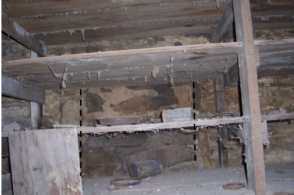
Figure 100. There also appears to have been a wall niche in the north wall of Room 000 (behind the existing shelving), which is delineated here by the dashed lines.
