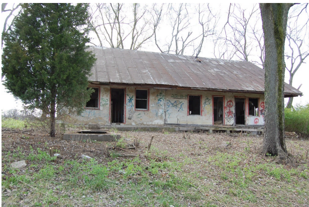
Figure 23. View of the east elevation of the house. The dwelling was constructed in two episodes. The earlier half-timbered section is at right, with the paired doorways. The later stone addition is at left. This image and those that follow show conditions in the Spring and Summer of 2009.
