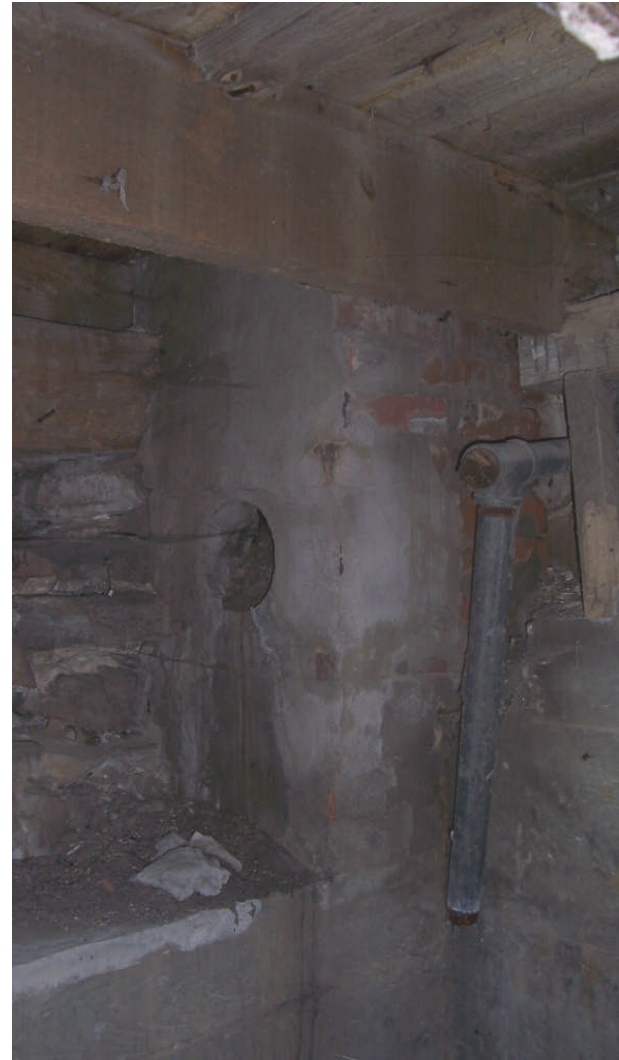
Figure 108. Two views of the brick chimney located in the northeast corner of Room 001. This is connected to the concrete-block chimney that presently rises through Room 101A—thereby suggesting that the latter is a replacement of an earlier brick stack. A stove vent is present in the north side of the chimney.
