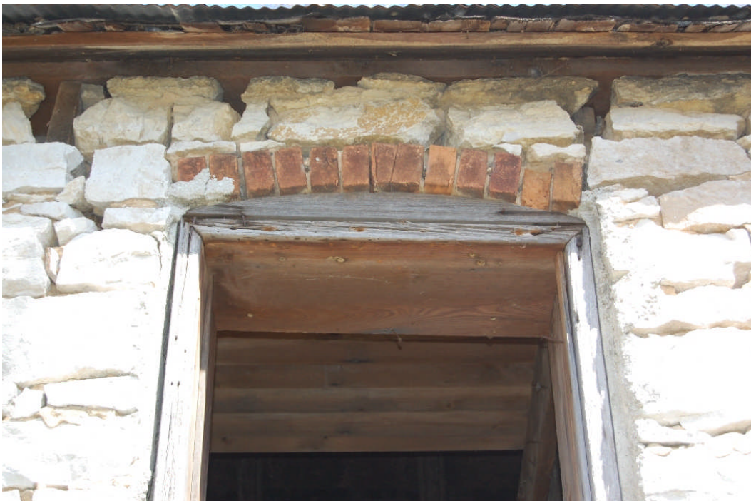
Figure 117. Detail of the window opening in the summer kitchen. Bricks were used to form the segmental arched opening, being arranged in a single rowlock.
