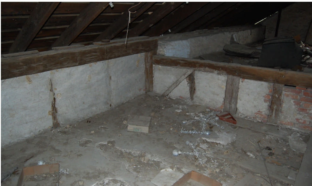
Figure 81. View into the southeast corner of Room 201 showing character of plastered walls and floor. The plaster on the walls is quite thin, leaving the framing partially exposed in some instances.
