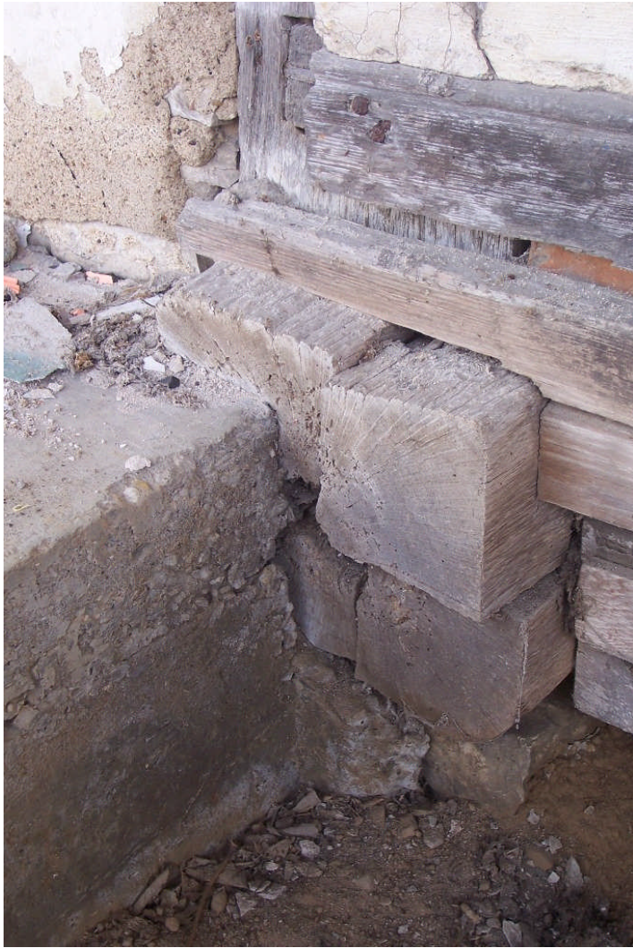
Figure 36. Close-up views of the sawn-off sill on the south end of the original house, illustrating the manner in which the porch sill was half-lapped around the southern house sill plate, which was extended 3" inches beyond the wall plane to accommodate the former. The images show the porch sill remnant before and after removal.
