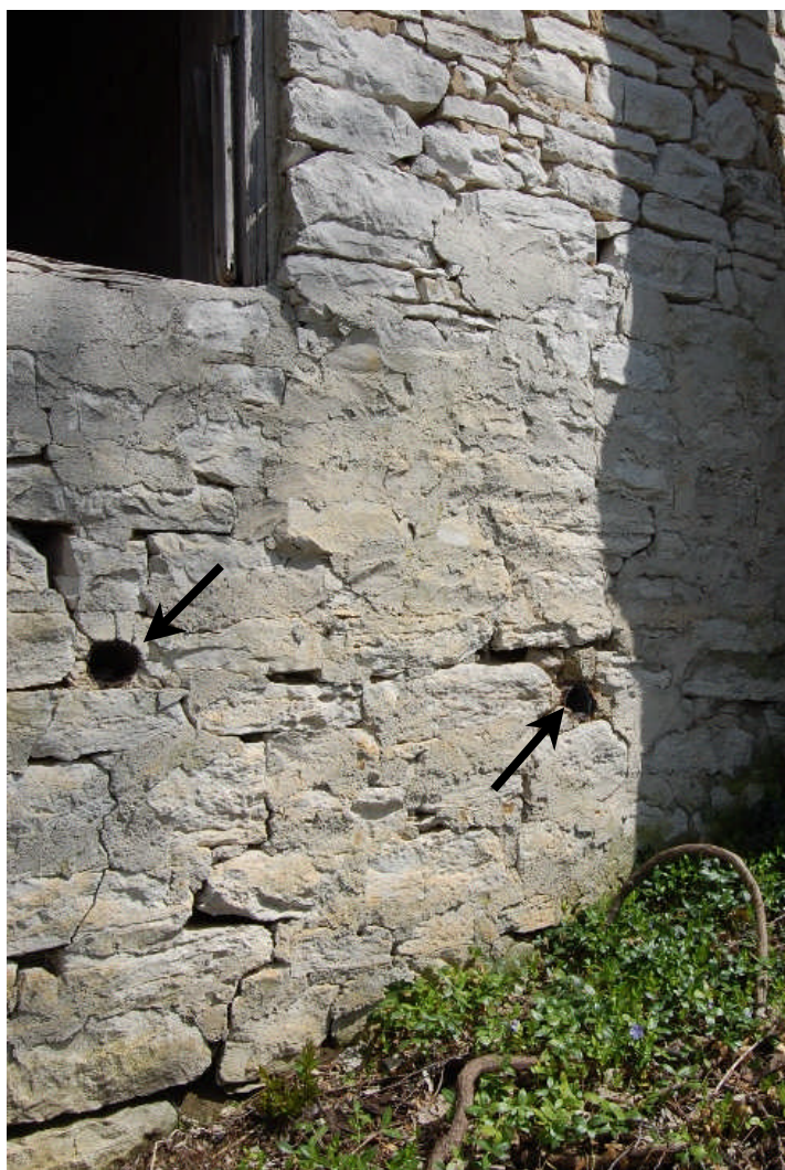
Figure 118. (LEFT) Detail of the west elevation of the summer kitchen showing the two drain pipes here (marked by arrows). Each pipe is connected to a floor drain in the two rooms on the interior. (RIGHT) Interior view of the washroom looking west. The machine shown is a cream separator. The brick wall separates the washroom from the adjacent smokehouse. This wall has been whitewashed in the past and later had been its lower half paged with concrete.
