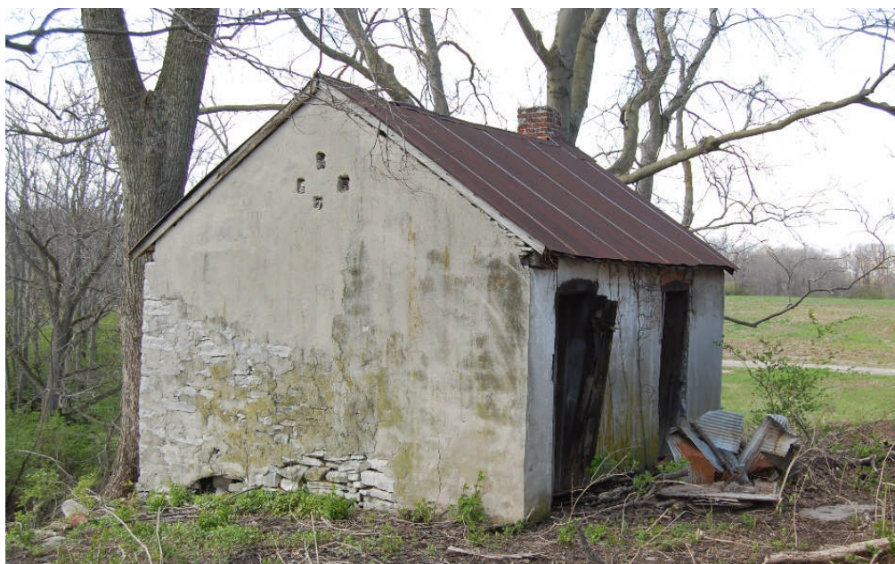
Figure 112. View of the summer kitchen looking northwest. The south and east elevations are shown. Note the vents in the gable end and plastered exterior. On its interior, the building is divided into rooms: a smokehouse and a washroom.
