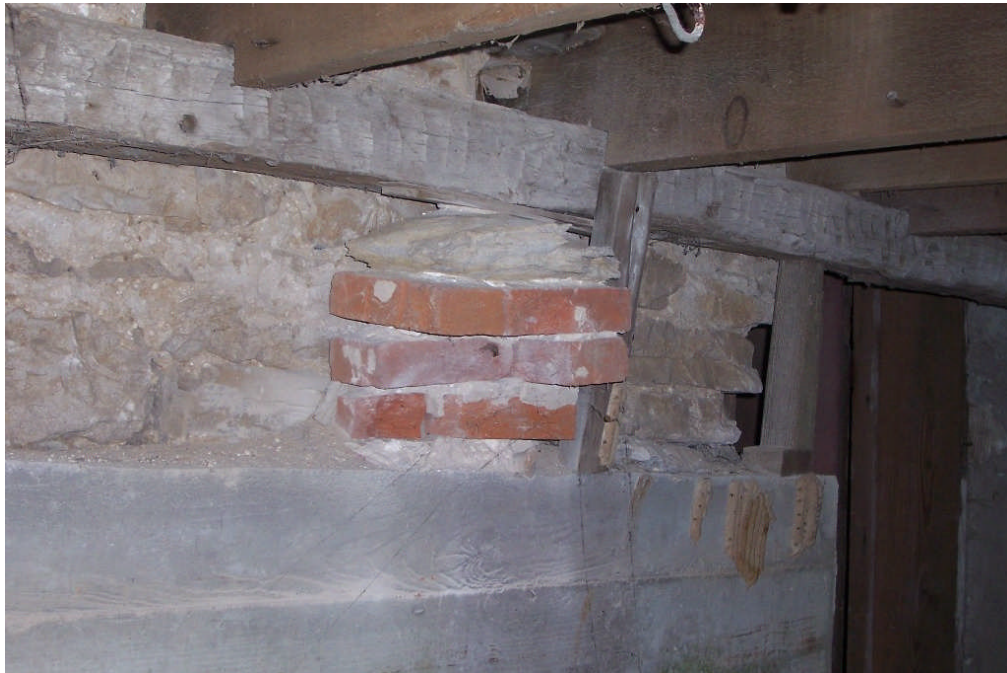
Figure 107. Another view of the eastern sill plate in Room 001, showing a fragment of a brick pier retained after this basement room was excavated in the 1940s. Note the new concrete wall below the pier.
