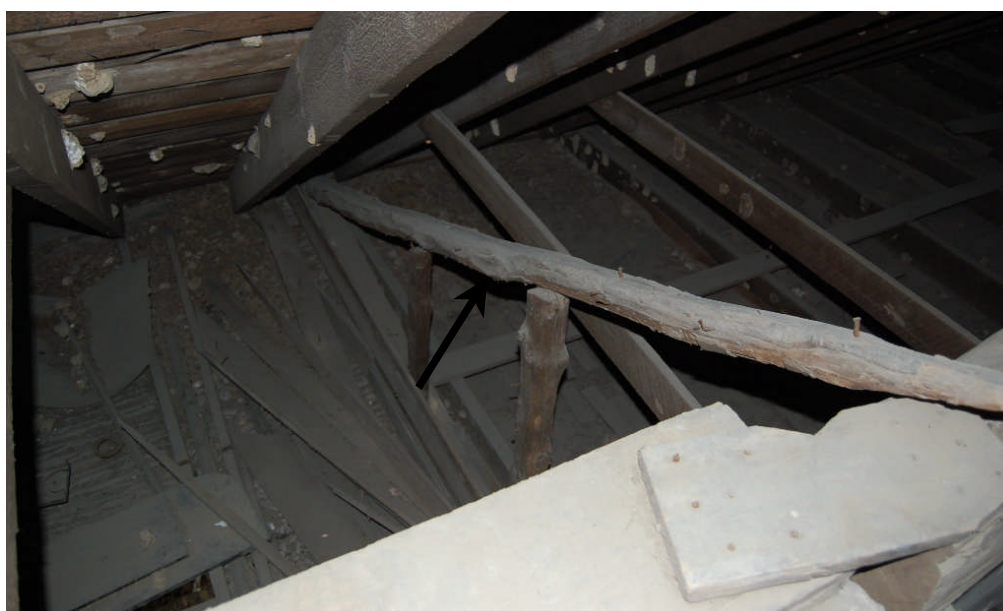
Figure 67. View of a surviving pole rafter associated with the early roof over the rear wing of the original house. The existing roof pitch over the wing is much steeper than what it was originally.
