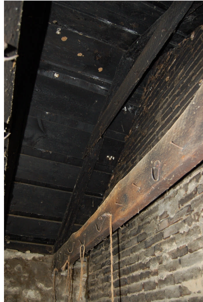
Figure 119. Interior views of the smokehouse room in the summer kitchen. (LEFT) In contrast the washroom, the smokehouse has a dirt floor. The steel tub shown appears to have been used to contain the smoldering fire used to cure the meat hung in the room. (RIGHT) The ceiling of the smokehouse was left open to the rafters and is blackened from years of smoking. Meat was hung from hooks and nails attached to the ceiling joists.
