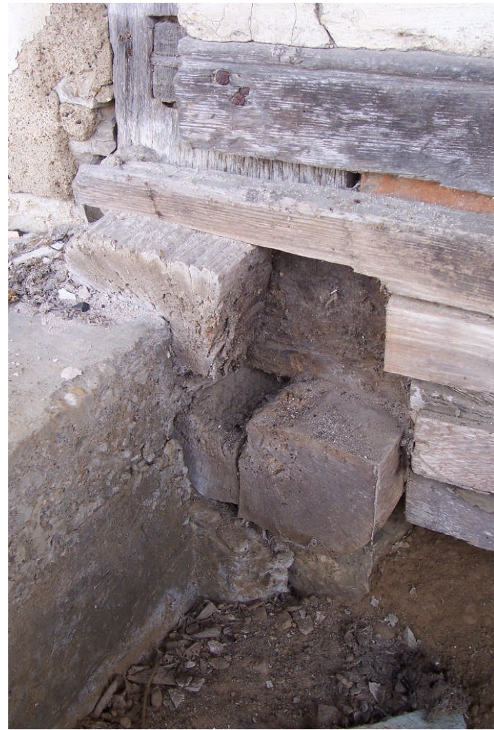
Figure 36. Close-up views of the sawn-off sill on the south end of the original house, illustrating the manner in which the porch sill was half-lapped around the southern house sill plate, which was extended 3" inches beyond the wall plane to accommodate the former. The images show the porch sill remnant before and after removal.
