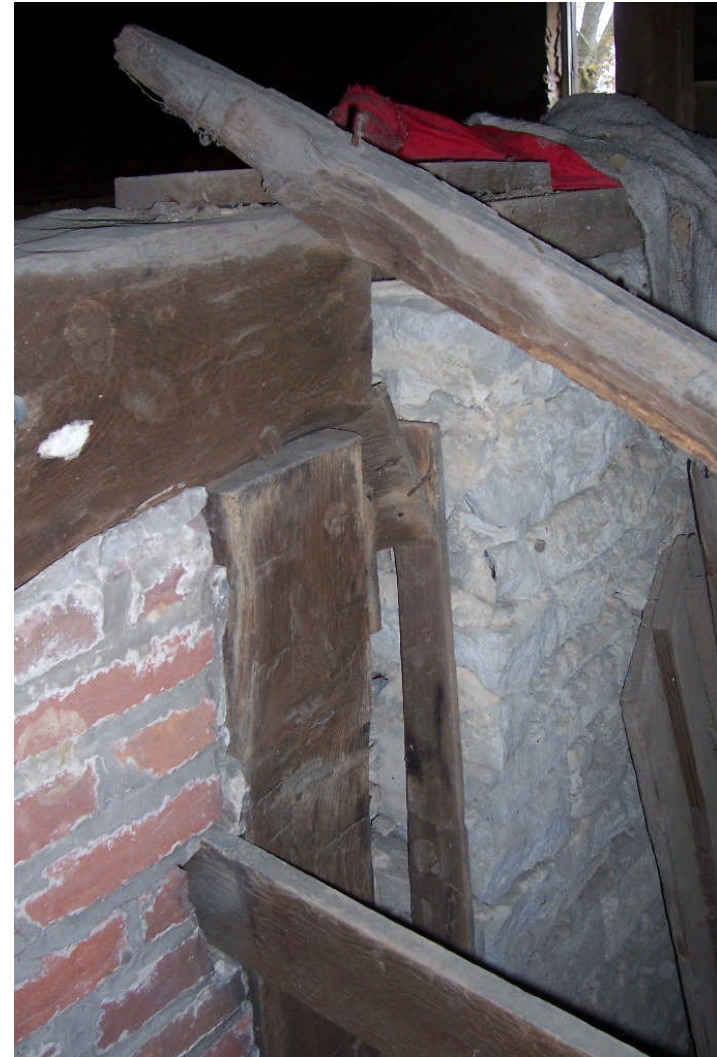
Figure 83. (LEFT) Detail showing main framing members on original house: A) post, B) bracing, C) girt, D) ceiling joist, and E) upper post for attic knee wall. (RIGHT) Interior juncture of the original frame house and the stone addition. This image also shows a corner post and the large girt that originally served as a rafter plate. The remnant pole rafter associated with rear wing also is pictured.
