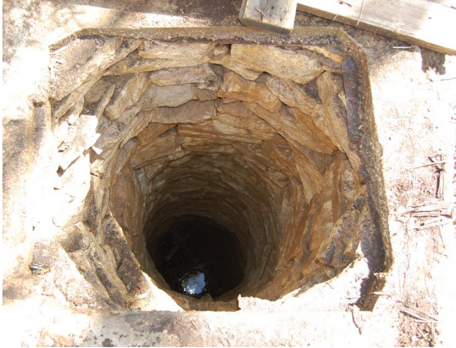
Figure 122. View looking down the stone-lined well shaft. The water level lies approximately 27' below grade.
