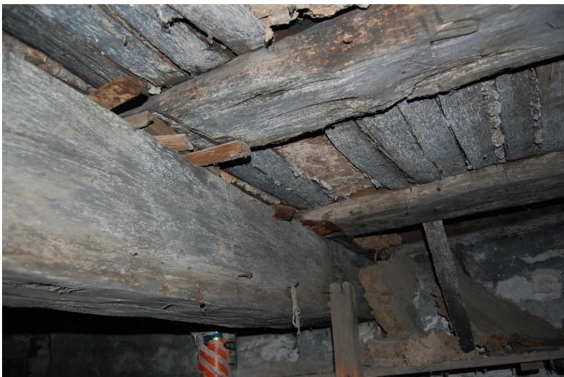
Figure 102. Two views of the large summer beam that supports the joists in the ceiling of Room 000 (showing its northern end). The summer beam is hand-hewn oak and runs east/west, essentially mirroring the system employed on the floor above.
