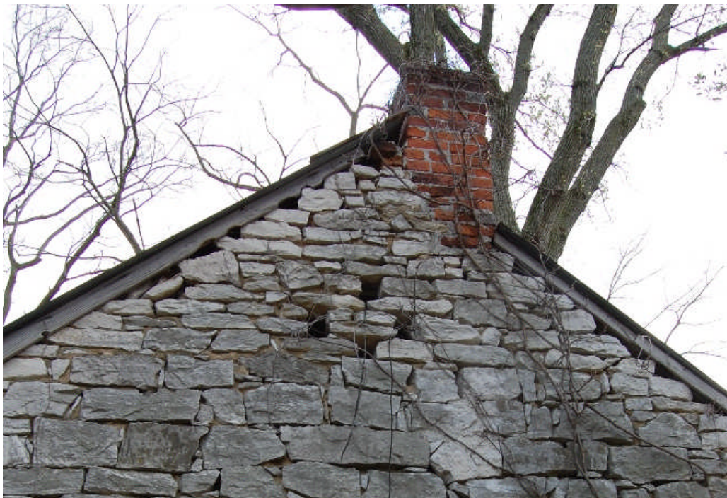
Figure 115. Detail of the north gable of the summer kitchen showing attic vents (arranged in a diamond pattern) and the brick chimney stack present here. The chimney vented a stove in the washroom.
