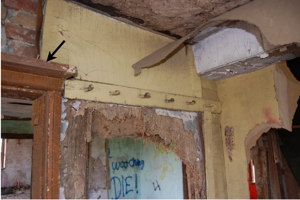
Figure 44. Detail of the south of Room 100 showing the shelf above the doorway between Rooms 100 and 101 (marked with arrow) and hat/clothes rack adjacent to it.
