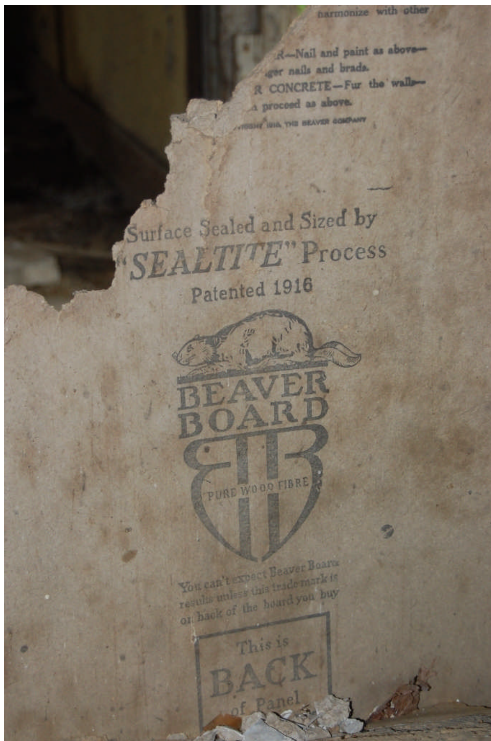
Figure 47. Detail of the rear of a Beaver Board panel used for enclosing a closet in Room 100. A new type of product at the time it patented (1916), Beaver Board included instructions and promotional information on its backside.
