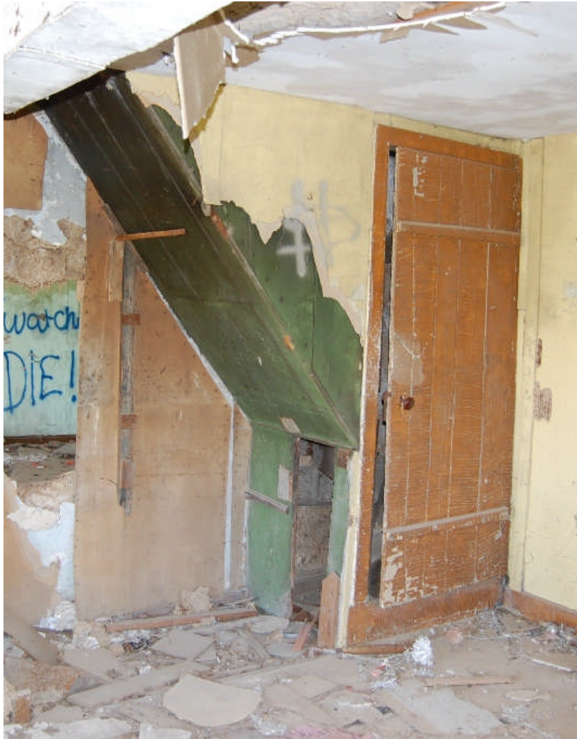
Figure 46. Two views of the enclosed stairway in the southwest corner of Room 100 leading to the upper story. The stairway is enclosed with planking, and the door is framed of vertical planks as well. The area beneath the stairway proper was enclosed with “Beaver Board”—a trade name for a manufactured fiberboard panel—during the first half of the twentieth century and was utilized as a closet.
