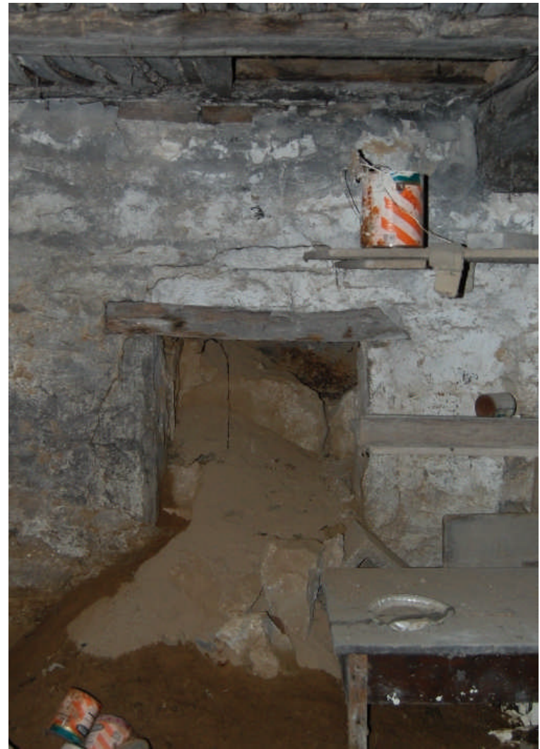
Figure 97. (LEFT) The original cellar entrance door appears to have been hung from hand-forged pintle, one of which is shown here. The existing door is hung with strap hinges. (RIGHT) View of a wall niche on the south side of Room 000. This is one of three once present in the cellar. Such niches have been documented at several other German farmstead in southwest Illinois.
