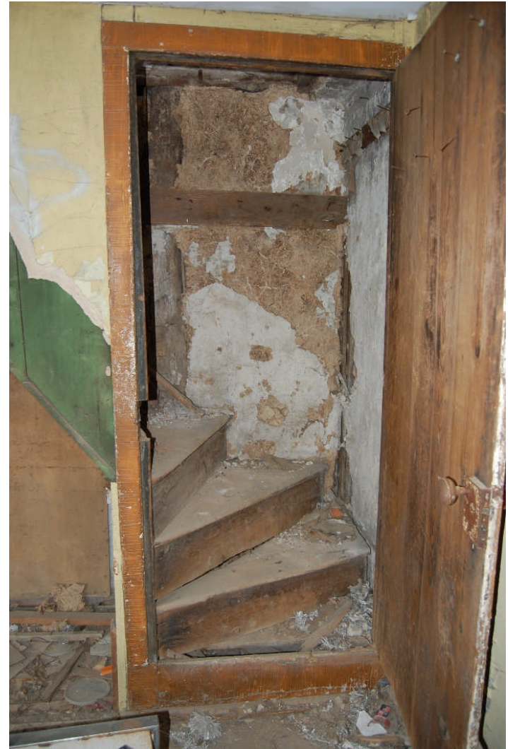
Figure 46. Two views of the enclosed stairway in the southwest corner of Room 100 leading to the upper story. The stairway is enclosed with planking, and the door is framed of vertical planks as well. The area beneath the stairway proper was enclosed with “Beaver Board”—a trade name for a manufactured fiberboard panel—during the first half of the twentieth century and was utilized as a closet.
