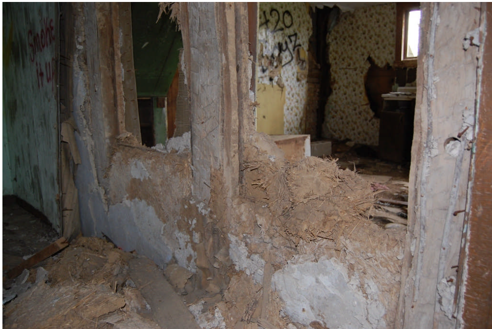
Figure 57. Detail of the partition wall between Rooms 100 and 101, as seen from Room 101. The wall is framed with widely spaced, hand-hewn, oak posts. In contrast to the ceiling joists (which are mitered to accommodate the lath), the posts have small-dimensional (approx. 1"x1") stock nailed to them to hold the lath, around which a straw-and-mud mixture is applied.
