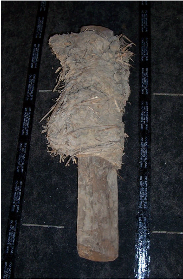
Figure 51. (LEFT) Clay and straw batt from the ceiling in the original house. Note the manner in which the straw and mud has been rolled or wrapped around the oak plank/lath. (RIGHT) Close-up of a hinge and screw from the doorway between Room 100 and 101. The screw is flat-tipped, which indicates a pre-1846 date of manufacture. This helps substantiate the 1846 date inscribed in the plaster above the front entrance door.
