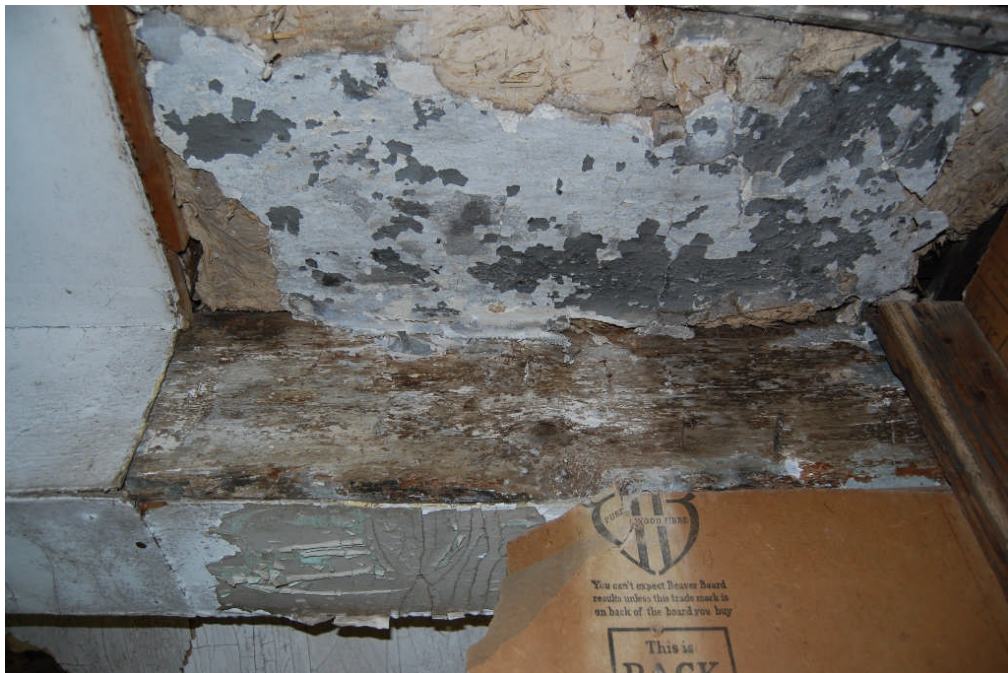
Figure 49. Detail of the central ceiling beam in Room 100. The beam originally was left exposed and whitewashed. It later was covered with Beaver Board.
