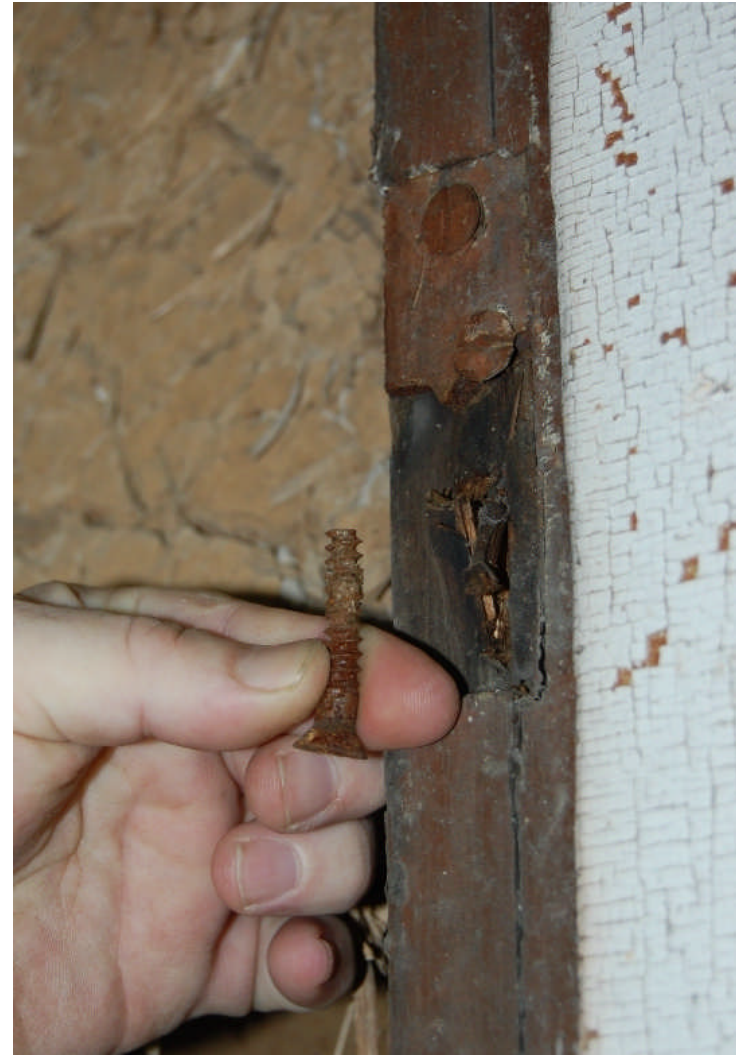
Figure 51. (LEFT) Clay and straw batt from the ceiling in the original house. Note the manner in which the straw and mud has been rolled or wrapped around the oak plank/lath. (RIGHT) Close-up of a hinge and screw from the doorway between Room 100 and 101. The screw is flat-tipped, which indicates a pre-1846 date of manufacture. This helps substantiate the 1846 date inscribed in the plaster above the front entrance door.
