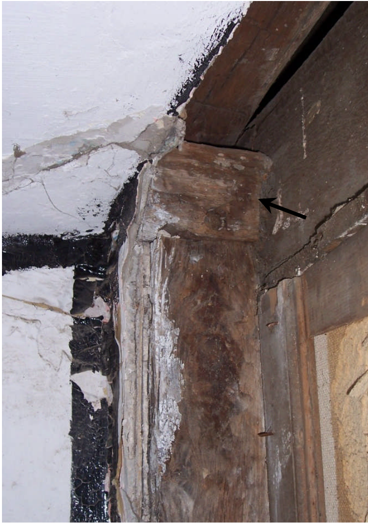
Figure 65. (LEFT) View of a remnant of the original rafter plate from the rear wing of the original house (marked with arrow). This plate was sawn off when the west wall of the wing was pushed outward late in the nineteenth century. The plate and post below it are hand-hewn oak. (RIGHT) View of the southeast corner of Room 102C showing original wall finishes. The walls shown have brick noggin between the framing and are plastered. Note the diagonal bracing.
