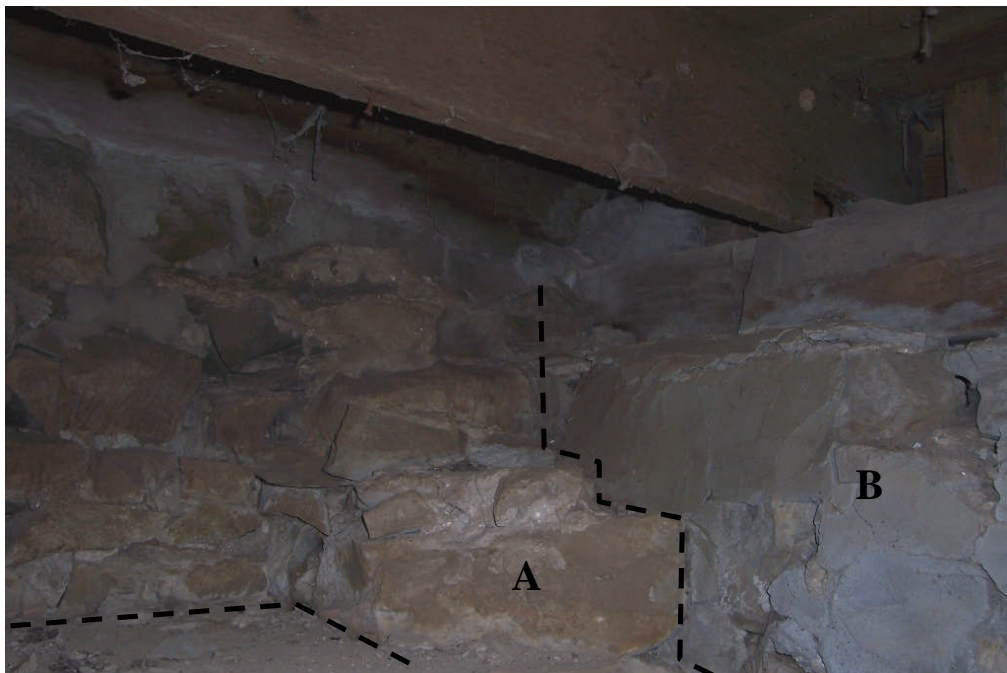
Figure 105. View of the southwest corner of Room 001 showing the remnant of the stone foundations associated with the original frame rear wing, which are marked here by the dashed lines and the “A”. When the west wall of the wing was pushed outward in the late nineteenth century, a new set of stone foundations (“B”) were built below the new wall.
