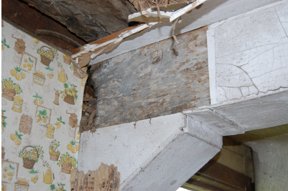
Figure 48. A large hand-hewn, oak summer beam supports the central span of the ceiling joists in Rooms 100 and 101. The image above shows the north end of the beam in Room 100. The diagonal brace was added when the north wall of the original house was rebuilt in the first half of the twentieth century.
