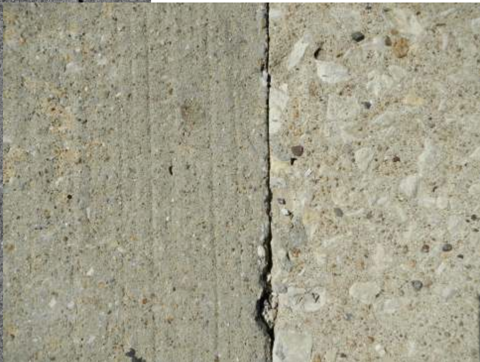
FIG. 31 Blends of cements and pozzolans to create a 'light grey buff tone' cementitious color.
