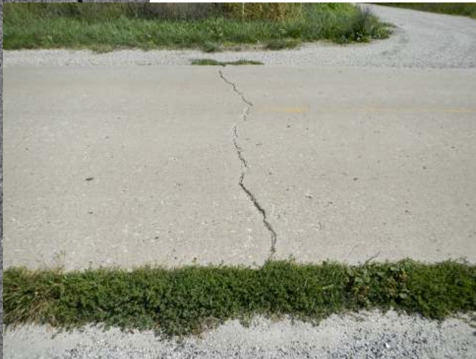
FIG. 1 Concrete in "good" condition (Girard, IL).
