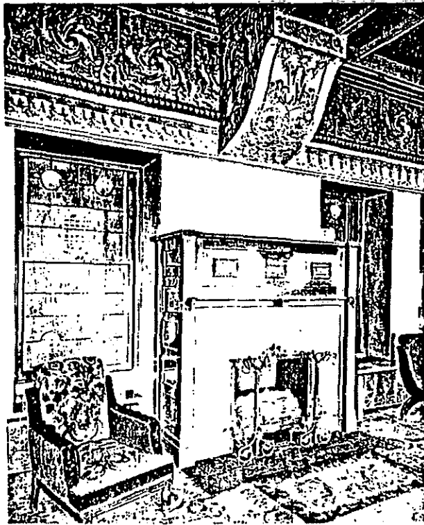
Fireplace – Original Condition
