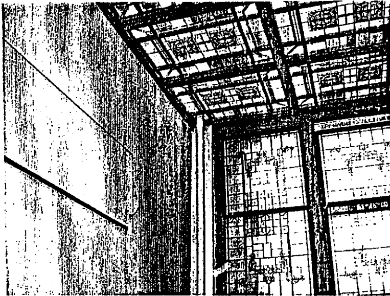
2 nd Floor Mezzanine - Existing Conditions
