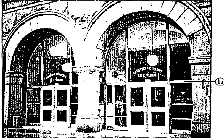
Current condition of exterior facade.
