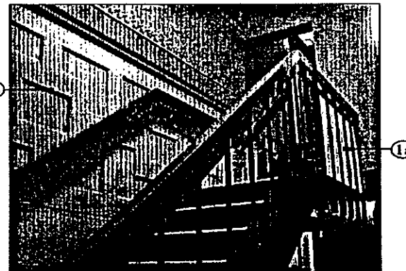
Staircase in north wing.
