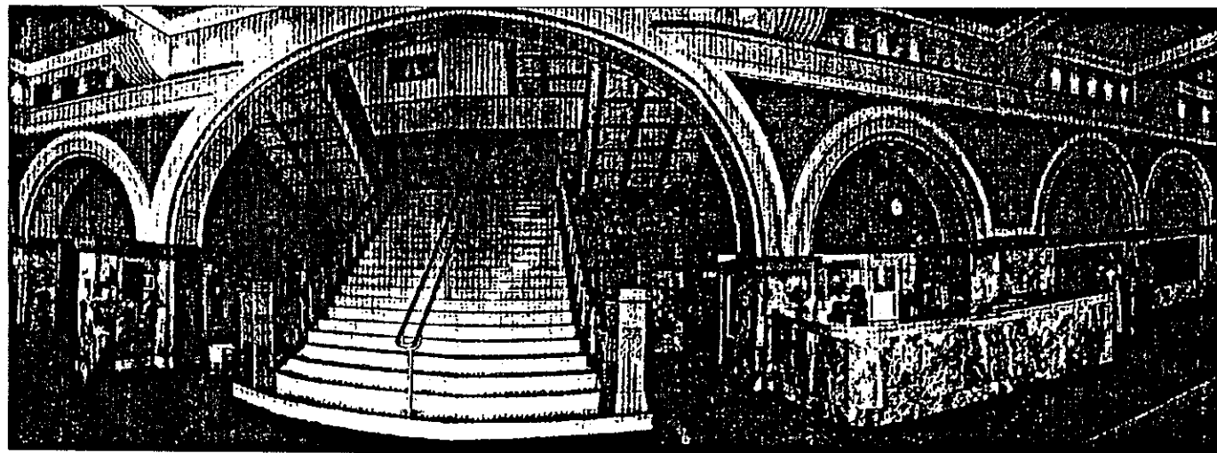
D - View looking West
