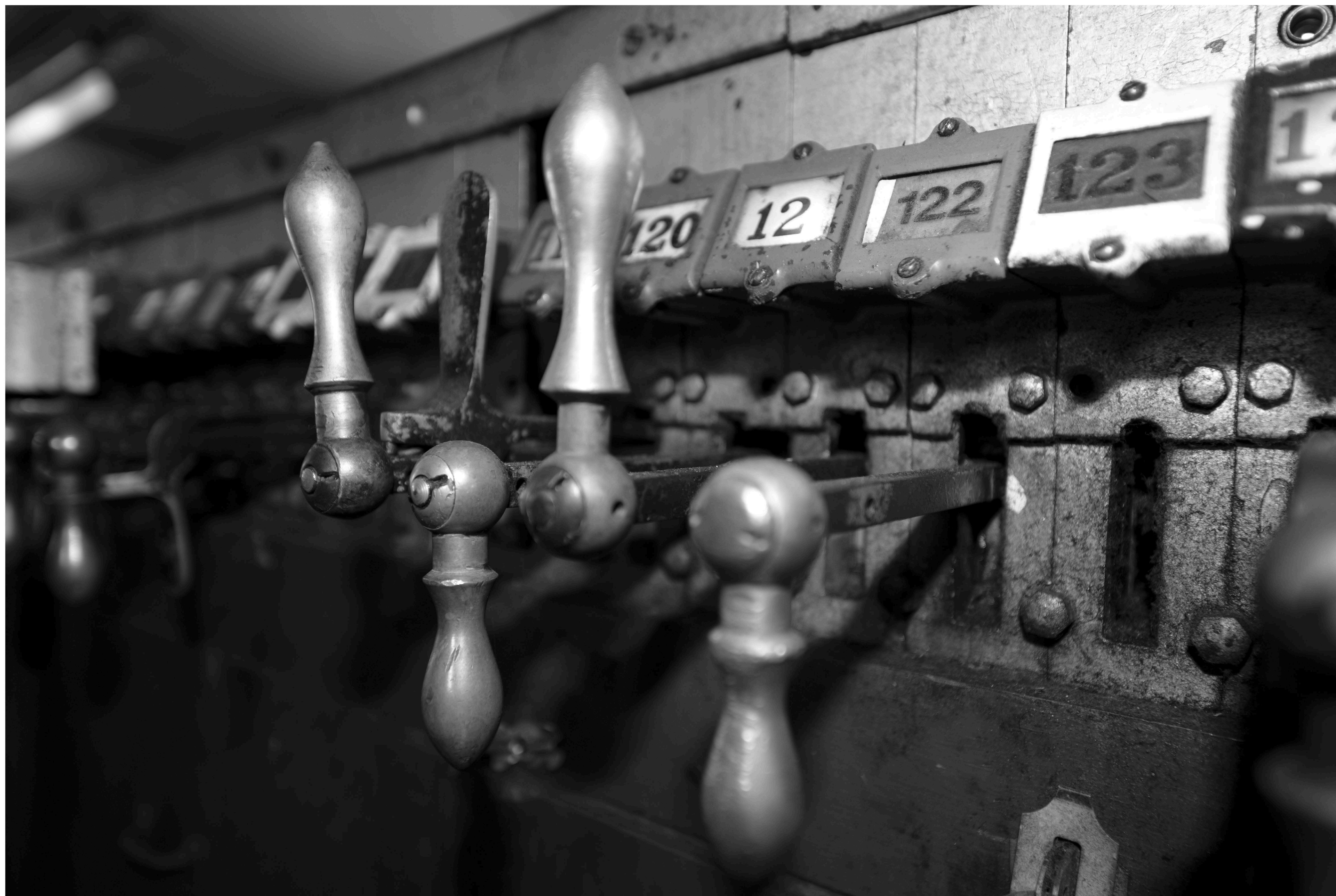
15 of 20 (IL_Cook_16thStreetTower_0015) Detail of 1901 Taylor Model 2 pistol grips, second floor, looking northeast.
