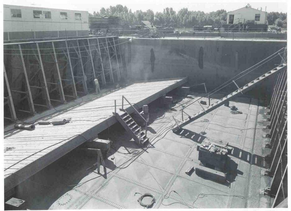
LOUISVILLE DISTRICT, CORPS OF ENGINEERS, U. S. ARMY. Date: 11 September 1951. File No. 25870 Ohio River--Lock & Dam No. 52. Repairs to Bear Traps. Looking upstream and landward from bear trap pier No. 2, showing condition of trap No. 2 prior to repairs.
