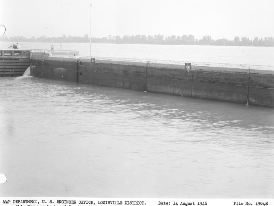
Ohio River -- Lock and Dam No. 52. Lock River Wall. View showing leakage in lock wall.
