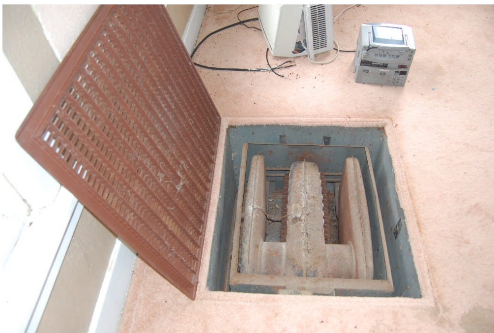
Figure 25. The house was heated with two floor furnaces, one of which was located in the living room (shown above) and the other in the dining room.
