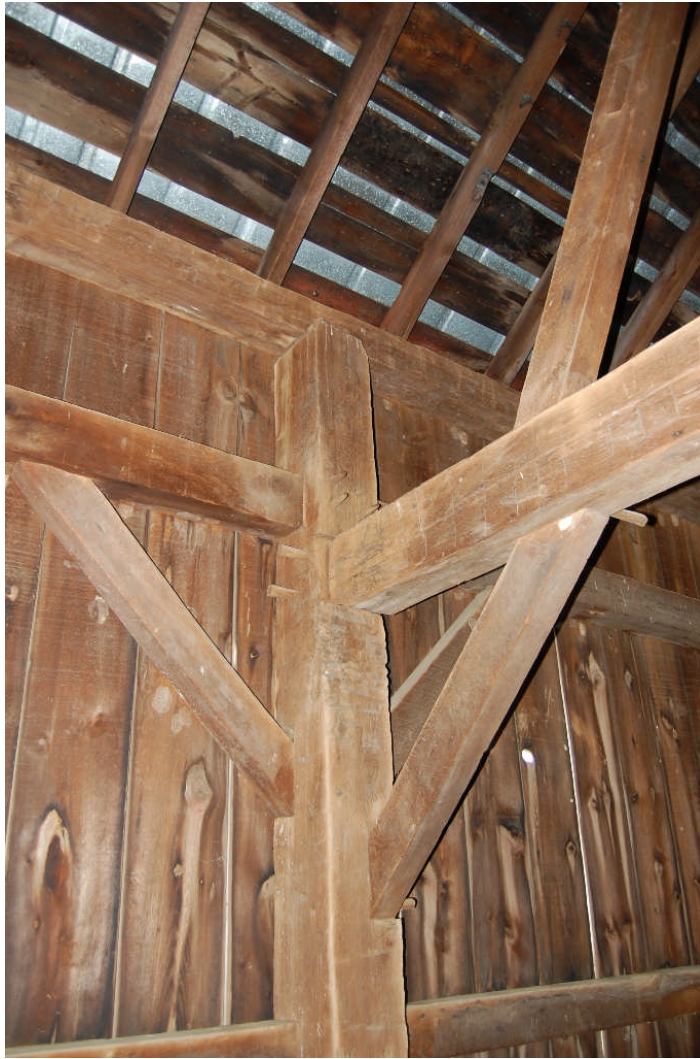
Figure 50. Detail views of the junction between the post and upper girt of one of central bents in the barn, illustrating character of framing and mortise-and-tenon construction. The sills, posts, girts, and rafter plate are hand-hewn oak, while the rails (or nailers) are circular-sawn white pine.
