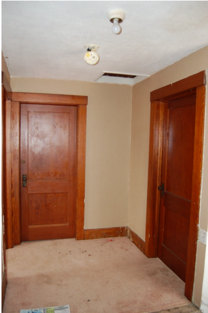
Figure 32. (LEFT) View of the second-floor hallway in the house looking west. Note character of two-panel doors. (RIGHT) The interior doors are hung with half-surface, butt hinges with a brass finish.
