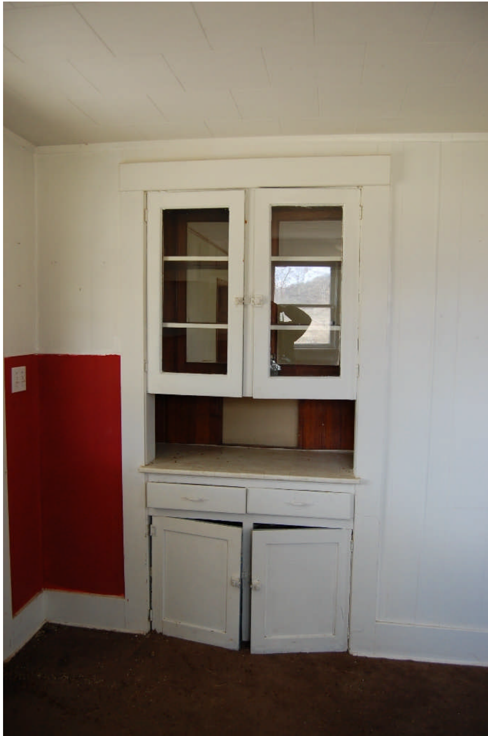
Figure 29. View of the built-in cabinet on the west side of the kitchen. The upper part of the cabinet is accessible from both the kitchen and dining room.
