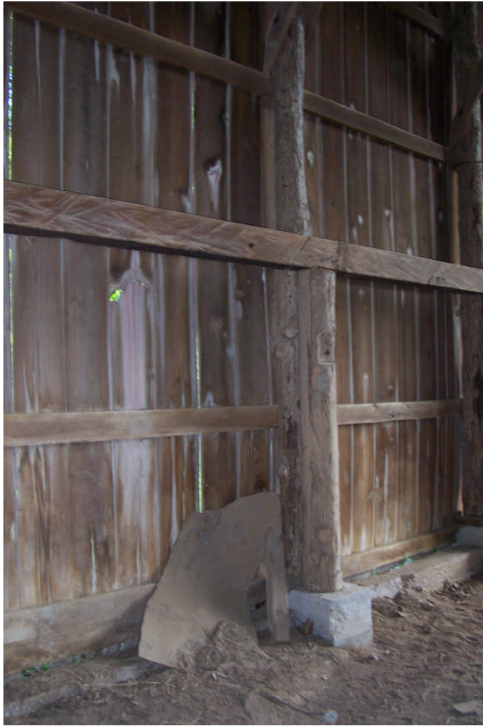
Figure 60. The construction of the feeder barn represents an amalgamation of modern “light” barn construction and vernacular techniques. Locally procured, in-the-round oak posts are used, but these are integrated into the barn structure with industrial methods—bolts and nails—as opposed to traditional mortise and tenon, as illustrated by the two images above. The expansion of the hay loft was accomplished by bolting a second oak post to the original ones and setting a sill plate on top of it. The sill plate for the loft on the east side of the barn appears to have been cut with a chain saw.
