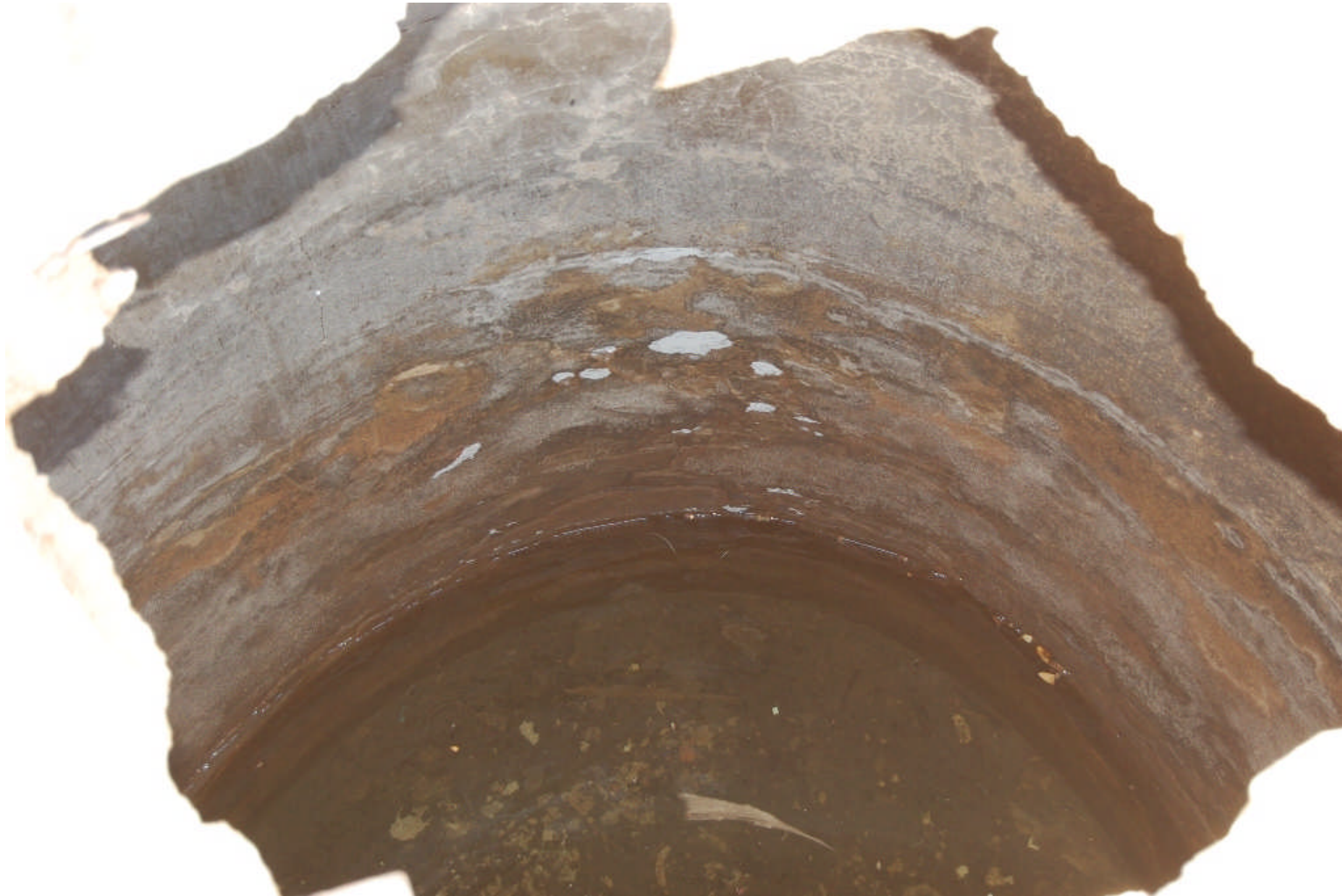
Figure 40. View looking down the concrete-lined cistern located on the east side of the house. The cistern is approximately 6' wide and 9' deep.
