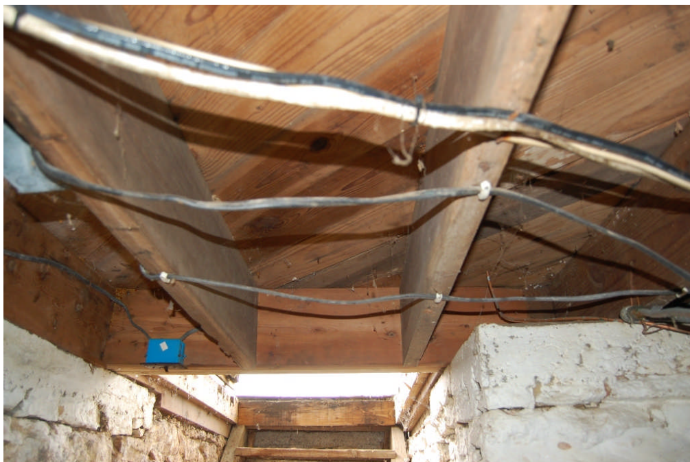
Figure 35. View of the floor framing in the house, as viewed from the cellar. The lumber used in the construction of the house is nominal-sized, fully-surfaced yellow-pine or fir.
