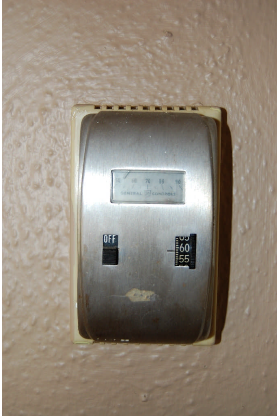
Figure 26. View of the wall thermostat on the east side of the living room. The feature has a sleek, “modern” design and was installed in the early part of the Post-World War II Era. It was during this period of prosperity that the original heating stoves in the house were abandoned in favor of the floor furnaces previously referenced.
