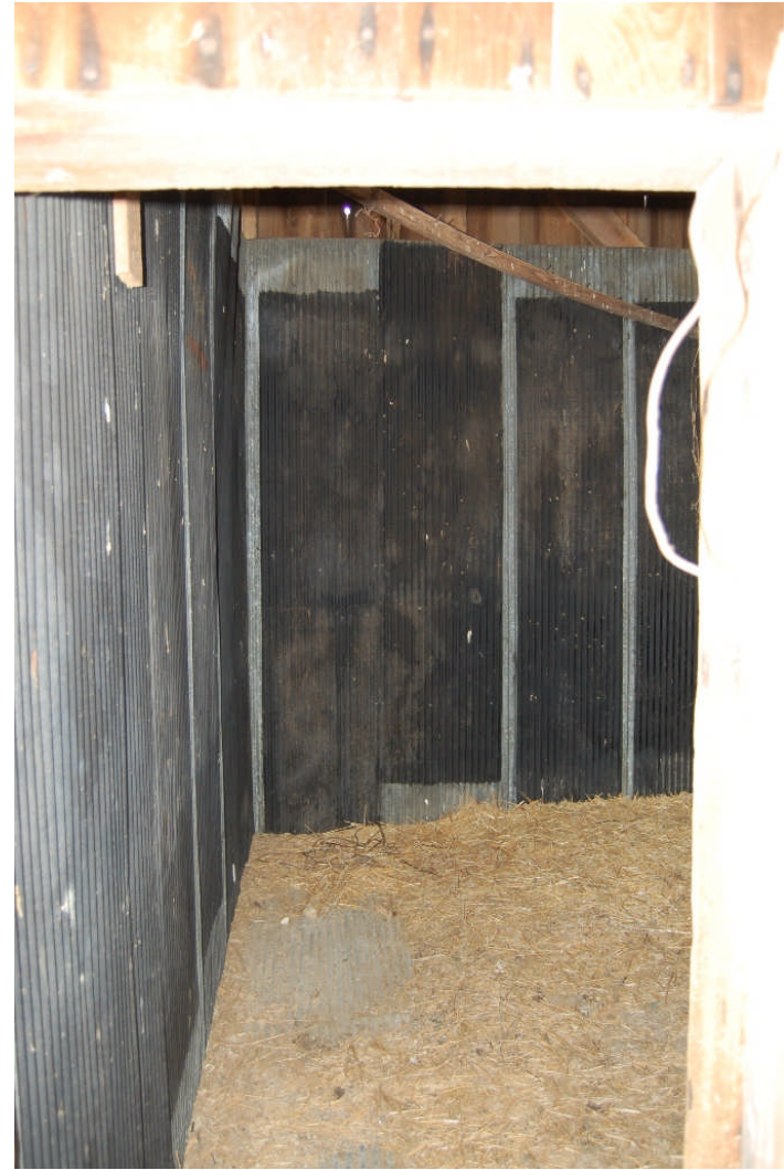
Figure 48. Views of the granary located in the southeast corner of the timber-frame barn. The image at LEFT shows the exterior of the granary, looking southeast. An interior view is shown at RIGHT. The interior walls of the granary are covered with corrugated steel panels.
