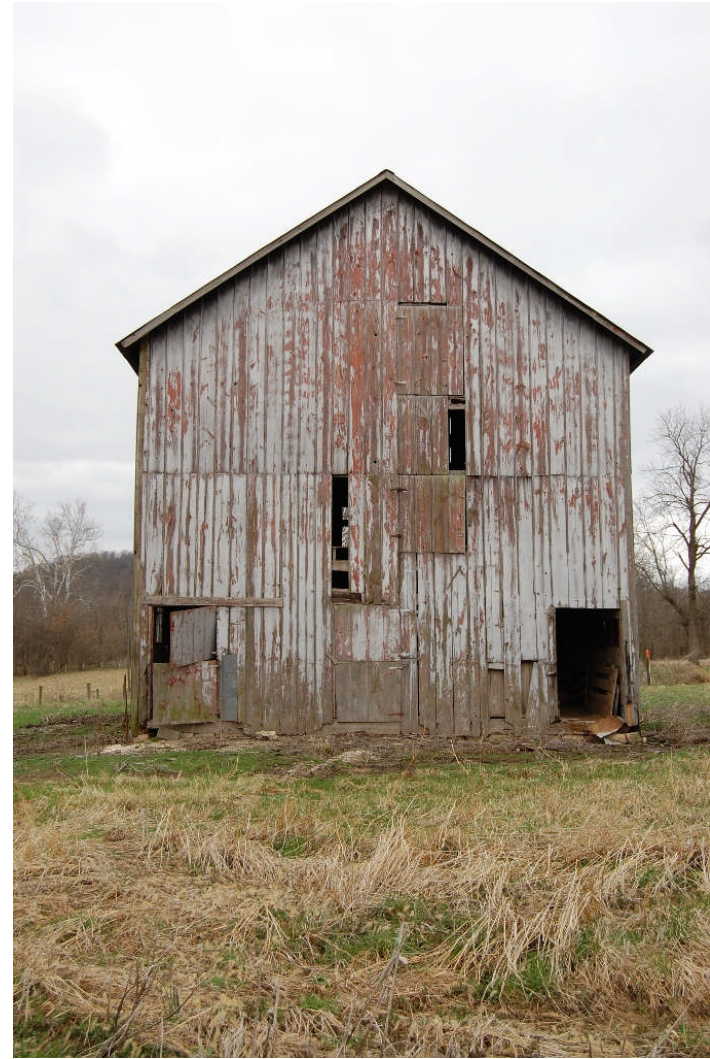
Figure 43. Views the south (Left) and north (RIGHT) gable-end walls of the timber-frame barn. A hay bonnet is present on the south.
