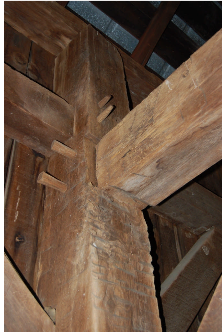
Figure 50. Detail views of the junction between the post and upper girt of one of central bents in the barn, illustrating character of framing and mortise-and-tenon construction. The sills, posts, girts, and rafter plate are hand-hewn oak, while the rails (or nailers) are circular-sawn white pine.
