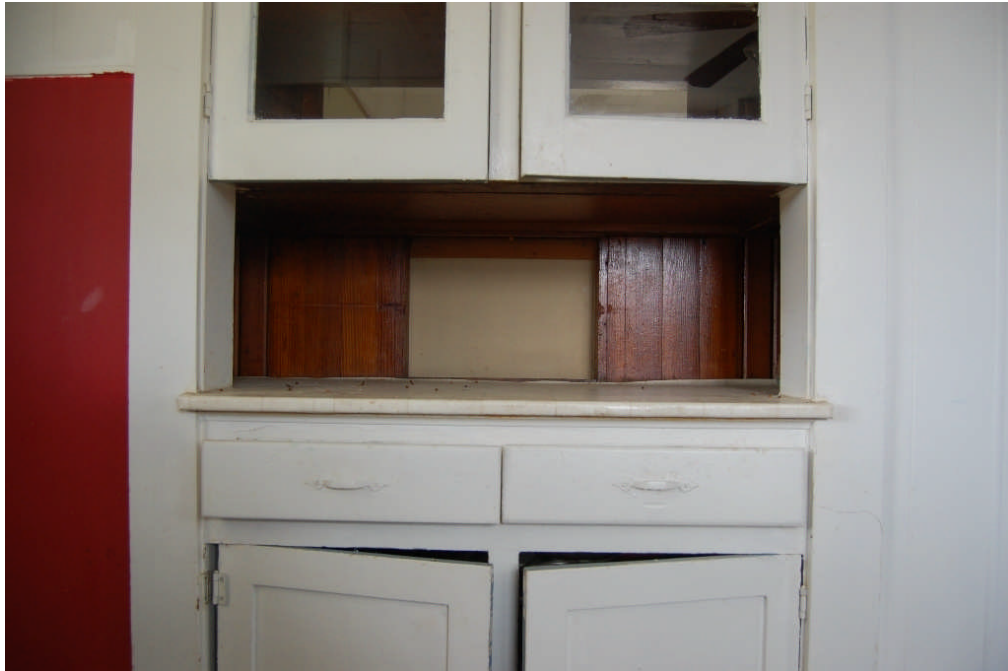
Figure 30. Detail of the built-in cabinet, showing the work counter and associated pass-through window to the dining room. The interior of the upper part of the cabinet is lined with varnished wainscoting.
