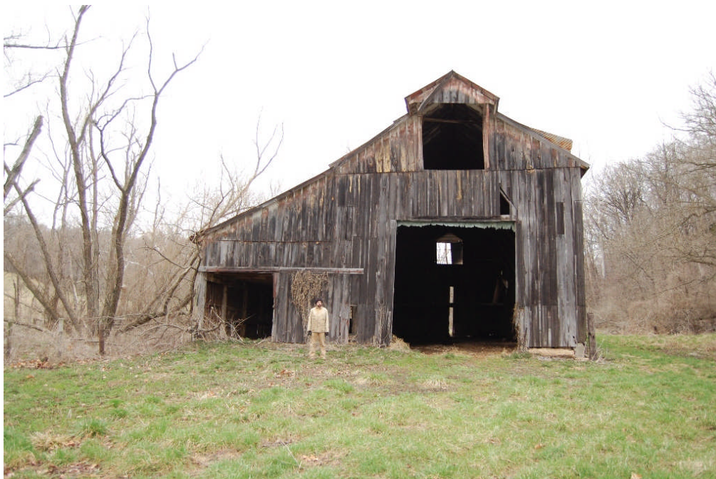
Figure 54. View of the south elevation of the feeder barn at the Belt Farm Site. This structure is located at the mouth of Barn Hollow (perhaps named after this very barn?). Note the wide vehicle door on right and hay bonnet above.
