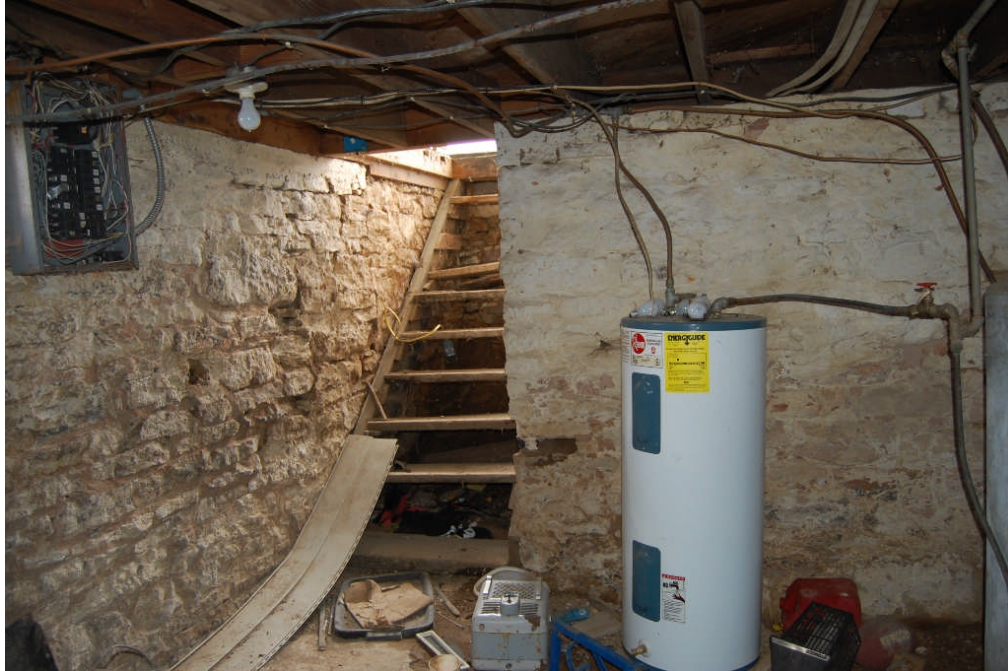
Figure 33. View of the small cellar located beneath the kitchen on the southeast corner of the house. The stone-walled cellar is accessed via the exterior bulkhead stairway shown above. The walls exhibit evidence of fire damage, which presents the possibility of the existing house being second-generation and being built upon the same foundations as an earlier dwelling.
