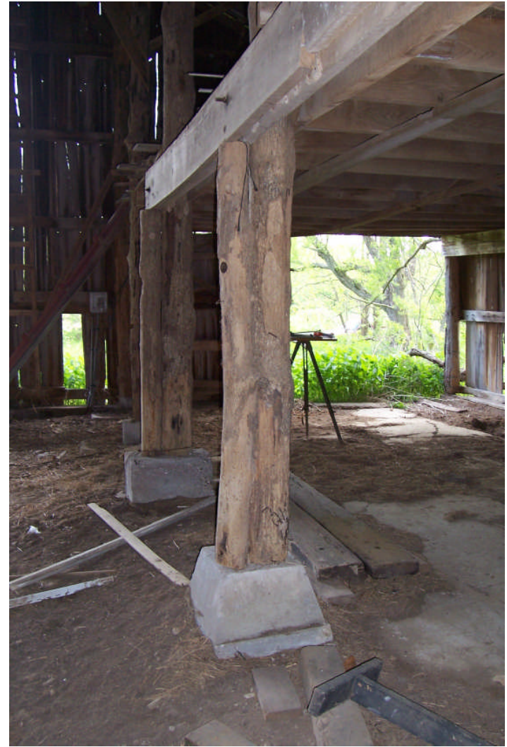
Figure 60. The construction of the feeder barn represents an amalgamation of modern “light” barn construction and vernacular techniques. Locally procured, in-the-round oak posts are used, but these are integrated into the barn structure with industrial methods—bolts and nails—as opposed to traditional mortise and tenon, as illustrated by the two images above. The expansion of the hay loft was accomplished by bolting a second oak post to the original ones and setting a sill plate on top of it. The sill plate for the loft on the east side of the barn appears to have been cut with a chain saw.
