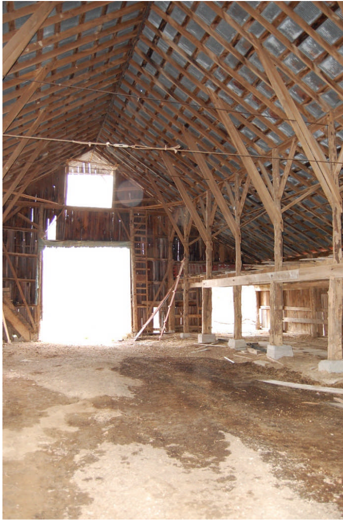
Figure 59. Interior views of the feeder barn, looking south (LEFT) and northwest (RIGHT). The barn was designed to accommodate a large amount of hay, as evidenced by its tall roof and hay bonnets on its gable-end walls. The eastern two-third of the barn was devoted to hay storage originally, while the western third was partitioned up into livestock stalls. Note the diagonal bracing supporting the roof.
