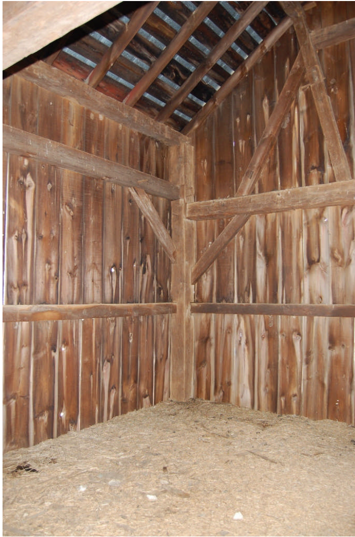
Figure 51. Details of the framing in the northwest (LEFT) and southwest (RIGHT) corners of the upper level of the barn. The timber frame remains in excellent condition, except on the southwest corner, where some damage has occurred due to roofing having blown off.
