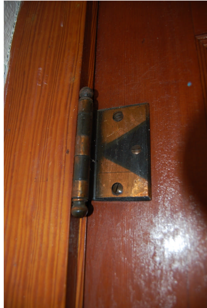
Figure 32. (LEFT) View of the second-floor hallway in the house looking west. Note character of two-panel doors. (RIGHT) The interior doors are hung with half-surface, butt hinges with a brass finish.
