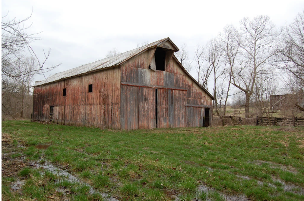
Figure 56. View of the feeder barn, looking southwest and showing the east and north elevations. The north elevation essentially mirrors that on the south, featuring a wide vehicle door and hay bonnet.
