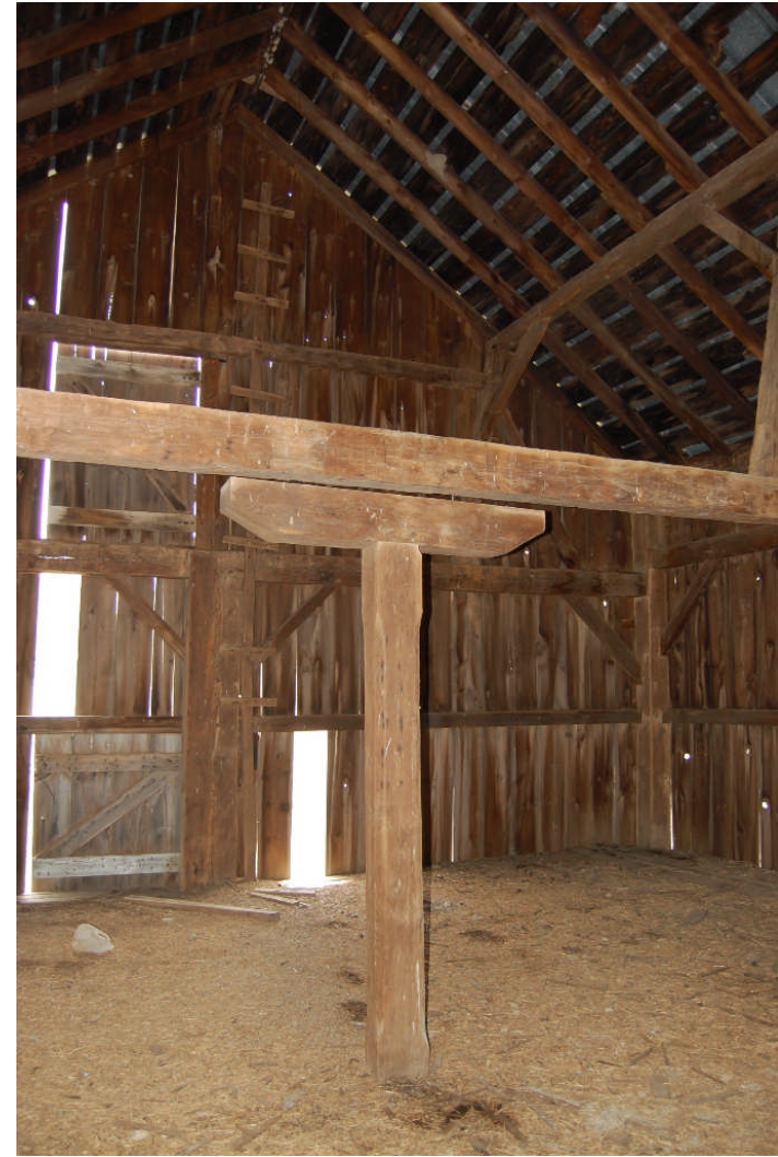
Figure 49. Views of the upper level of the barn, looking northeast (LEFT) and southwest (RIGHT). This level is completely open, aside from the two posts that support the upper girts in the central bents on which the canted queen posts are set. The upper level of the barn was last used as a hay loft. An examination of the framing indicates that a third floor was once present in the building but has been removed. The joists for this removed third floor would have rested on the upper girts shown here.
