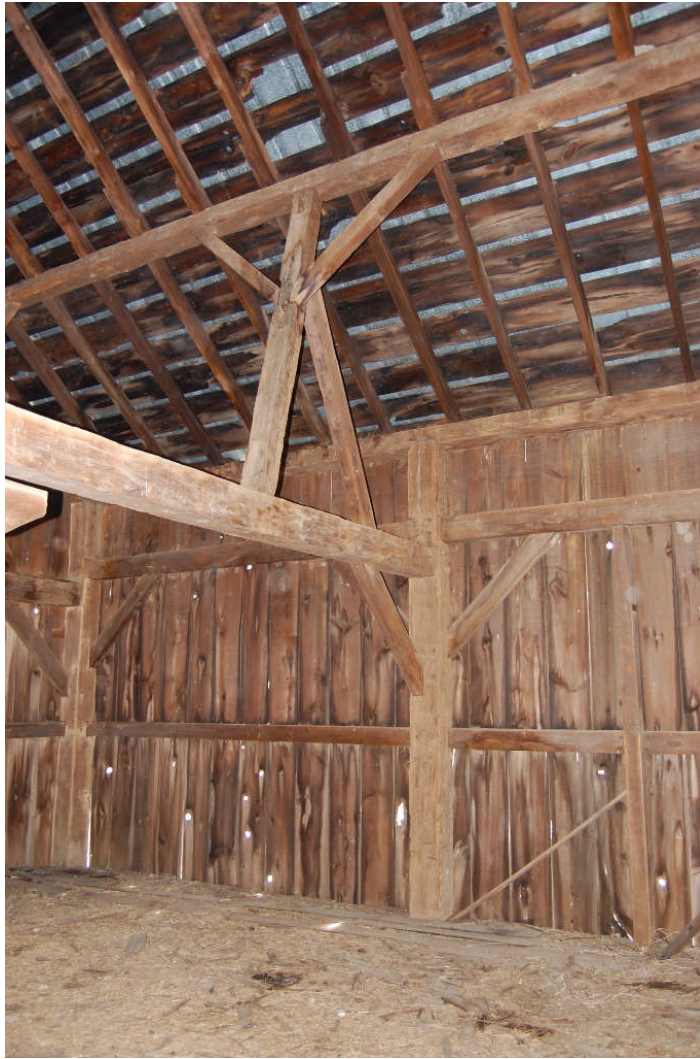
Figure 49. Views of the upper level of the barn, looking northeast (LEFT) and southwest (RIGHT). This level is completely open, aside from the two posts that support the upper girts in the central bents on which the canted queen posts are set. The upper level of the barn was last used as a hay loft. An examination of the framing indicates that a third floor was once present in the building but has been removed. The joists for this removed third floor would have rested on the upper girts shown here.
