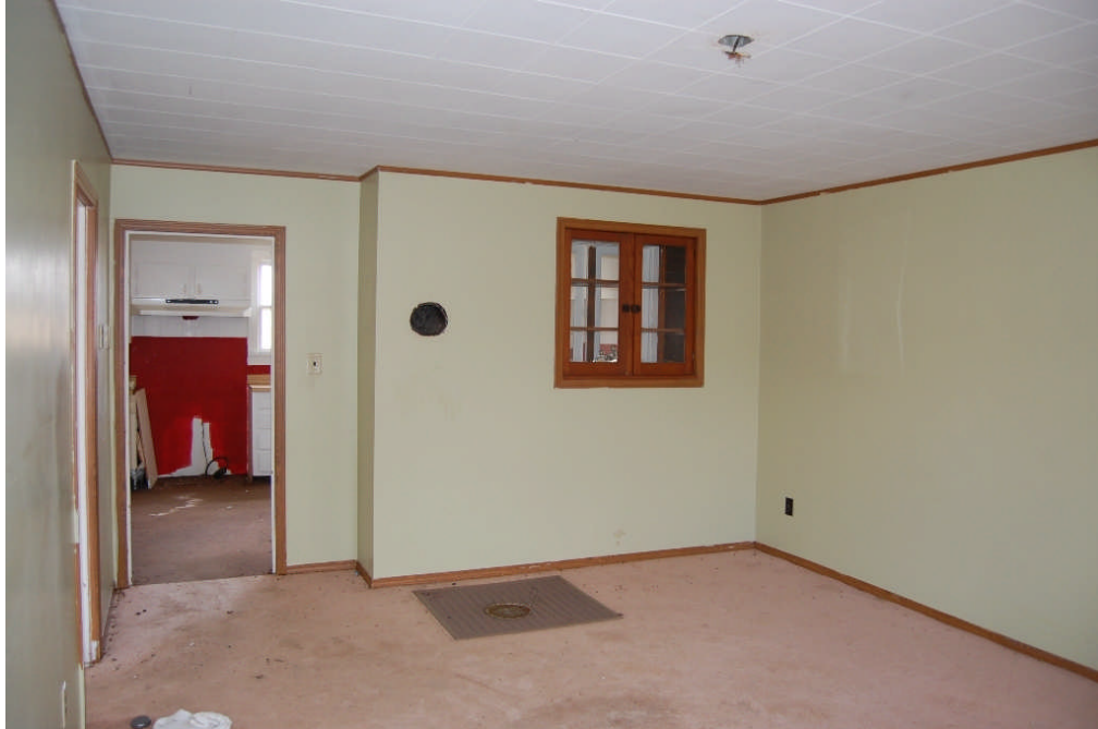
Figure 27. View of the dining room in the house, looking east towards the kitchen. A built-in cabinet is present in the common wall between the dining room and kitchen. A chimney is located along this same wall (note the stove vent to the left of the cabinet). The floor grate shown is associated with the second furnace.
