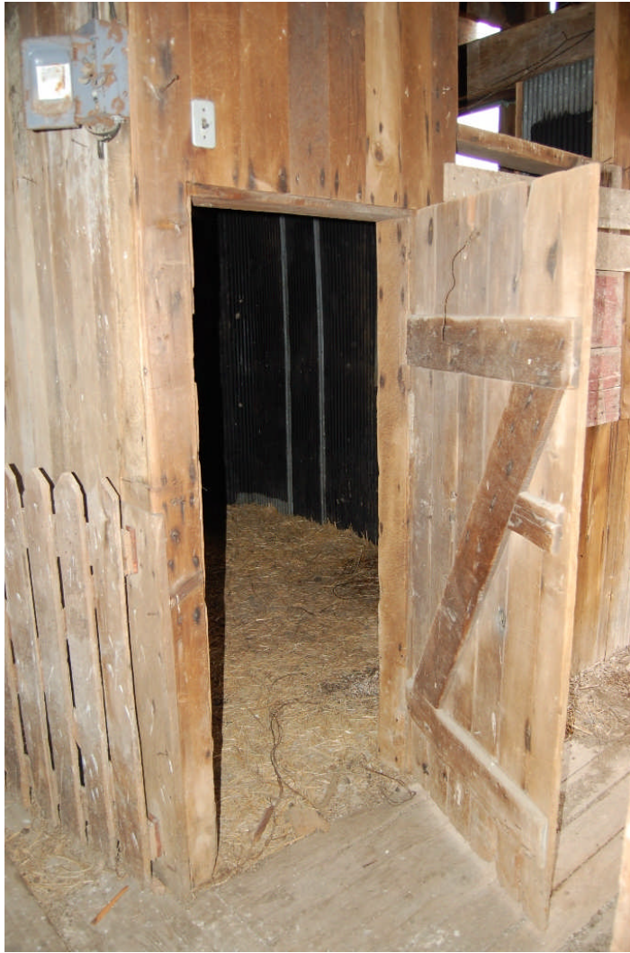
Figure 48. Views of the granary located in the southeast corner of the timber-frame barn. The image at LEFT shows the exterior of the granary, looking southeast. An interior view is shown at RIGHT. The interior walls of the granary are covered with corrugated steel panels.
