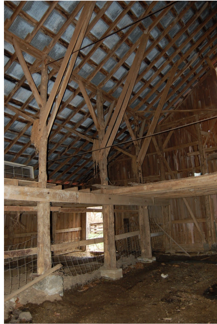
Figure 59. Interior views of the feeder barn, looking south (LEFT) and northwest (RIGHT). The barn was designed to accommodate a large amount of hay, as evidenced by its tall roof and hay bonnets on its gable-end walls. The eastern two-third of the barn was devoted to hay storage originally, while the western third was partitioned up into livestock stalls. Note the diagonal bracing supporting the roof.
