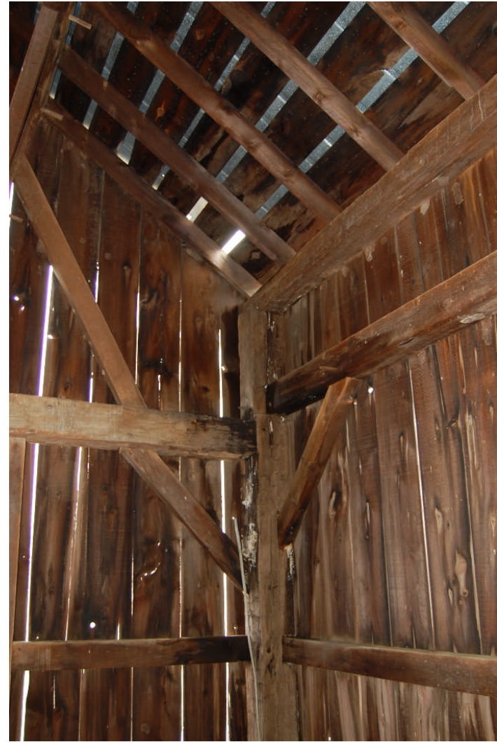
Figure 51. Details of the framing in the northwest (LEFT) and southwest (RIGHT) corners of the upper level of the barn. The timber frame remains in excellent condition, except on the southwest corner, where some damage has occurred due to roofing having blown off.
