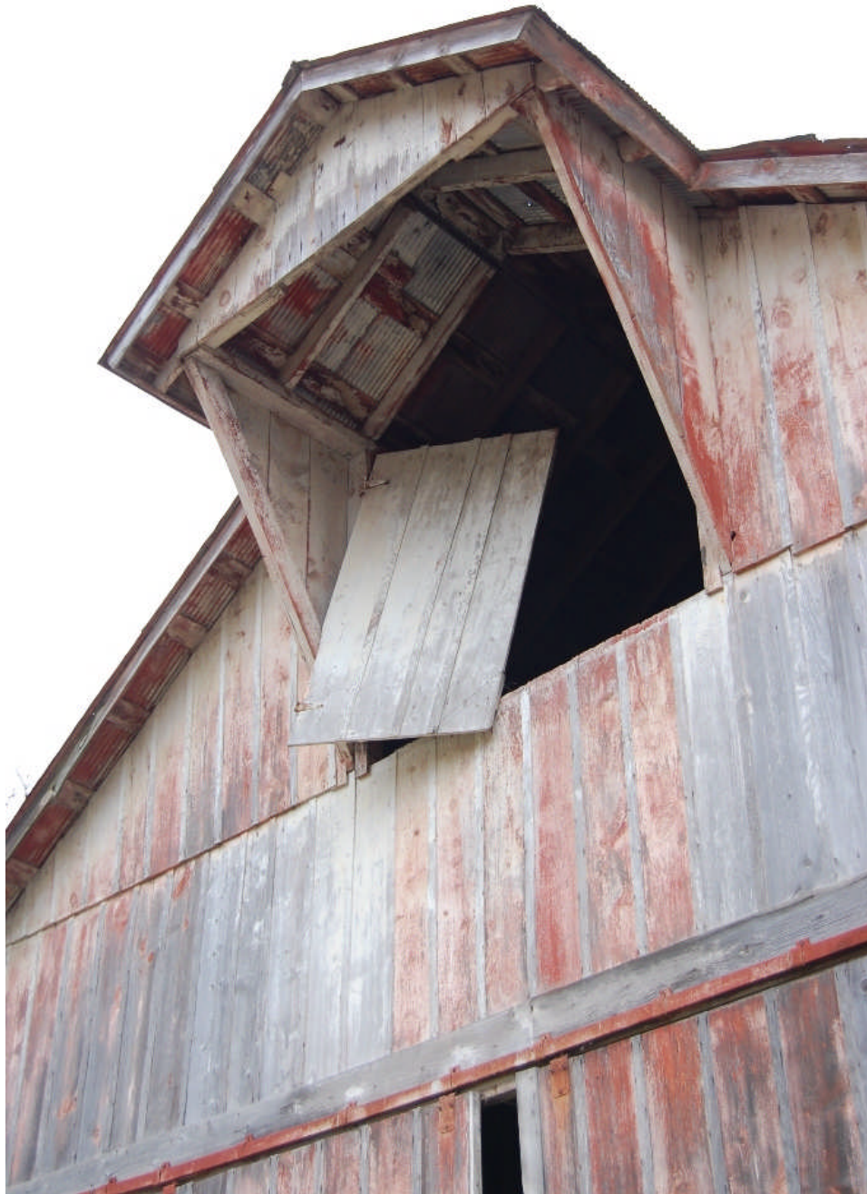
Figure 58. Detail of the hay bonnet on the north side of the feeder barn. Also note the vertical board-and-batten siding.
