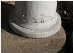
As part of the annual inspection process, Quarters 201 was identified as needing repair to entrance columns. The exterior wood was scraped, areas of deterioration were consolidated and the column was painted. Where excessive decay had occurred, rotted wood was replaced in-kind.
