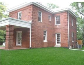
**Enclosed South Porch** – Demolish non-original structure, walls, and windows, retain concrete curbing and brick piers, reconstruct roof, repair and/or replace cedar bead board ceiling and brick paver floor as approved by SHPO. Add compatible wood French door in existing masonry opening to Living Room.
