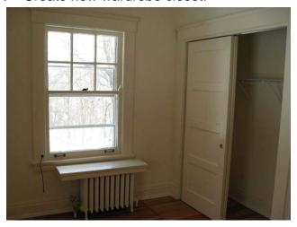
**Bedroom 2 & Enclosed Porch** – Demolish non-original porch enclosure and infill with compatible exterior brick, insert new double wood windows into previous doorway as approved by SHPO, remove wardrobe closet and relocate.
