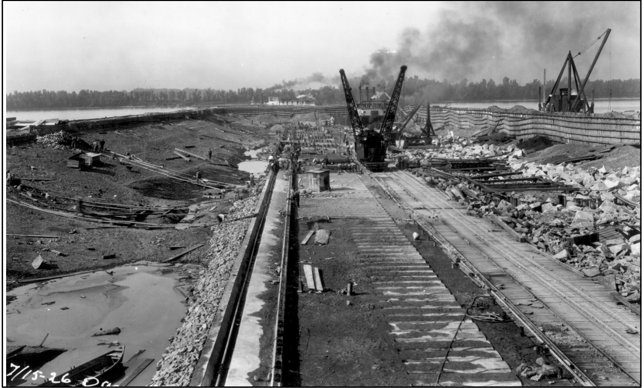
Figure 6. Marine Based Construction Activity at L&D 52, July 1926.
