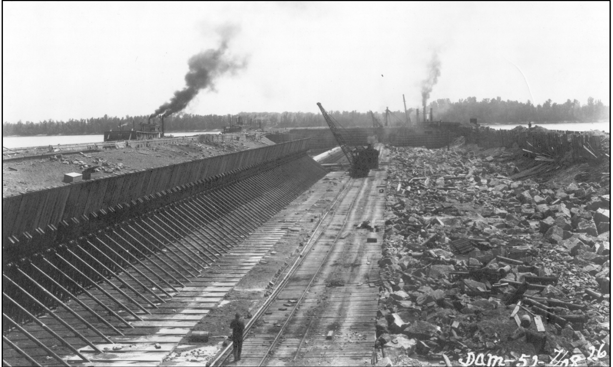
Figure 5. Marine Based Construction Activity at L&D 52, July 1926.
