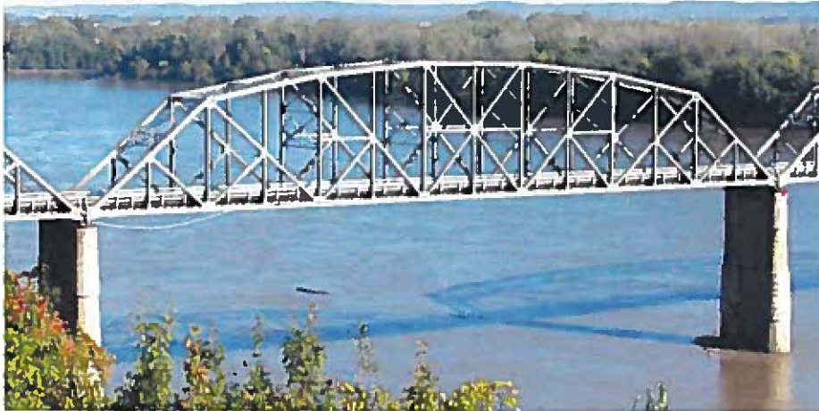
Figure 12: The main channel span of the Champ Clark Bridge, facing northeast
