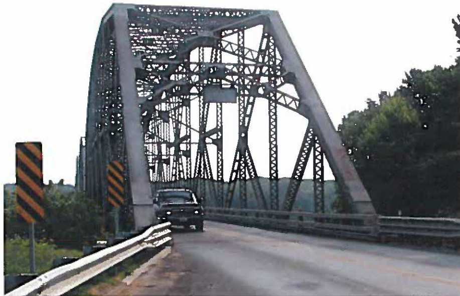
Figure 13: West portal of the Champ Clark Bridge, facing southeast
