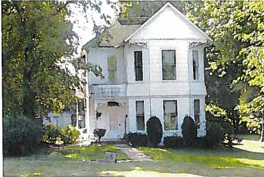
Figure 8: Architectural Resource 40, facing south
