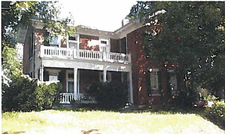
Figure 9: Architectural Resource 41, facing northeast
