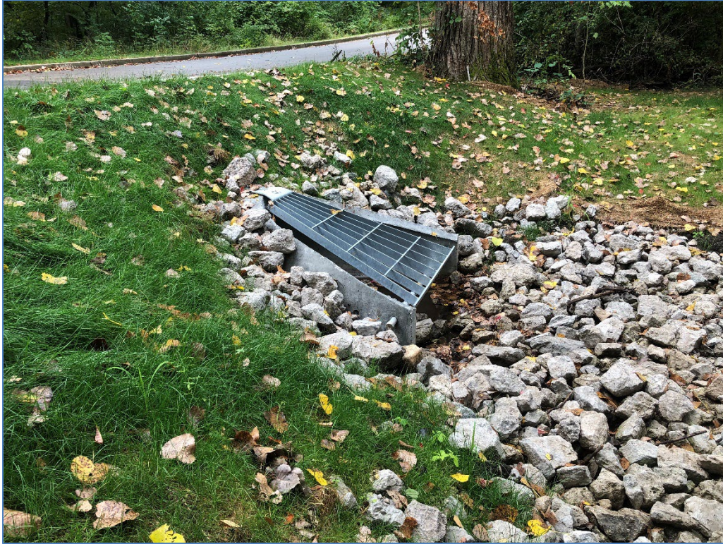
North Side Flared End Section
