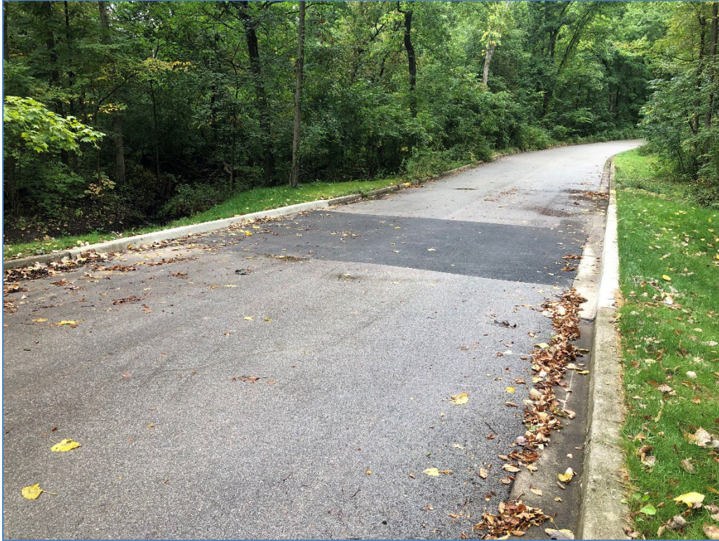
Asphalt Drive above Culvert Repair
