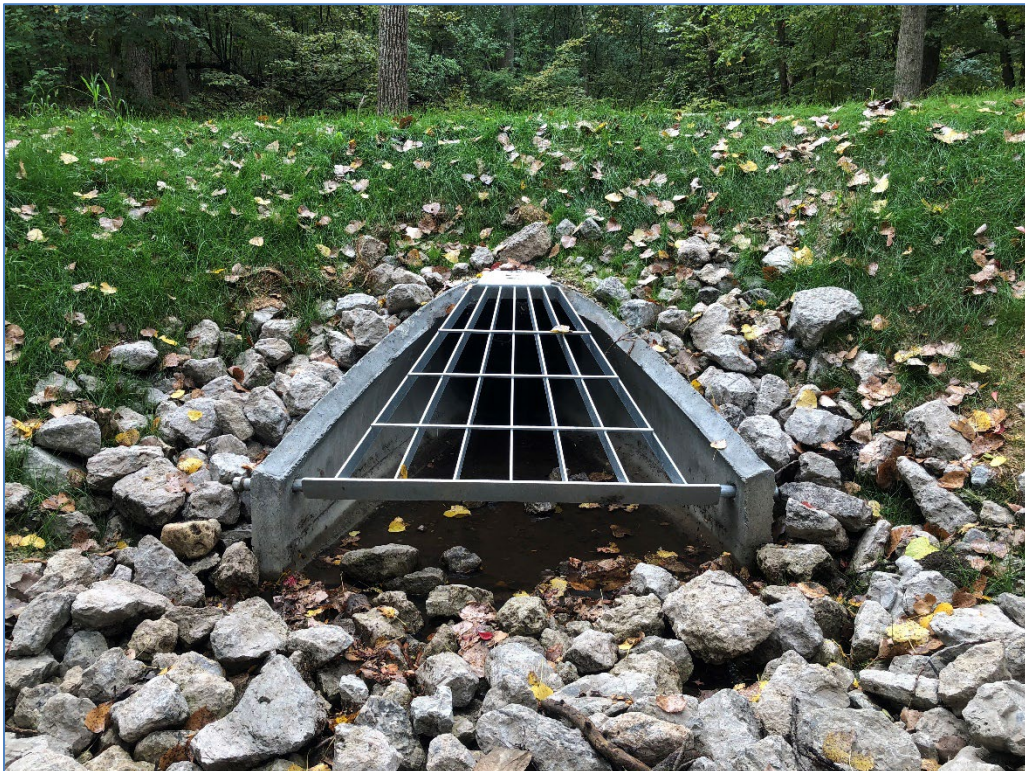
North Side Flared End Section
