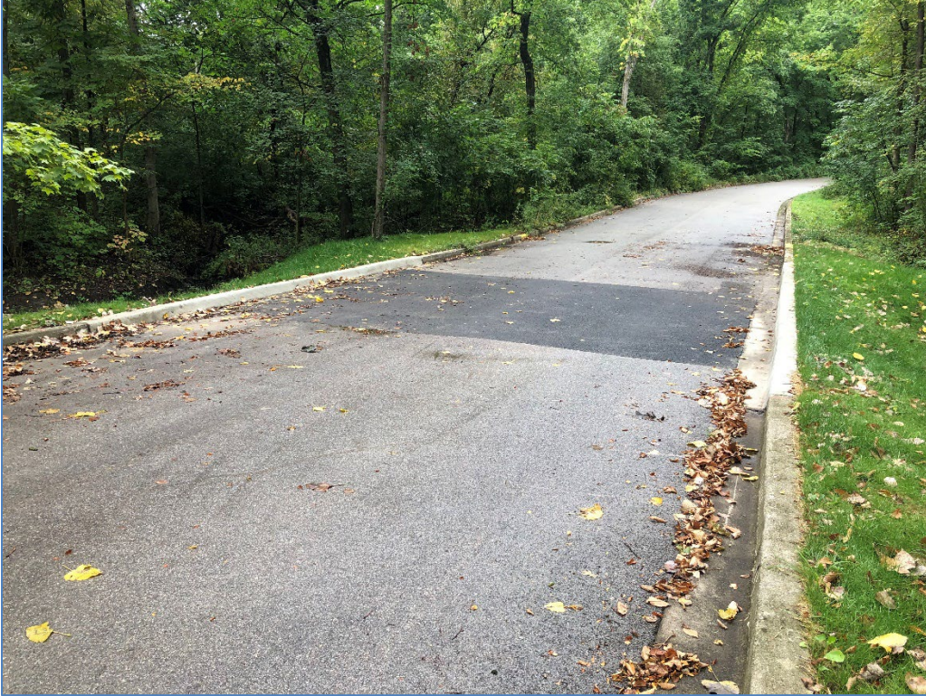
Asphalt Drive above Culvert Repair
