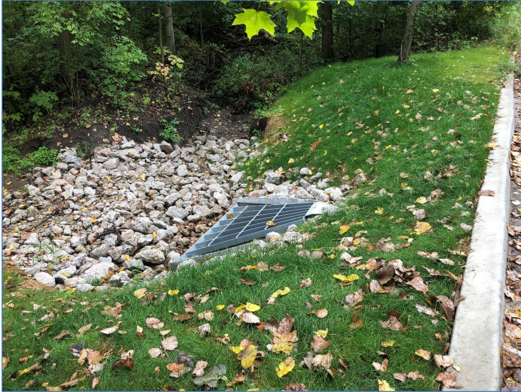
North Side Flared End Section
