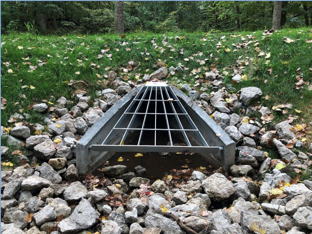
North Side Flared End Section
