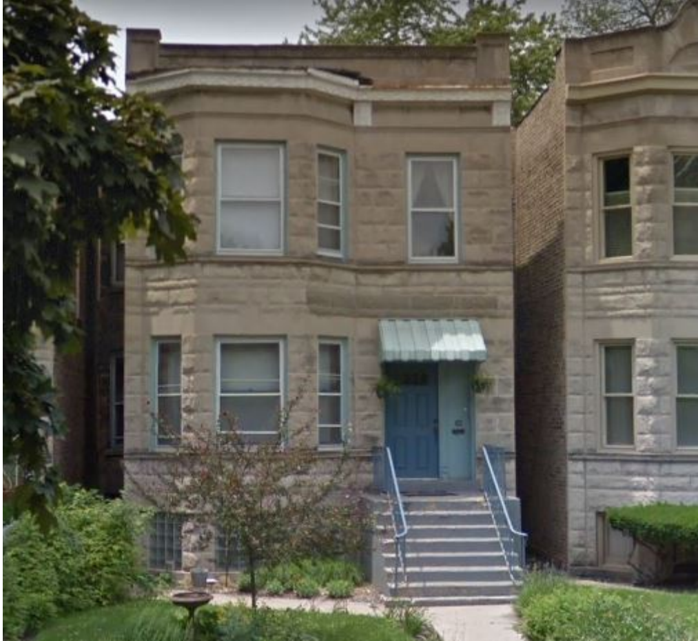
403 N Humphrey Ave 2011 Google Street View image
