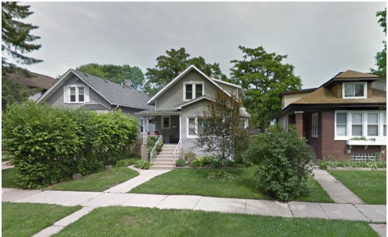
806 Mapleton Ave Google Streetview (2011)
