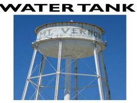
The water tank held 150,000 gallons of water and was 25 feet tall and 34 feet in diameter. It was encircled by a catwalk balcony.
