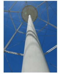
Water for the tank was pumped through this uptake pipe. At the time, the tower was first erected the water came from the adjacent L & N Reservoir. When that source became inadequate to supply the growing city of Mt. Vernon, J.C. Lake and Miller Lake north of Mt. Vernon were constructed. After 1972, the water came from Rend Lake.
