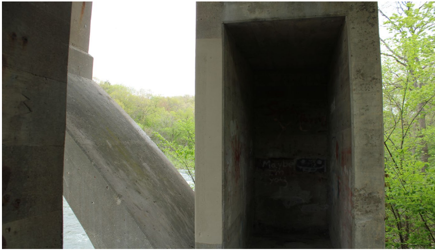
107. Looking East at Patching on S.N. 050-0096 inside East Pier #6
