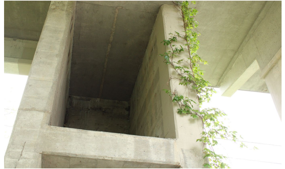
112. Looking West at Patching on S.N. 050-0096 inside West Pier #6
