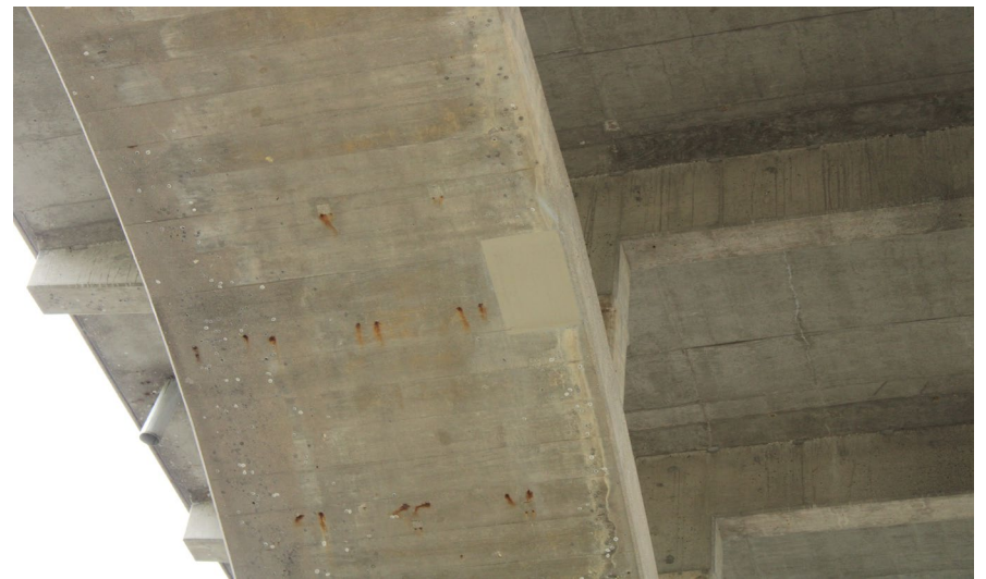
35. Looking East at Patching underneath S.N. 050-0096 East Span #4
