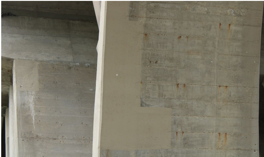
29. Looking North-East at Patching underneath S.N. 050-0096 West Span #4
