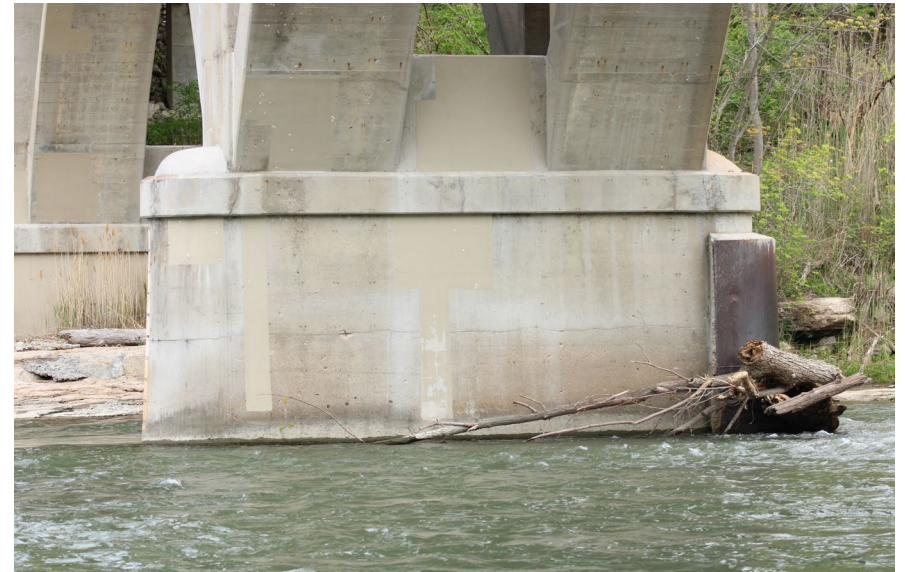
150. Looking North-West at Patching on S.N. 050-0096 South Profile of Pier #4
