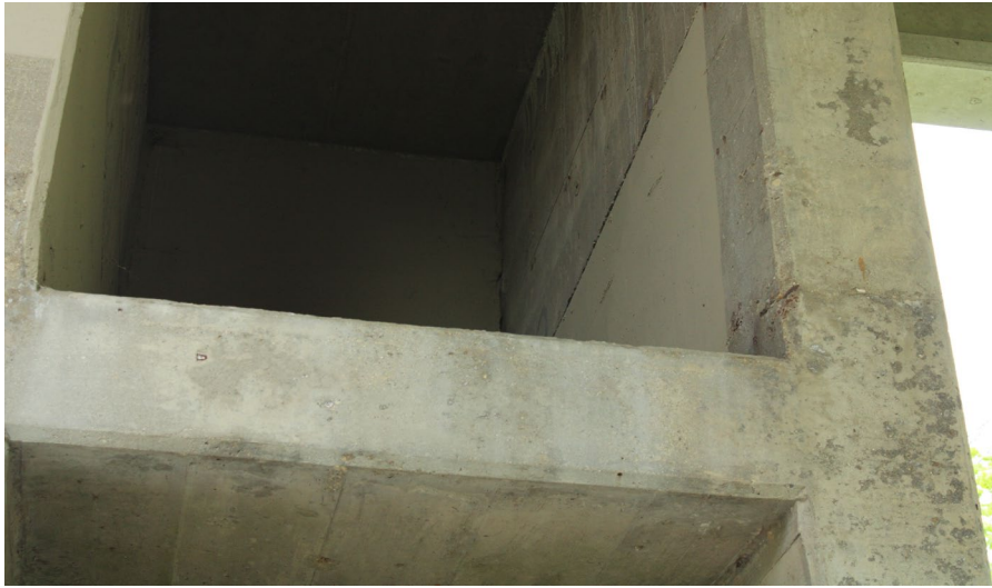
111. Looking East at Patching on S.N. 050-0096 inside East Pier #6
