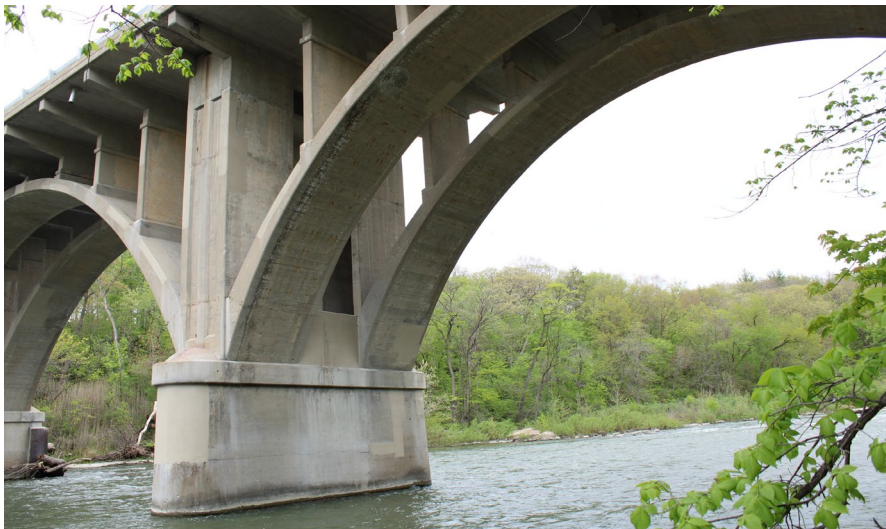
97. Looking North-East at Patching on S.N. 050-0096 underneath Span #6
