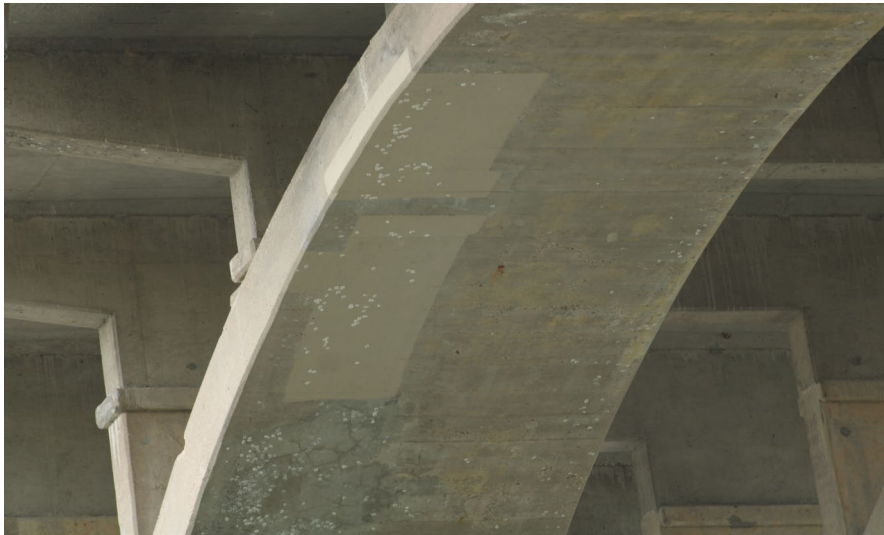
74. Looking South at Patching on S.N. 050-0096 underneath East Span #5
