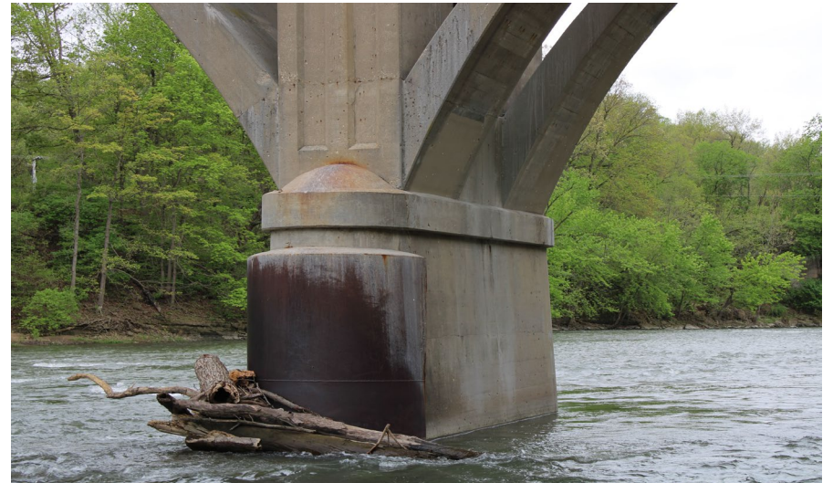
49. Looking West at Patching on S.N. 050-0096 Span #4
