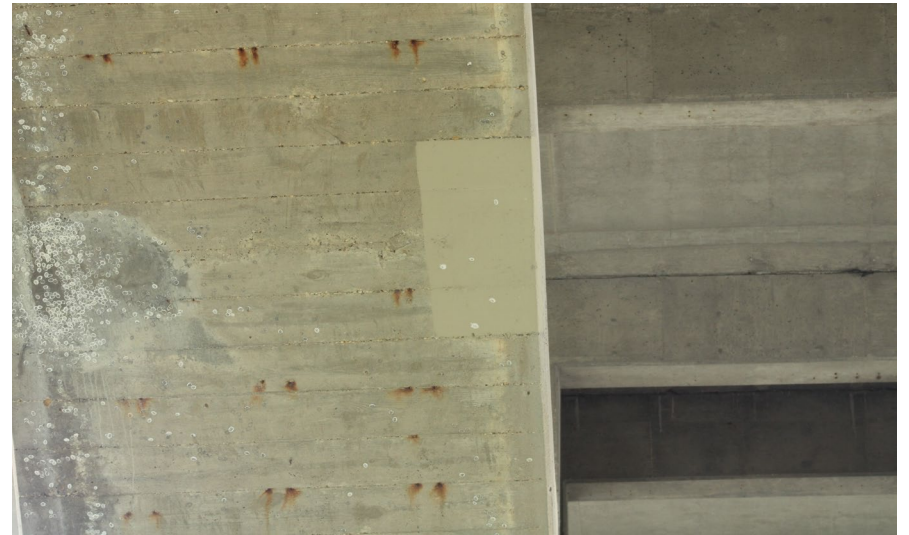
94. Looking North at Patching on S.N. 050-0096 underneath West Span #6
