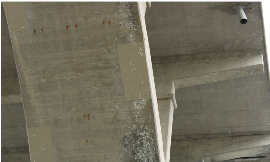
38. Looking South-East at Patching underneath S.N. 050-0096 West Span #4
