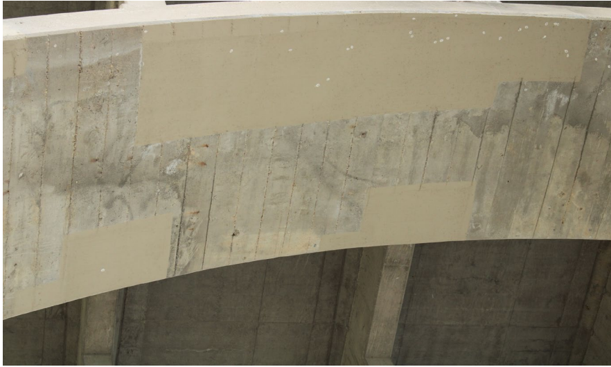
32. Looking East at Patching underneath S.N. 050-0096 West Span #4
