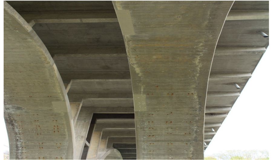
186. Looking North at Patching underneath S.N. 050-0096 Span #6
