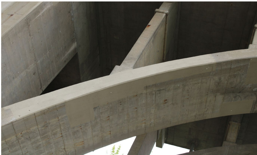
31. Looking East at Patching underneath S.N. 050-0096 West Span #4
