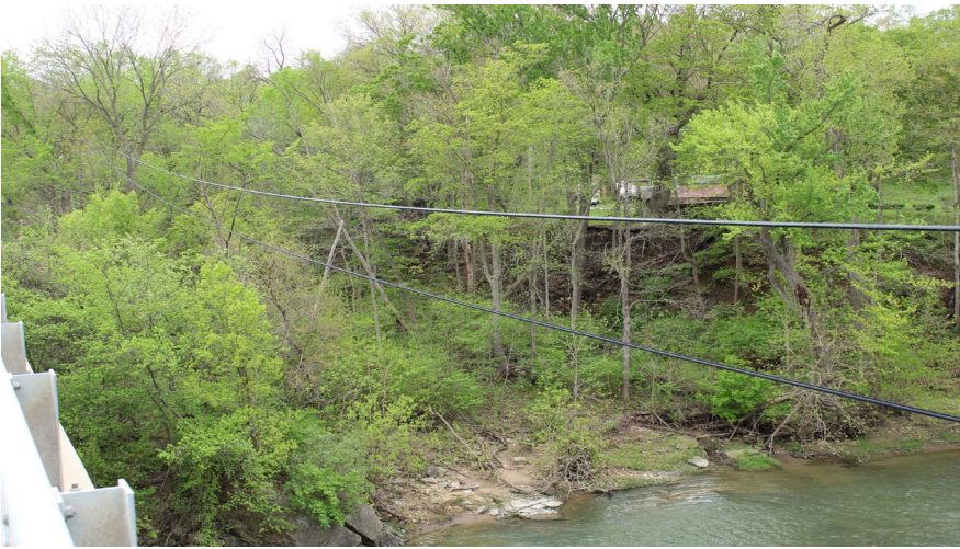
11. Looking South-West at the SW Quad of S.N. 050-0096 at Sta. 196+85
