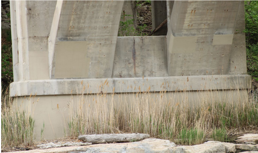
129. Looking North-East at Patching underneath S.N. 050-0096 Span #4
