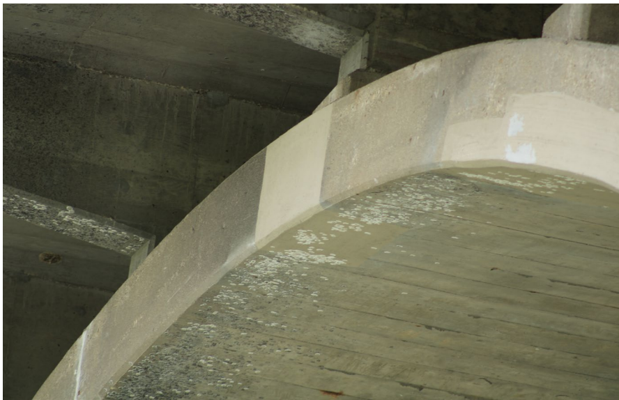
171. Looking North-East at Patching on S.N. 050-0096 West Profile of West Span #5
