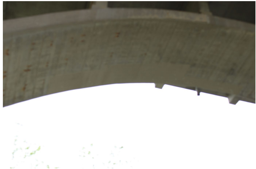
188. Looking West at Patching underneath S.N. 050-0096 West Span #6
