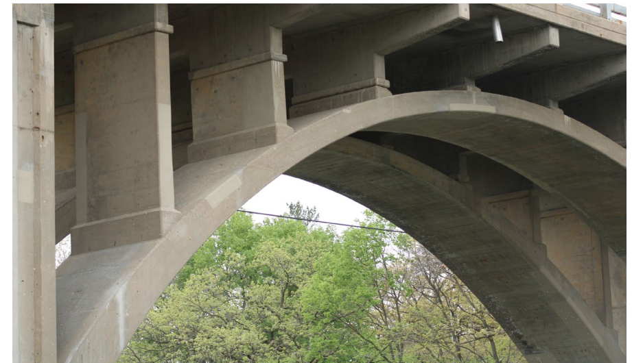
156. Looking North-West at Patching on S.N. 050-0096 East Profile of East Span #5
