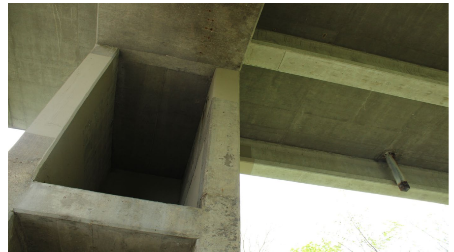
110. Looking East at Patching on S.N. 050-06 inside East Pier #6
