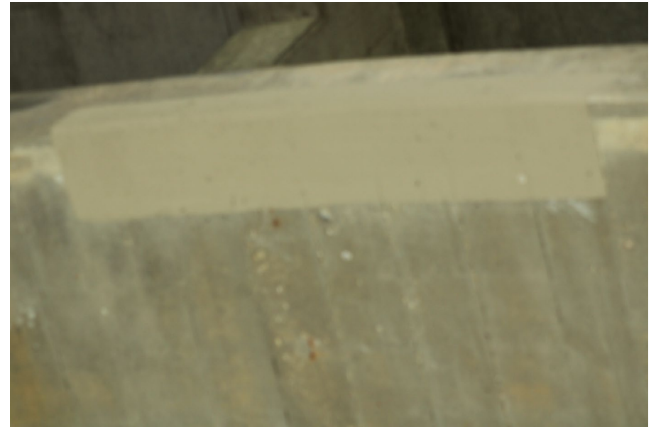
182. Looking directly up at patching underneath S.N. 050-0096 East Span #6
