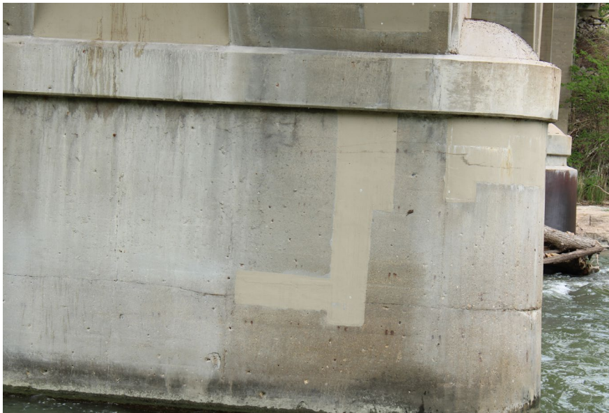
143. Looking North-East at Patching on S.N. 050-0096 South Profile of Pier #5
