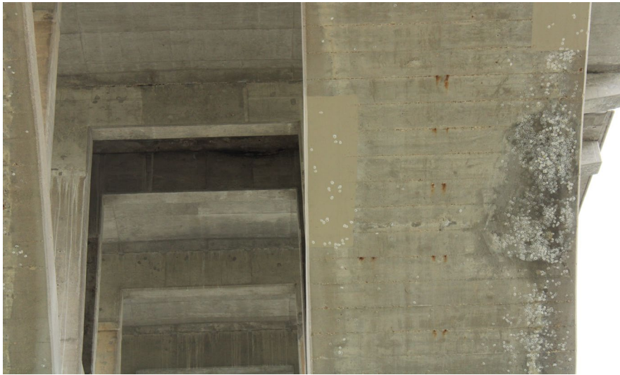
36. Looking South-East at Patching underneath S.N. 050-0096 West Span #4
