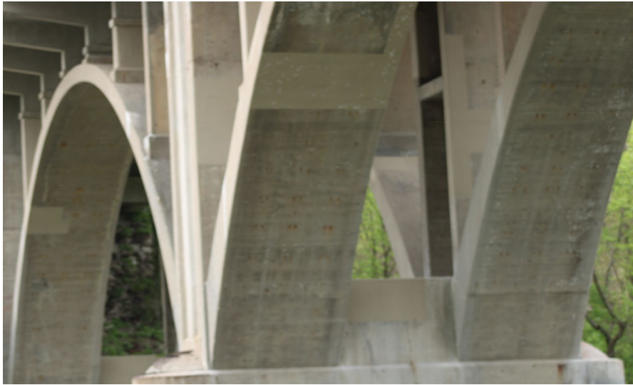
72. Looking South at Patching on S.N. 050-0096 underneath East Span #5
