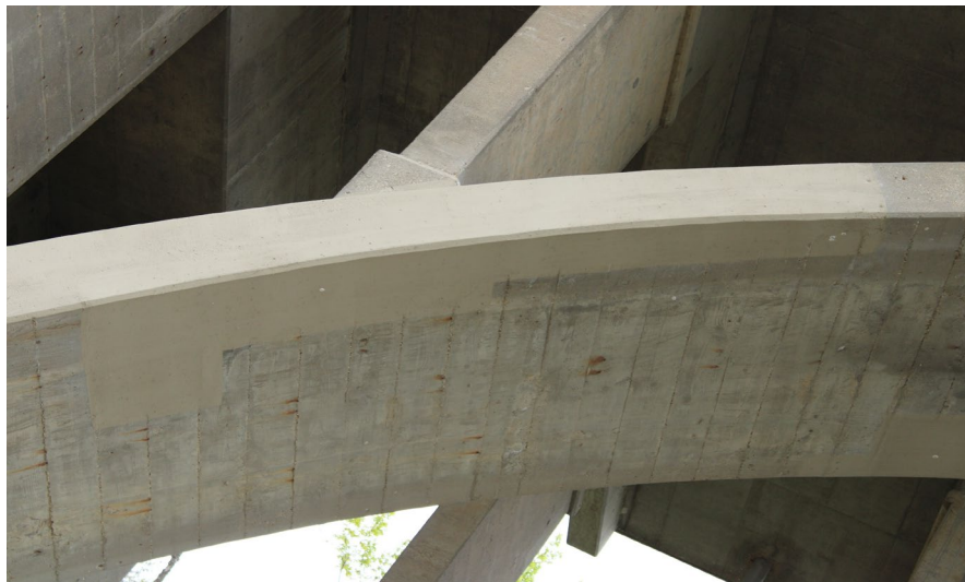
27. Looking East at Patching underneath S.N. 050-0096 West Span #4
