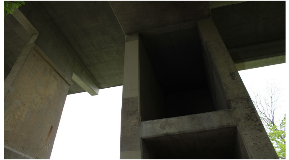
108. Looking East at Patching on S.N. 050-0096 inside East Pier #6
