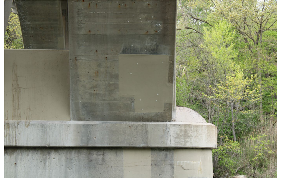
88. Looking North at Patching on S.N. 050-0096 underneath East Span #6
