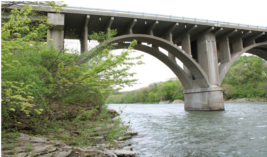
123. Looking West at S.N. 050-0096 East Profile of Span #6
