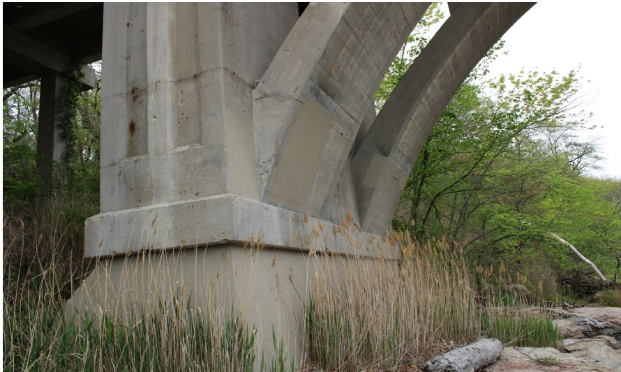
21. Looking North-East at Patching underneath S.N. 050-0096 Span #4
