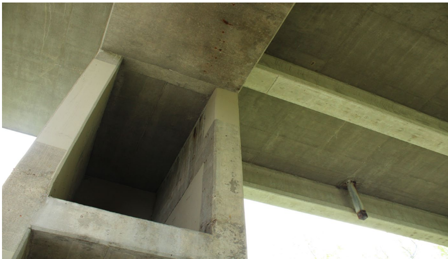
109. Looking East at Patching on S.N. 050-0096 inside East Pier #6
