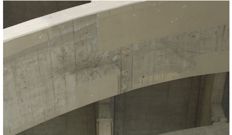
26. Looking East at Patching underneath S.N. 050-0096 West Span #4
