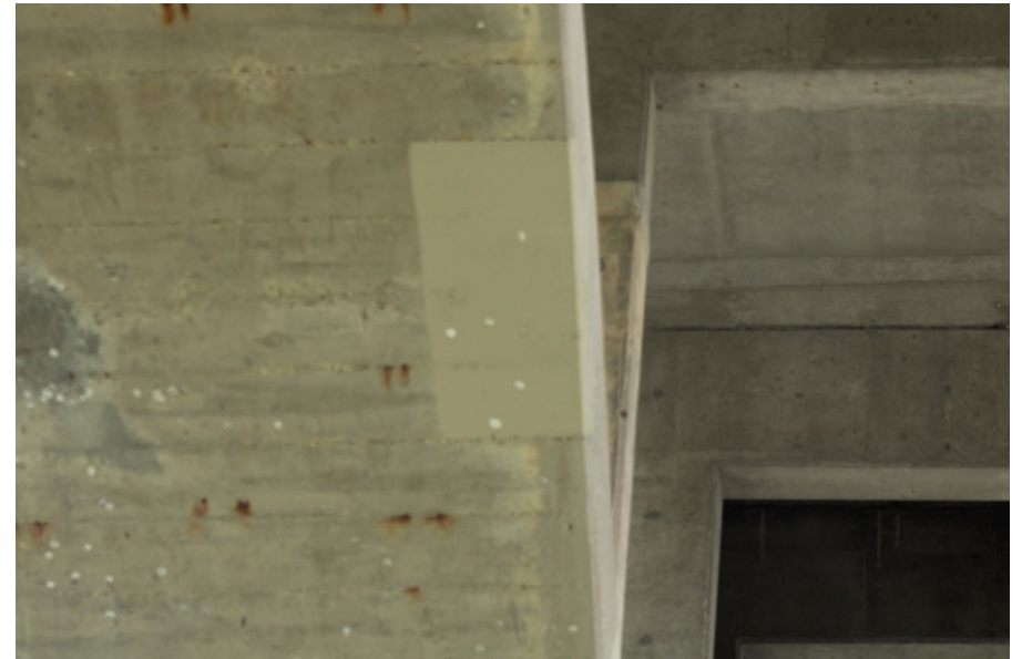
178. Looking North at Patching underneath S.N. 050-0096 Span #6
