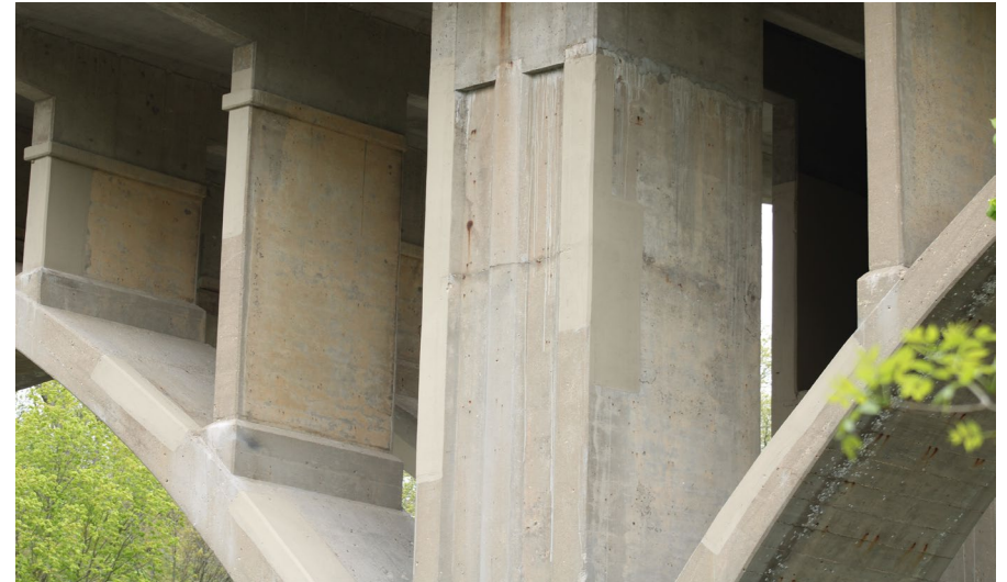
134. Looking East at S.N. 050-0096 West Profile of Pier #5
