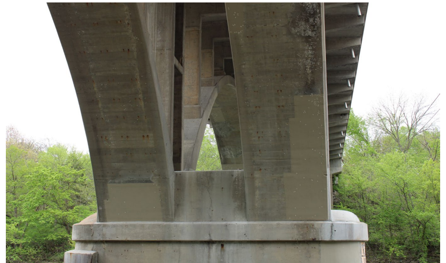
43. Looking South at Patching underneath S.N. 050-0096 Span #4
