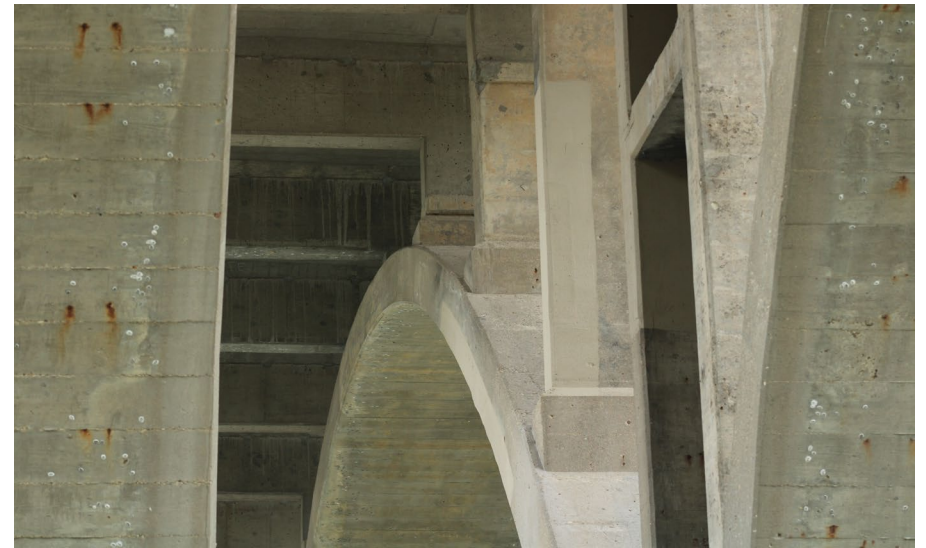
76. Looking North at Patching on S.N. 050-0096 West Profile of East Span #5
