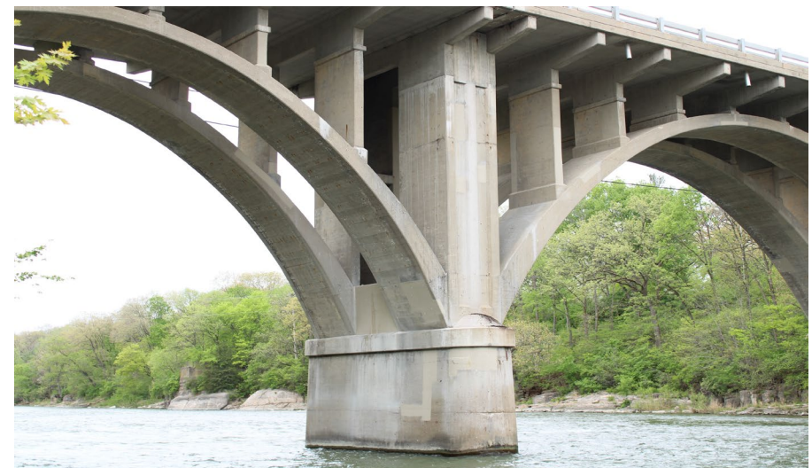
136. Looking West at S.N. 050-0096 East Profile of Pier #5
