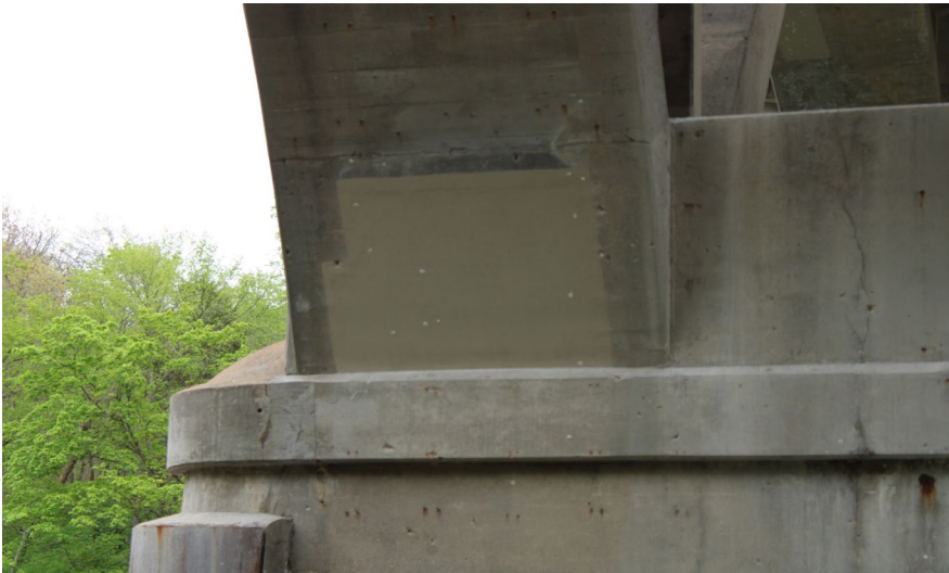
40. Looking South-East at Patching underneath S.N. 050-0096 East Span #4
