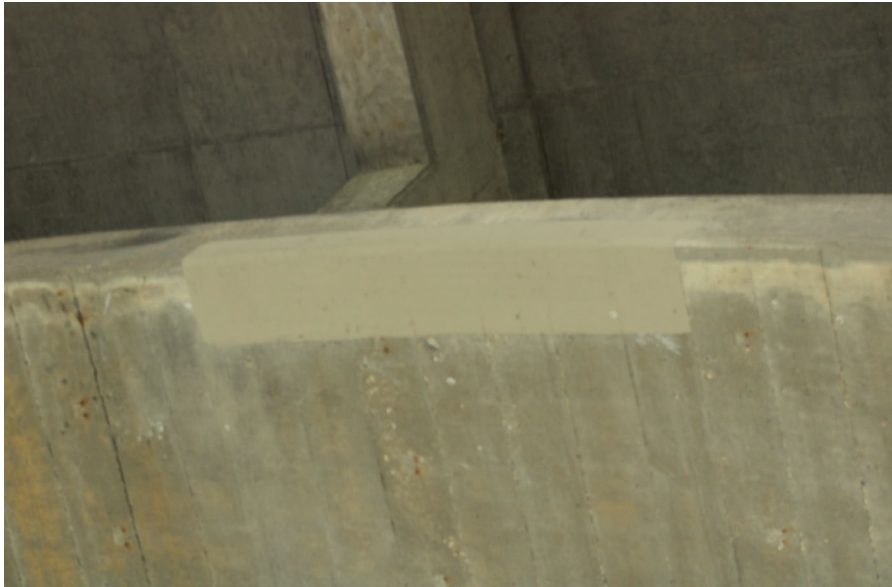
181. Looking directly up at patching underneath S.N. 050-0096 East Span #6
