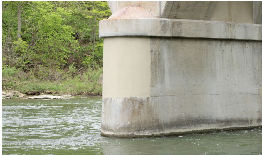
135. Looking East at S.N. 050-0096 West Profile of Pier #5
