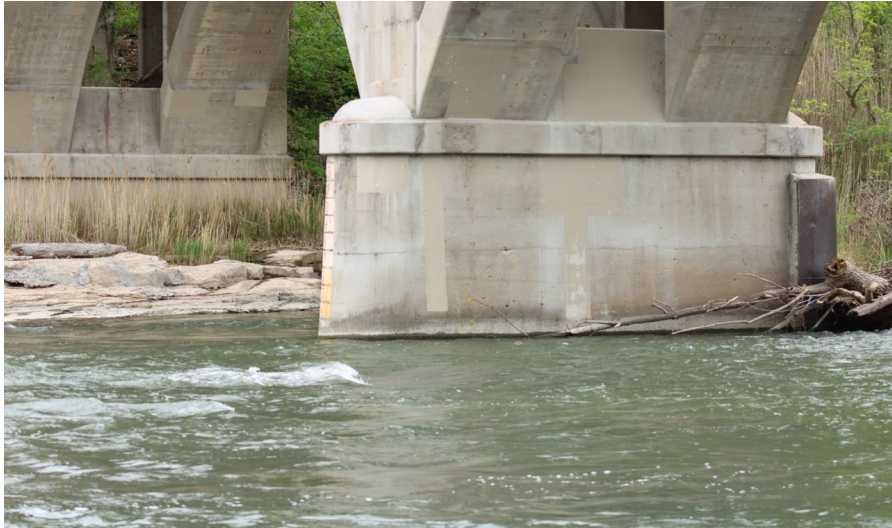
133. Looking North-East at S.N. 050-0096 West Profile of Pier #4
