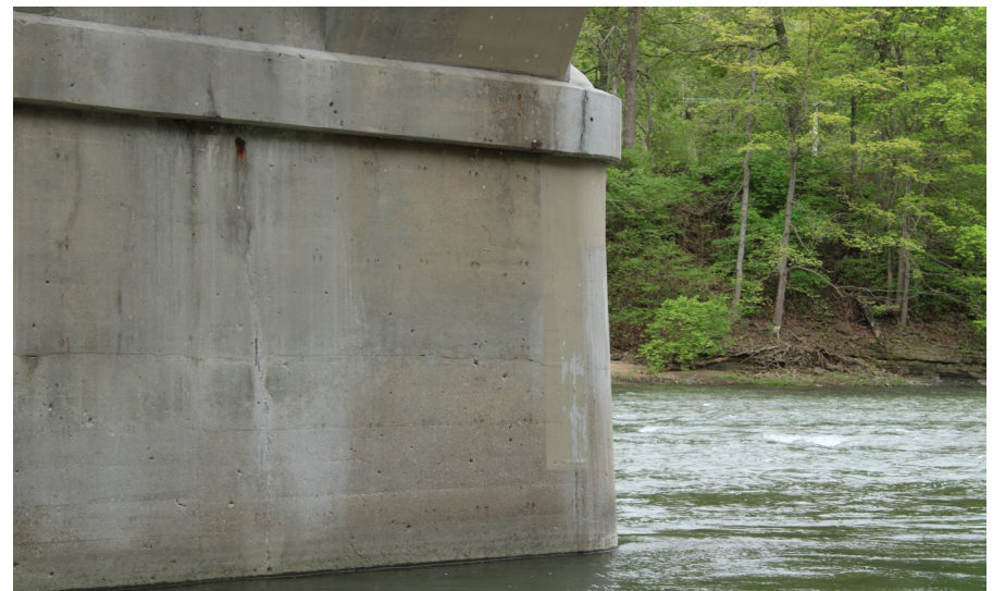
47. Looking South at Patching on the North Profile of S.N. 050-0096 Pier #4
