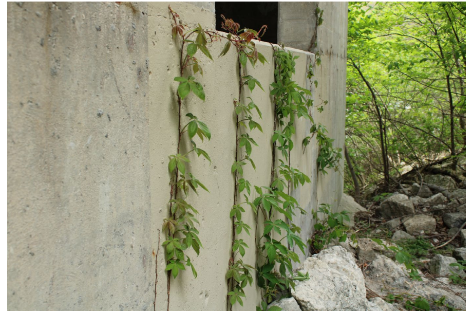
138. Looking North-East at Patching on S.N. 050-0096 South Profile of Pier #6
