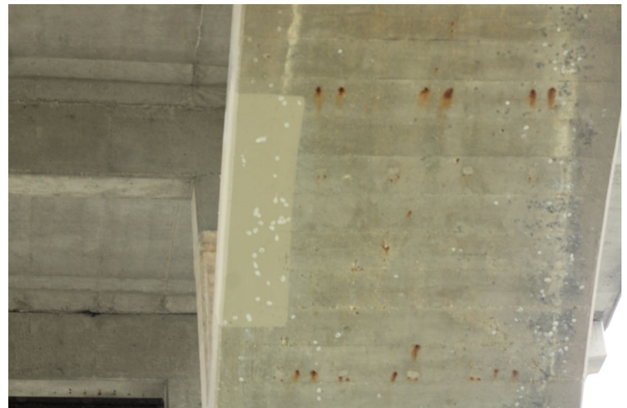
176. Looking North at Patching underneath S.N. 050-0096 East Span #6
