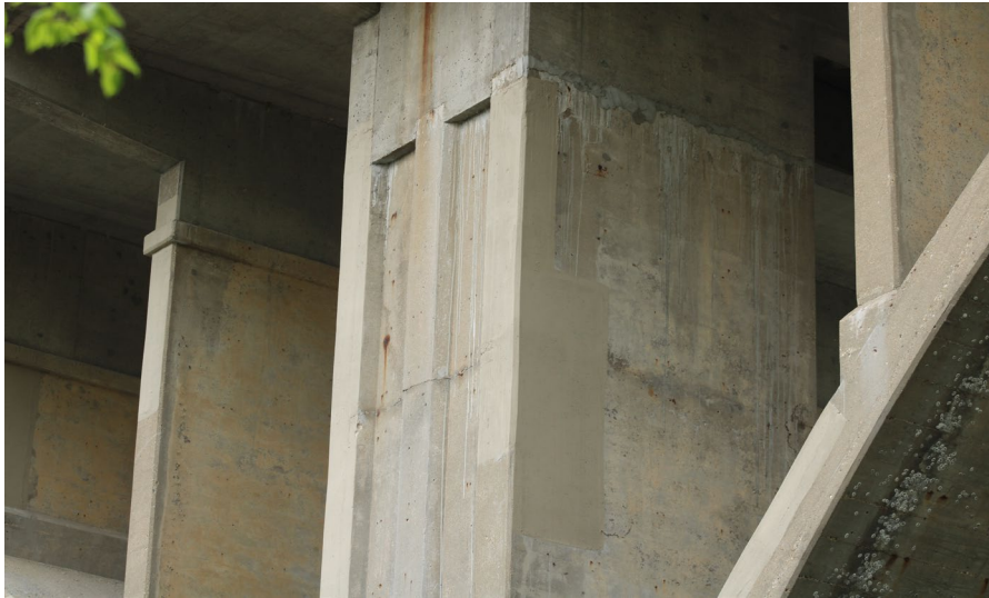
91. Looking North-East at Patching on S.N. 050-0096 West Profile of Pier #5
