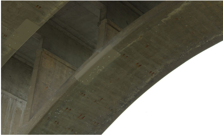
99. Looking North-East at Patching on S.N. 050-0096 East Span #6
