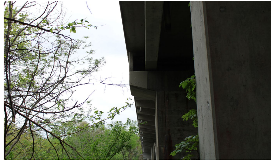
14. Looking South-East at Patching on the North Profile of S.N. 50-0096 East Pier #3
