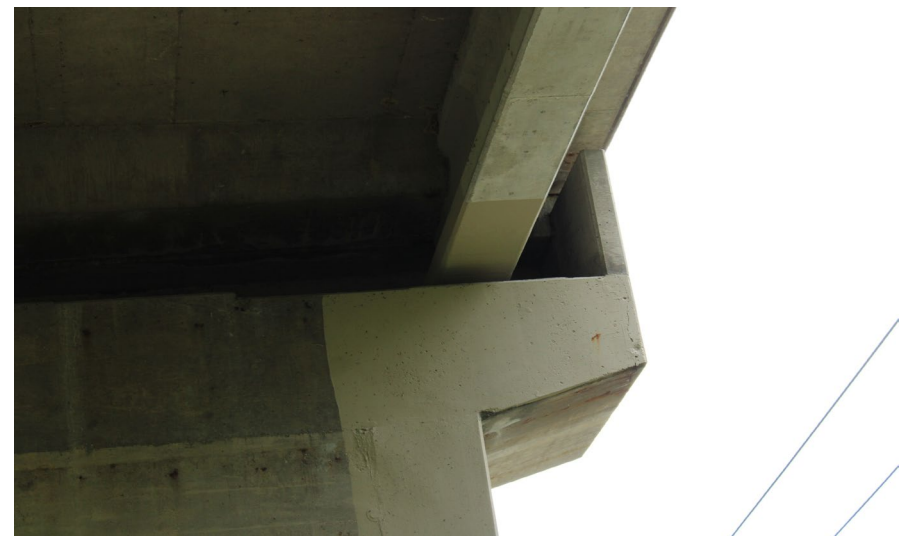
16. Looking South-West at Patching along the beams on the North Profile of S.N. 050-0096 East West Pier #3
