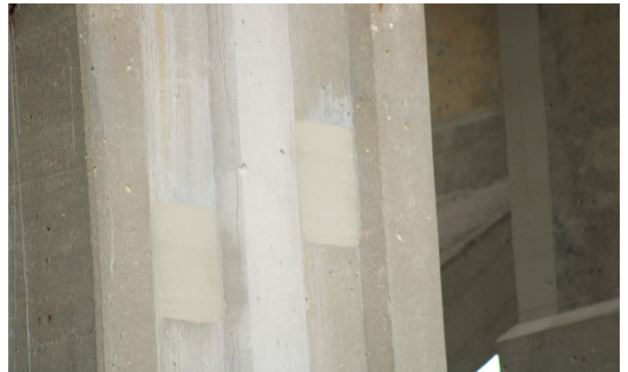
164. Looking North-West at Patching on S.N. 050-0096 East Profile of Pier #5
