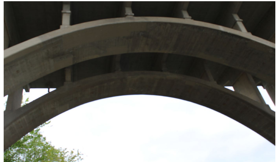
28. Looking East at Patching underneath S.N. 050-0096 Span #4
