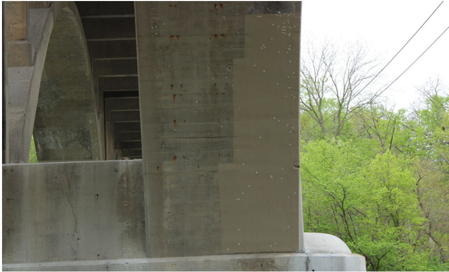
44. Looking South at Patching underneath S.N. 050-0096 West Span #4
