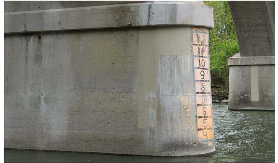
53. Looking South at Patching on the North Profile of S.N. 050-0096 Pier #4
