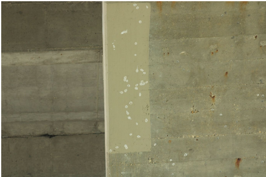
175. Looking North at Patching underneath S.N. 050-0096 East Span #6
