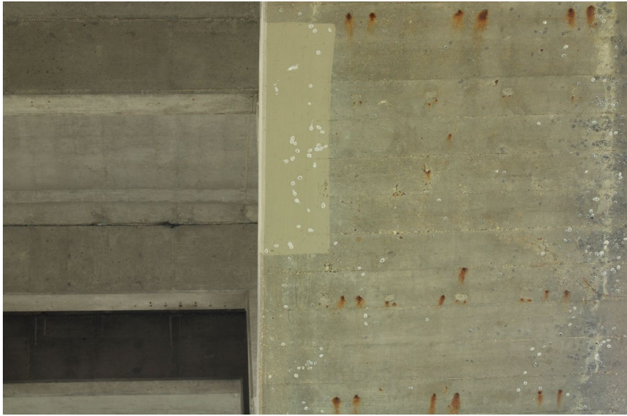
185. Looking North at Patching underneath S.N. 050-0096 East Span #6
