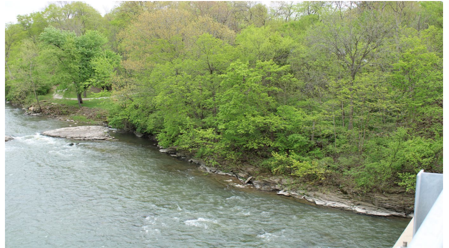
12. Looking South-East at the SE Quad of S.N. 050-0096 at Sta. 196+85
