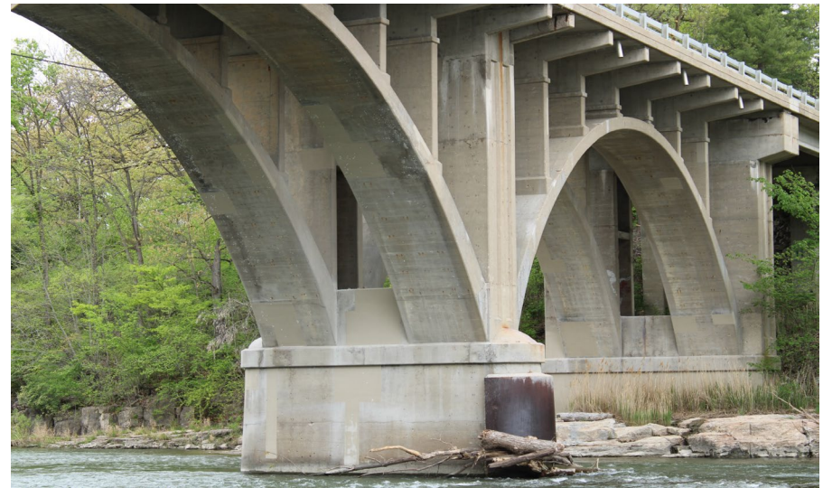
132. Looking North-West at S.N. 050-0096 East Profile of Pier #4
