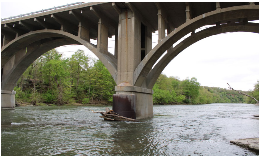
50. Looking West at Patching on the South Profile of S.N. 050-0096 Pier #4
