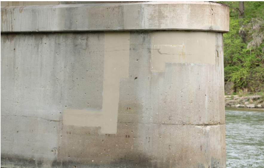
151. Looking North-West at Patching on S.N. 050-0096 South Profile of Pier #5
