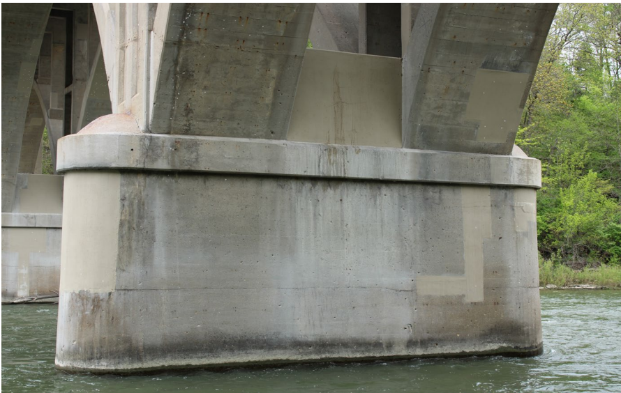
85. Looking East at Patching on S.N. 050-0096 underneath Span #6
