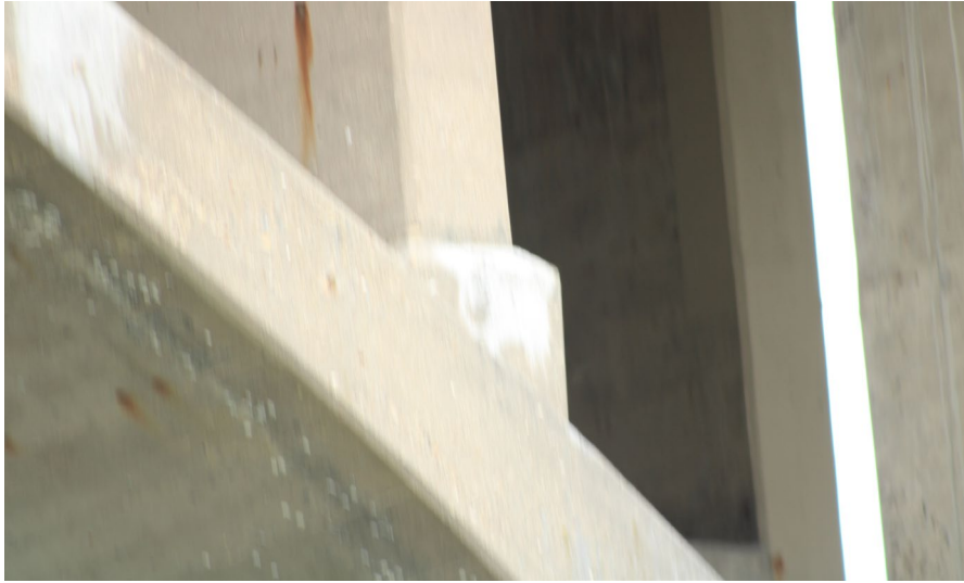
169. Looking North-West at Patching on S.N. 050-0096 West Profile of Pier #5
