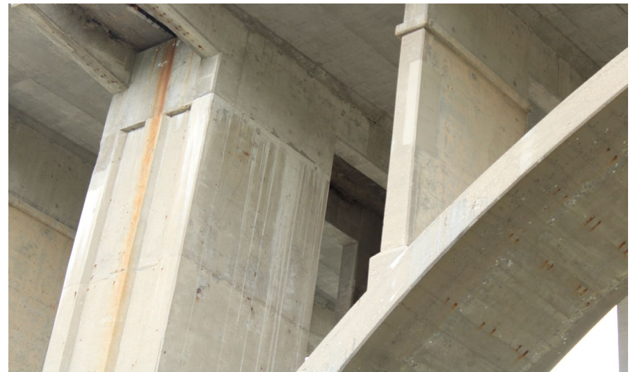
55. Looking West at Patching on S.N. 050-0096 East Span #4
