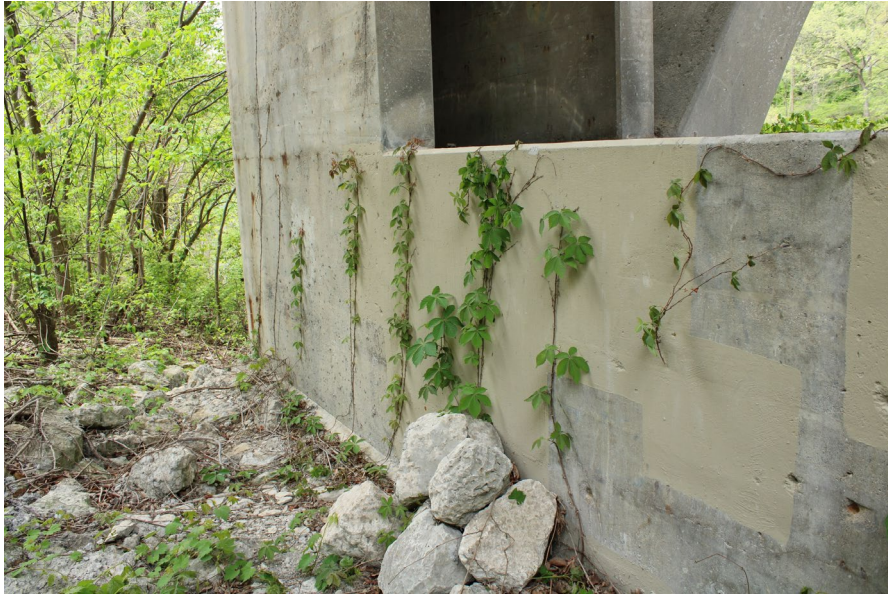
137. Looking West at Patching on S.N. 050-0096 South Profile of Pier #6
