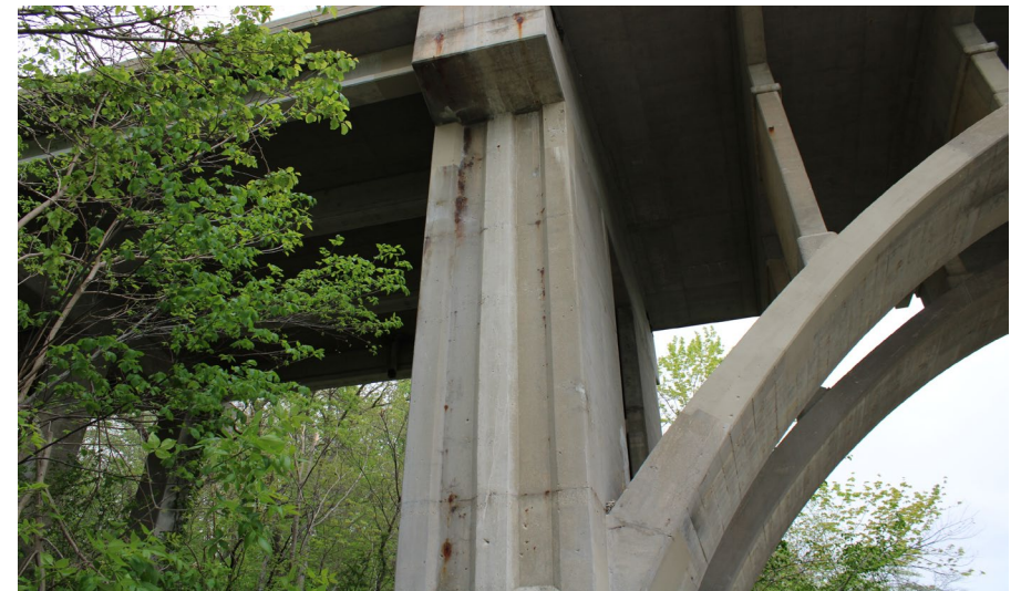
20. Looking East at Patching on the West Profile of S.N. 050-0096 West Pier #3
