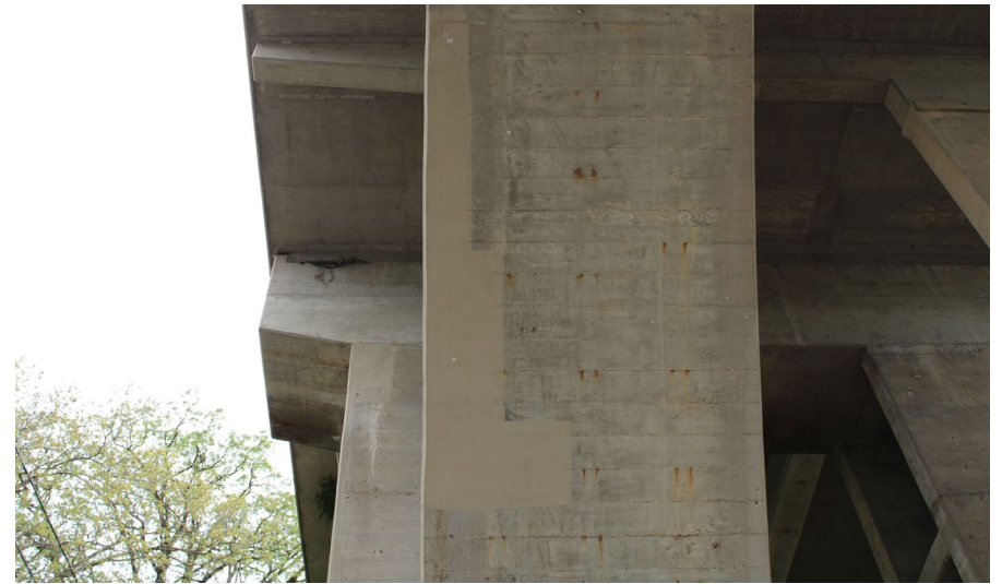
30. Looking North-East at Patching underneath S.N. 050-0096 West Span #4
