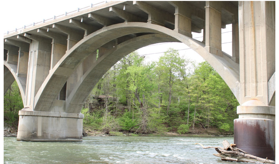
69. Looking South-West at S.N. 050-0096 Span #5
