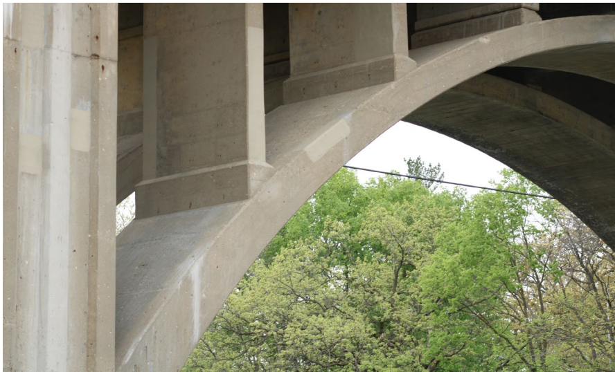
155. Looking North-West at Patching on S.N. 050-0096 East Profile of East Span #5
