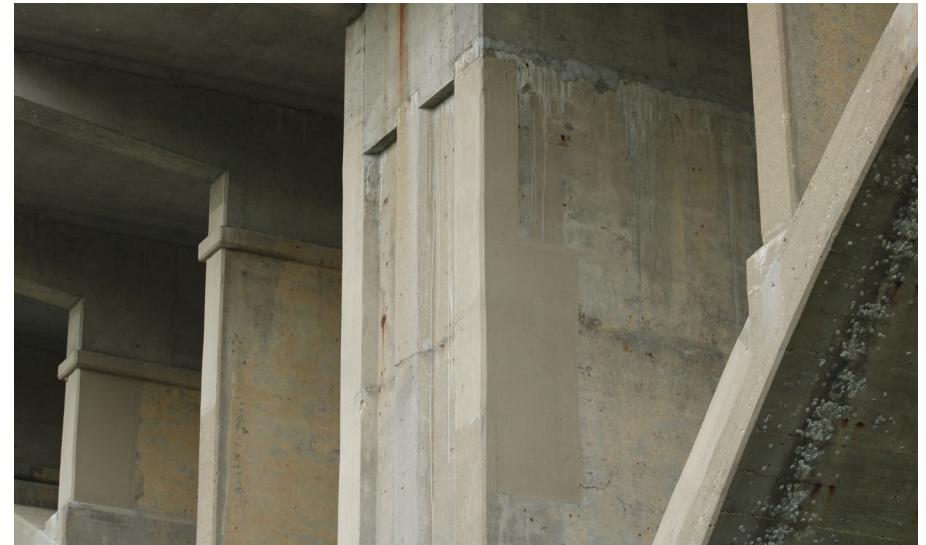
78. Looking North-East at S.N. 050-0096 West Profile of Pier #5
