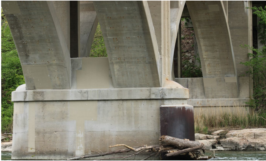
79. Looking North at Patching on S.N. 050-0096 underneath Span #5
