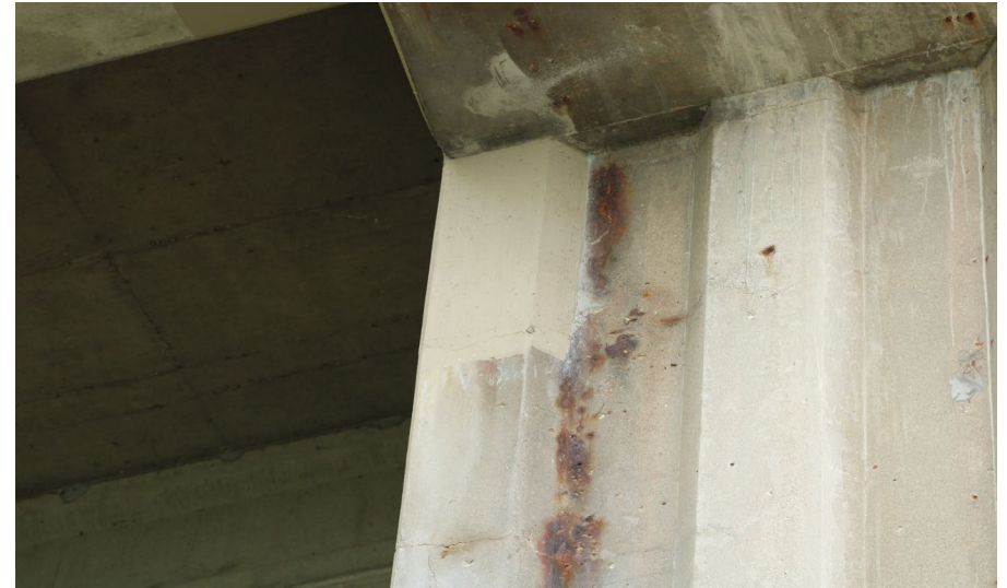
18. Looking East at Patching on the West Profile of S.N. 050-0096 West Pier #3
