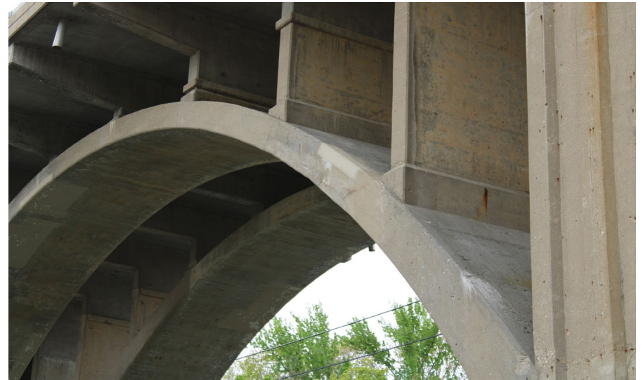
57. Looking West at Patching on S.N. 050-0096 East Span #5
