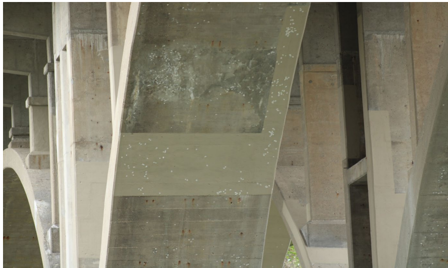
62. Looking South-East at Patching on S.N. 050-0096 East Span #5
