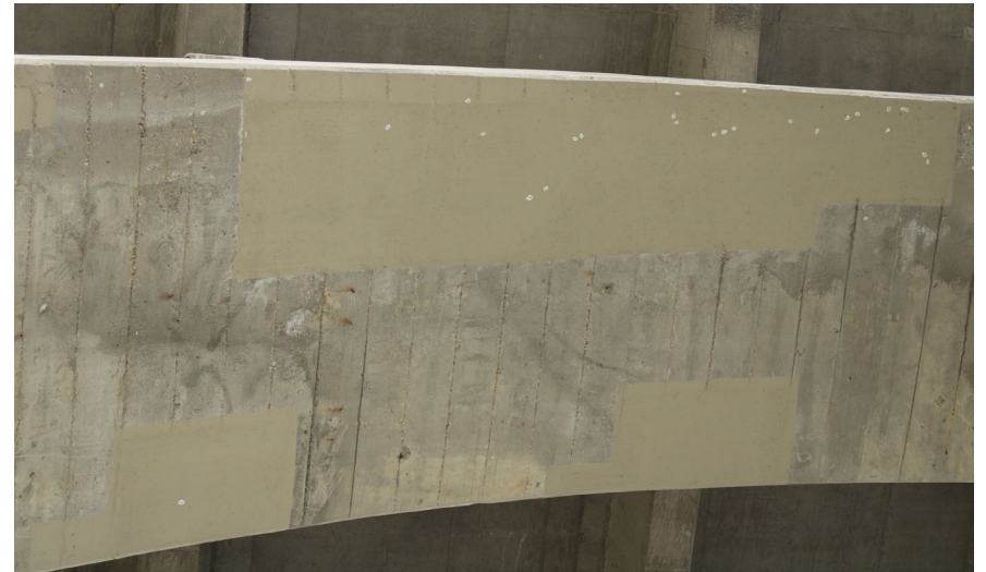
33. Looking East at Patching underneath S.N. 050-0096 West Span #4
