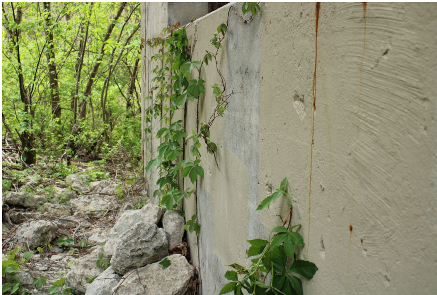
139. Looking North-West at Patching on S.N. 050-0096 South Profile of Pier #6
