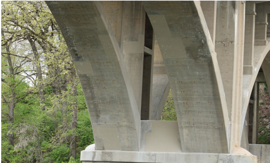
75. Looking North-West at Patching on S.N. 050-0096 underneath Span #5
