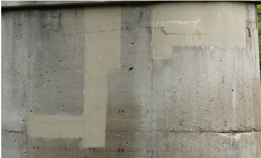
81. Looking West at Patching on S.N. 050-0096 Pier #5
