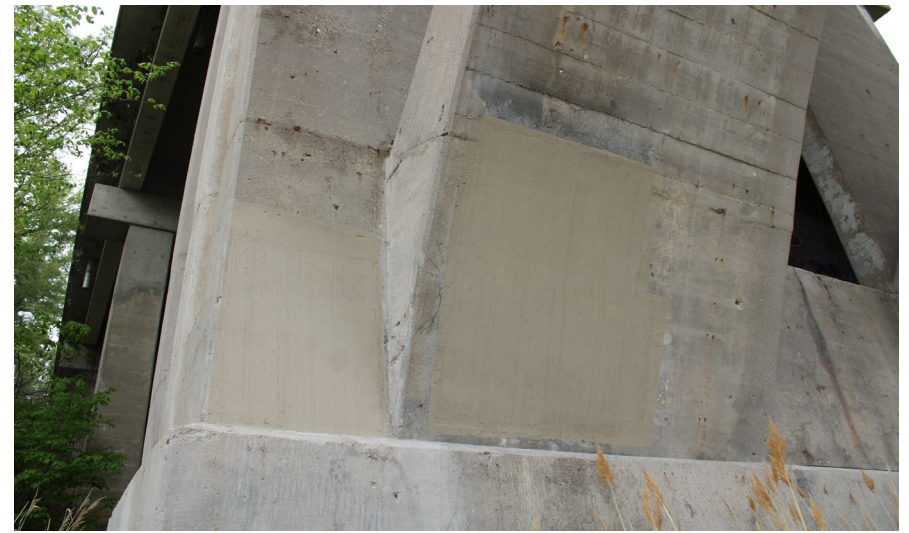
22. Looking North-East at Patching underneath S.N. 050-0096 West Span #4
