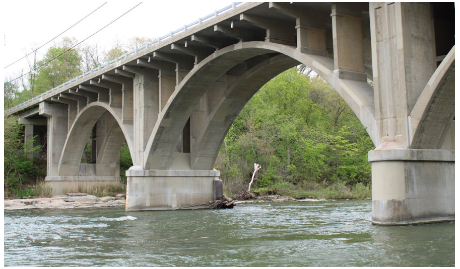
128. Looking North at S.N. 050-0096 West Profile
