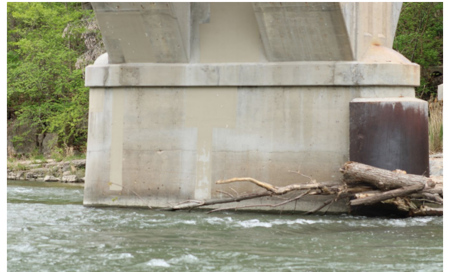
152. Looking North-West at Patching on S.N. 050-0096 South Profile of Pier #4
