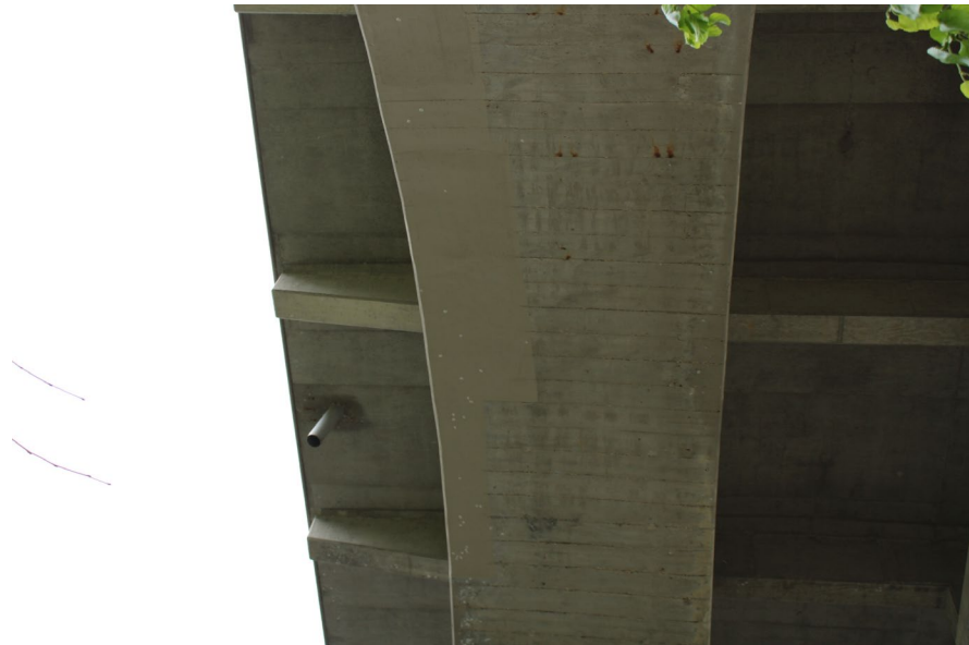
187. Looking North at Patching underneath S.N. 050-0096 West Span #6
