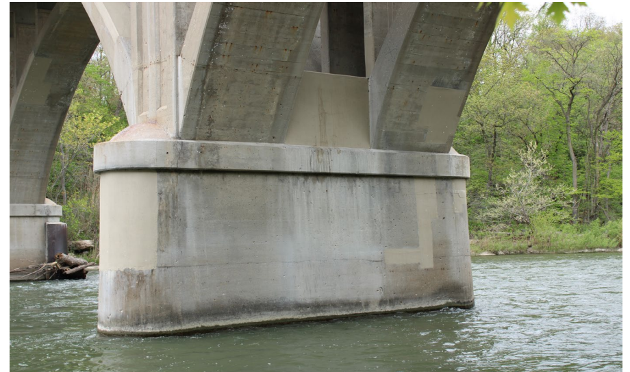
96. Looking East at Patching on S.N. 050-0096 underneath Span #6
