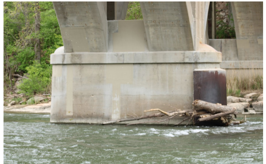
144. Looking North-West at Patching underneath S.N. 050-0096 Span #5
