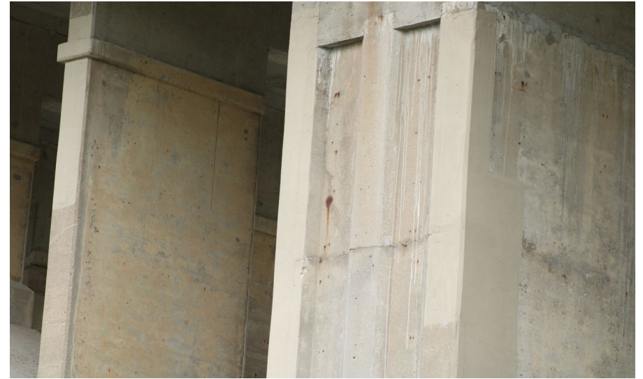
166. Looking North-East at Patching on S.N. 050-0096 West Profile of Pier #5
