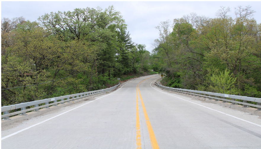
7. Looking North along IL 178 from S.N. 050-0096 at Sta. 196+85
