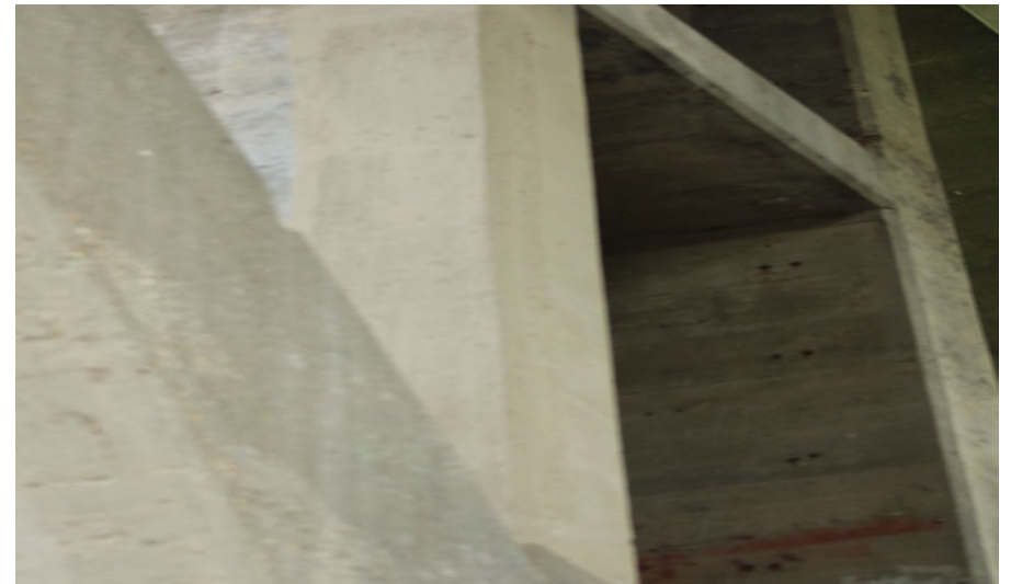
180. Looking South at Patching on the inside of S.N. 050-0096 Pier #6
