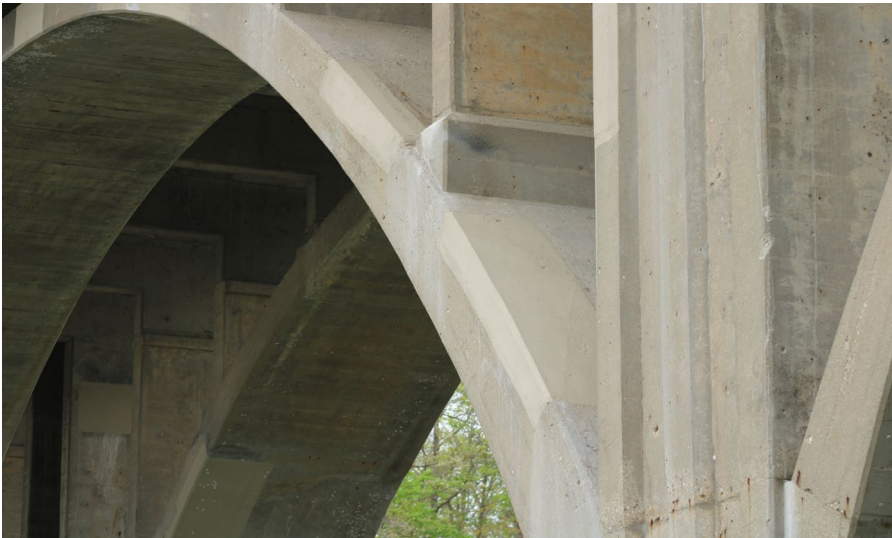
77. Looking North-East at S.N. 050-0096 West Span #5
