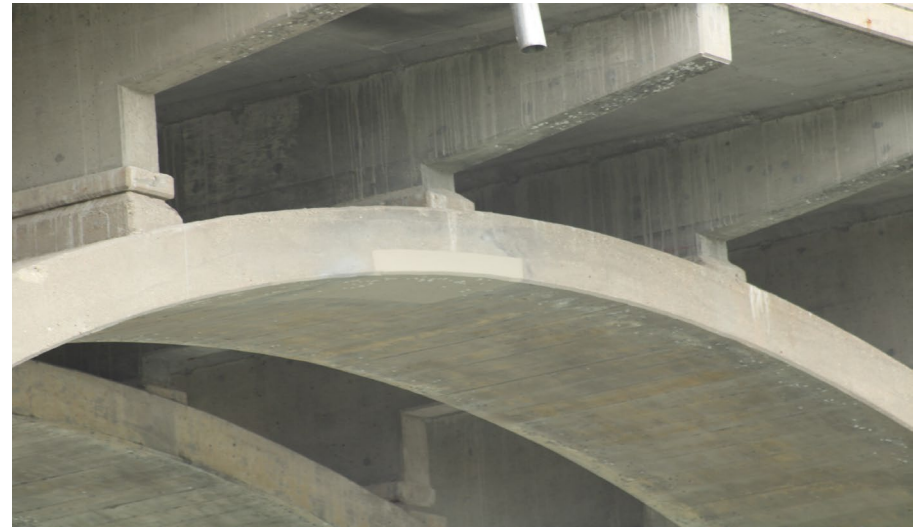
158. Looking North-West at Patching on S.N. 050-0096 East Profile of East Span #5
