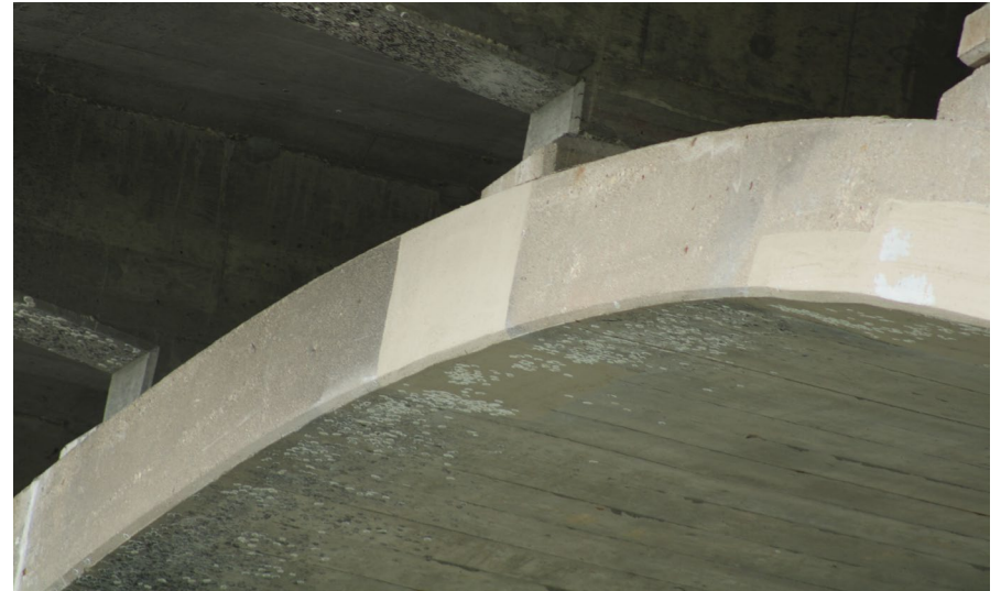
92. Looking North-East at Patching on S.N. 050-0096 West Span #5
