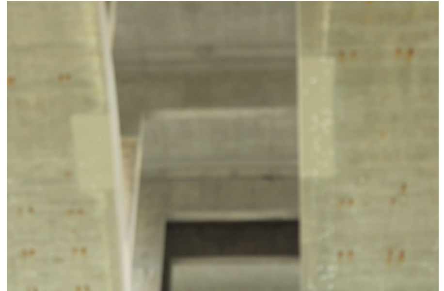
142. Looking North at Patching underneath S.N. 050-0096 Span #6
