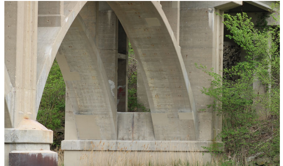
130. Looking North-West at S.N. 050-0096 East Profile of Pier #3
