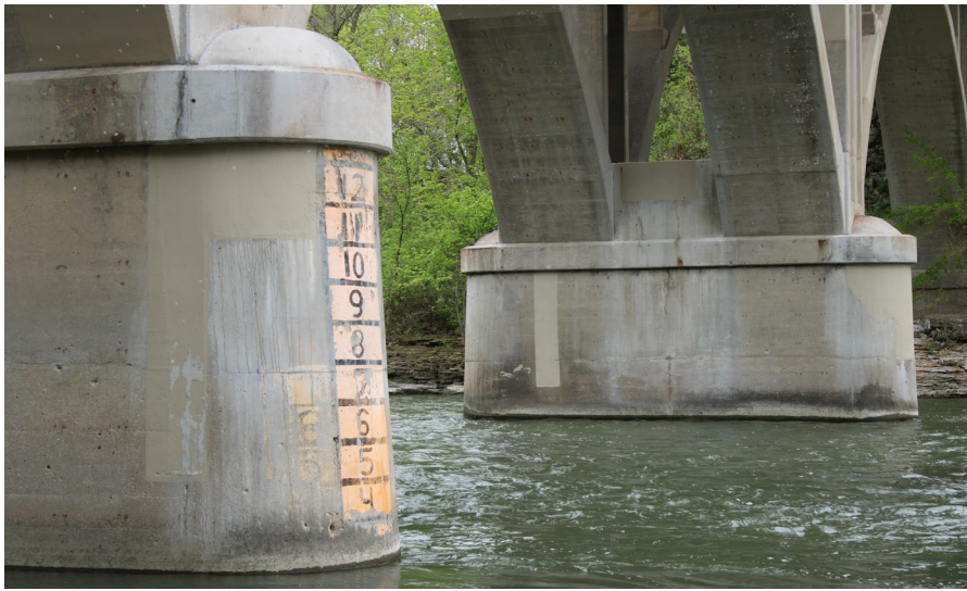
52. Looking South at Patching on the North Profile of S.N. 050-0096 Pier #4
