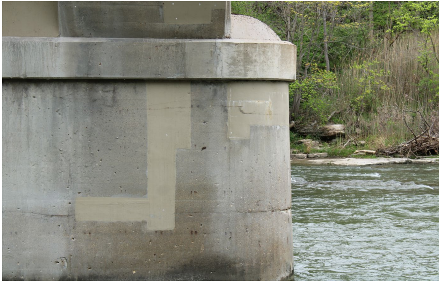
87. Looking North-East at Patching on S.N. 050-0096 South Profile of Pier #5
