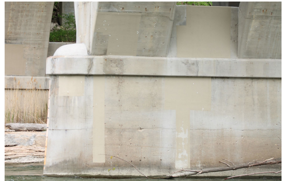
98. Looking North-East at Patching on S.N. 050-0096 underneath Span #5
