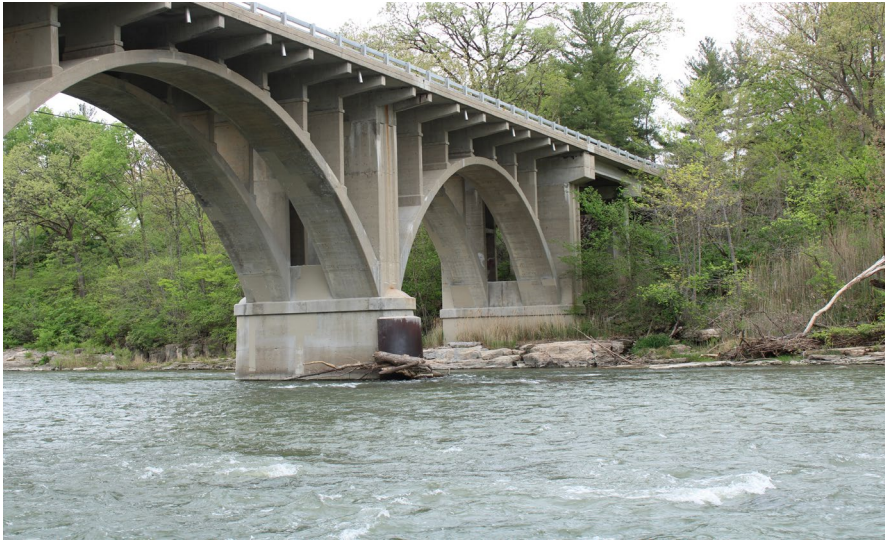
121. Looking North-West at S.N. 050-0096 East Profile of Span #5
