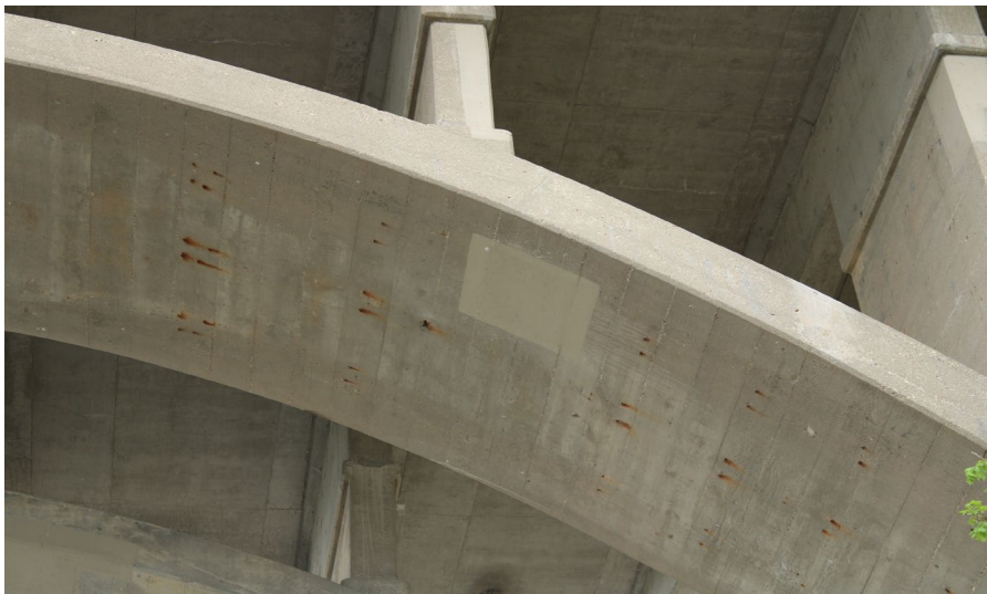
54. Looking West at Patching on S.N. 050-0096 East Span #4
