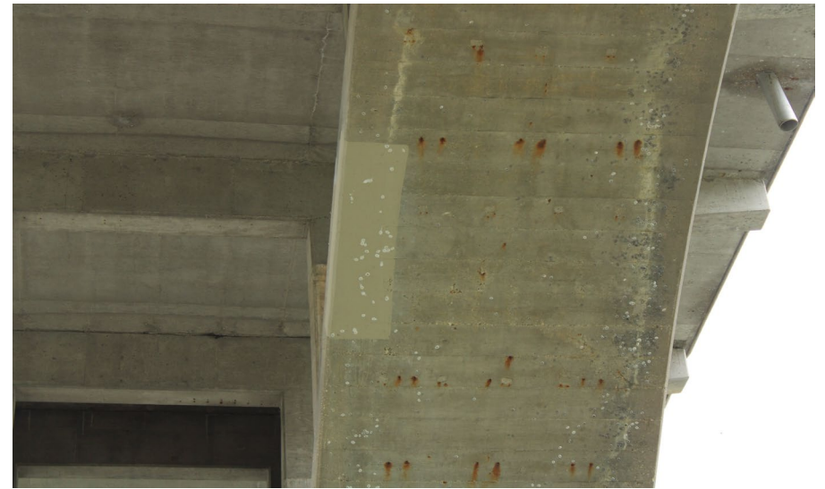
100. Looking North at Patching on S.N. 050-0096 underneath East Span #6
