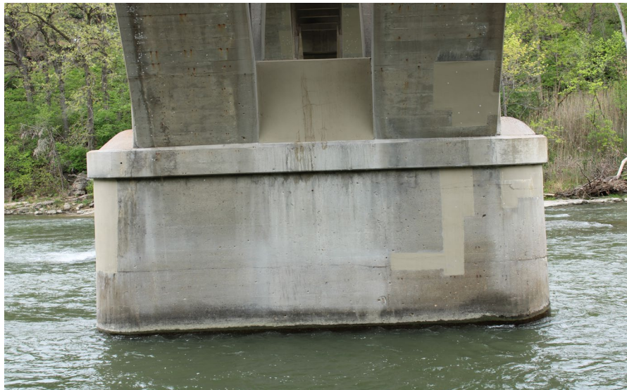
89. Looking North at Patching on S.N. 050-0096 underneath Span #6
