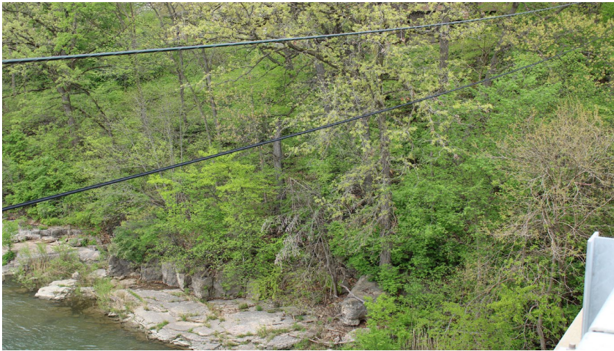
9. Looking North-West at the NW Quad of S.N. 050-0096 from S.N. 050-0096 at Sta. 196+85
