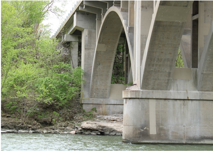
117. Looking South-West at S.N. 050-0096 East Profile of Span #6
