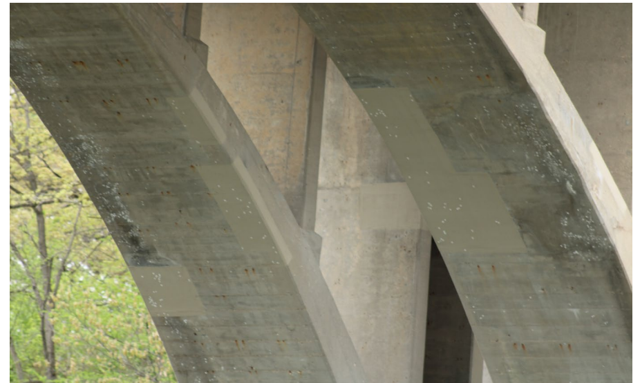
146. Looking North-West at Patching underneath S.N. 050-0096 Span #5
