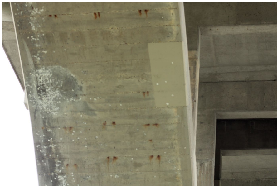
179. Looking North at Patching underneath S.N. 050-0096 Span #6
