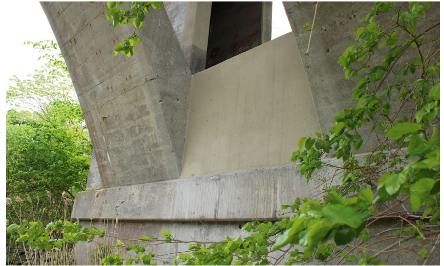
104. Looking South-East at Patching on S.N. 050-0096 North Profile of Pier #6
