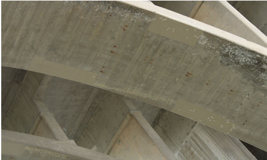
25. Looking East at Patching underneath S.N. 050-0096 West Span #4
