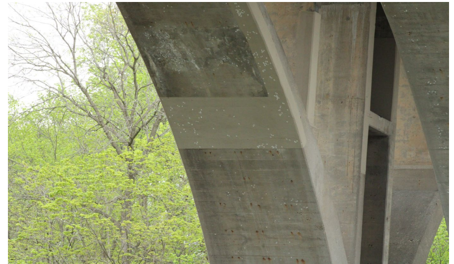
63. Looking South-East at Patching on S.N. 050-0096 East Span #5
