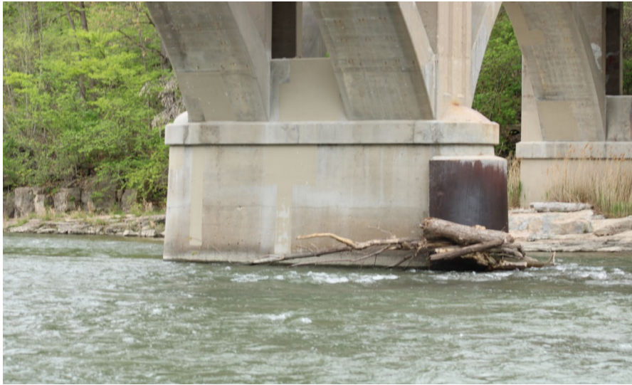
153. Looking North-West at Patching on S.N. 050-0096 Pier #4
