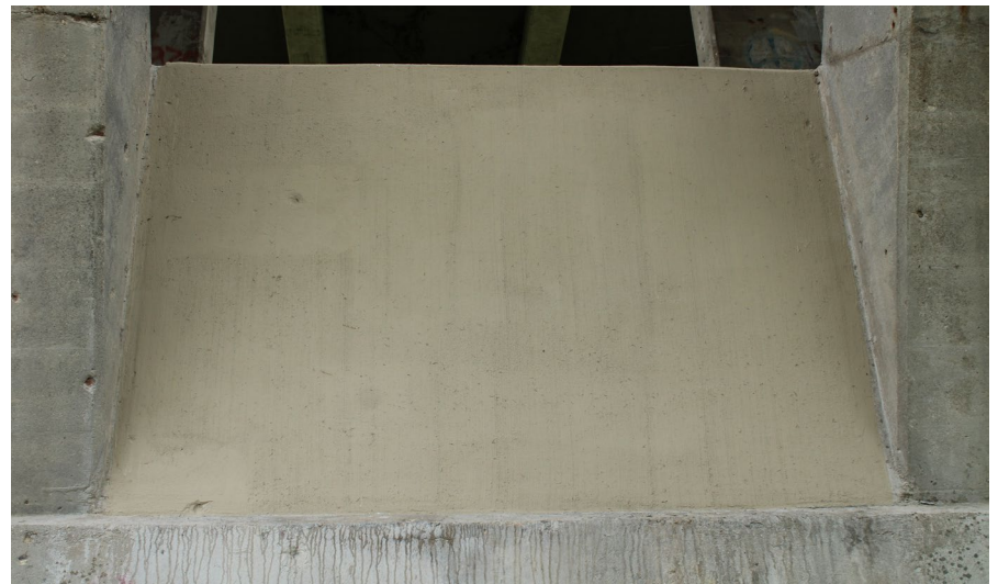
106. Looking South at Patching on S.N. 050-0096 North Profile of Pier #6
