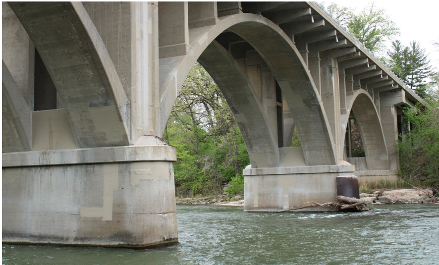
127. Looking North-West at S.N. 050-0096 East Profile of Span #4
