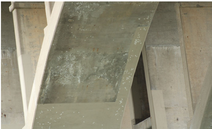
58. Looking West at Patching underneath S.N. 050-0096 East Span #5
