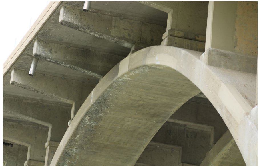
172. Looking North-East at Patching on S.N. 050-0096 West Profile of West Span #5
