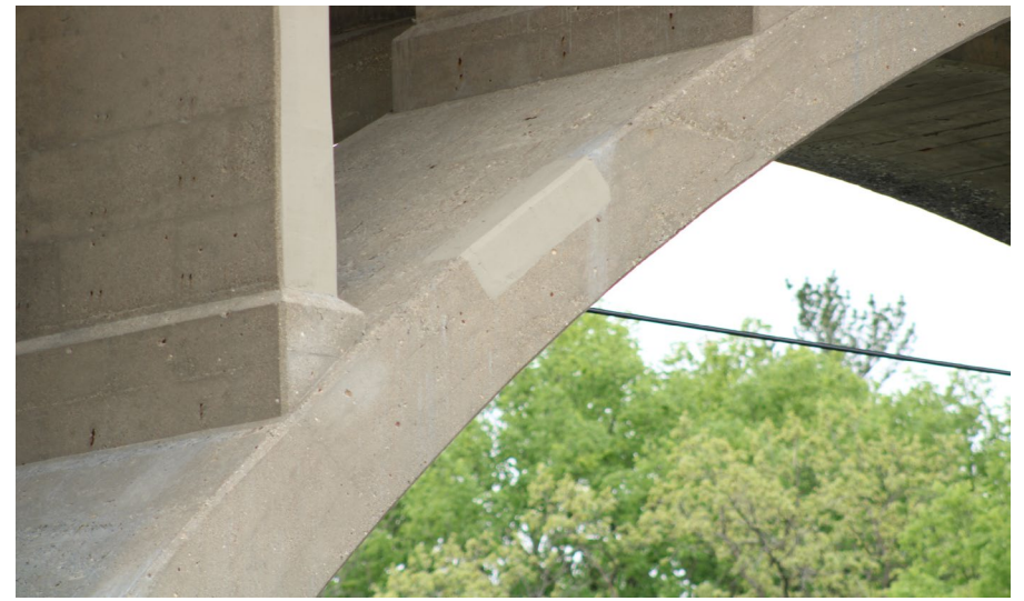
154. Looking North-West at Patching on S.N. 050-0096 East Profile of East Span #5
