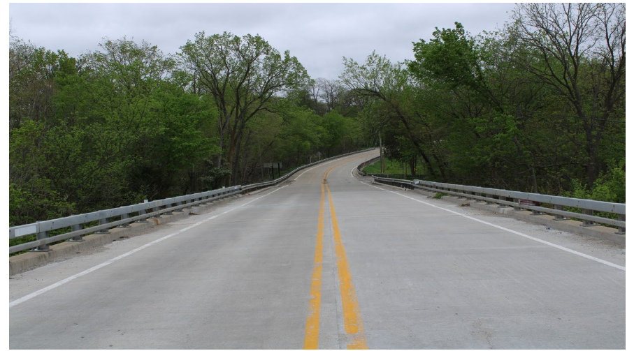
8. Looking South along IL 178 from S.N. 050-0096 at Sta. 196+85
