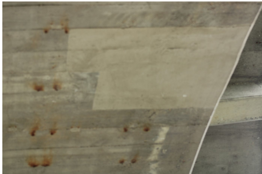
183. Looking directly up at Patching underneath S.N. 050-0096 Span #6
