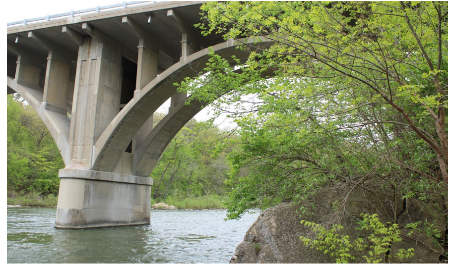
126. Looking East at S.N. 050-0096 West Profile of Span #6
