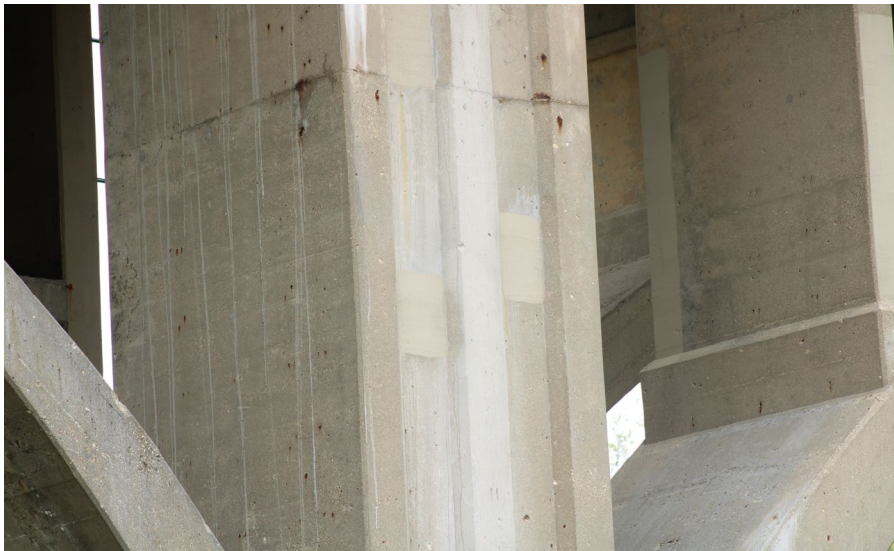
163. Looking North-West at Patching on S.N. 050-0096 East Profile of Pier #5
