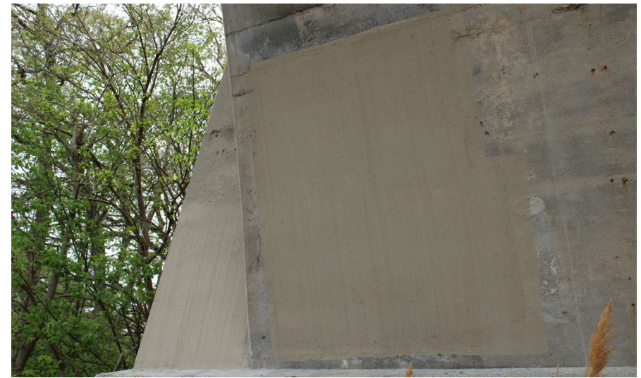
24. Looking North-East at Patching underneath S.N. 050-0096 West Span #4
