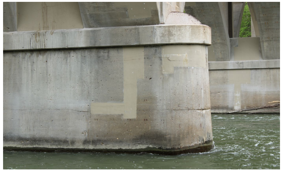
90. Looking North-East at Patching on S.N. 050-0096 South Profile of Pier #5
