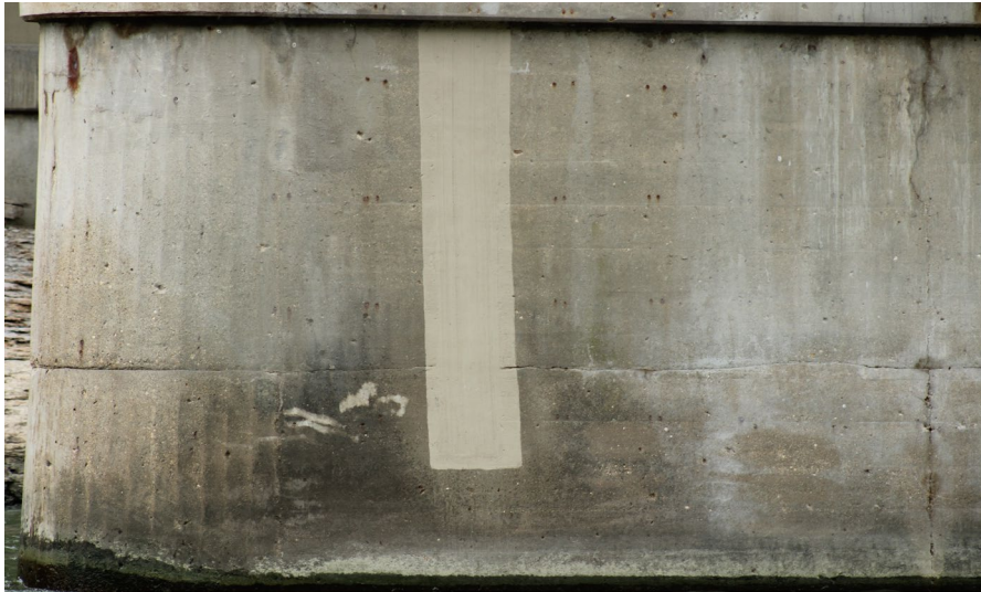
60. Looking South-West at Patching on S.N. 050-0096 Pier #5
