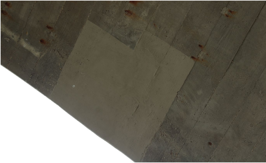
93. Looking East at Patching on S.N. 050-0096 underneath East Span #6
