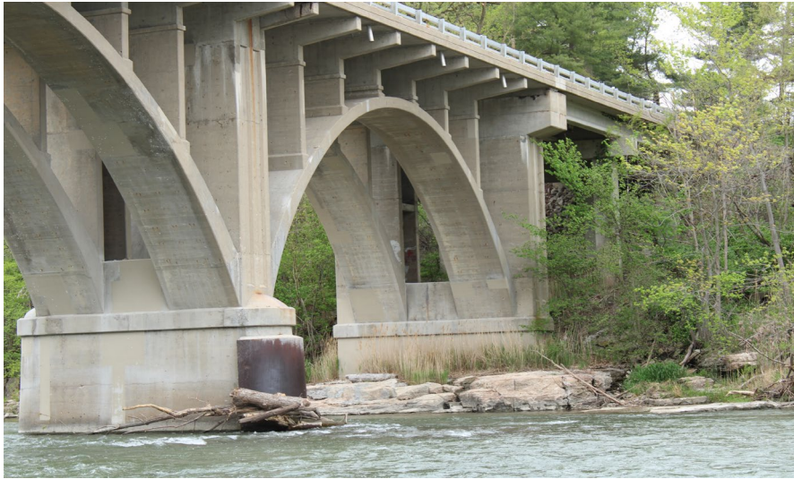
125. Looking North-West at S.N. 050-0096 East Profile of Span #4
