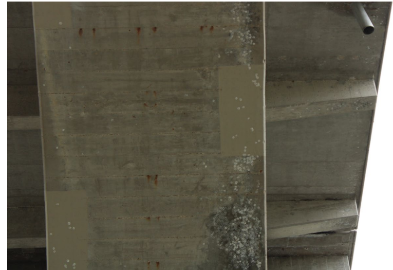
37. Looking South-East at Patching underneath S.N. 050-0096 West Span #4
