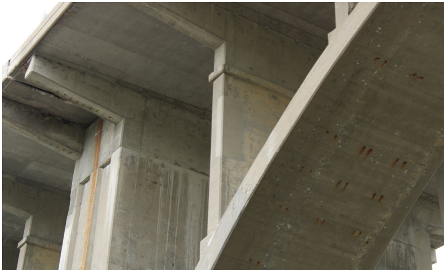
56. Looking West at Patching on S.N. 050-0096 East Span #4
