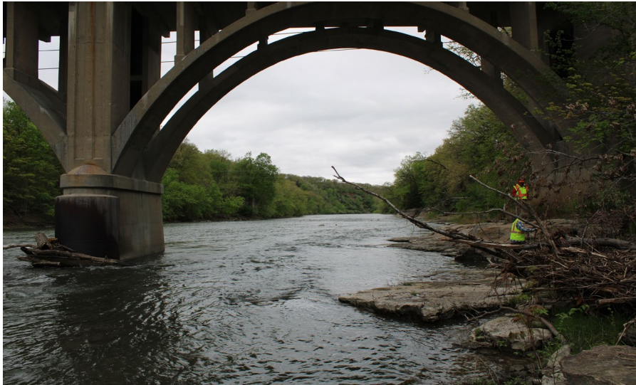
48. Looking West at Patching on S.N. 050-0096 Span #4
