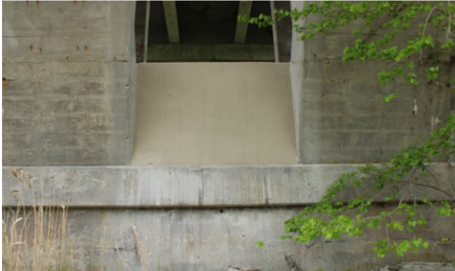
103. Looking South at Patching on S.N. 050-0096 North Profile of Pier #6
