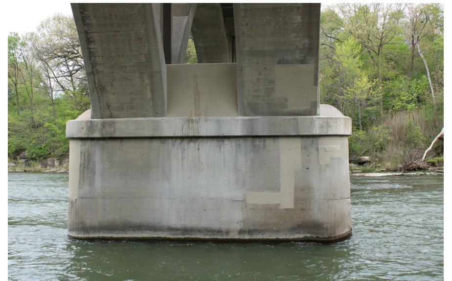
86. Looking North at Patching on S.N. 050-0096 underneath Span #6
