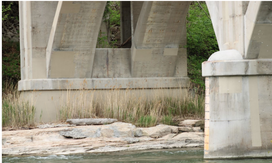
131. Looking North-East at S.N. 050-0096 West Profile of Pier #3
