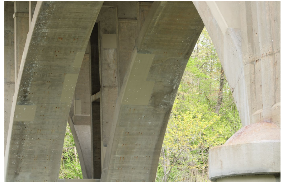
174. Looking North-East at Patching underneath S.N. 050-0096 Span #5
