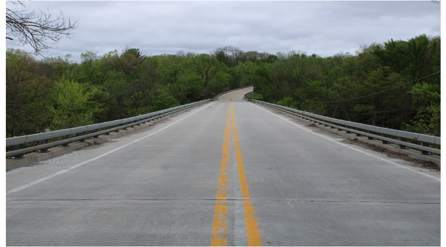
6. Looking South along IL 178 through S.N. 050-0096
