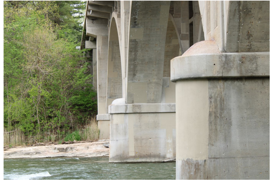
170. Looking North-East at Patching on S.N. 050-0096 South Profile of Pier #4
