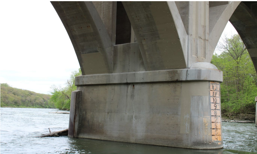
42. Looking South-East at Patching underneath S.N. 050-0096 Span #4
