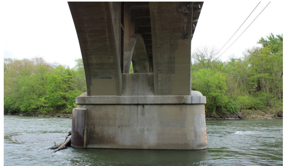
39. Looking South at Patching underneath S.N. 050-0096 Span #4
