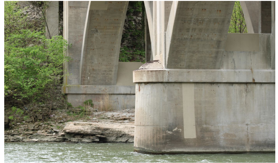
73. Looking South at Patching on S.N. 050-0096 underneath East Span #5
