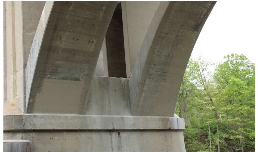
45. Looking South at Patching underneath S.N. 050-0096 West Span #4
