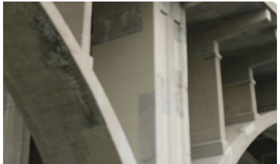
51. Looking South at Patching on the North Profile of S.N. 050-0096 Pier #4
