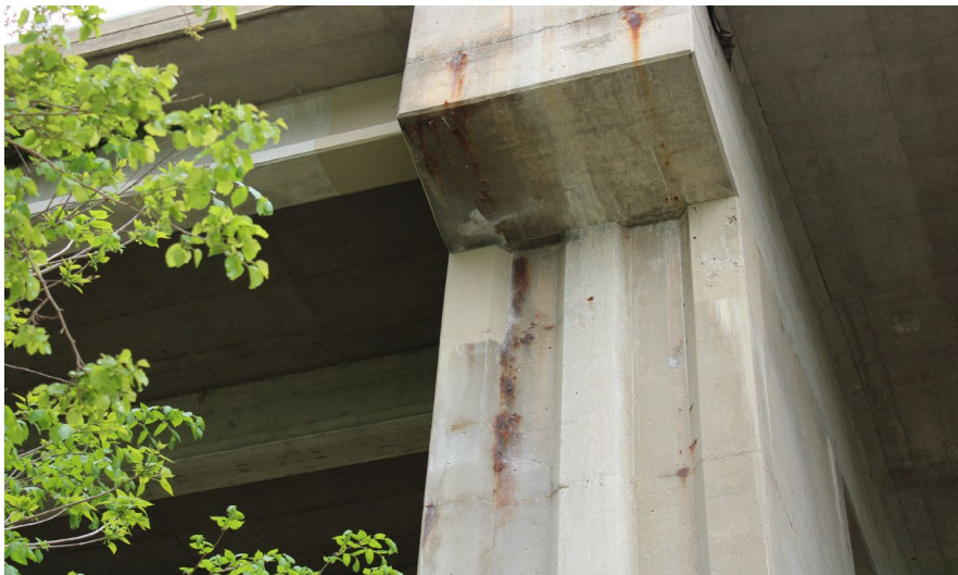
19. Looking East at Patching on the West Profile of S.N. 050-0096 West Pier #3
