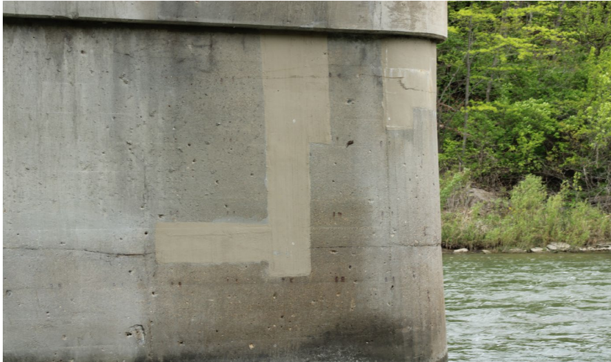
95. Looking East at Patching on S.N. 050-0096 South Profile of Pier #5
