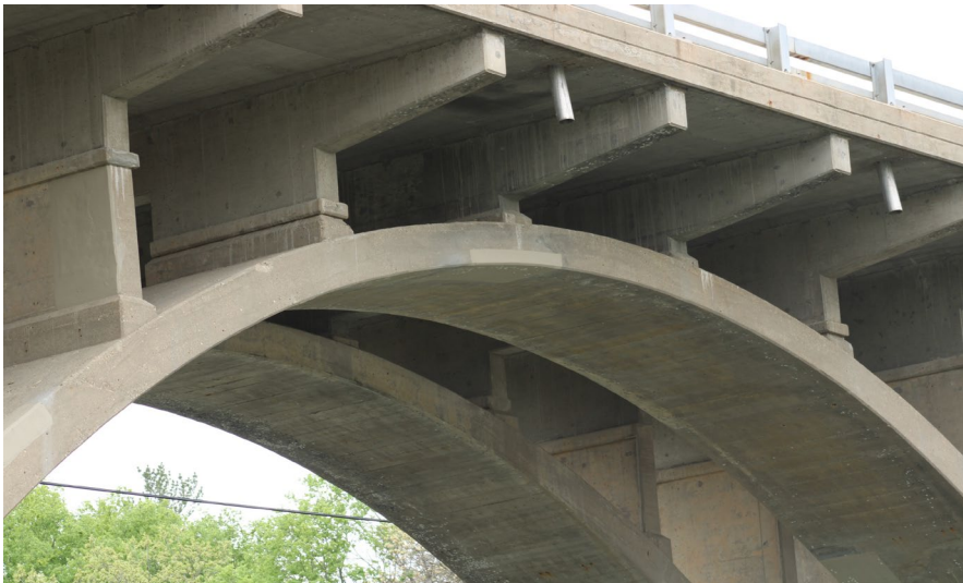
159. Looking North-West at Patching on S.N. 050-0096 East Profile of East Span #5
