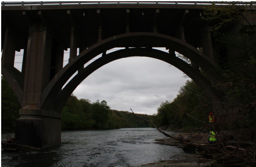
46. Looking South-West at Patching underneath S.N. 050-0096 West Span #4
