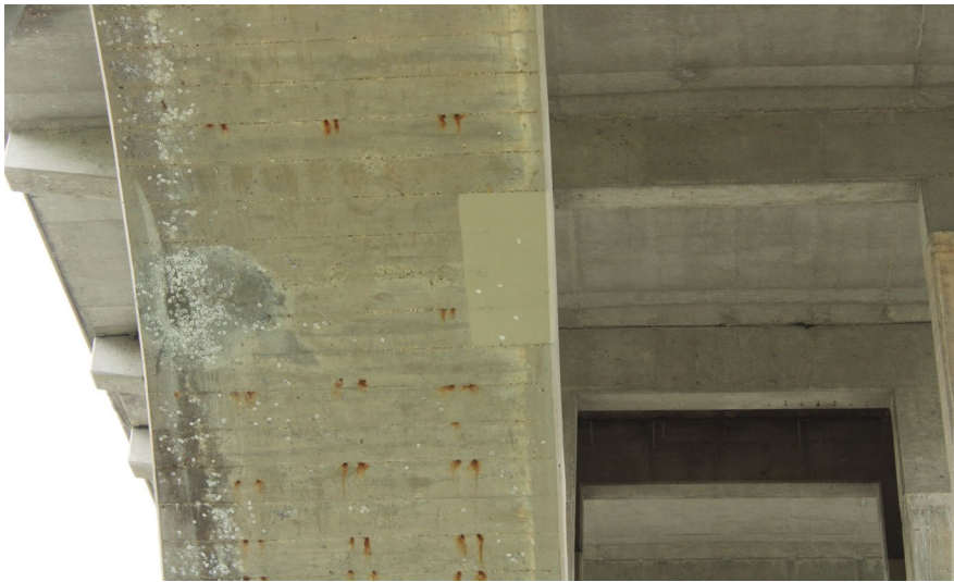
101. Looking North at Patching on S.N. 050-006 underneath Span #6
