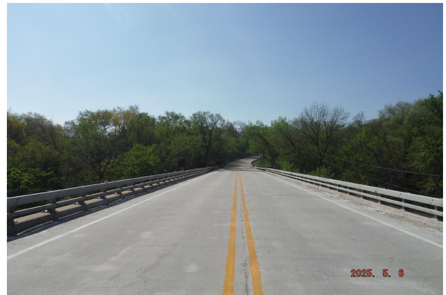
8. Looking South along IL 178 from S.N. 050-0096 at Sta. 196+85
