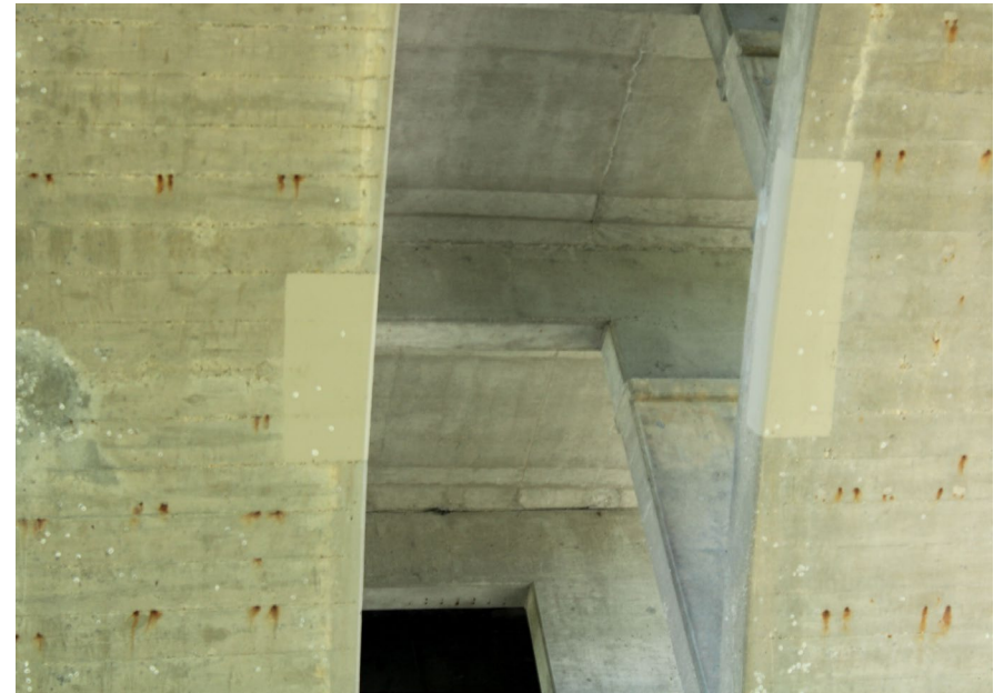
142. Looking North at Patching underneath S.N. 050-0096 Span #6
