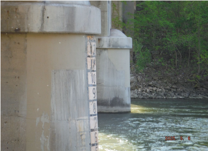
52. Looking South at Patching on the North Profile of S.N. 050-0096 Pier #4
