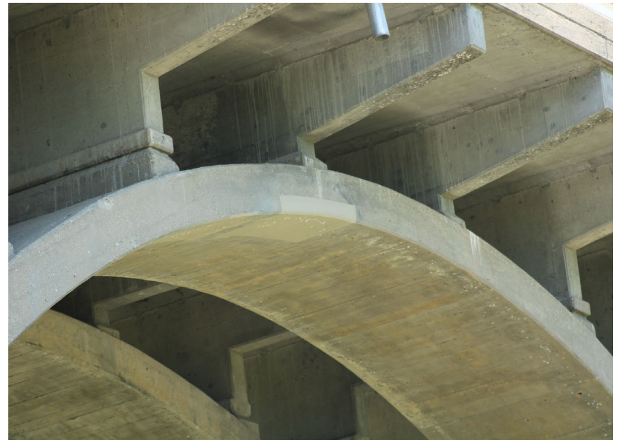
158. Looking North-West at Patching on S.N. 050-0096 East Profile of East Span #5
