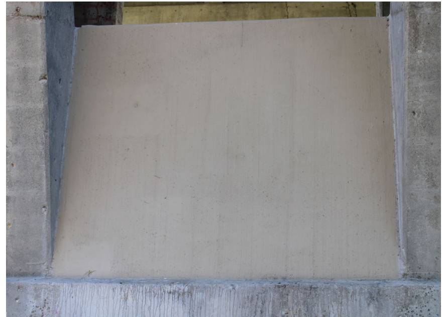
106. Looking South at Patching on S.N. 050-0096 North Profile of Pier #6
