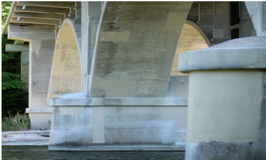
147. Looking North at Patching underneath S.N. 050-0096 West Span #5
