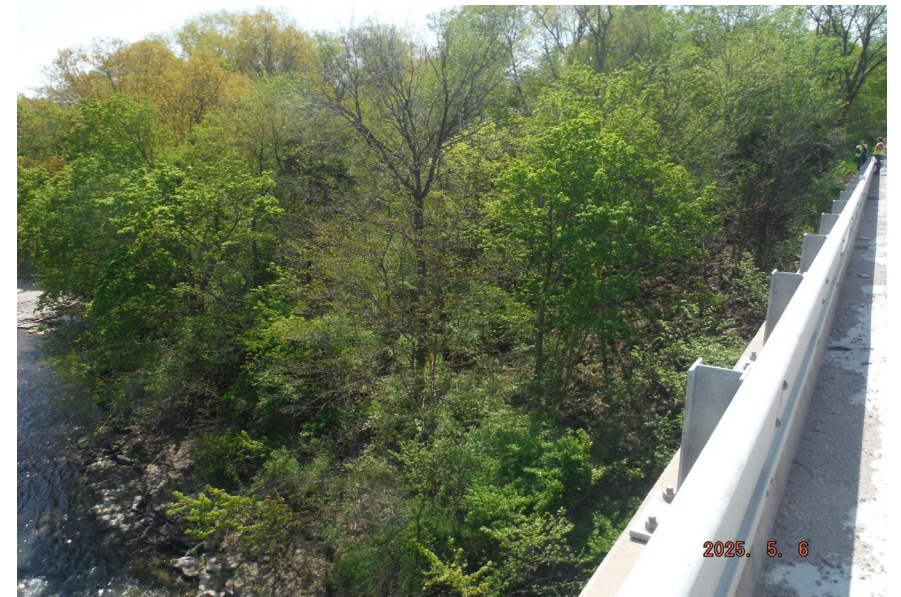
12. Looking South-East at the SE Quad of S.N. 050-0096 at Sta. 196+85
