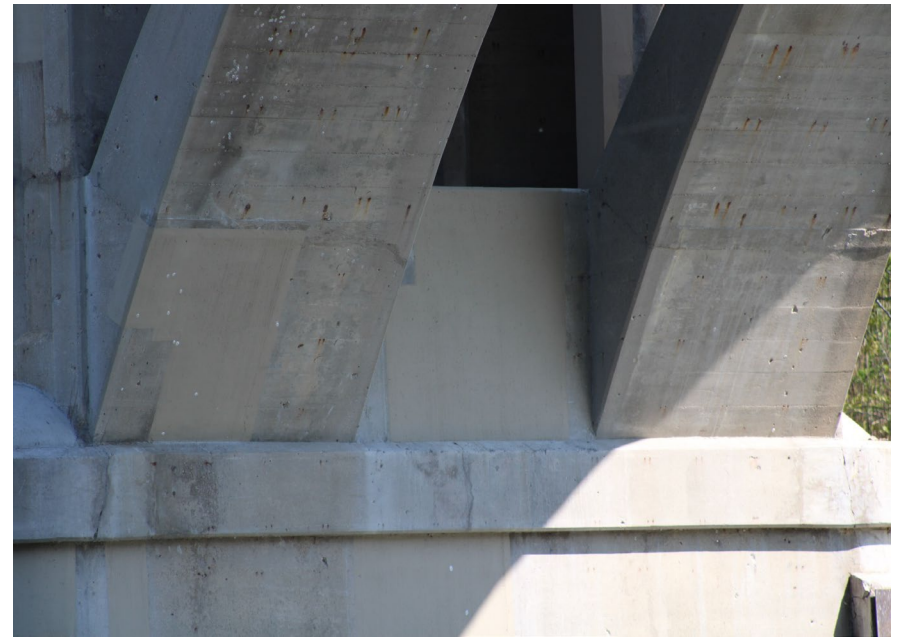
98. Looking North-East at Patching on S.N. 050-0096 underneath Span #6
