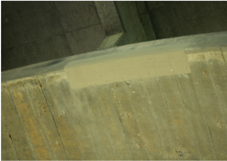
181. Looking directly up at patching underneath S.N. 050-0096 East Span #6
