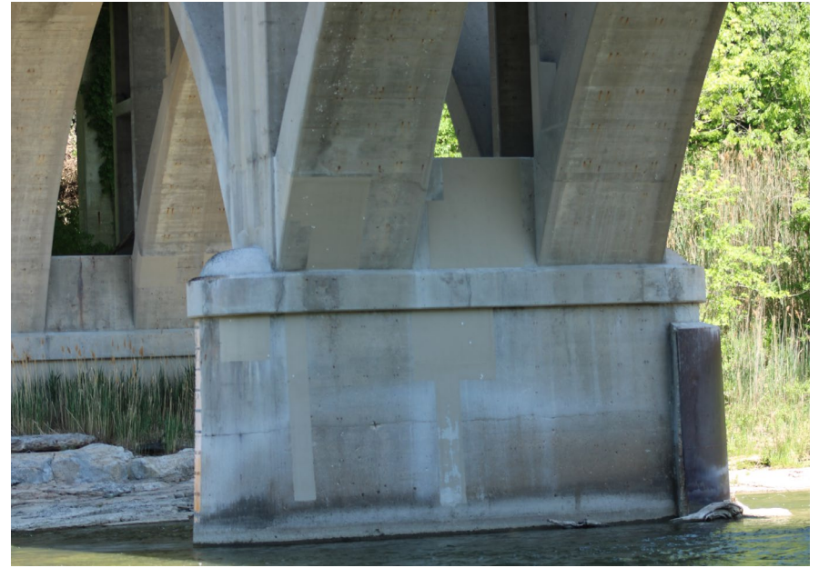
170. Looking North-East at Patching on S.N. 050-0096 South Profile of Pier #4
