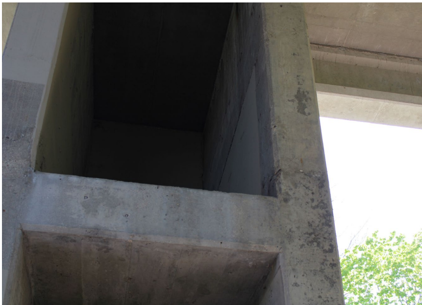
111. Looking East at Patching on S.N. 050-0096 inside East Pier #6
