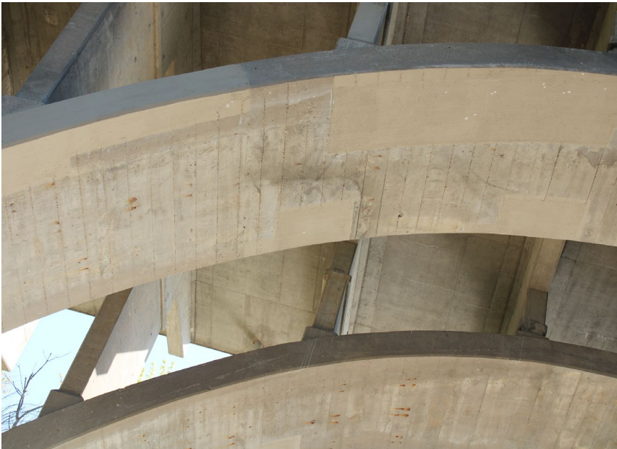
27. Looking East at Patching underneath S.N. 050-0096 West Span #4
