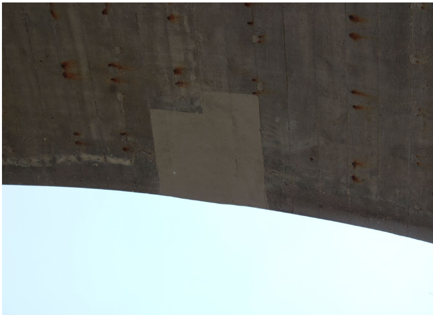
93. Looking East at Patching on S.N. 050-0096 underneath East Span #6
