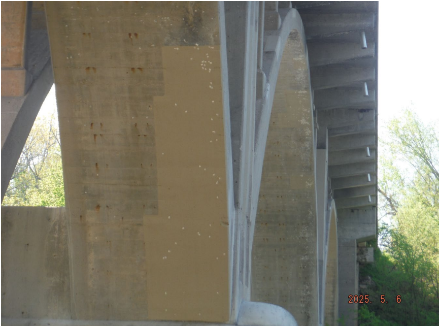
44. Looking South at Patching underneath S.N. 050-0096 West Span #4
