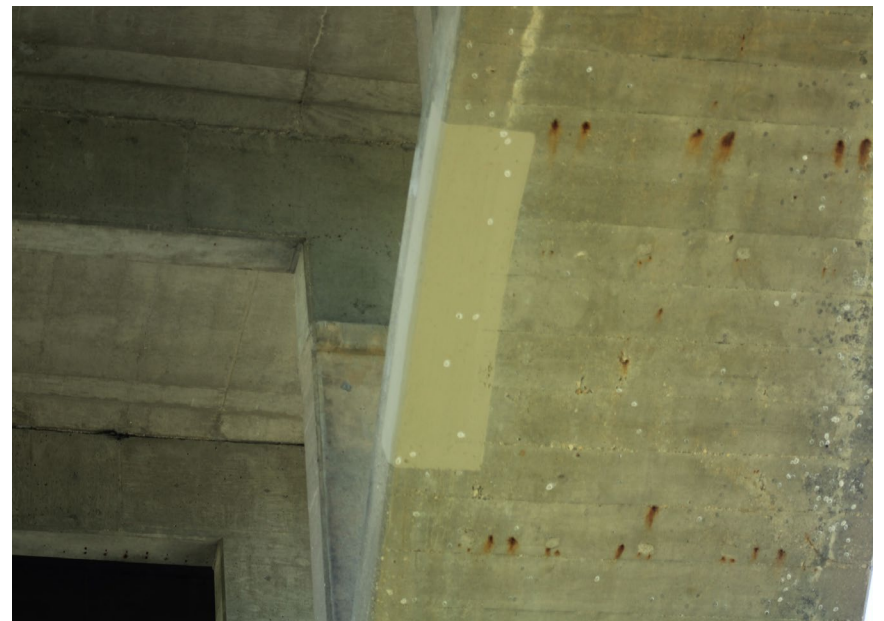
176. Looking North at Patching underneath S.N. 050-0096 East Span #6
