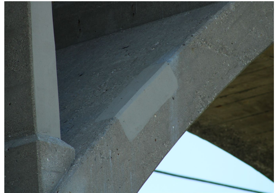
154. Looking North-West at Patching on S.N. 050-0096 East Profile of East Span #5
