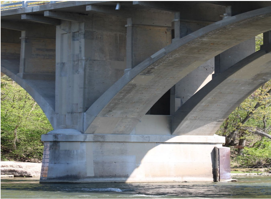
133. Looking North-East at S.N. 050-0096 West Profile of Pier #4
