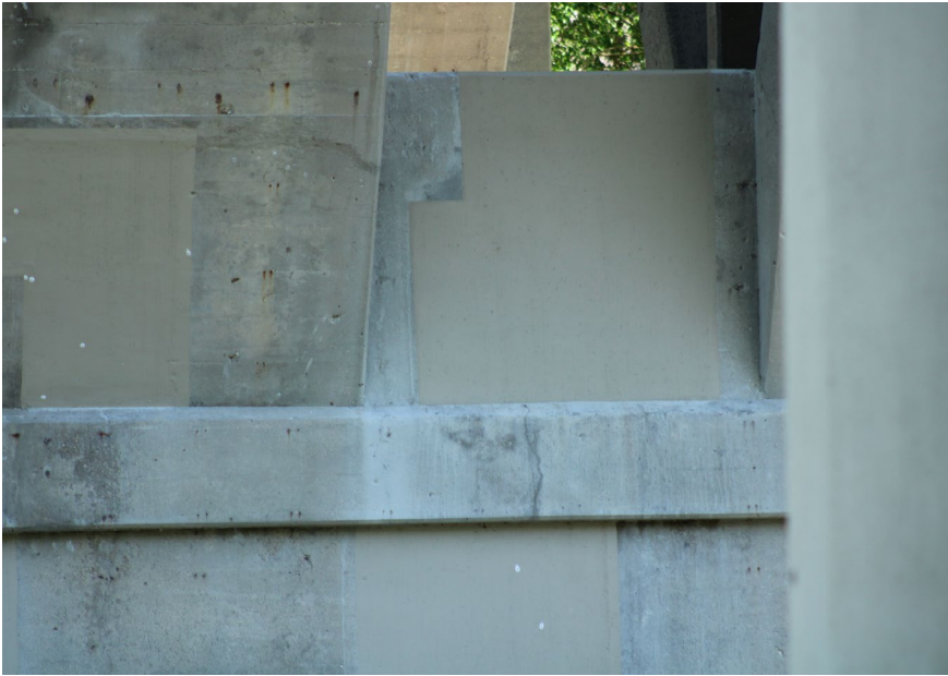
145. Looking North-East at Patching on S.N. 050-0096 South Profile of Pier #4
