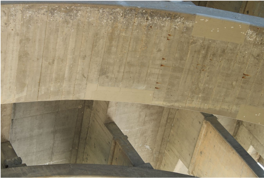
25. Looking East at Patching underneath S.N. 050-0096 West Span #4
