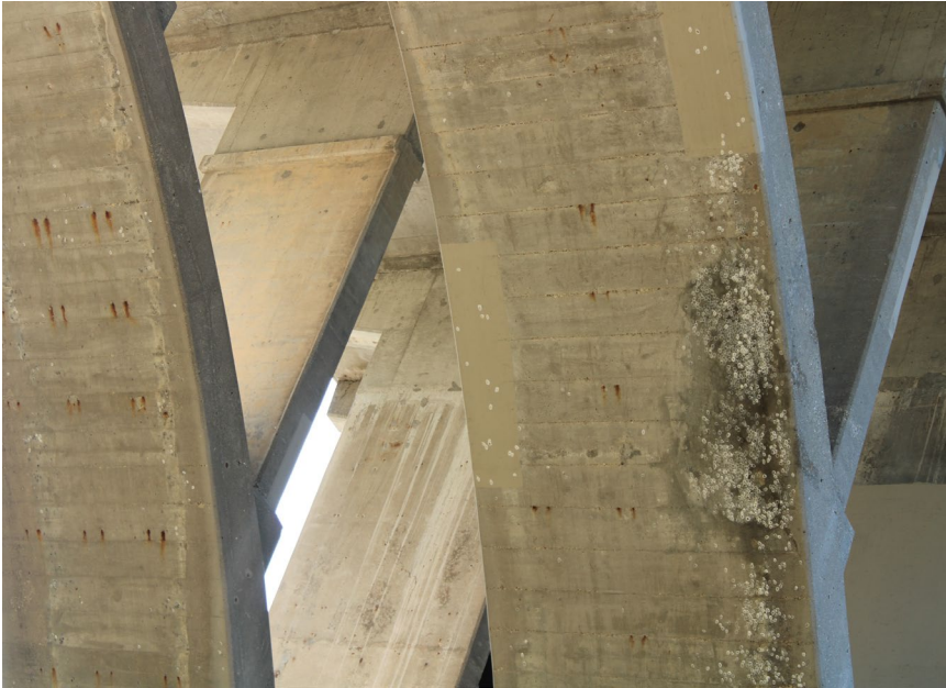
36. Looking South-East at Patching underneath S.N. 050-0096 West Span #4
