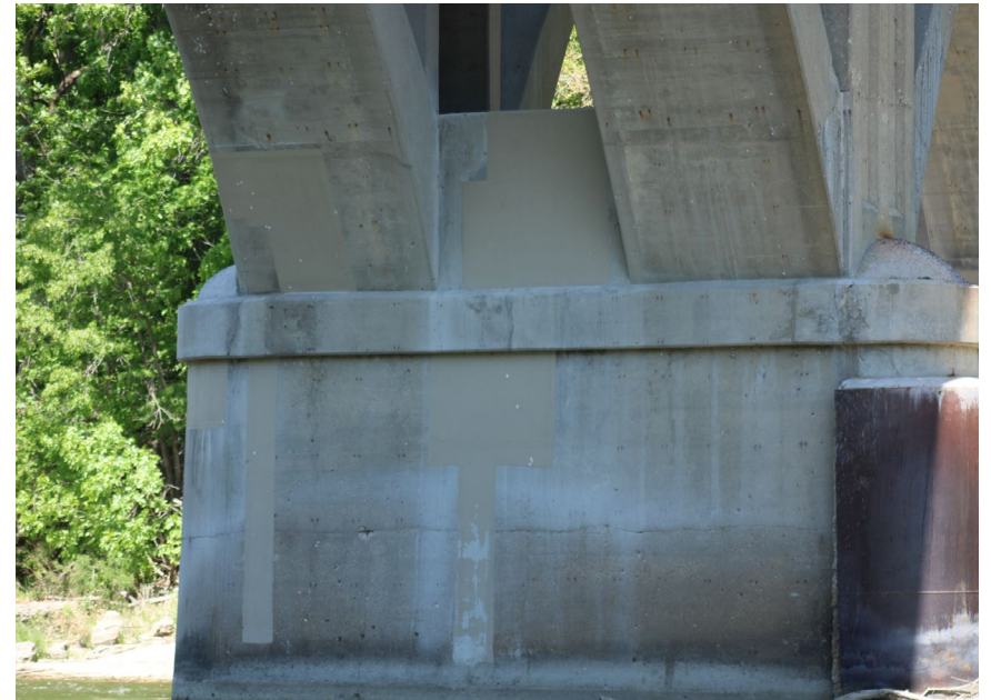
150. Looking North-West at Patching on S.N. 050-0096 South Profile of Pier #4
