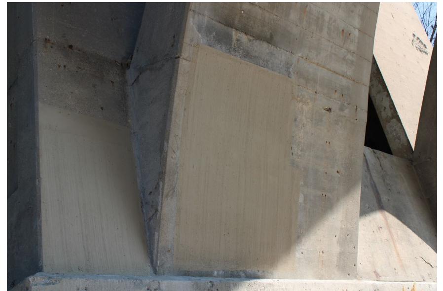
24. Looking North-East at Patching underneath S.N. 050-0096 West Span #4
