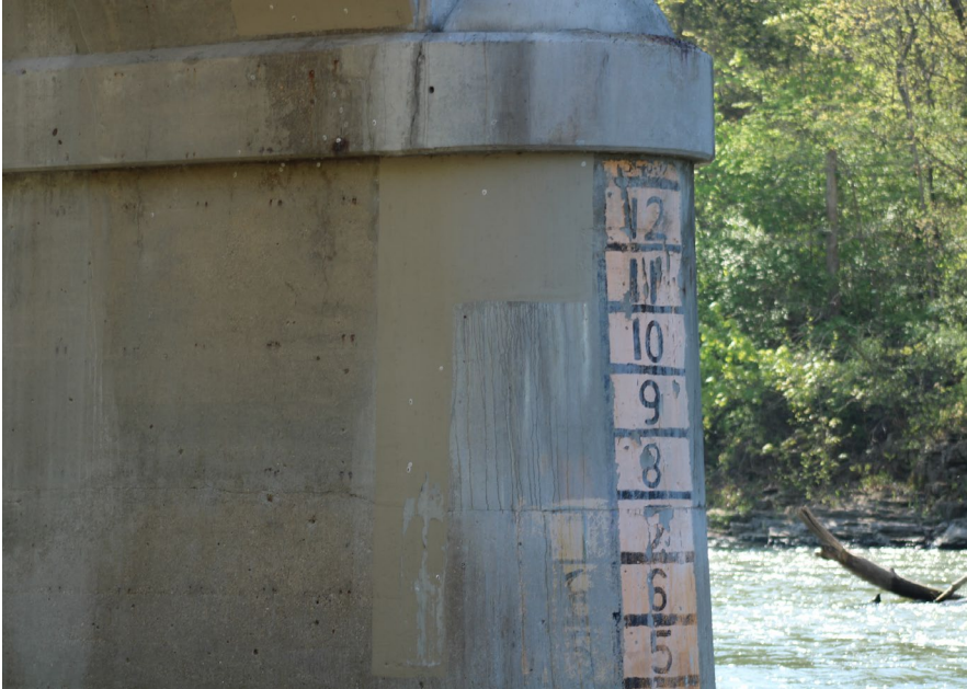
53. Looking South at Patching on the North Profile of S.N. 050-0096 Pier #4
