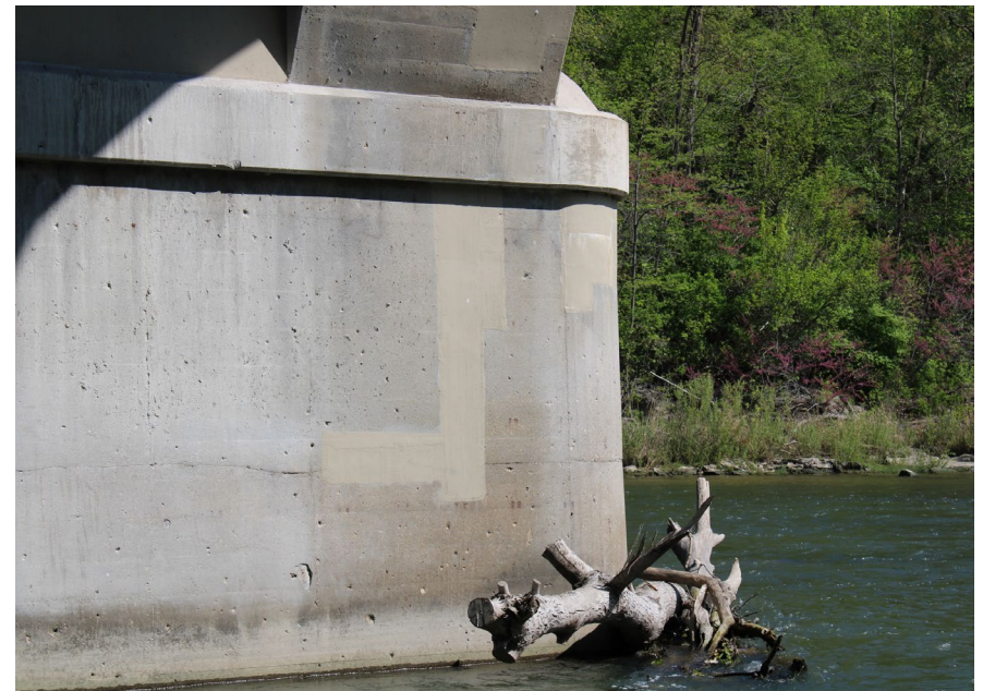
90. Looking North-East at Patching on S.N. 050-0096 South Profile of Pier #5
