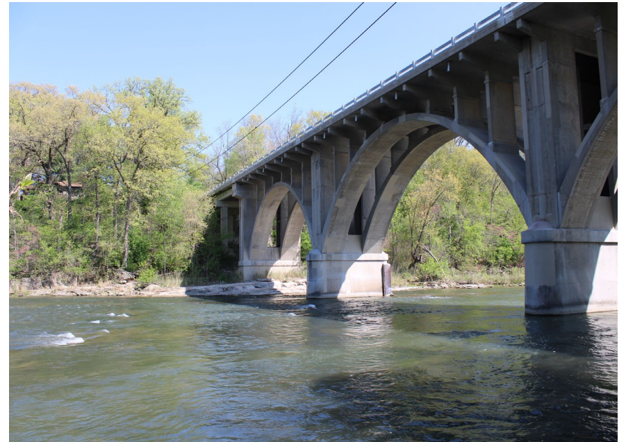
128. Looking North at S.N. 050-0096 West Profile
