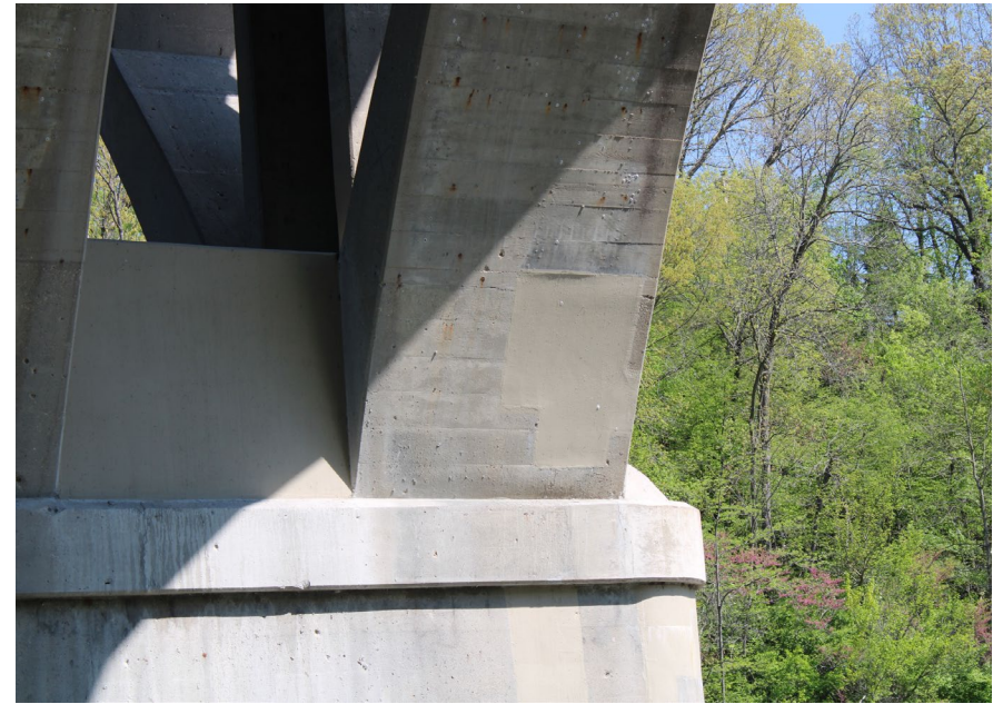
88. Looking North at Patching on S.N. 050-0096 underneath East Span #6
