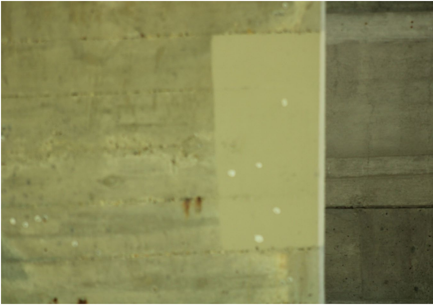
177. Looking North at Patching underneath S.N. 050-0096 Span #6
