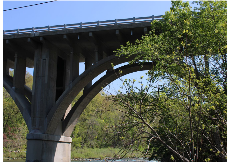
126. Looking East at S.N. 050-0096 West Profile of Span #6
