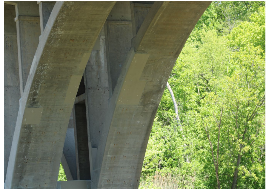
174. Looking North-East at Patching underneath S.N. 050-0096 Span #5
