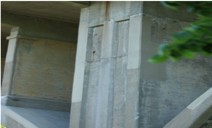
167. Looking North-East at Patching on S.N. 050-0096 West Profile of Pier #5
