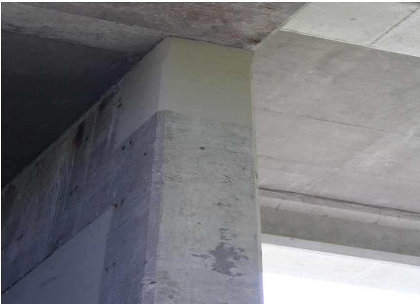
109. Looking East at Patching on S.N. 050-0096 inside East Pier #6
