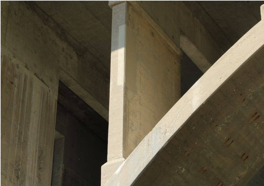
56. Looking West at Patching on S.N. 050-0096 East Span #4
