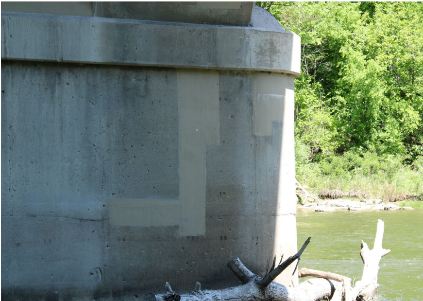
143. Looking North-East at Patching on S.N. 050-0096 South Profile of Pier #5
