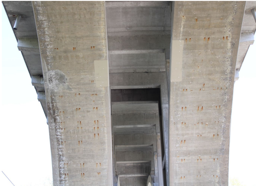
101. Looking North at Patching on S.N. 050-006 underneath Span #6
