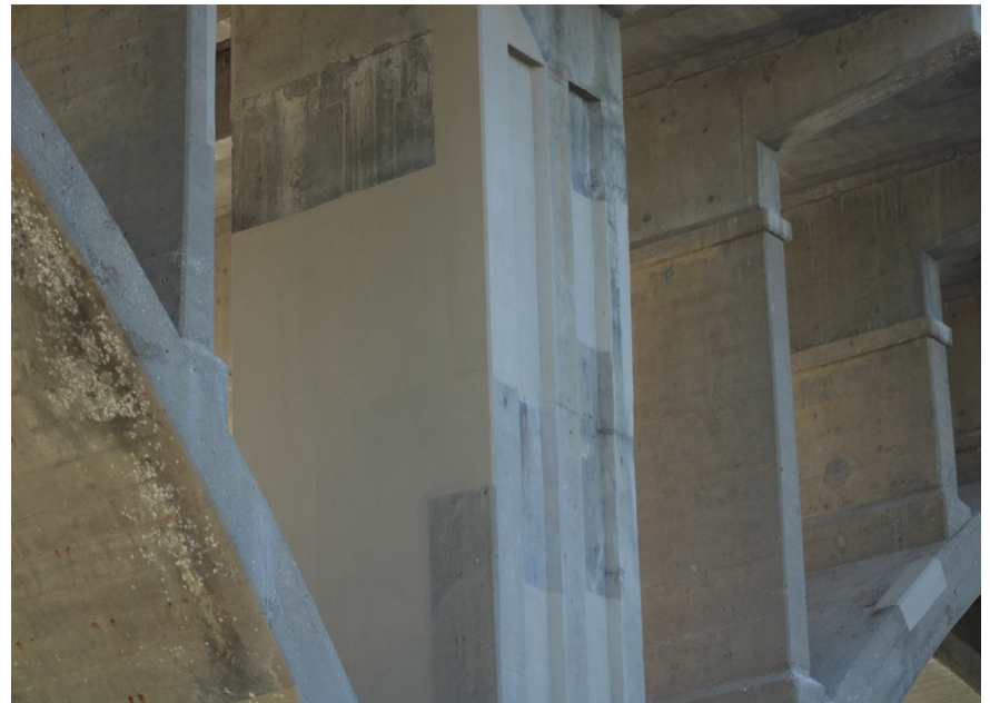
51. Looking South at Patching on the North Profile of S.N. 050-0096 Pier #4
