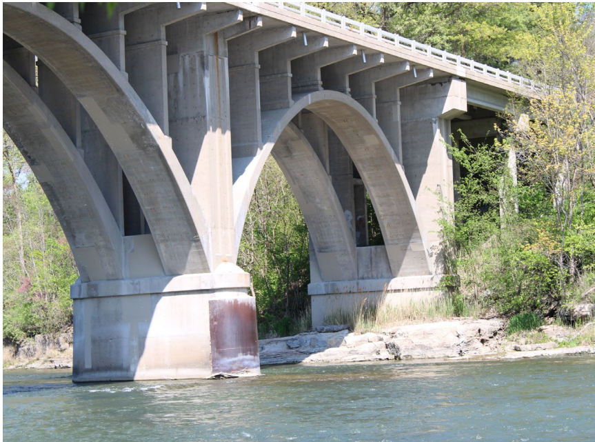
127. Looking North-West at S.N. 050-0096 East Profile of Span #4
