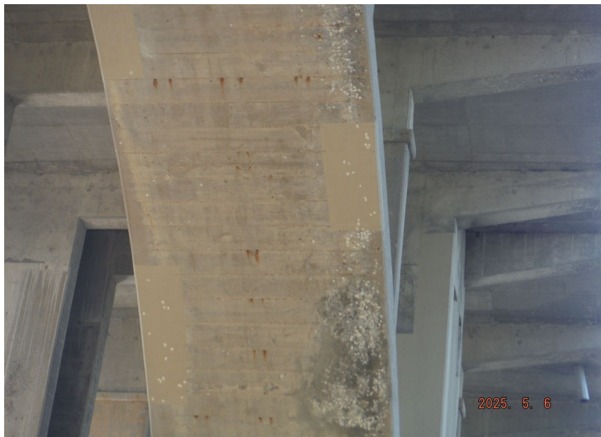
38. Looking South-East at Patching underneath S.N. 050-0096 West Span #4
