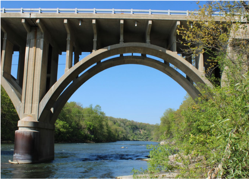
48. Looking West at Patching on S.N. 050-0096 Span #4
