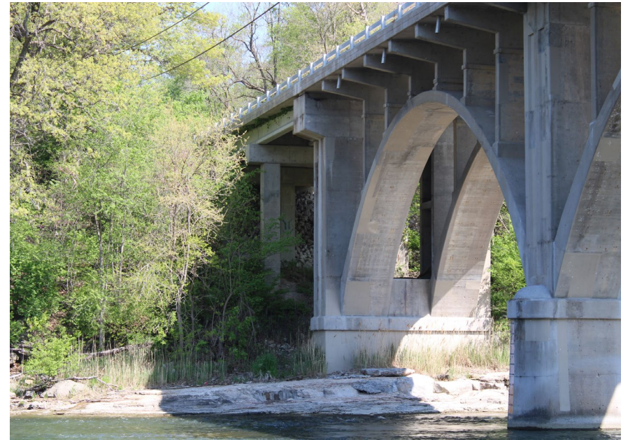
122. Looking North-East at S.N. 050-0096 West Profile of Span #4
