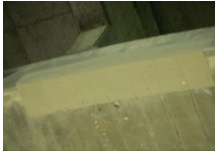
182. Looking directly up at patching underneath S.N. 050-0096 East Span #6
