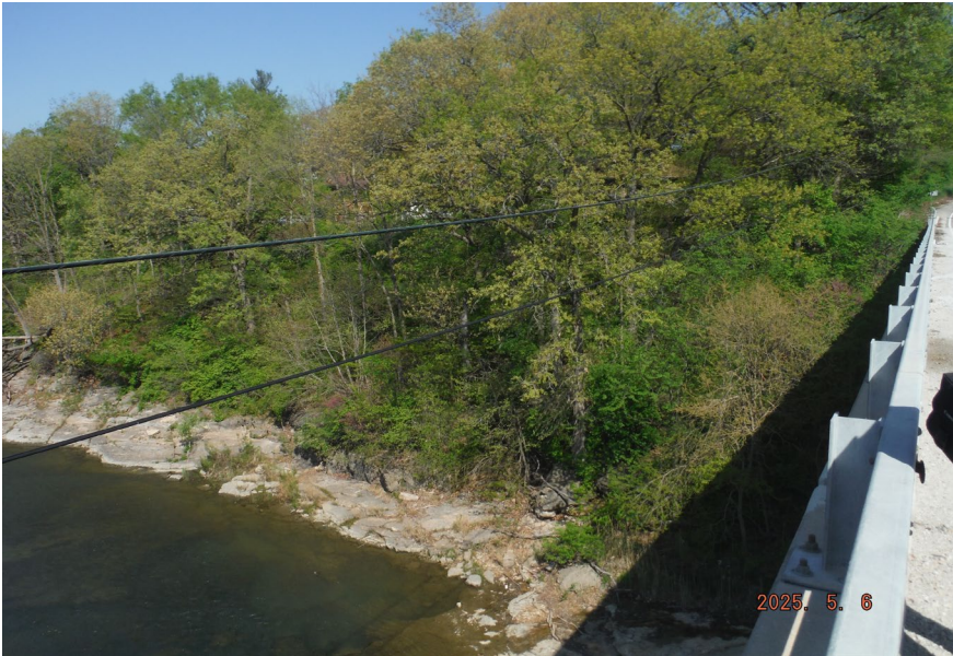
9. Looking North-West at the NW Quad of S.N. 050-0096 from S.N. 050-0096 at Sta. 196+85
