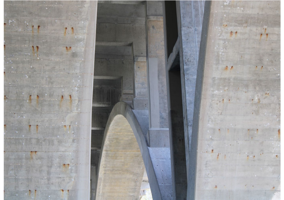
76. Looking North at Patching on S.N. 050-0096 West Profile of East Span #5
