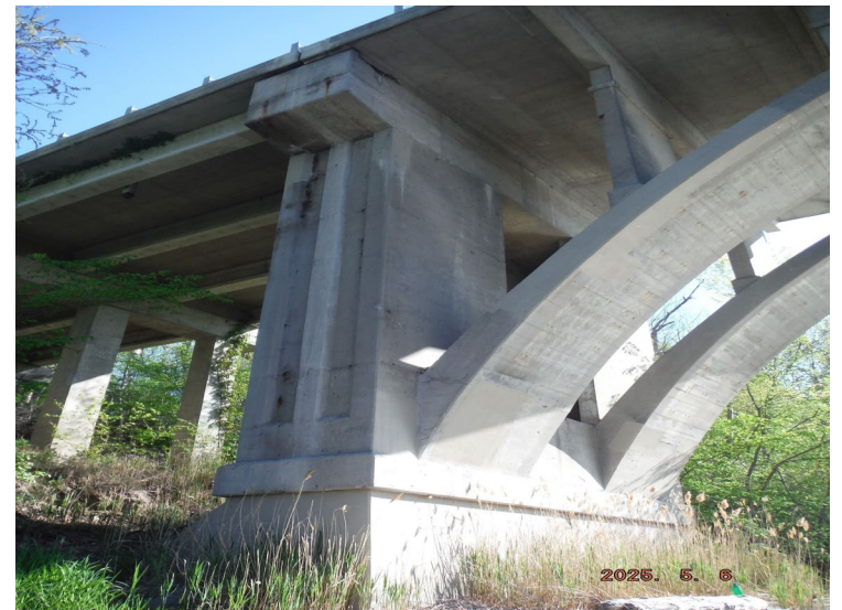
20. Looking East at Patching on the West Profile of S.N. 050-0096 West Pier #3
