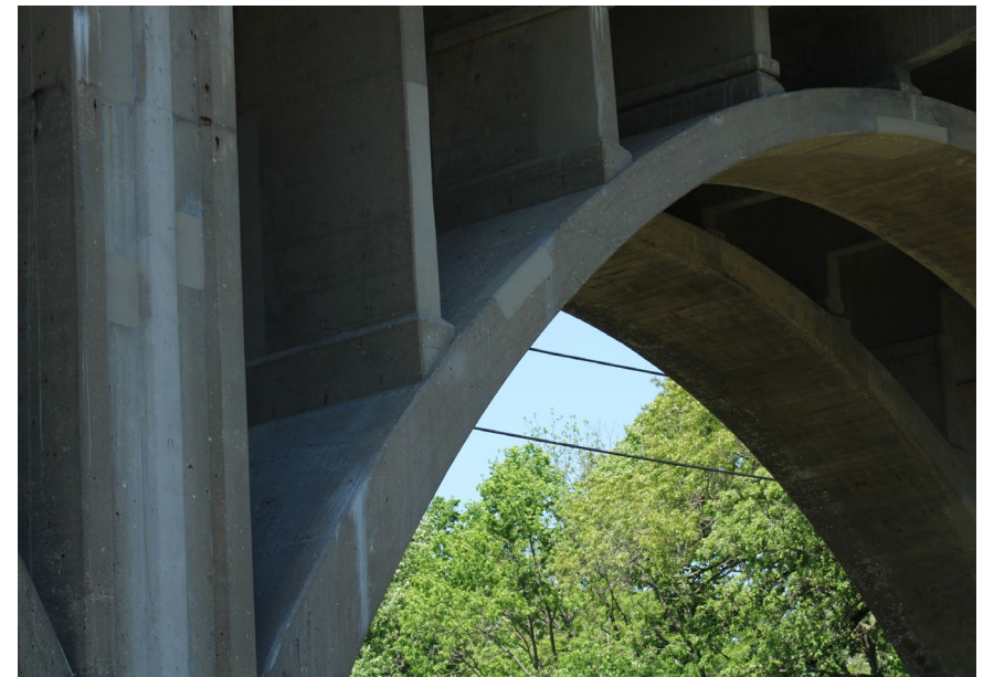
156. Looking North-West at Patching on S.N. 050-0096 East Profile of East Span #5
