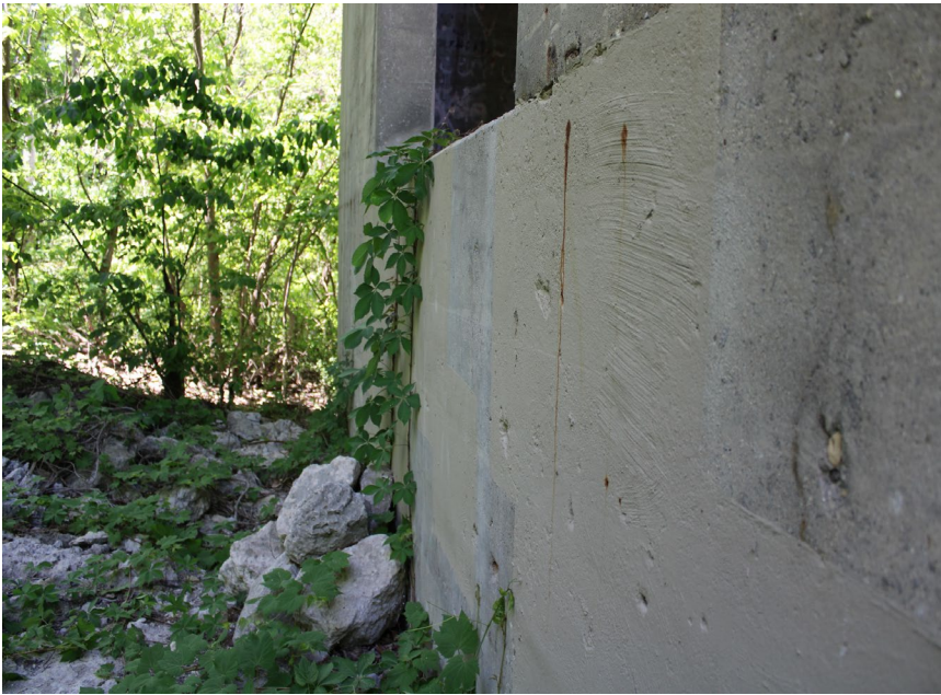
137. Looking West at Patching on S.N. 050-0096 South Profile of Pier #6
