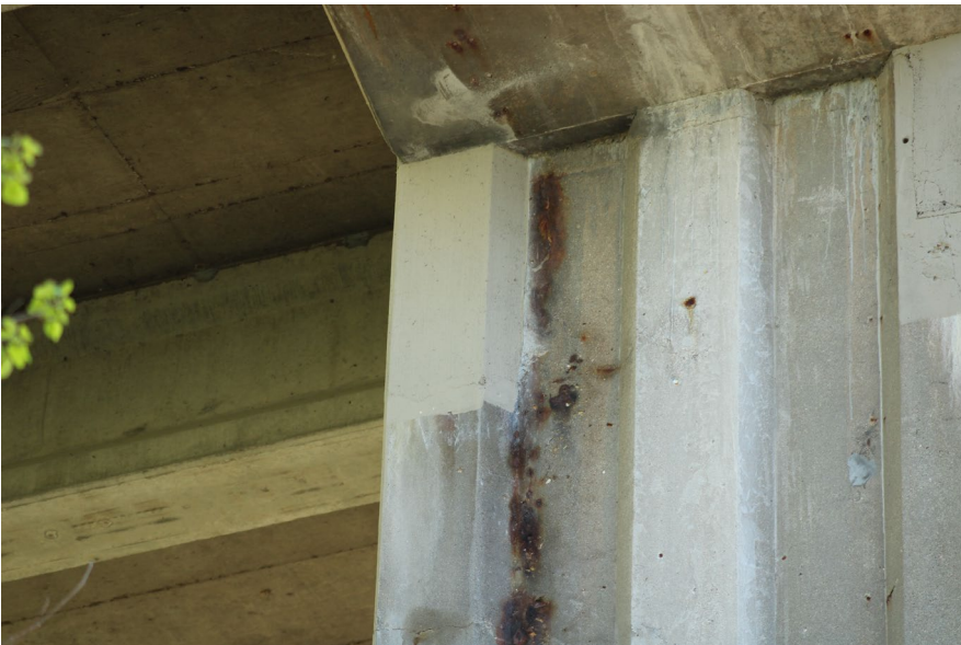
19. Looking East at Patching on the West Profile of S.N. 050-0096 West Pier #3
