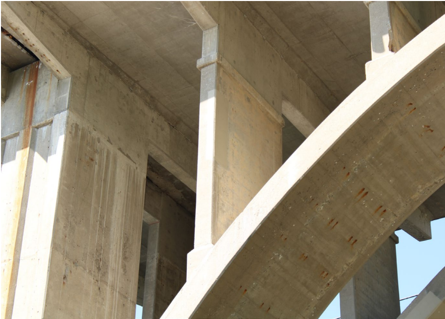
55. Looking West at Patching on S.N. 050-0096 East Span #4
