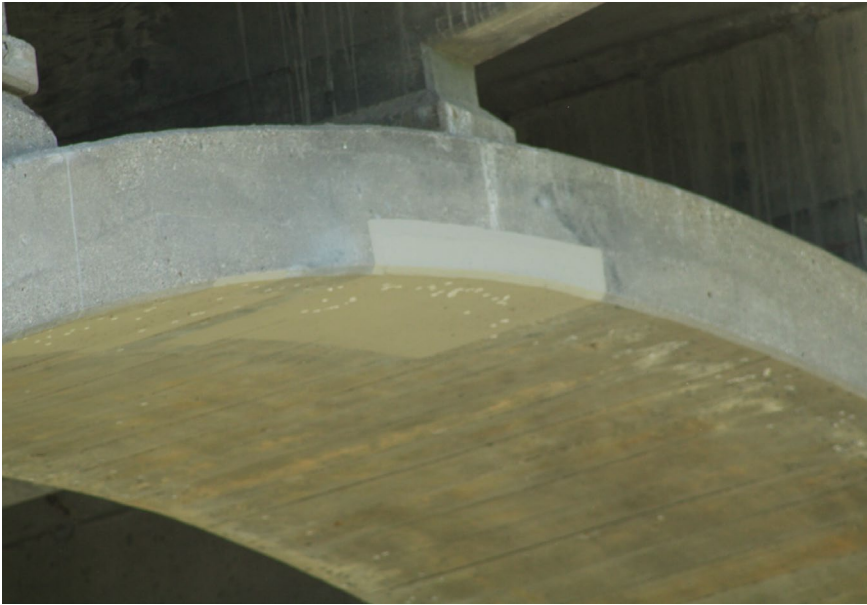
157. Looking North-West at Patching on S.N. 050-0096 East Profile of East Span #5
