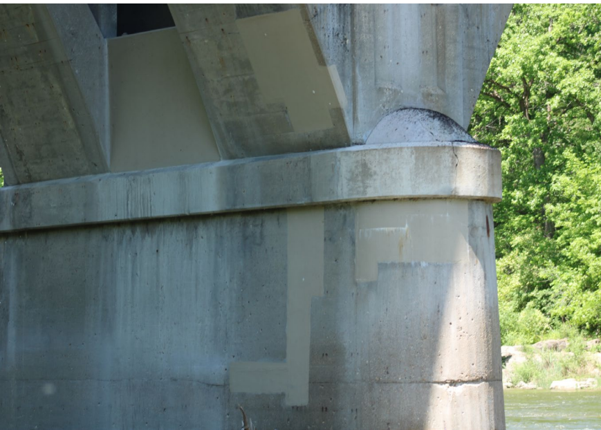
151. Looking North-West at Patching on S.N. 050-0096 South Profile of Pier #5
