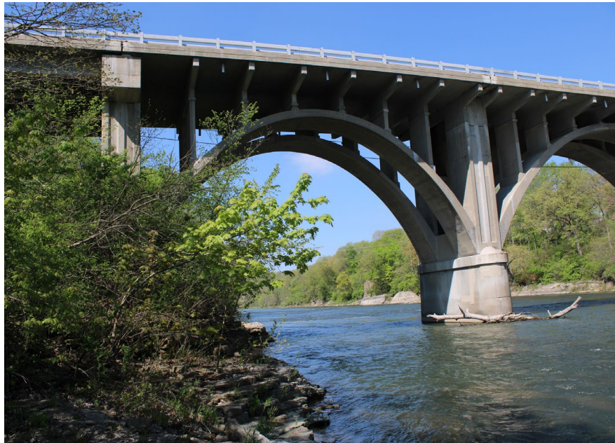
123. Looking West at S.N. 050-0096 East Profile of Span #6
