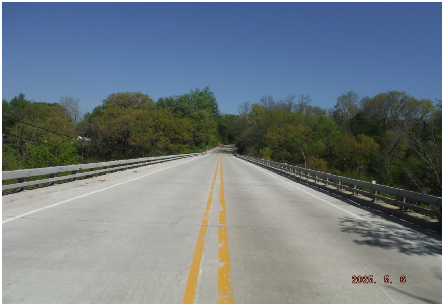
5. Looking North along IL 178 through S.N. 050-0096
