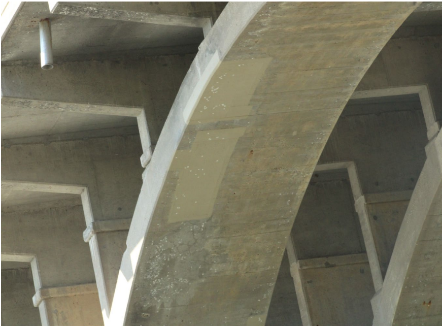
74. Looking South at Patching on S.N. 050-0096 underneath East Span #5
