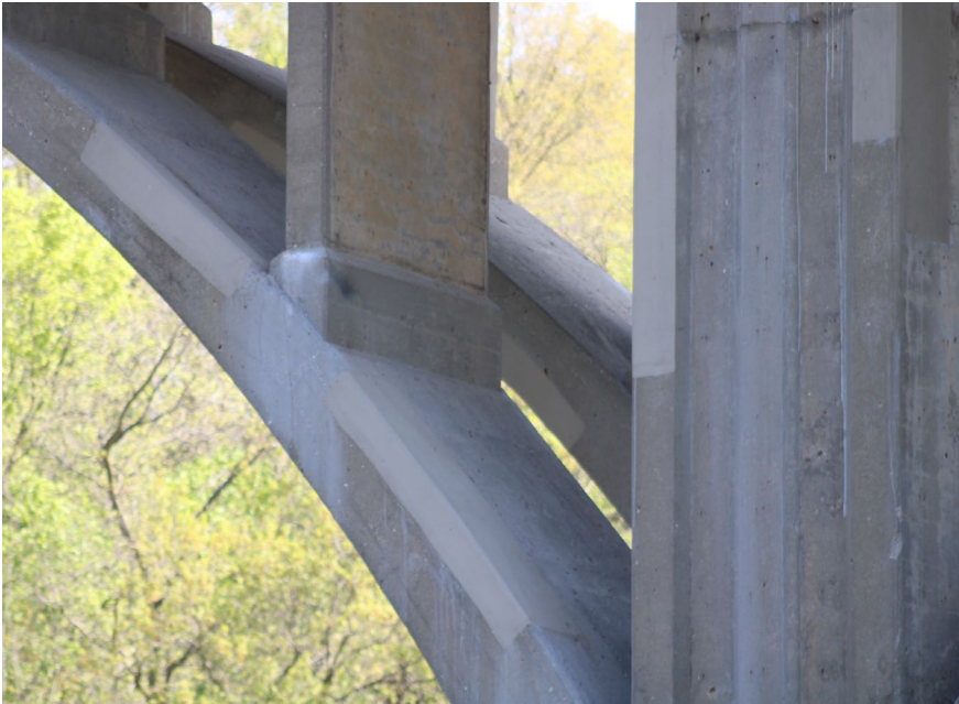
77. Looking North-East at S.N. 050-0096 West Span #5
