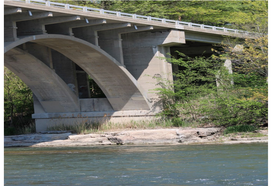
130. Looking North-West at S.N. 050-0096 East Profile of Pier #3
