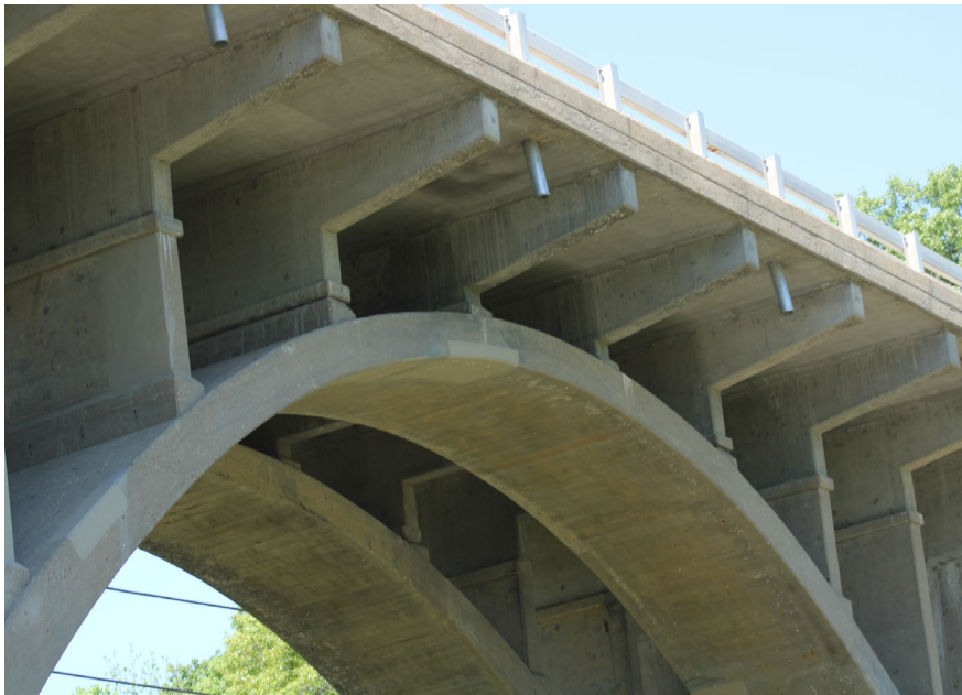
159. Looking North-West at Patching on S.N. 050-0096 East Profile of East Span #5
