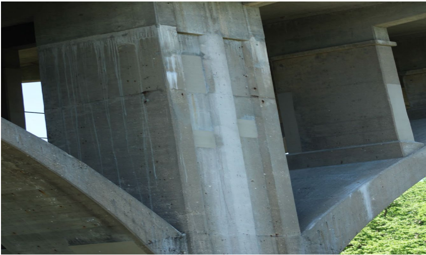
165. Looking North-West at Patching on S.N. 050-0096 East Profile of Pier #5
