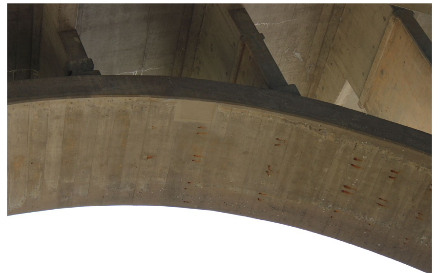
33. Looking East at Patching underneath S.N. 050-0096 West Span #4
