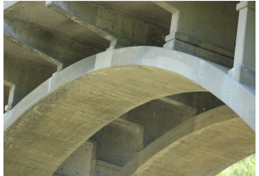
172. Looking North-East at Patching on S.N. 050-0096 West Profile of West Span #5
