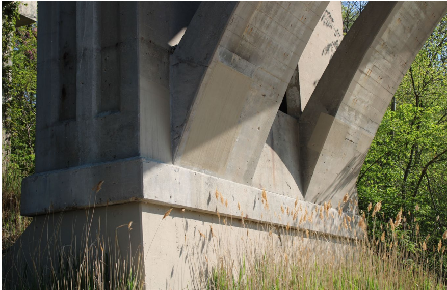
21. Looking North-East at Patching underneath S.N. 050-0096 Span #4
