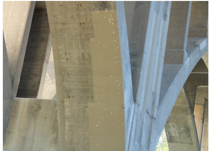
45. Looking South at Patching underneath S.N. 050-0096 West Span #4
