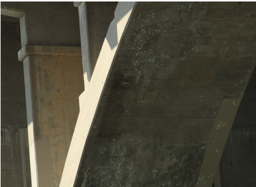
58. Looking West at Patching underneath S.N. 050-0096 East Span #5
