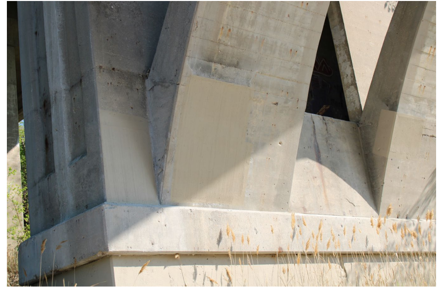
22. Looking North-East at Patching underneath S.N. 050-0096 West Span #4
