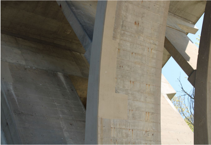
29. Looking North-East at Patching underneath S.N. 050-0096 West Span #4
