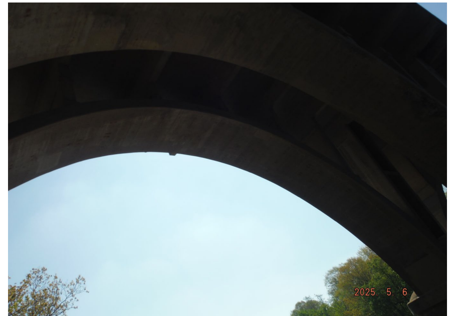
28. Looking East at Patching underneath S.N. 050-0096 Span #4
