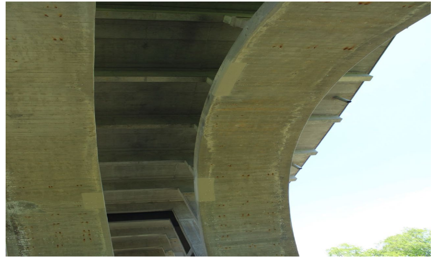
186. Looking North at Patching underneath S.N. 050-0096 Span #6
