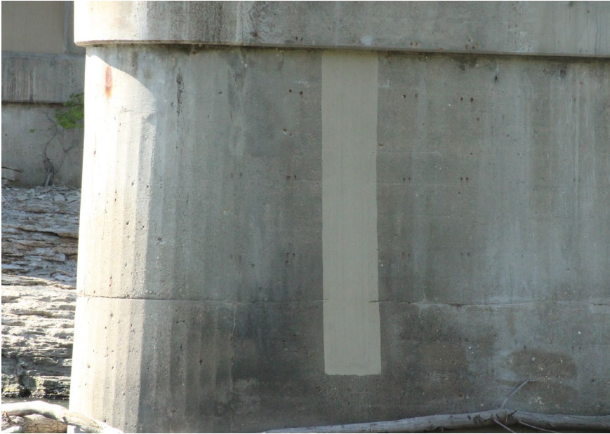
60. Looking South-West at Patching on S.N. 050-0096 Pier #5
