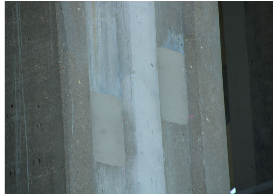
164. Looking North-West at Patching on S.N. 050-0096 East Profile of Pier #5
