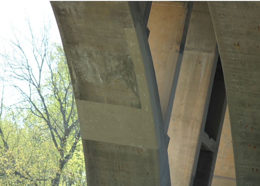
62. Looking South-East at Patching on S.N. 050-0096 East Span #5
