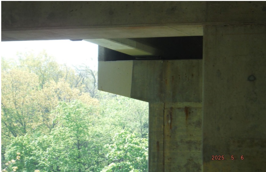
13. Looking South-East at Patching on the North Profile of S.N. 50-0096 East Pier #3
