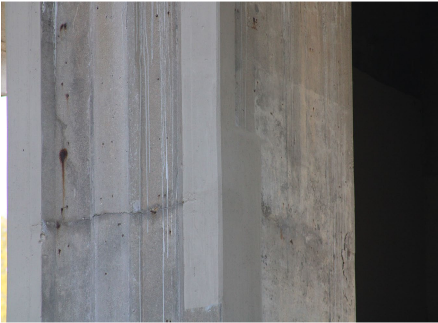
91. Looking North-East at Patching on S.N. 050-0096 West Profile of Pier #5
