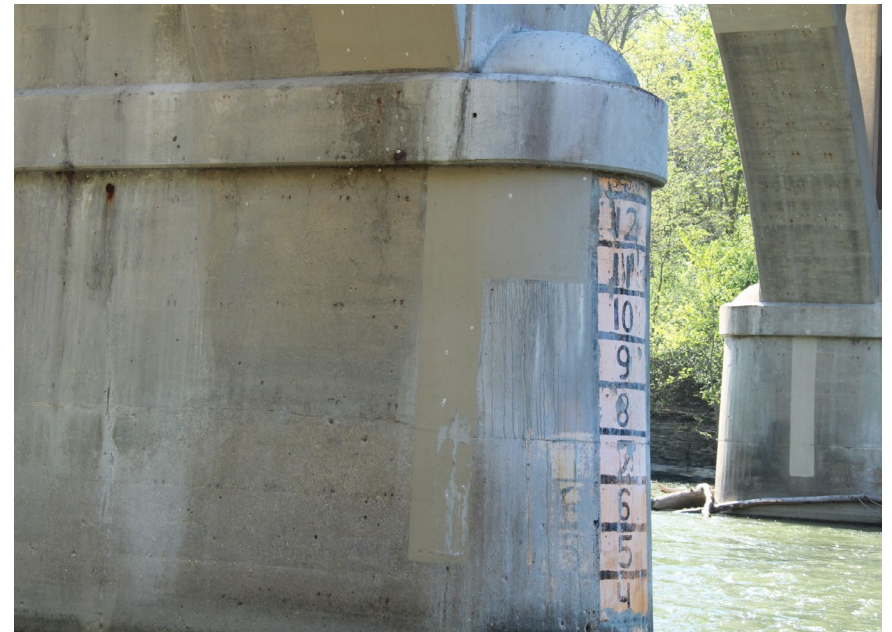
47. Looking South at Patching on the North Profile of S.N. 050-0096 Pier #4
