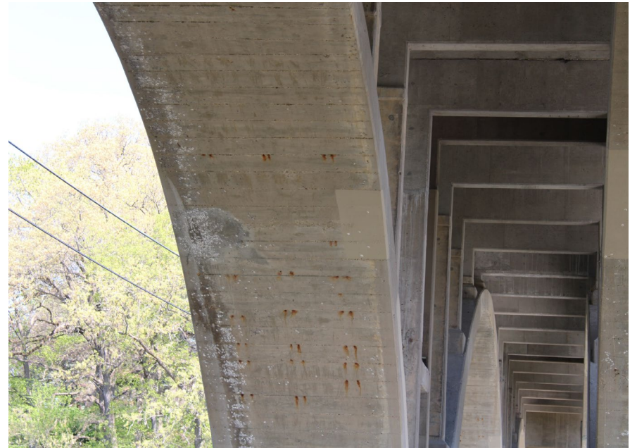
94. Looking North at Patching on S.N. 050-0096 underneath West Span #6
