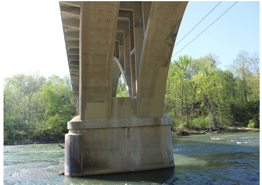
39. Looking South at Patching underneath S.N. 050-0096 Span #4
