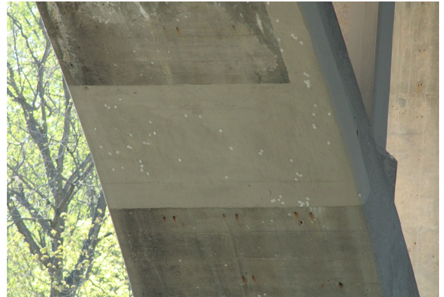
63. Looking South-East at Patching on S.N. 050-0096 East Span #5
