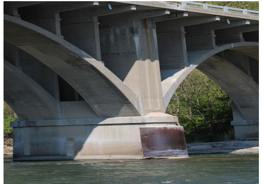
132. Looking North-West at S.N. 050-0096 East Profile of Pier #4
