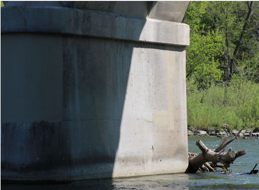
95. Looking East at Patching on S.N. 050-0096 South Profile of Pier #5
