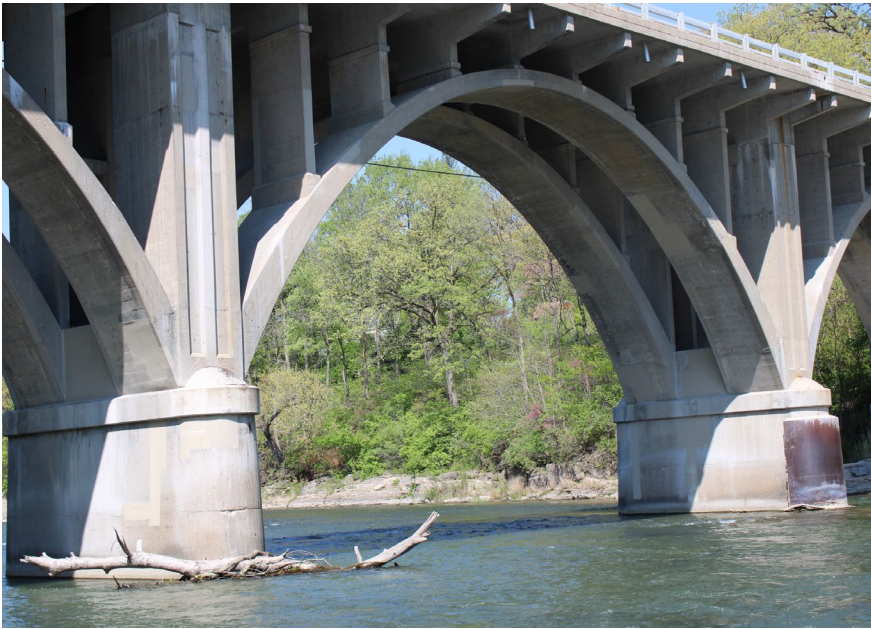
121. Looking North-West at S.N. 050-0096 East Profile of Span #5
