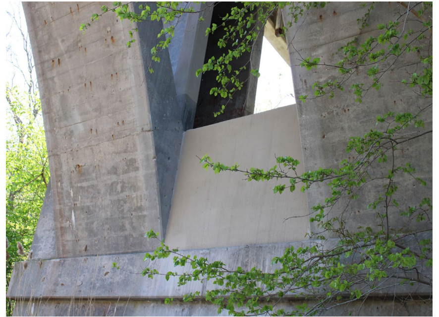
104. Looking South-East at Patching on S.N. 050-0096 North Profile of Pier #6
