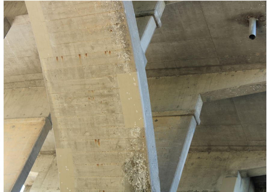
37. Looking South-East at Patching underneath S.N. 050-0096 West Span #4
