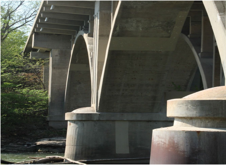
72. Looking South at Patching on S.N. 050-0096 underneath East Span #5
