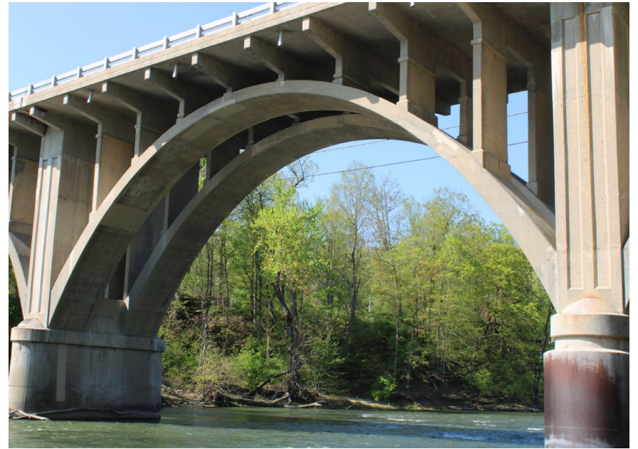
69. Looking South-West at S.N. 050-0096 Span #5
