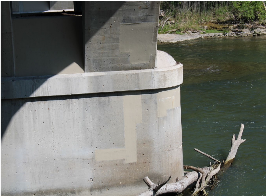
87. Looking North-East at Patching on S.N. 050-0096 South Profile of Pier #5
