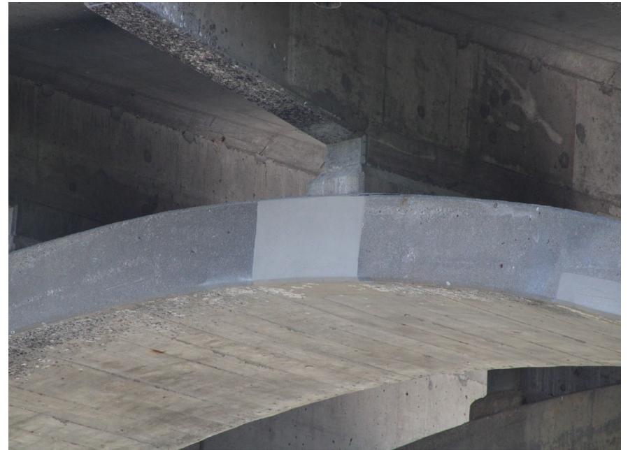
92. Looking North-East at Patching on S.N. 050-0096 West Span #5
