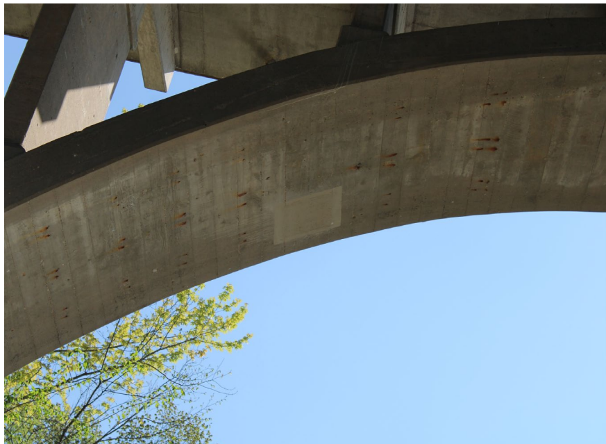
34. Looking East at Patching underneath S.N. 050-0096 East Span #4
