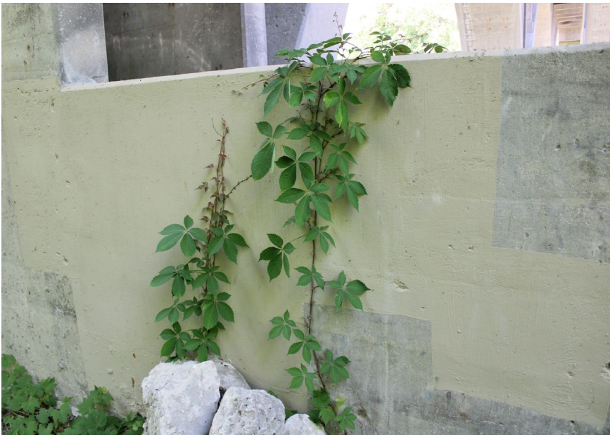
139. Looking North-West at Patching on S.N. 050-0096 South Profile of Pier #6
