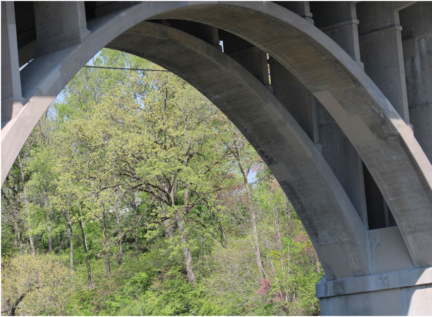
75. Looking North-West at Patching on S.N. 050-0096 underneath Span #5
