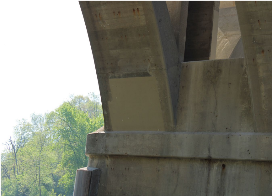
40. Looking South-East at Patching underneath S.N. 050-0096 East Span #4
