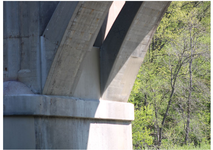
96. Looking East at Patching on S.N. 050-0096 underneath Span #6
