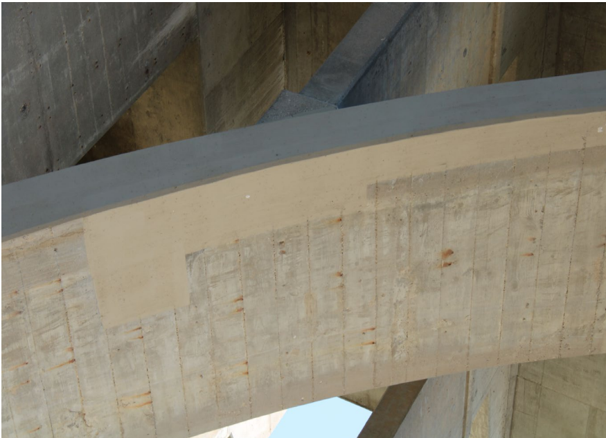
31. Looking East at Patching underneath S.N. 050-0096 West Span #4
