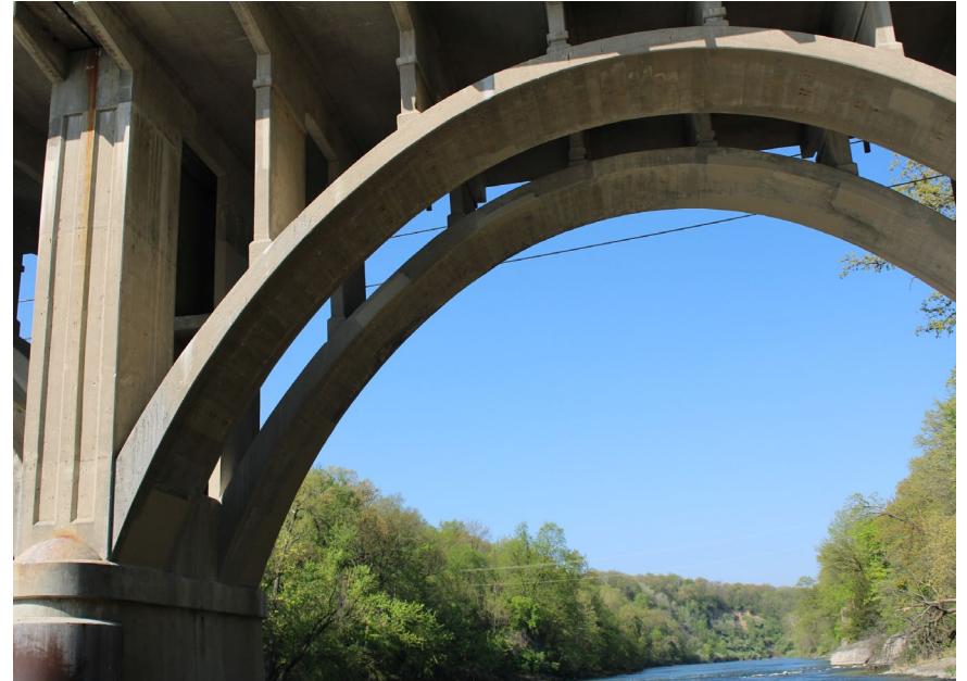
49. Looking West at Patching on S.N. 050-0096 Span #4
