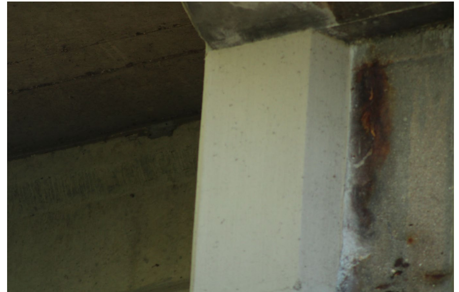
18. Looking East at Patching on the West Profile of S.N. 050-0096 West Pier #3
