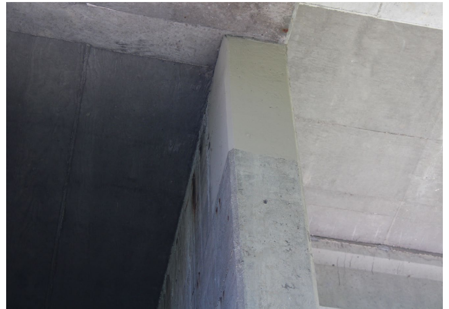
110. Looking East at Patching on S.N. 050-06 inside East Pier #6
