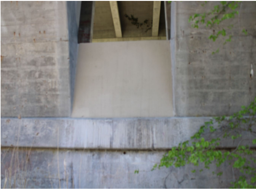
103. Looking South at Patching on S.N. 050-0096 North Profile of Pier #6
