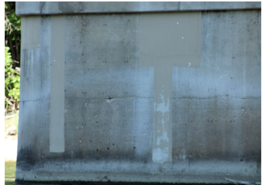
152. Looking North-West at Patching on S.N. 050-0096 South Profile of Pier #4
