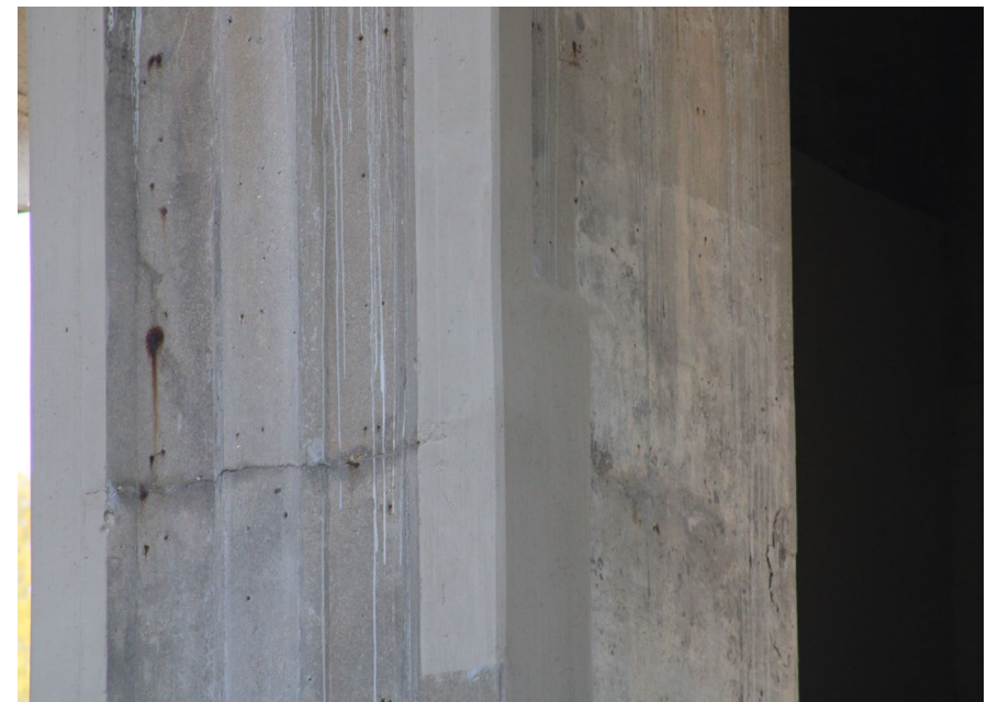
78. Looking North-East at S.N. 050-0096 West Profile of Pier #5
