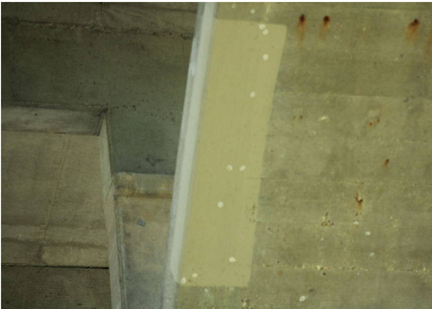
175. Looking North at Patching underneath S.N. 050-0096 East Span #6
