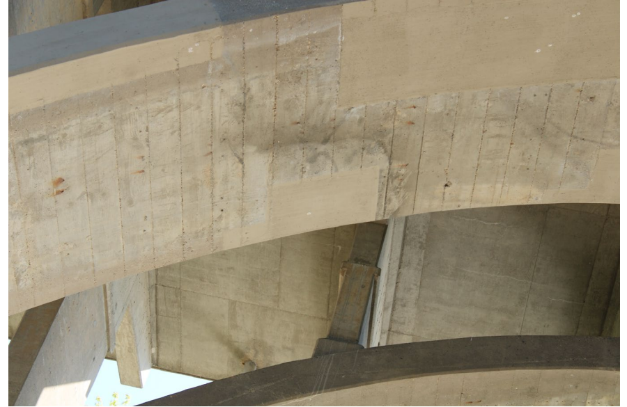
26. Looking East at Patching underneath S.N. 050-0096 West Span #4
