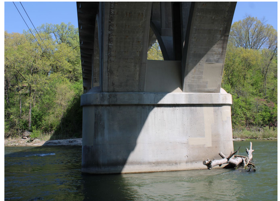
86. Looking North at Patching on S.N. 050-0096 underneath Span #6
