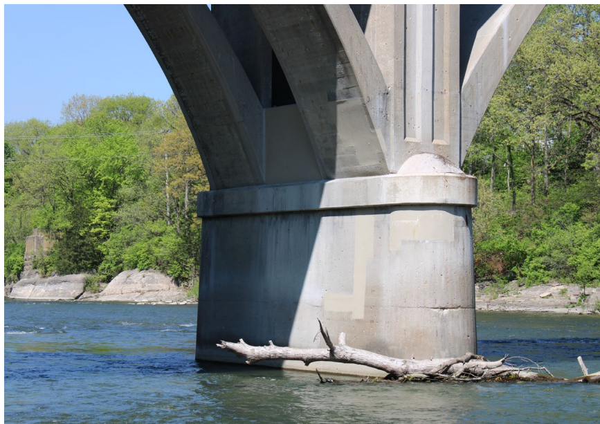
81. Looking West at Patching on S.N. 050-0096 Pier #5
