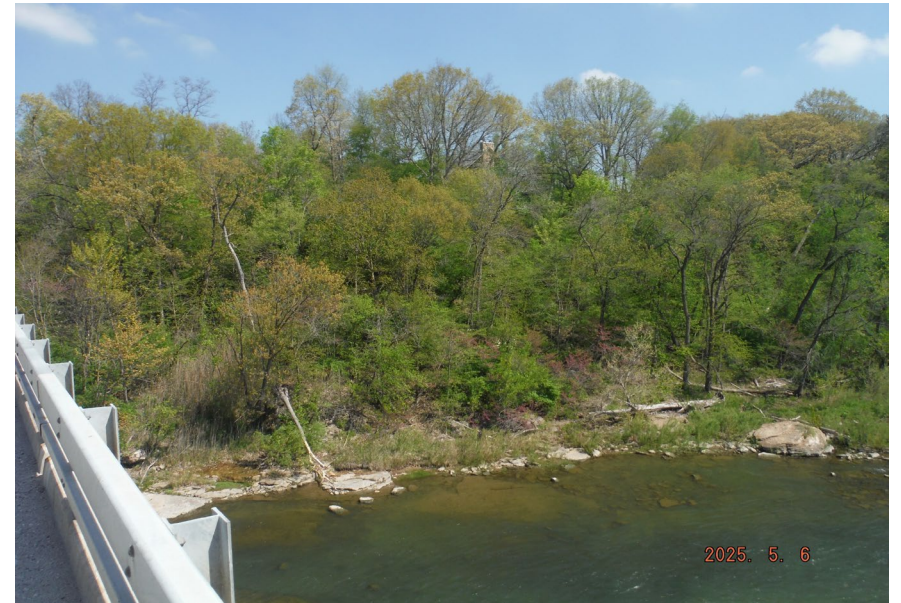
10. Looking North-East at the NE Quad of S.N. 050-0096 at Sta. 196+85
