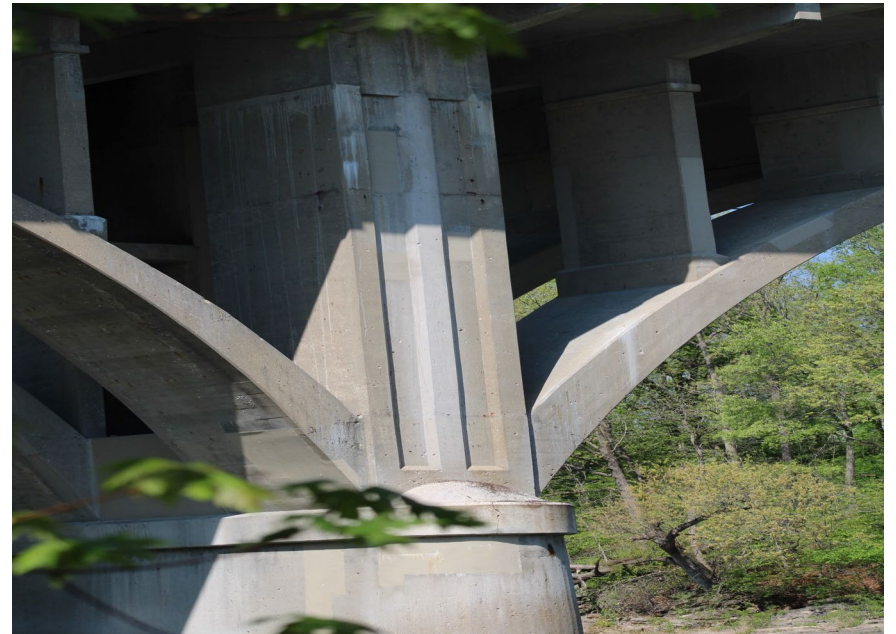
136. Looking West at S.N. 050-0096 East Profile of Pier #5
