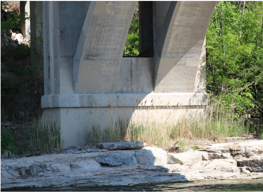
129. Looking North-East at Patching underneath S.N. 050-0096 Span #4
