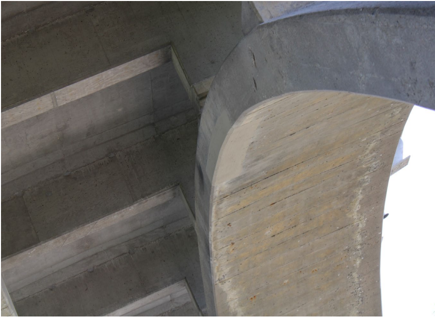
99. Looking North-East at Patching on S.N. 050-0096 East Span #6
