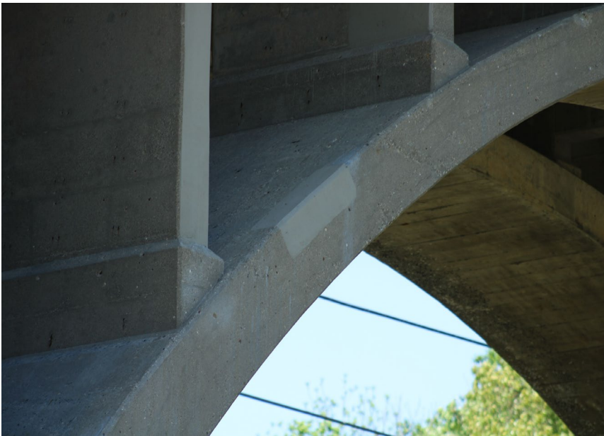
155. Looking North-West at Patching on S.N. 050-0096 East Profile of East Span #5
