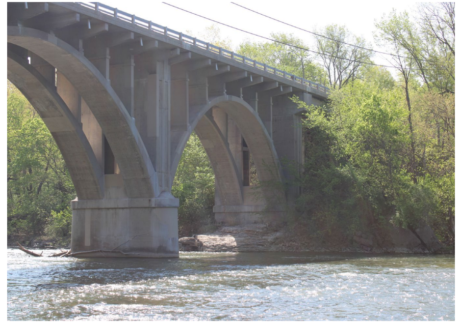
118. Looking South-East at S.N. 050-0096 West Profile of Span #6
