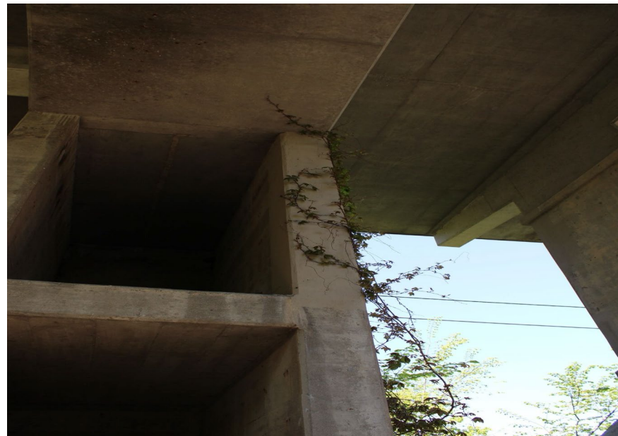
112. Looking West at Patching on S.N. 050-0096 inside West Pier #6
