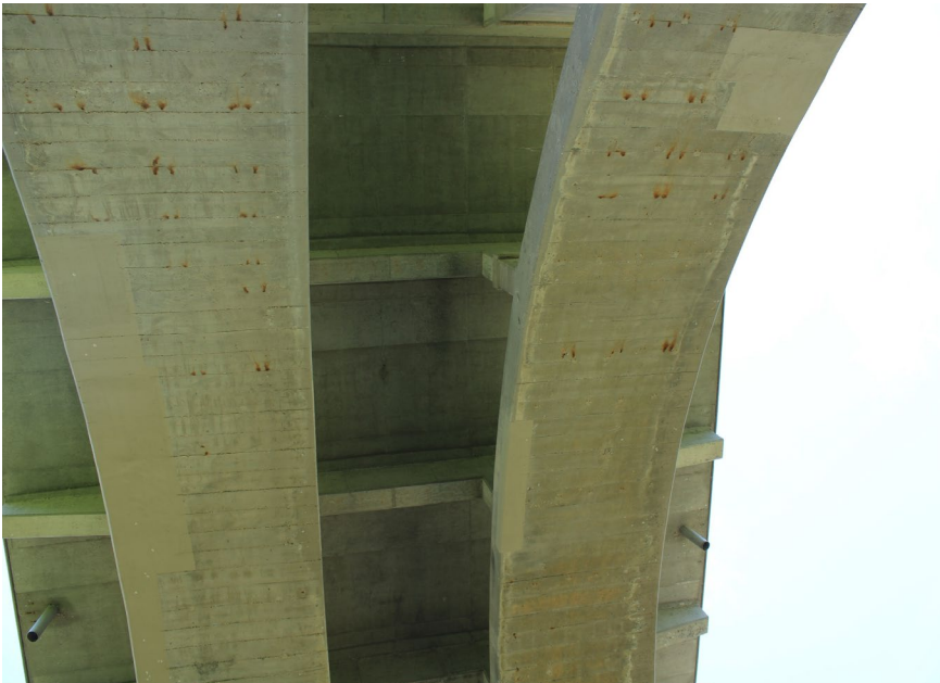
183. Looking directly up at Patching underneath S.N. 050-0096 Span #6
