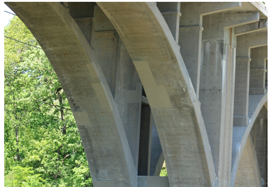
146. Looking North-West at Patching underneath S.N. 050-0096 Span #5
