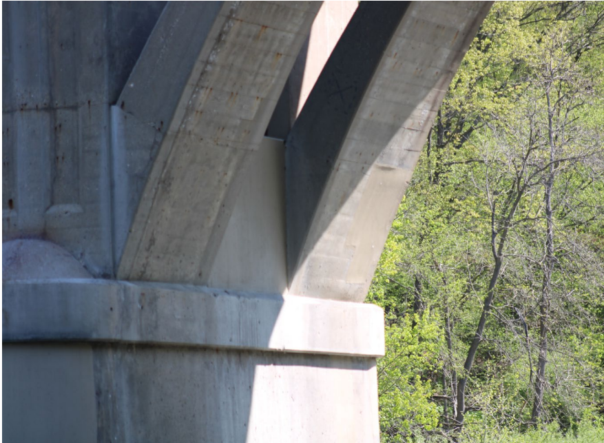
85. Looking East at Patching on S.N. 050-0096 underneath Span #6
