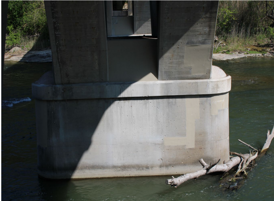
89. Looking North at Patching on S.N. 050-0096 underneath Span #6
