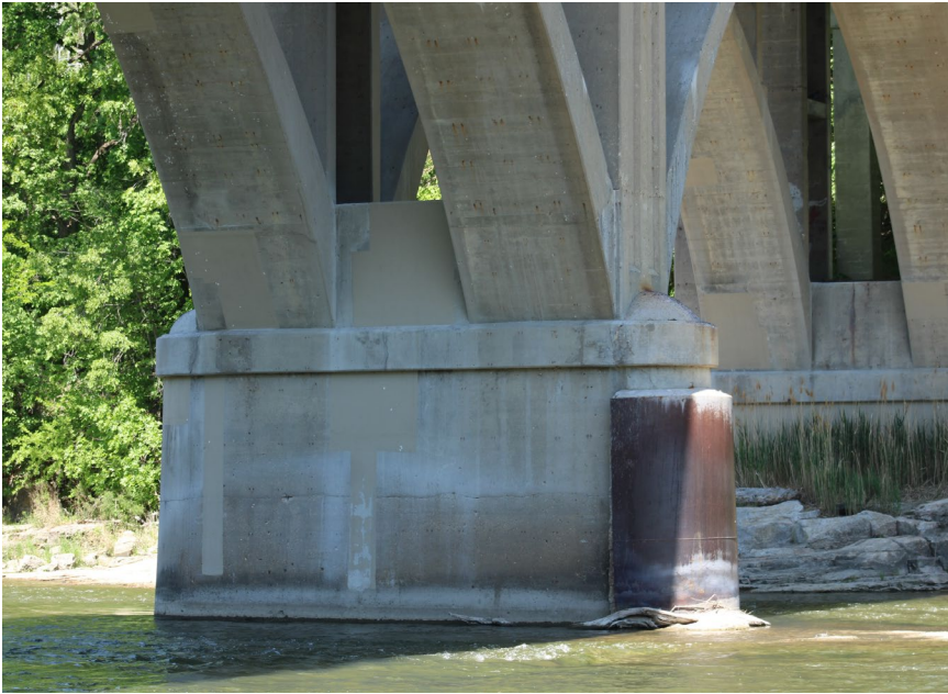
153. Looking North-West at Patching on S.N. 050-0096 Pier #4
