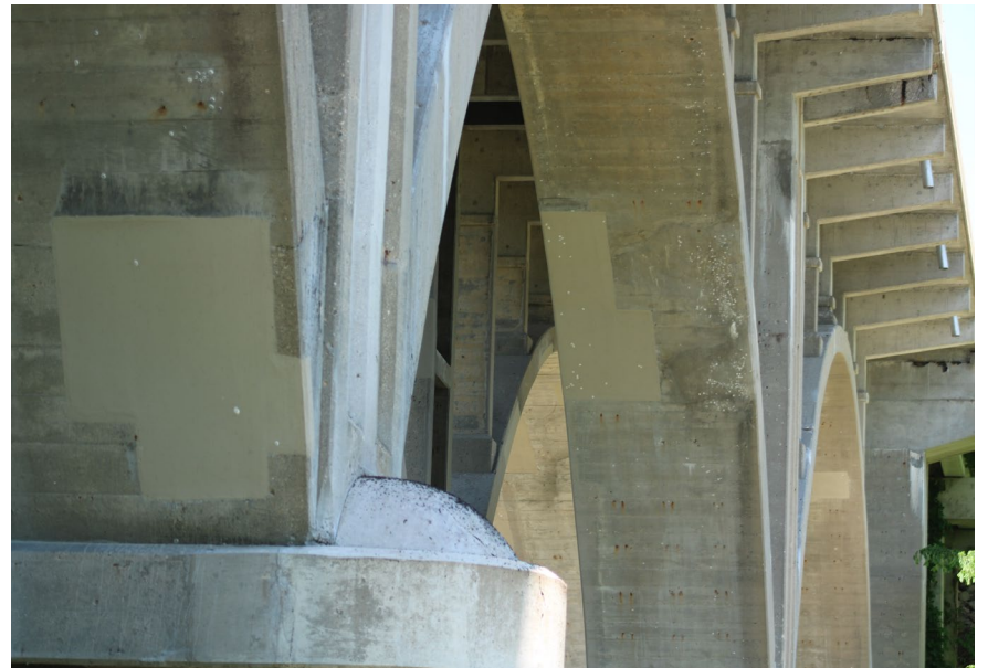
148. Looking North at Patching underneath S.N. 050-0096 East Span #5
