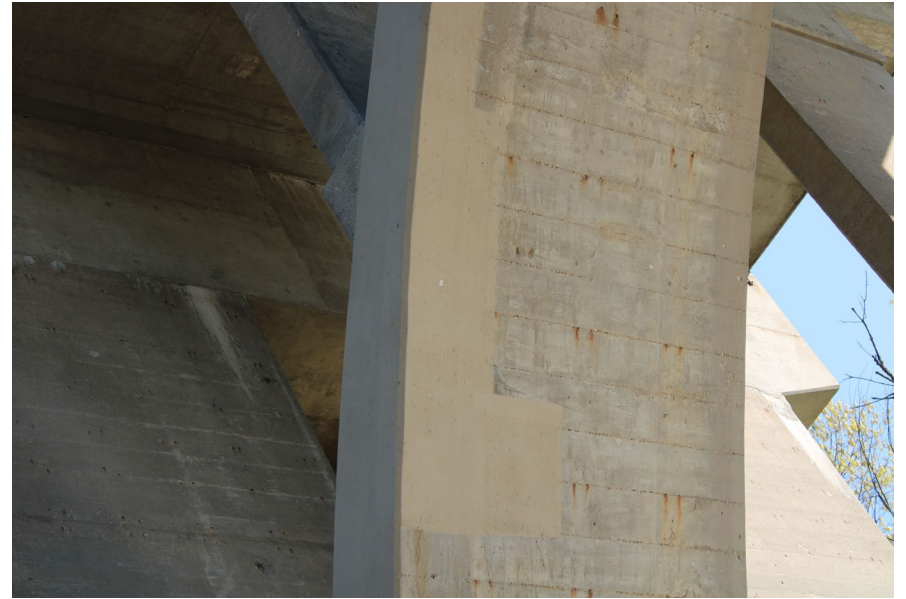
30. Looking North-East at Patching underneath S.N. 050-0096 West Span #4
