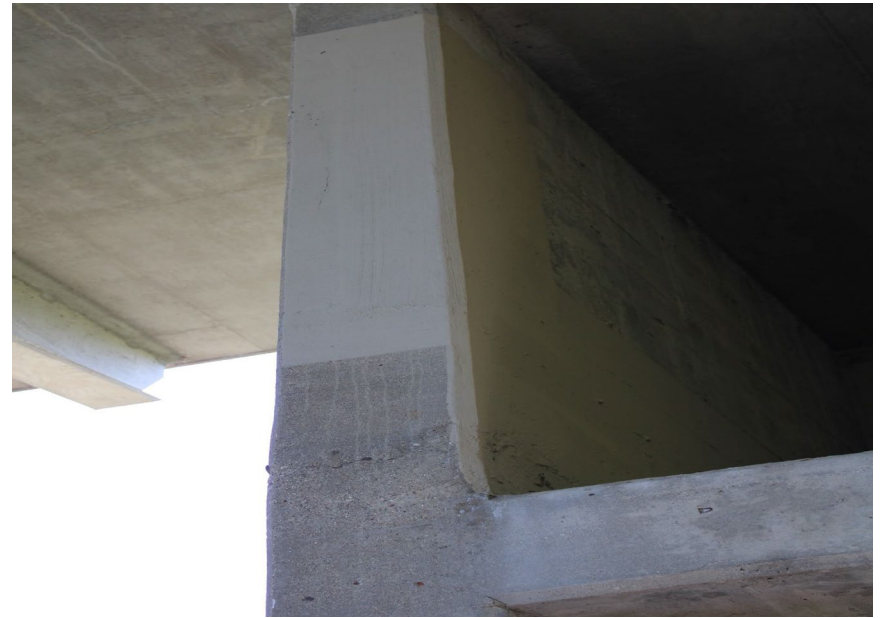
108. Looking East at Patching on S.N. 050-0096 inside East Pier #6
