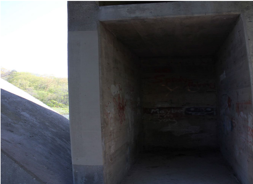
107. Looking East at Patching on S.N. 050-0096 inside East Pier #6
