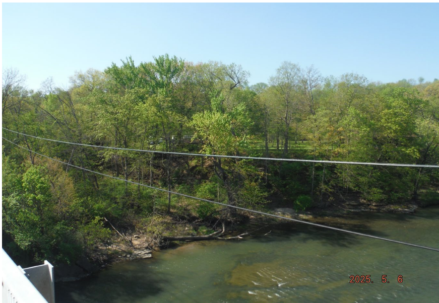
11. Looking South-West at the SW Quad of S.N. 050-0096 at Sta. 196+85
