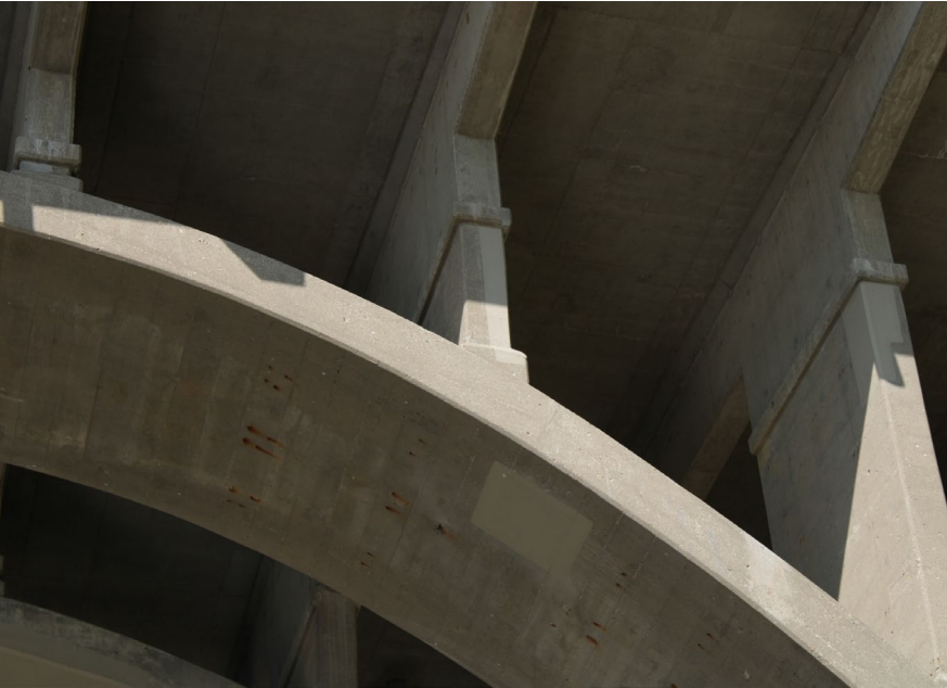
54. Looking West at Patching on S.N. 050-0096 East Span #4
