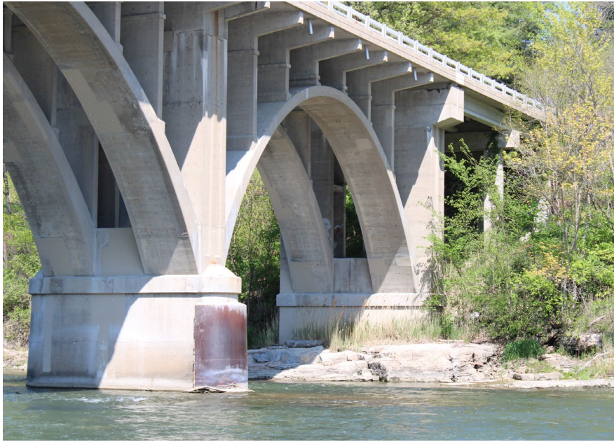
125. Looking North-West at S.N. 050-0096 East Profile of Span #4
