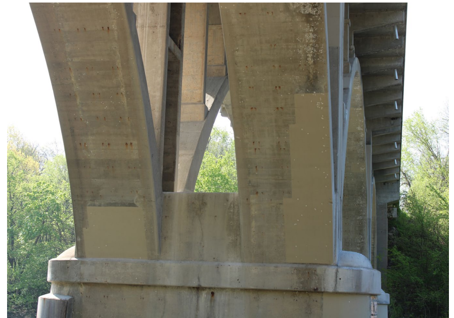
43. Looking South at Patching underneath S.N. 050-0096 Span #4
