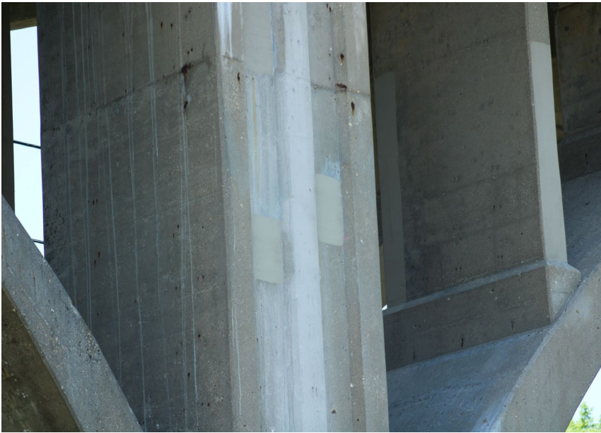
163. Looking North-West at Patching on S.N. 050-0096 East Profile of Pier #5
