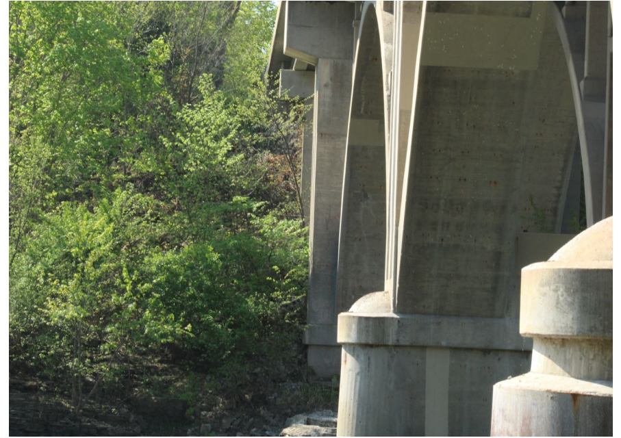
73. Looking South at Patching on S.N. 050-0096 underneath East Span #5
