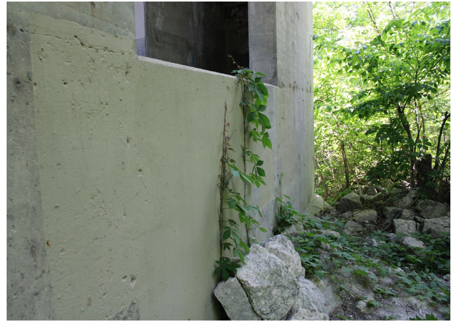
138. Looking North-East at Patching on S.N. 050-0096 South Profile of Pier #6
