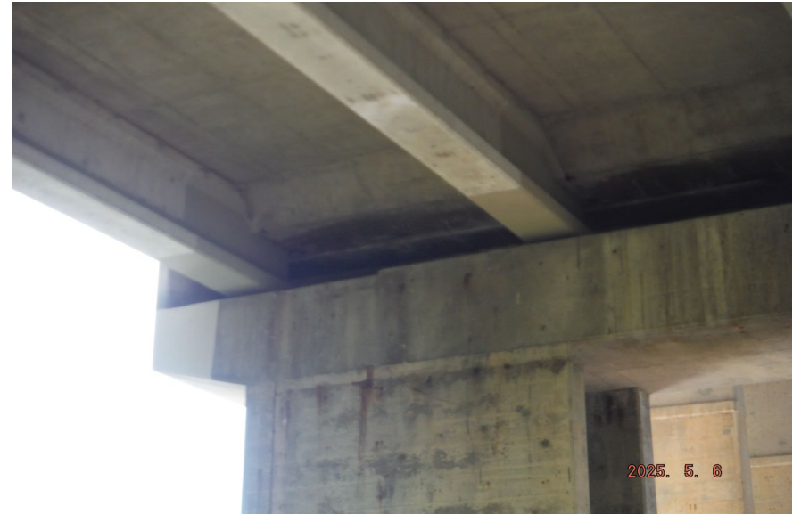
14. Looking South-East at Patching on the North Profile of S.N. 50-0096 East Pier #3
