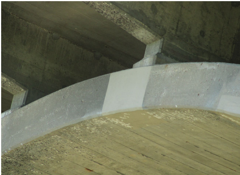
171. Looking North-East at Patching on S.N. 050-0096 West Profile of West Span #5
