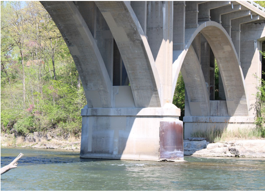
79. Looking North at Patching on S.N. 050-0096 underneath Span #5
