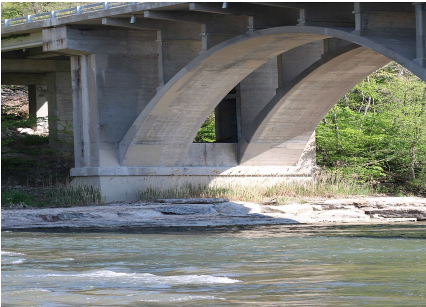
131. Looking North-East at S.N. 050-0096 West Profile of Pier #3
