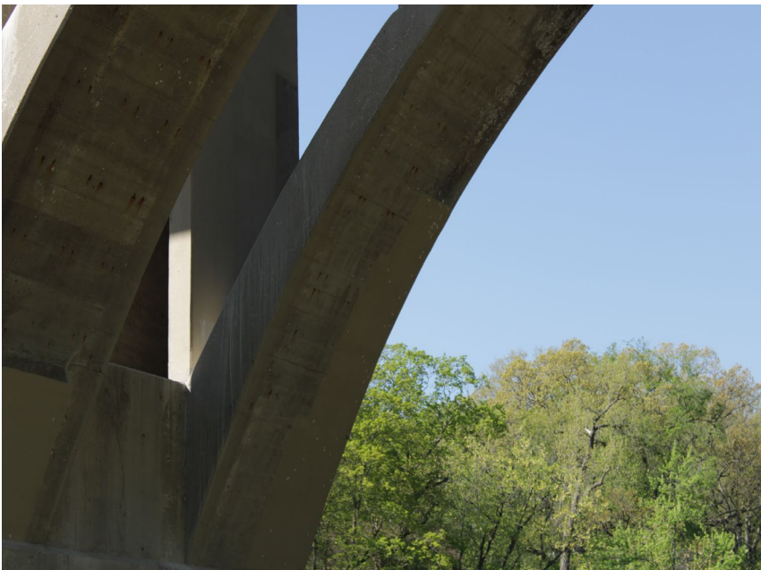
46. Looking South-West at Patching underneath S.N. 050-0096 West Span #4
