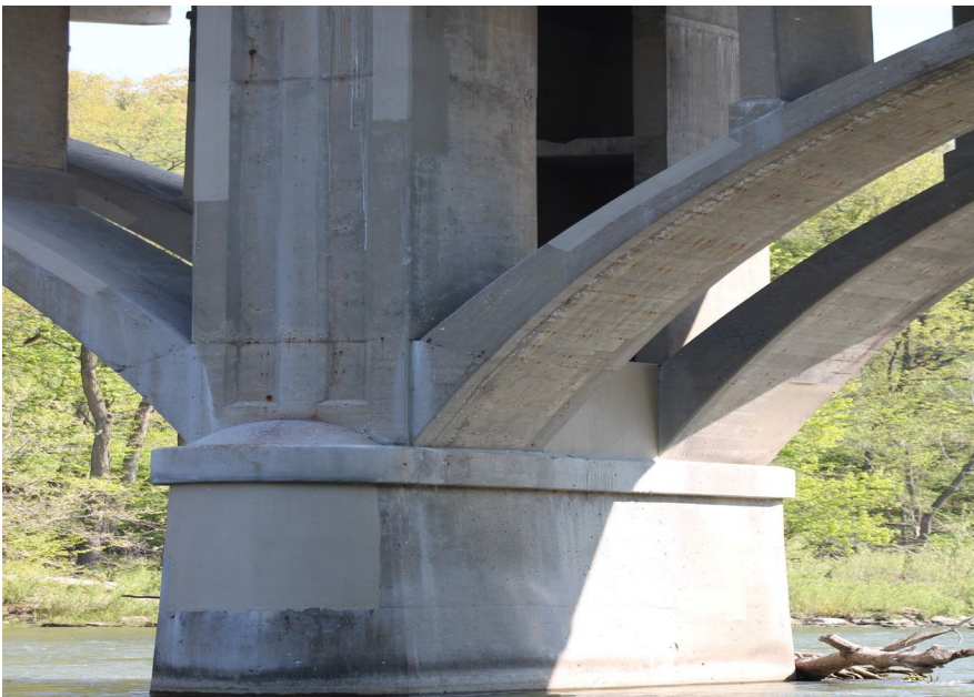
135. Looking East at S.N. 050-0096 West Profile of Pier #5
