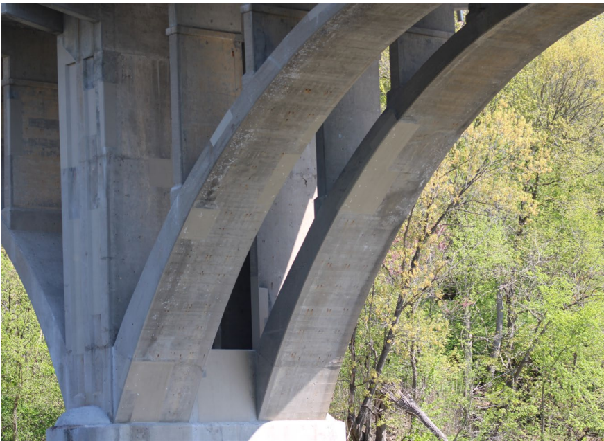
97. Looking North-East at Patching on S.N. 050-0096 underneath Span #6
