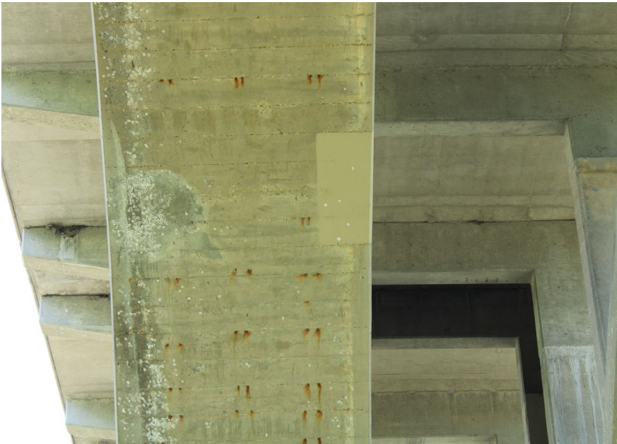
179. Looking North at Patching underneath S.N. 050-0096 Span #6
