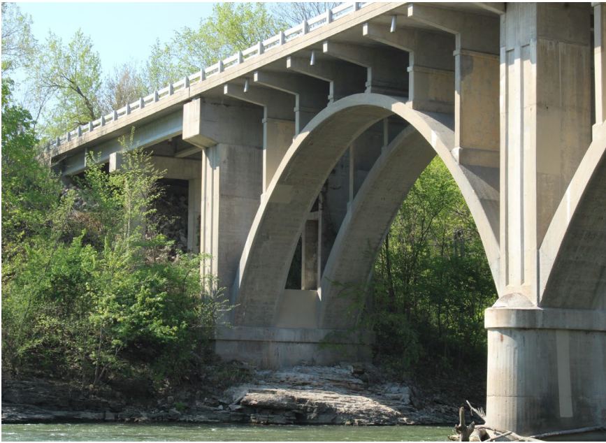
117. Looking South-West at S.N. 050-0096 East Profile of Span #6
