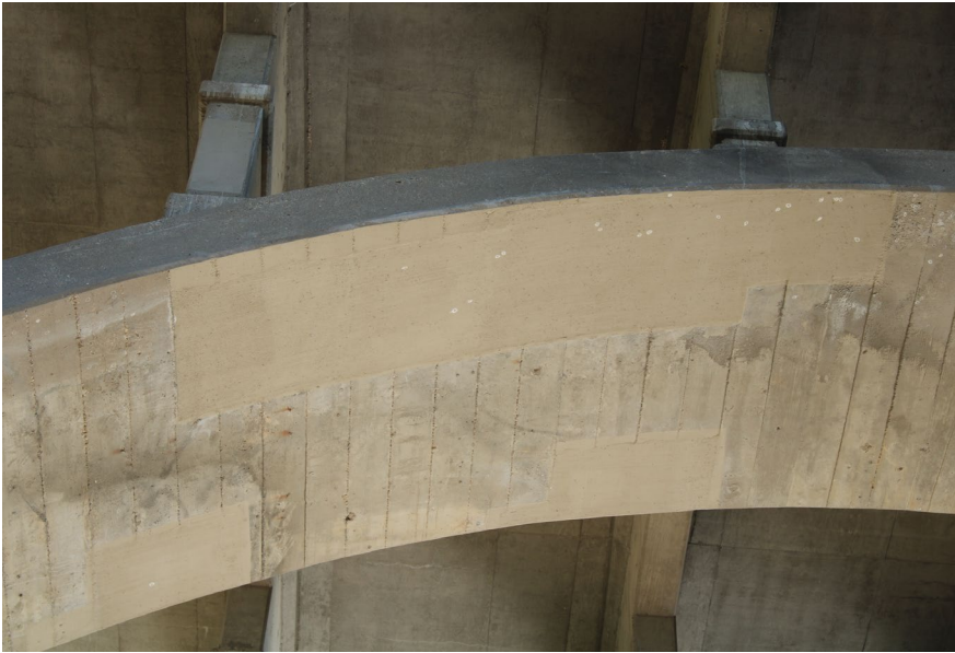
32. Looking East at Patching underneath S.N. 050-0096 West Span #4
