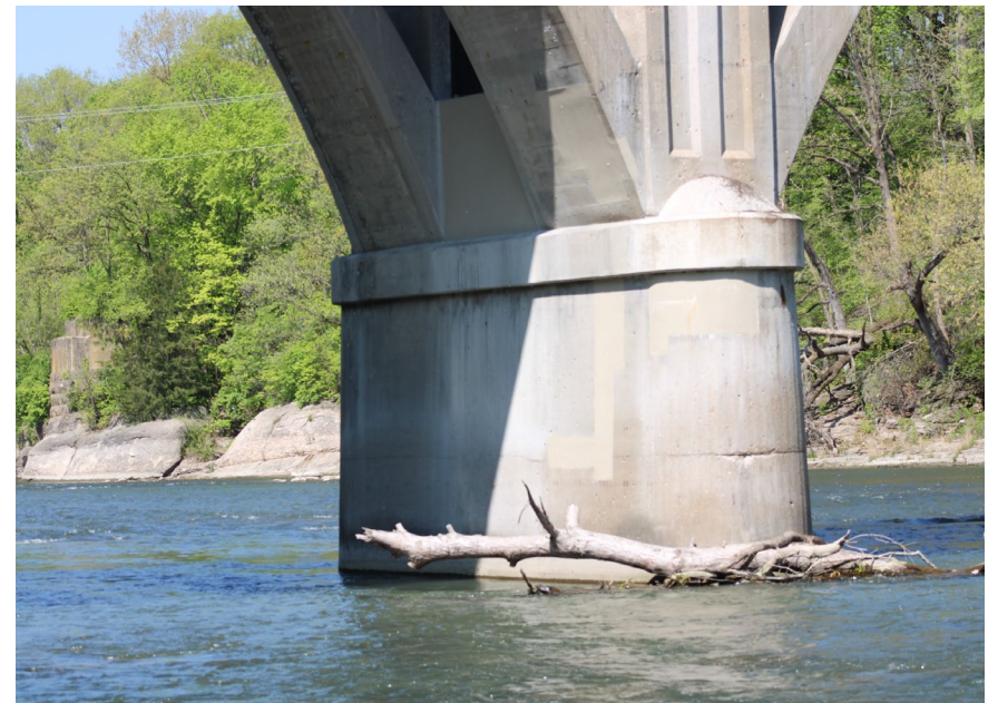
82. Looking West at Patching on S.N. 050-0096 Pier #5
