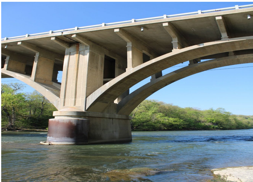
50. Looking West at Patching on the South Profile of S.N. 050-0096 Pier #4
