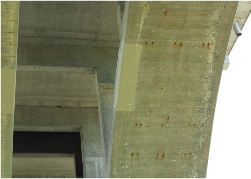
185. Looking North at Patching underneath S.N. 050-0096 East Span #6
