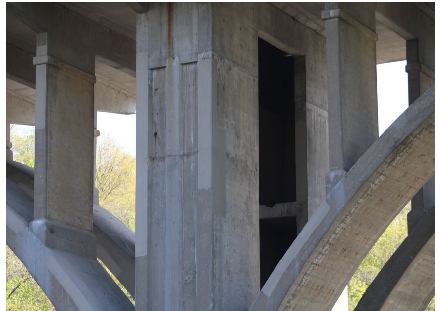
134. Looking East at S.N. 050-0096 West Profile of Pier #5
