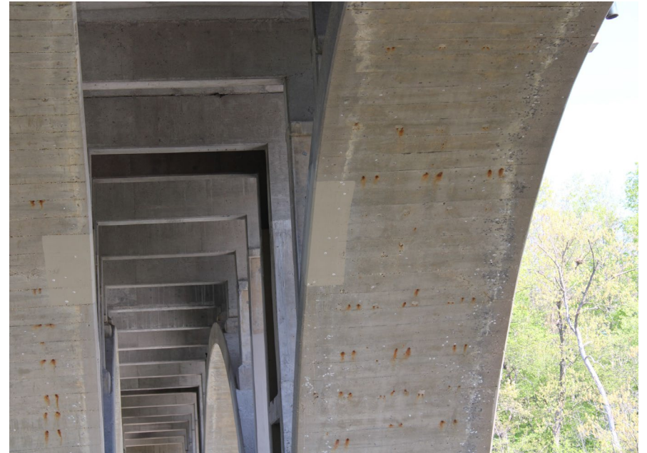
100. Looking North at Patching on S.N. 050-0096 underneath East Span #6
