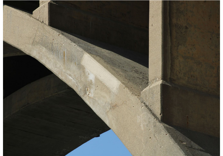
57. Looking West at Patching on S.N. 050-0096 East Span #5
