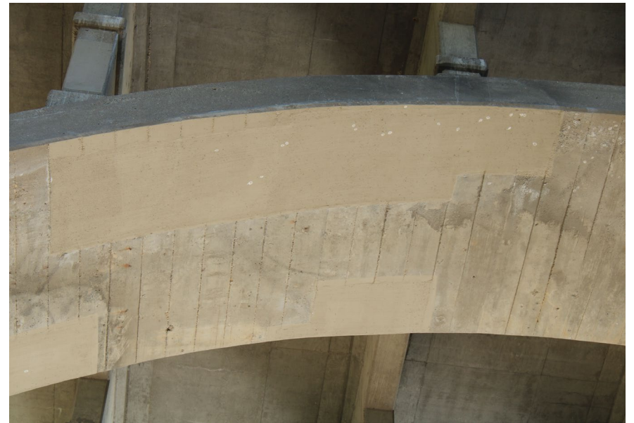
33. Looking East at Patching underneath S.N. 050-0096 West Span #4
