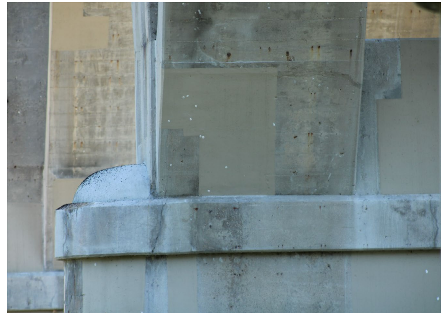
144. Looking North at Patching underneath S.N. 050-0096 Span #5
