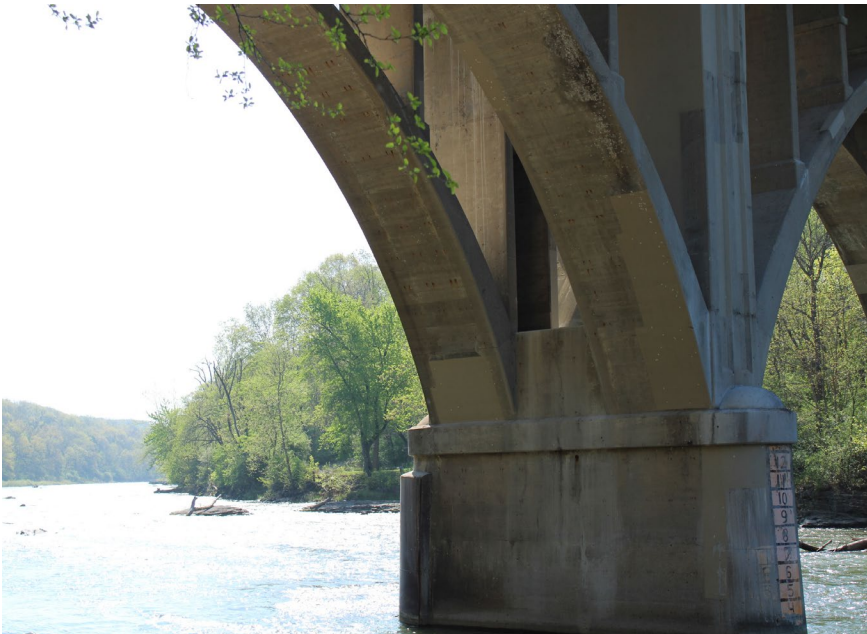
42. Looking South-East at Patching underneath S.N. 050-0096 Span #4
