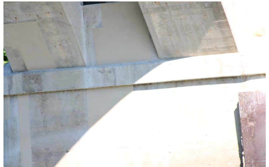
96. Looking North-West at Patching on the South Profile of S.N. 050-0096 Pier #4
