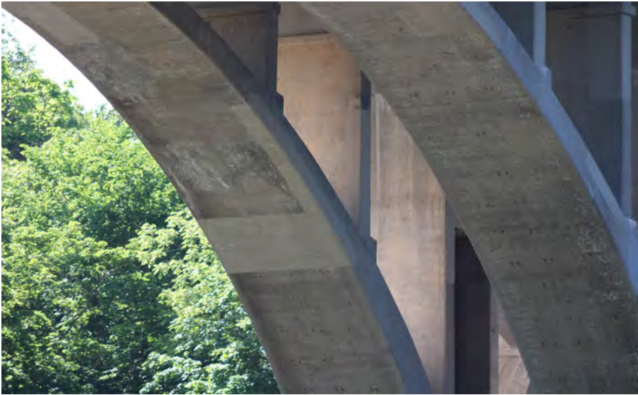
117. Looking South-East at Patching underneath S.N. 050-0096 Span #5
