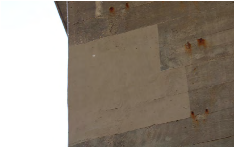
187. Looking Directly Up at Patching underneath S.N. 050-0096 East Span #6
