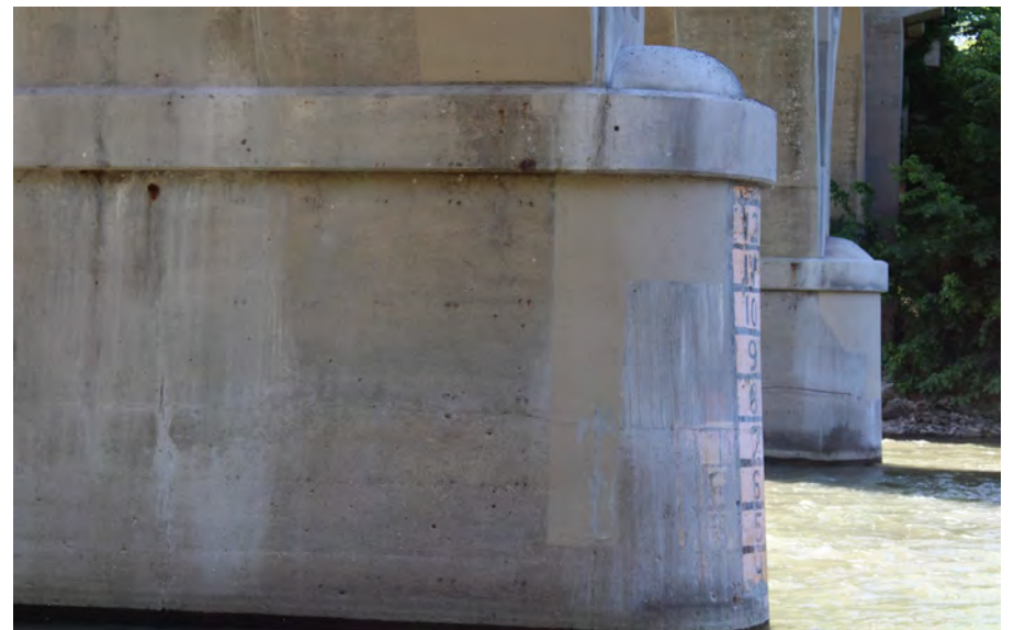
72. Looking South at Patching on the North Profile of S.N. 050-0096 Pier #4
