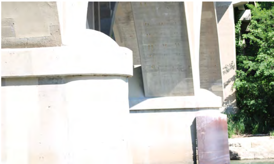
135. Looking North at Patching on the West Profile of S.N. 050-0096 Pier #5
