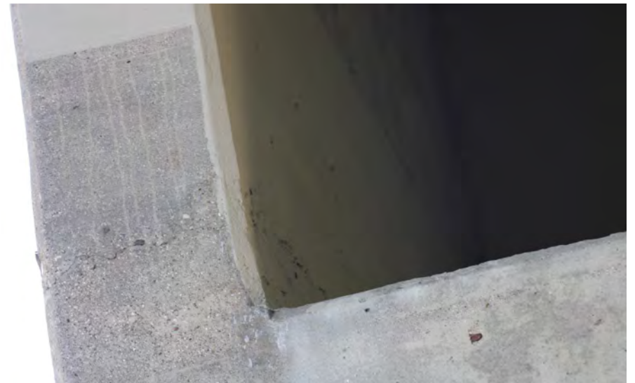
208. Looking East at Patching on the inside of S.N. 050-0096 Pier #6
