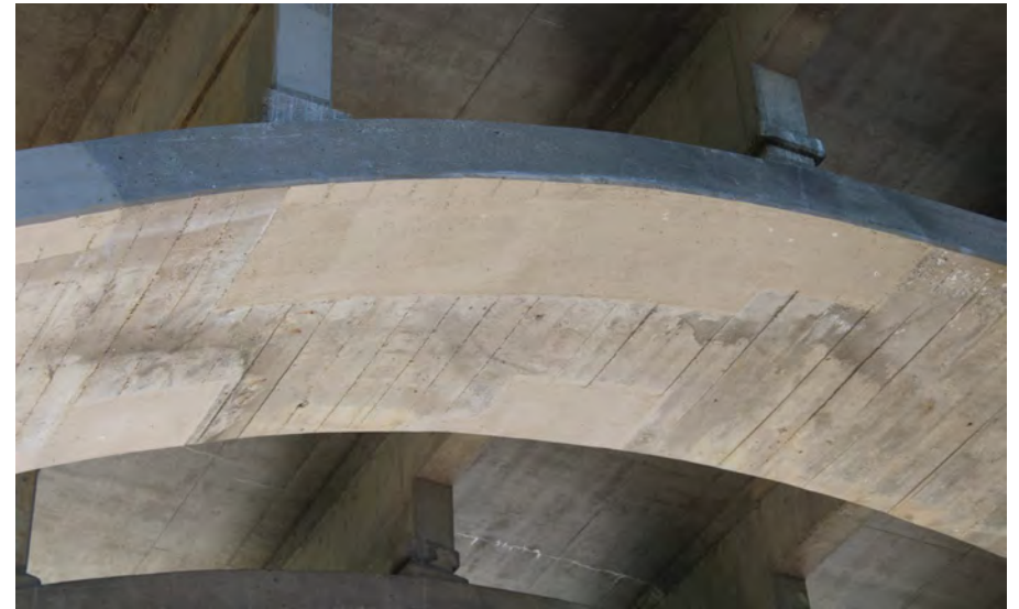
62. Looking East at Patching underneath S.N. 050-0096 West Span #4
