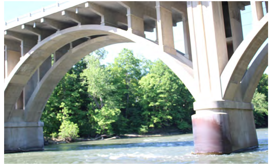
86. Looking West at Patching on the East Profile of S.N. 050-0096 Pier #4
