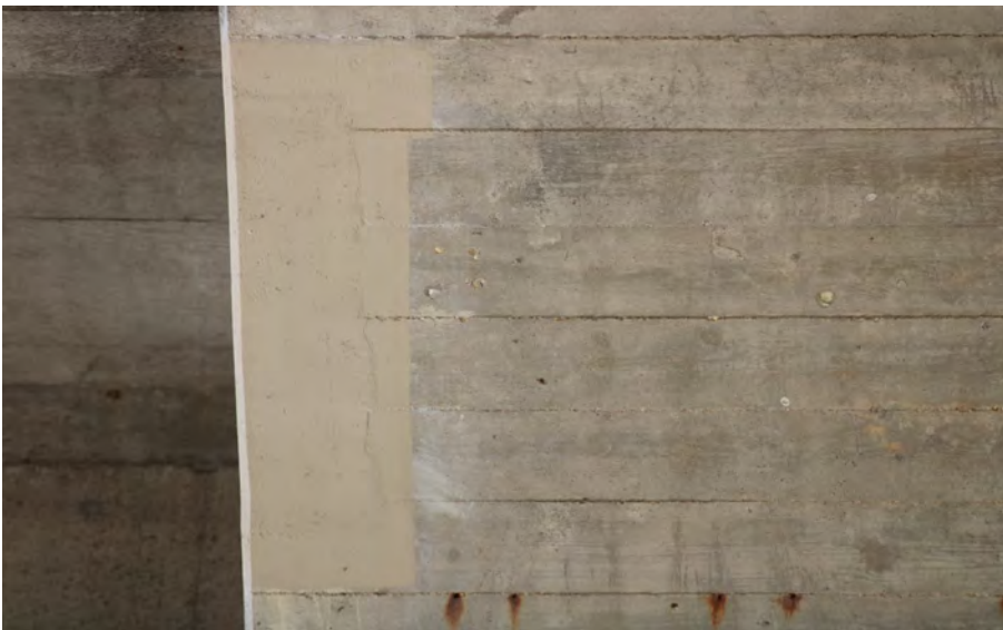
59. Looking South at Patching underneath S.N. 050-0096 West Span #4
