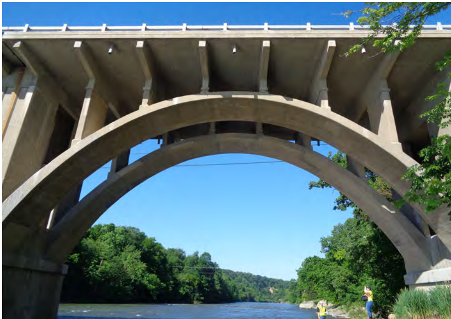
67. Looking West at Patching on S.N. 050-0096 Span #4
