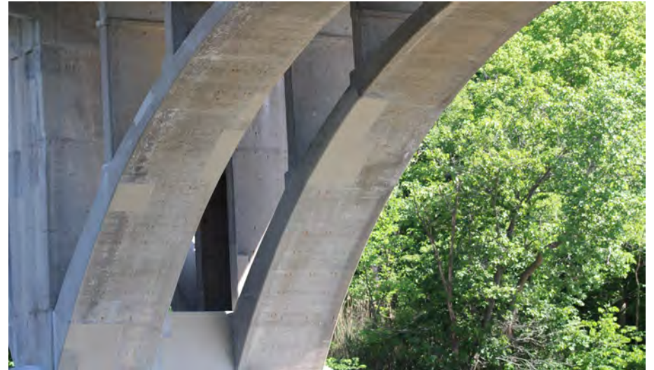
90. Looking North-East at Patching on the South Profile of S.N. 050-0096 Pier #4
