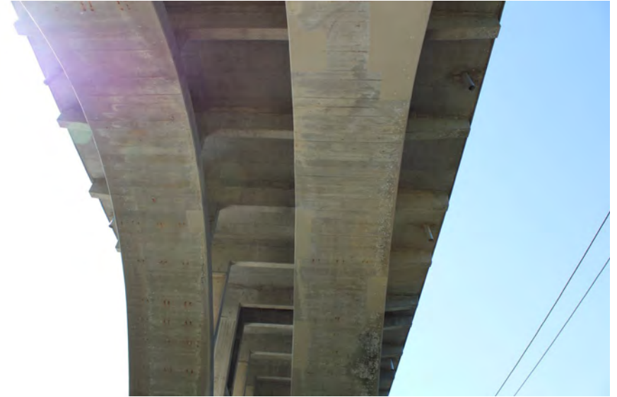
54. Looking South at Patching underneath S.N. 050-0096 Span #4
