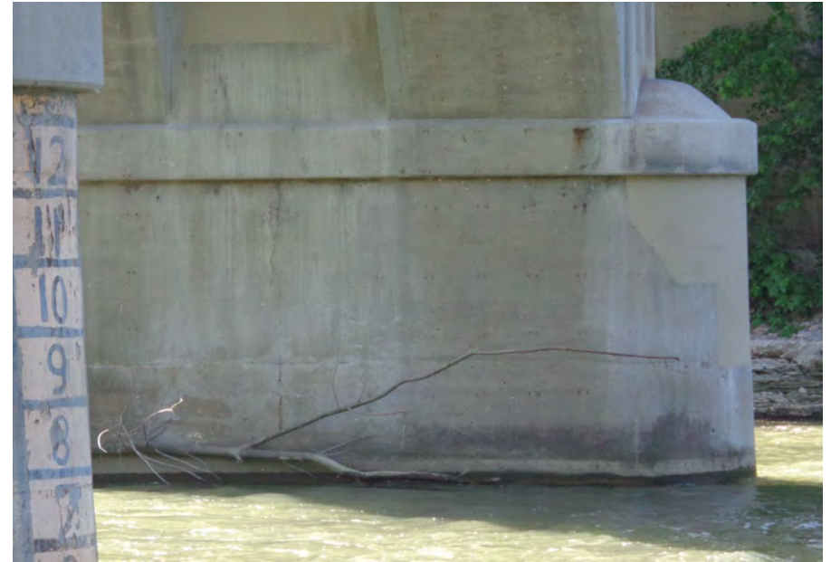
130. Looking South at Patching on the North Profile of S.N. 050-0096 Pier #5
