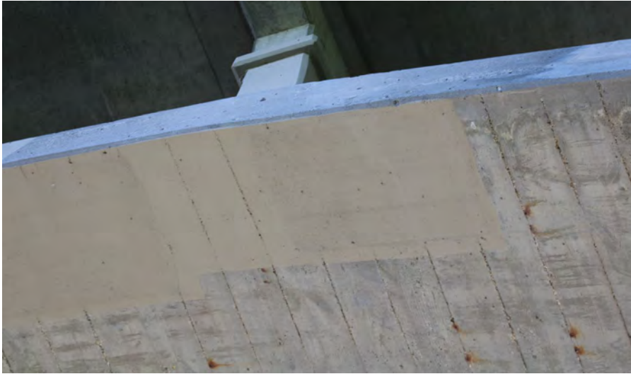
197. Looking Directly Up at Patching underneath S.N. 050-0096 West Span #6
