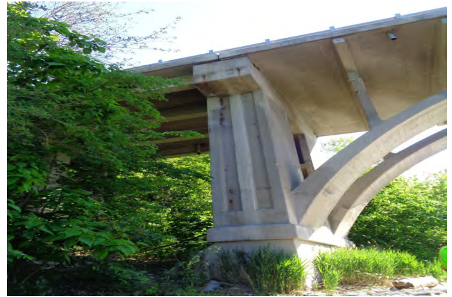
22. Looking East at Patching on the West Profile of S.N. 050-0096 West Pier #3
