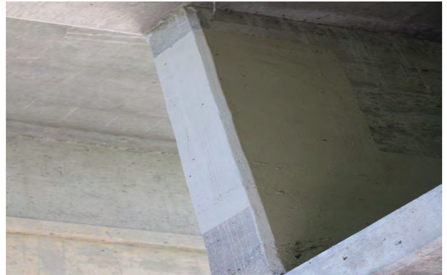
202. Looking North-East at Patching on the inside of S.N. 050-0096 Pier #6
