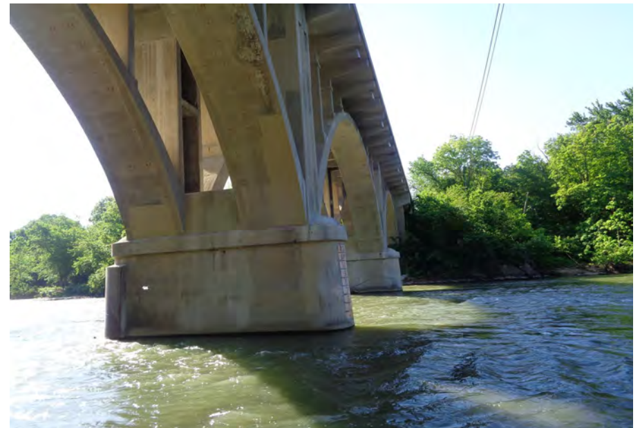
44. Looking South at Patching underneath S.N. 050-0096 Span #4
