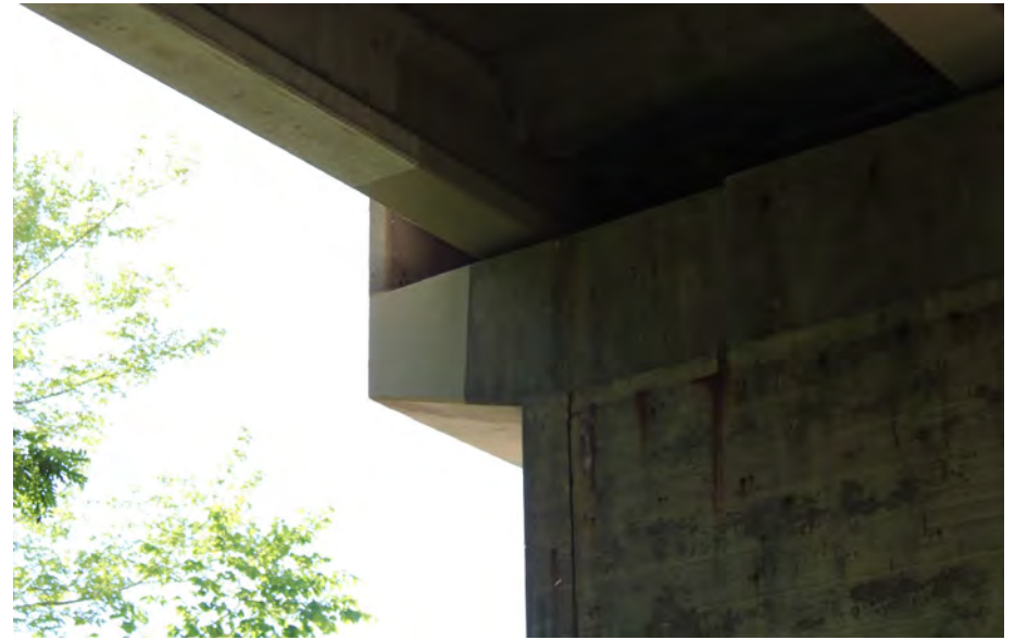
18. Looking South-East at Patching on the North Profile of S.N. 50-0096 East Pier #3
