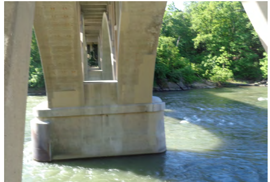
38. Looking South at Patching underneath S.N. 050-0096 West Span #4
