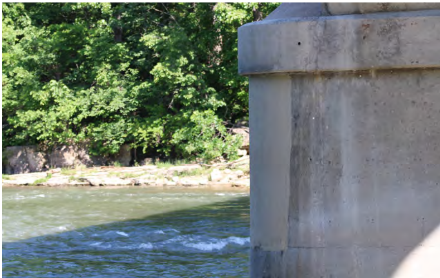
131. Looking North at Patching on the South Profile of S.N. 050-0096 Pier #5
