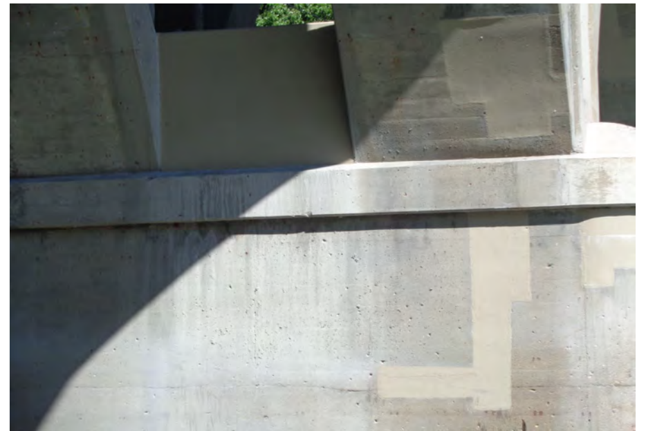
136. Looking North-West at Patching on the South Profile of S.N. 050-0096 Pier #5
