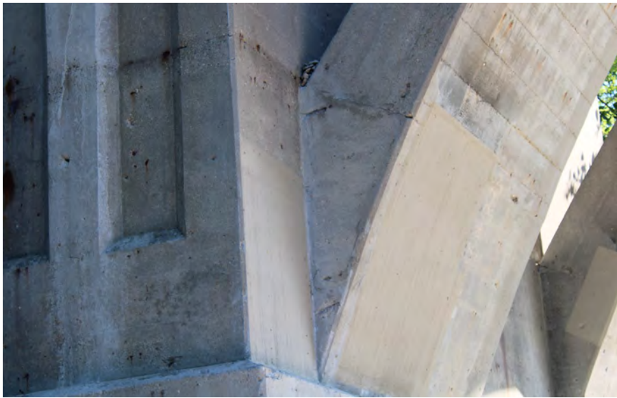
29. Looking East at Patching on the South Profile of S.N. 050-0096 West Pier #3
