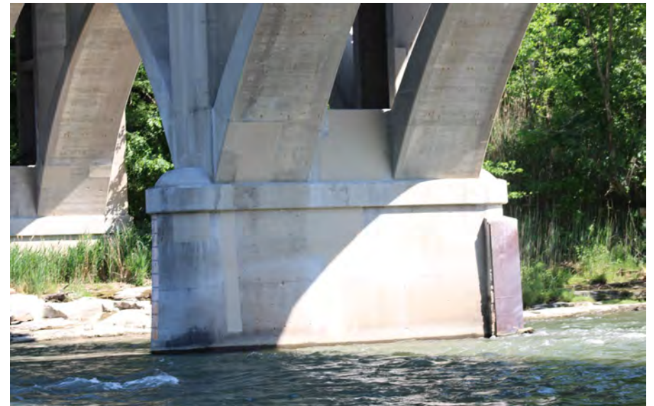
94. Looking North-East at Patching on the South Profile of S.N. 050-0096 Pier #4
