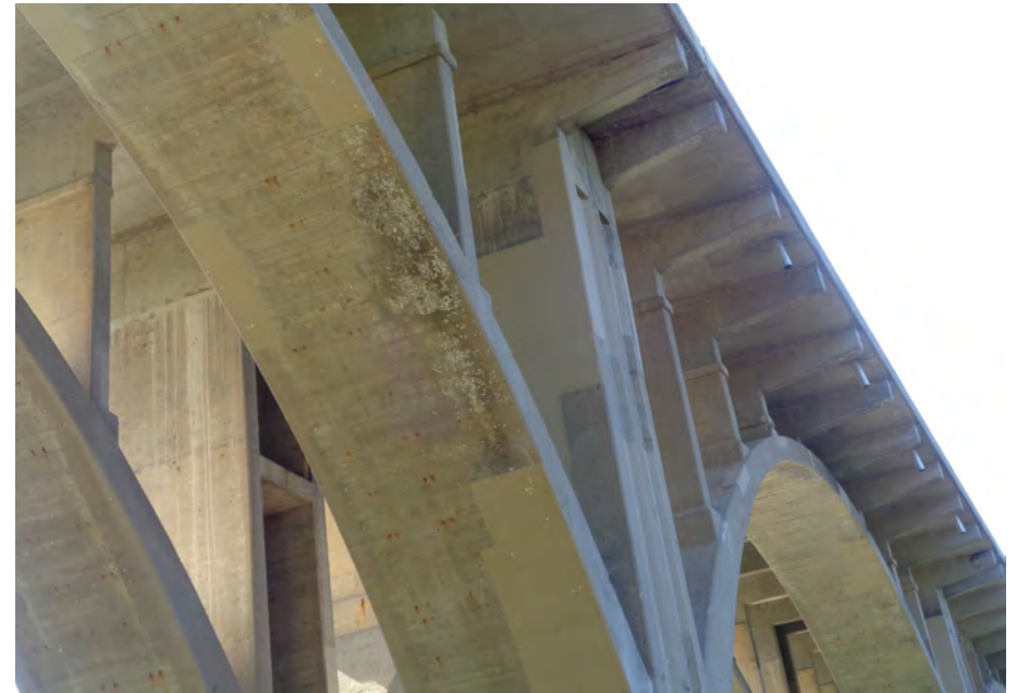
42. Looking South-East at Patching underneath S.N. 050-0096 West Span #4
