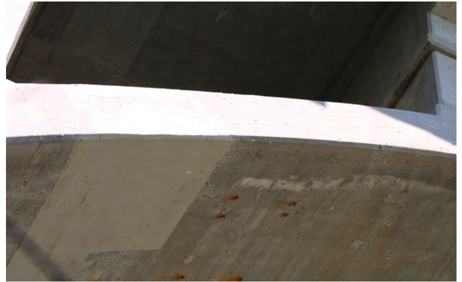
186. Looking Directly up at Patching underneath S.N. 050-0096 East Span #6
