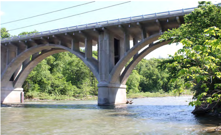
11. Looking East at Patching on the West Profile of S.N. 050-0096
