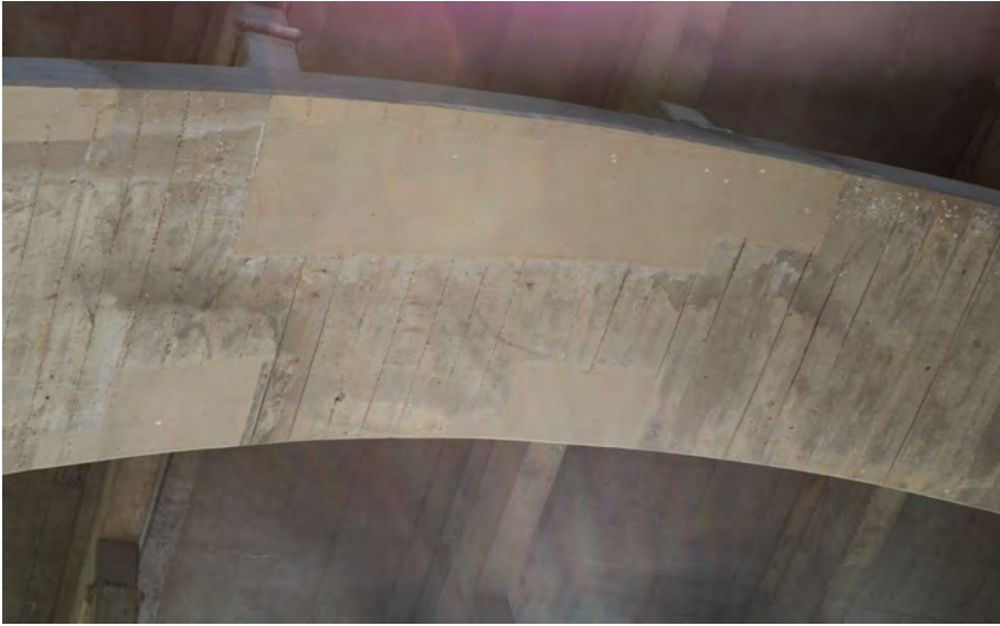
61. Looking Directly Up at Patching underneath S.N. 050-0096 West Span #4
