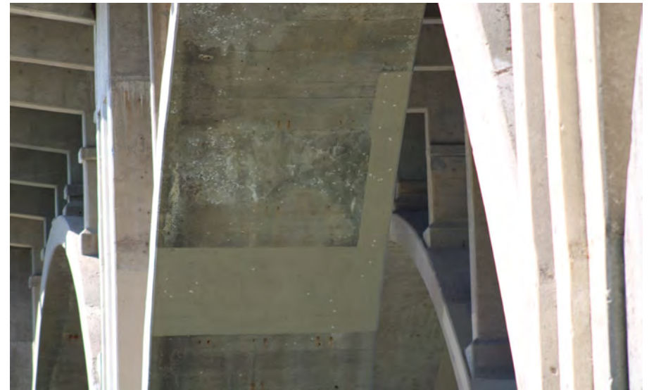
106. Looking South at Patching underneath S.N. 050-0096 East Span #5
