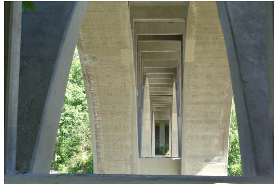
172. Looking North at Patching underneath S.N. 050-0096 Span #6
