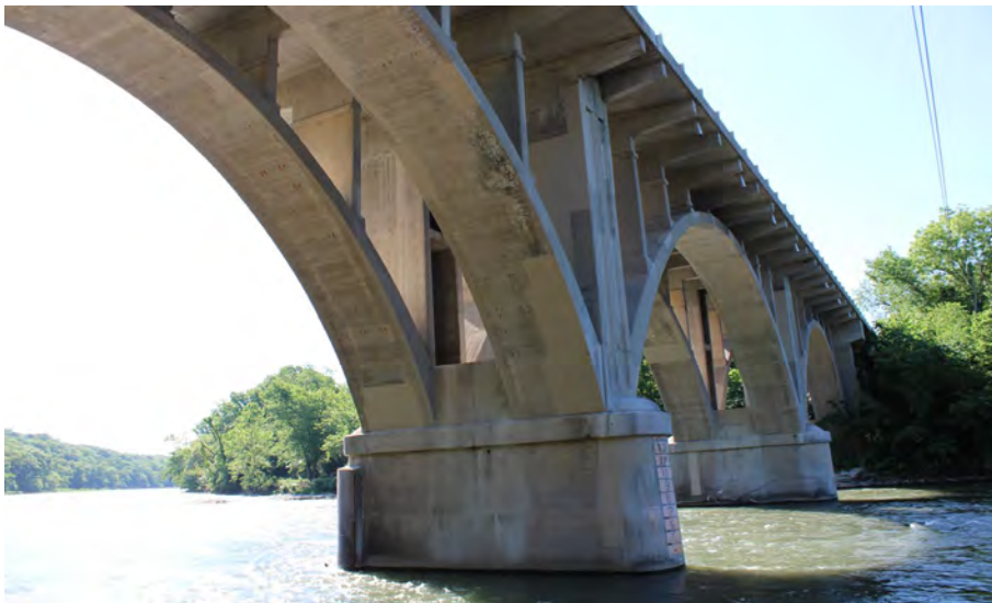
3. Looking South at Patching on the West Profile of S.N. 050-0096
