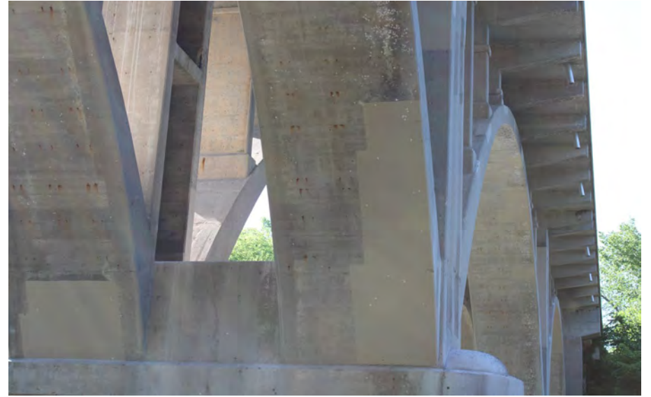
50. Looking South at Patching underneath S.N. 050-0096 West Span #4
