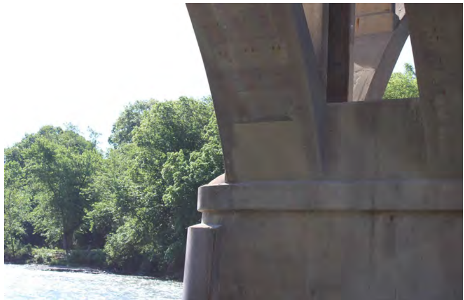
47. Looking South-East at Patching underneath S.N. 050-0096 East Span #4
