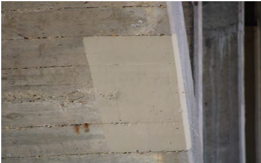
189. Looking North at Patching underneath S.N. 050-0096 West Span #6
