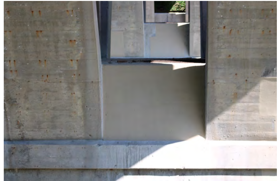
160. Looking North at Patching on the South Profile of S.N. 050-0096 Pier #5
