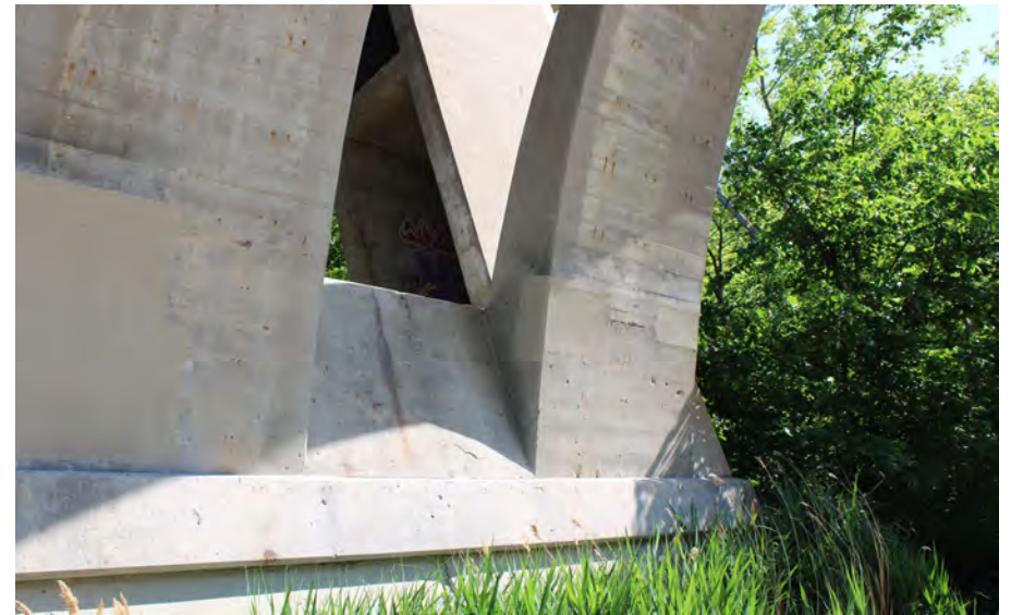
28. Looking North-East at Patching underneath S.N. 050-0096 Span #4
