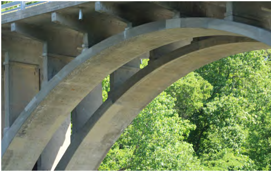
121. Looking North-East at Patching underneath S.N. 050-0096 Span #5
