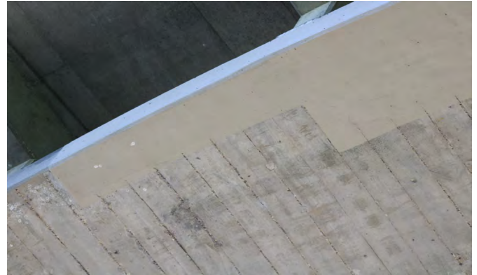
198. Looking Directly Up at Patching underneath S.N. 050-0096 West Span #6
