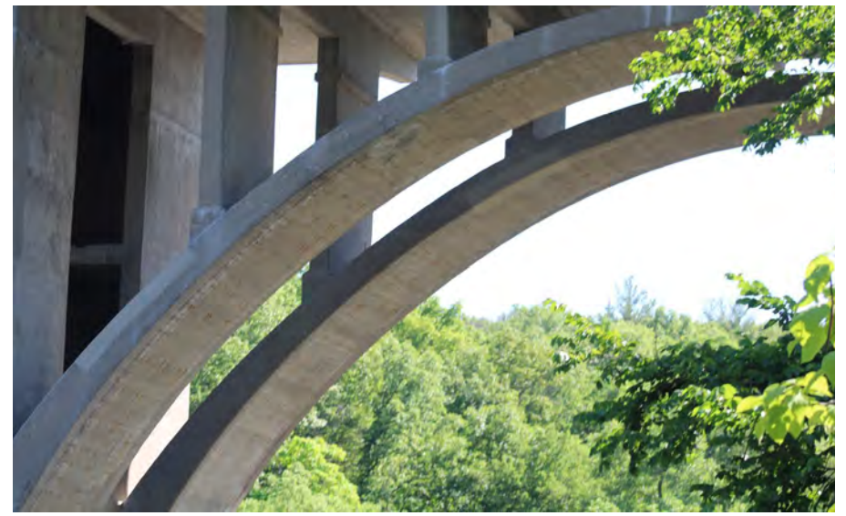
166. Looking East at Patching underneath S.N. 050-0096 Span #6
