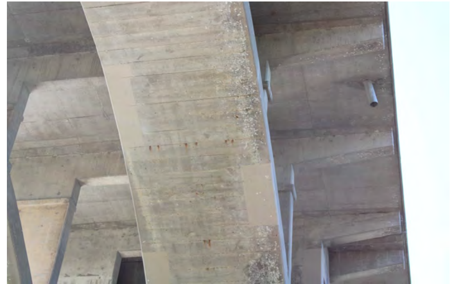
46. Looking South at Patching underneath S.N. 050-0096 West Span #4
