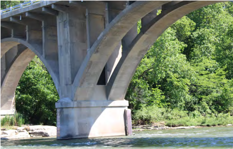
93. Looking North-East at Patching on the South Profile of S.N. 050-0096 Pier #4
