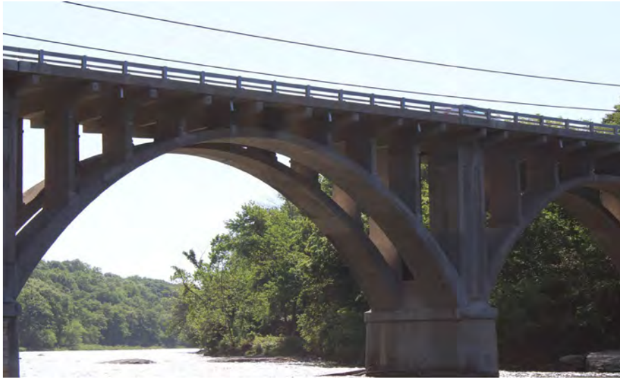
1. Looking East at Patching on the West Profile of S.N. 050-0096
