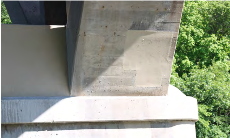
201. Looking North at patching underneath S.N. 050-0096 East Span #6
