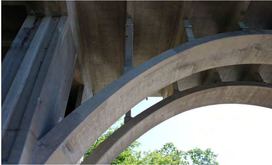
65. Looking East at Patching on S.N. 050-0096 Span #4
