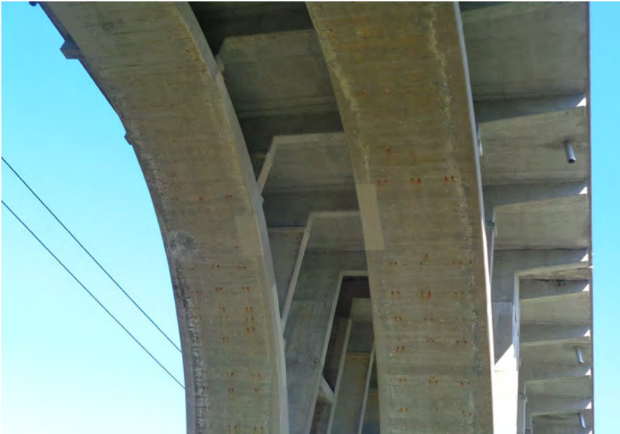
169. Looking North at Patching underneath S.N. 050-0096 Span #6
