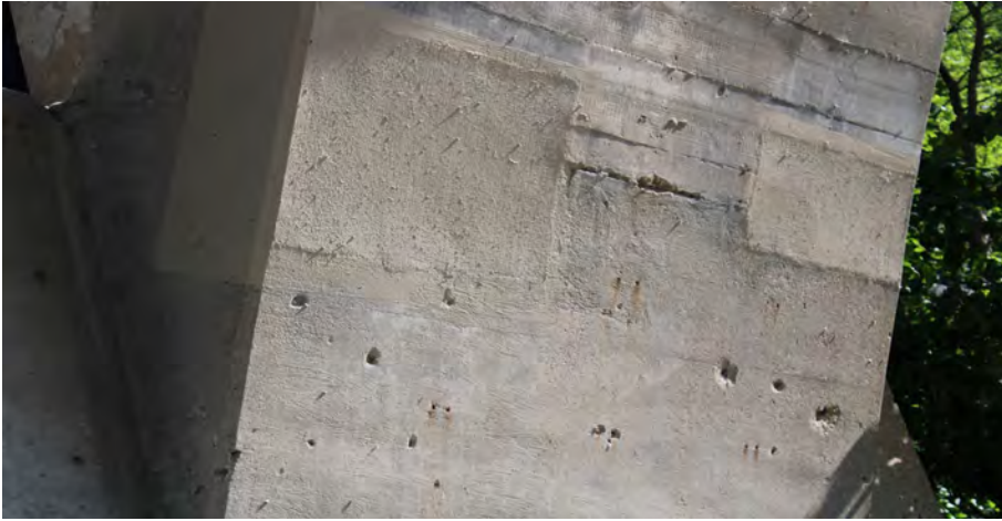
33. Looking North at Patching underneath S.N. 050-0096 East Span #4
