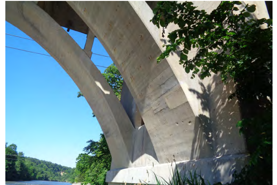
36. Looking West at Patching underneath S.N. 050-0096 East Span #4
