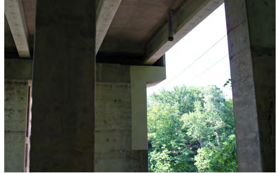
14. Looking South-West at Patching on the North Profile of S.N. 050-0096 West Pier #3
