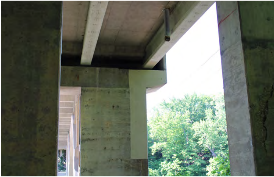
13. Looking South-West at Patching on the North Profile of S.N. 050-0096 West Pier #3
