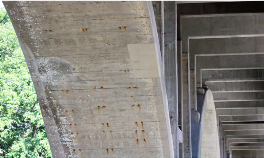
193. Looking North-West at Patching underneath S.N. 050-0096 West Span #6
