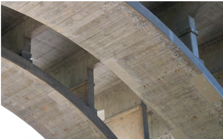
55. Looking South-East at Patching underneath S.N. 050-0096 West Span #4
