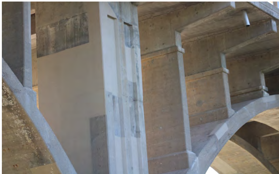
155. Looking South-East at Patching on the West Profile of S.N. 050-0096 Pier #5
