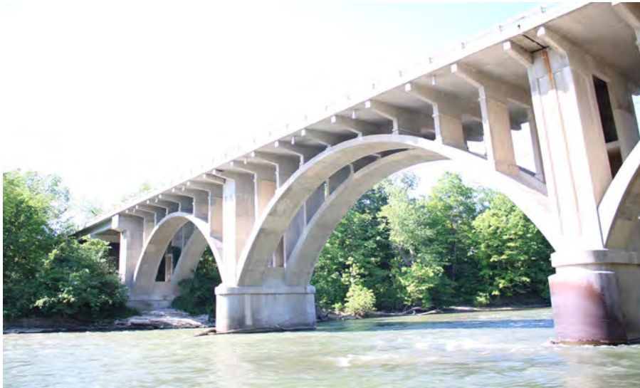
5. Looking South-West at Patching on the East Profile of S.N. 050-0096
