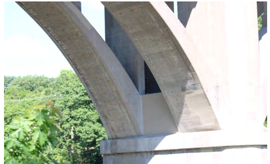
164. Looking North-West at Patching on the South Profile of S.N. 050-0096 Pier #5
