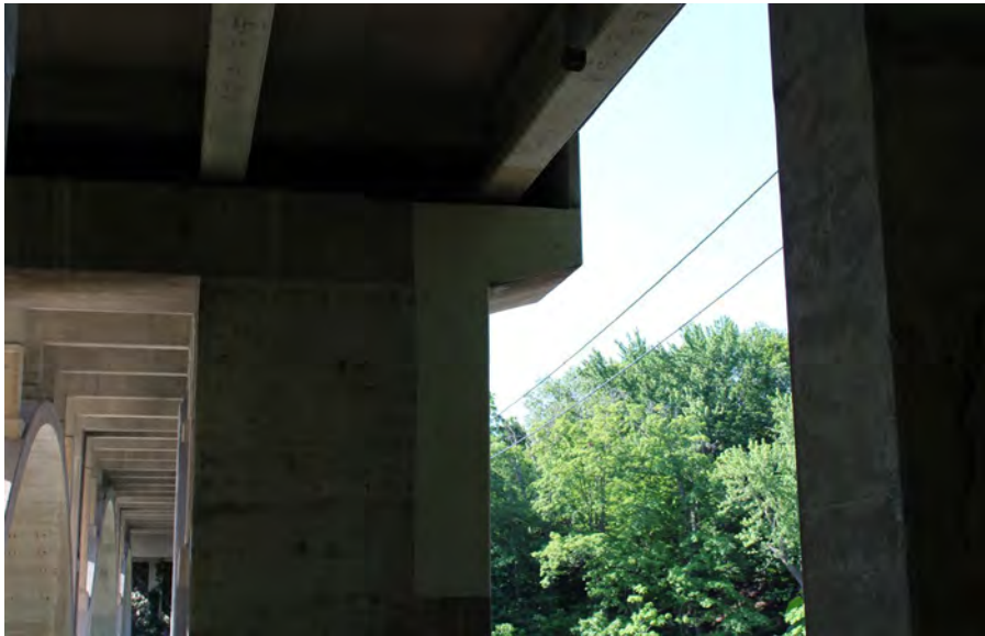
15. Looking South-West at Patching on the North Profile of S.N. 050-0096 West Pier #3
