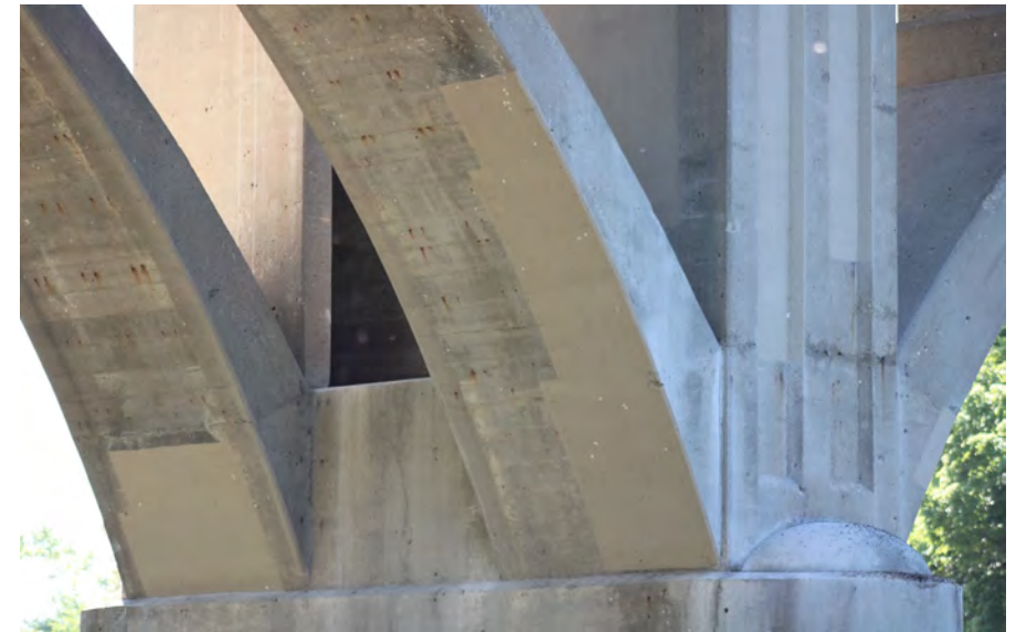
48. Looking South-East at Patching underneath S.N. 050-0096 Span #4
