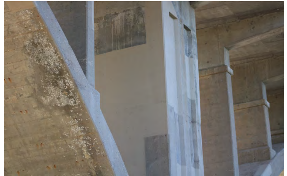
154. Looking South-East at Patching on the West Profile of S.N. 050-0096 Pier #5
