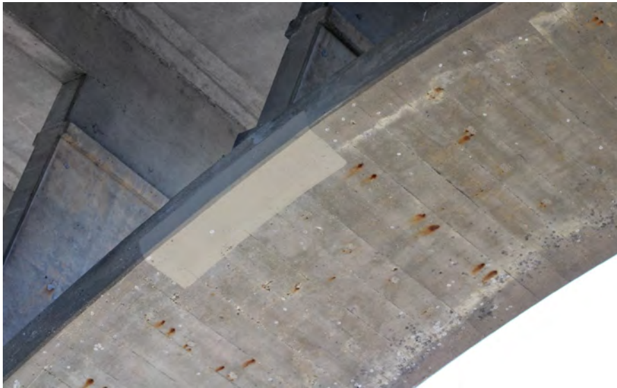
181. Looking Directly Up at Patching underneath S.N. 050-0096 East Span #6
