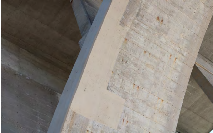
49. Looking North at Patching underneath S.N. 050-0096 West Span #4
