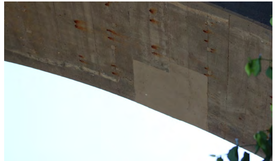
200. Looking East at Patching underneath S.N. 050-0096 East Span #6
