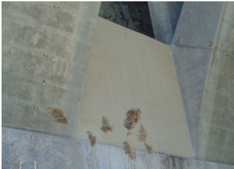
203. Looking South at Patching on the North Profile of S.N. 050-0096 Pier #6
