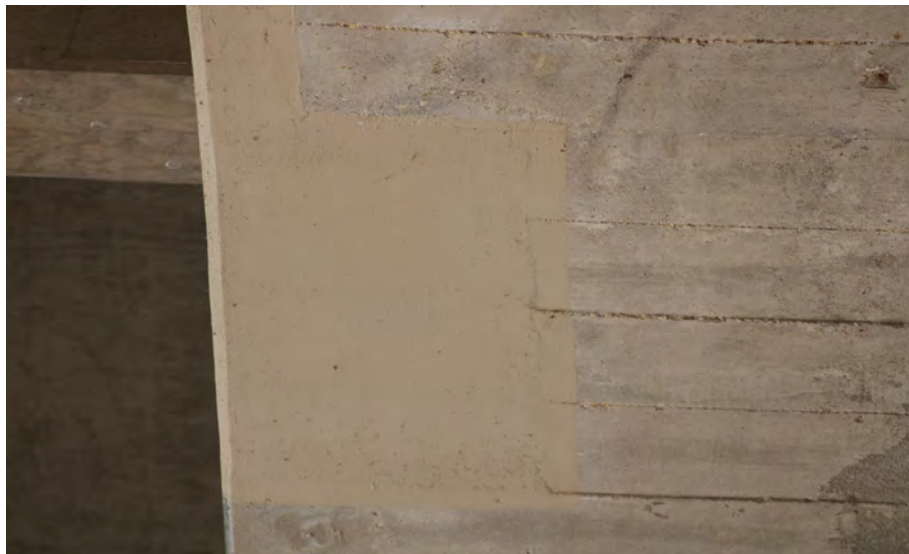
63. Looking South at Patching underneath S.N. 050-0096 West Span #4
