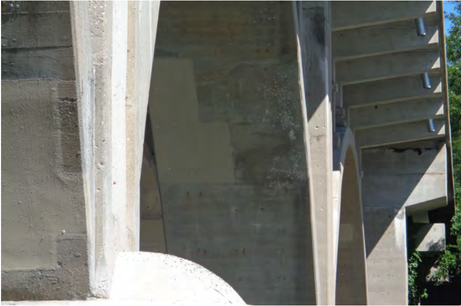
161. Looking North at Patching underneath S.N. 050-0096 East Span #5
