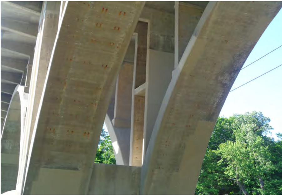
41. Looking South-West at Patching underneath S.N. 050-0096 West Span #4
