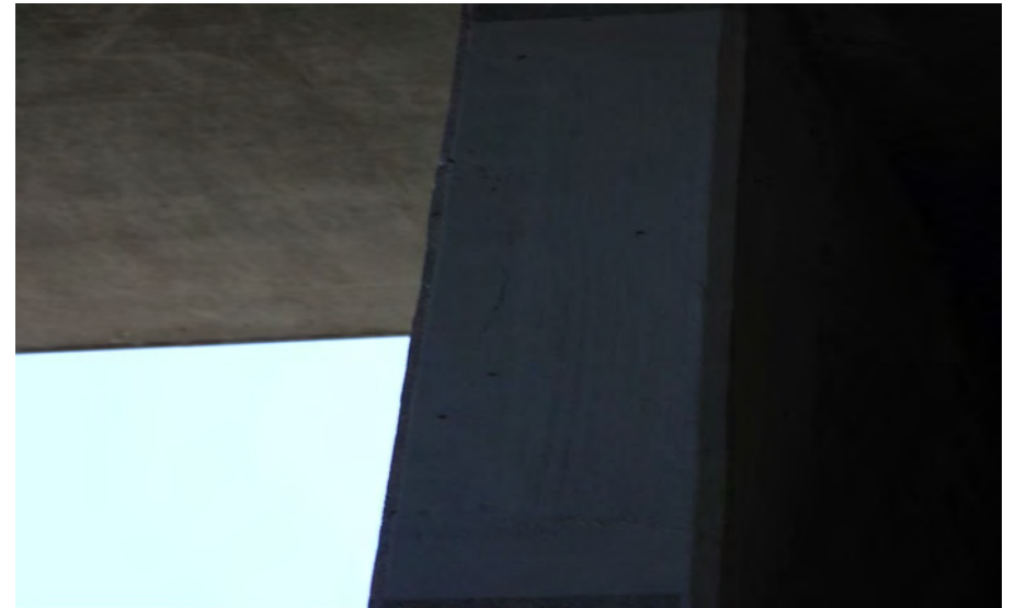
206. Looking East at Patching on the inside of S.N. 050-0096 Pier #6
