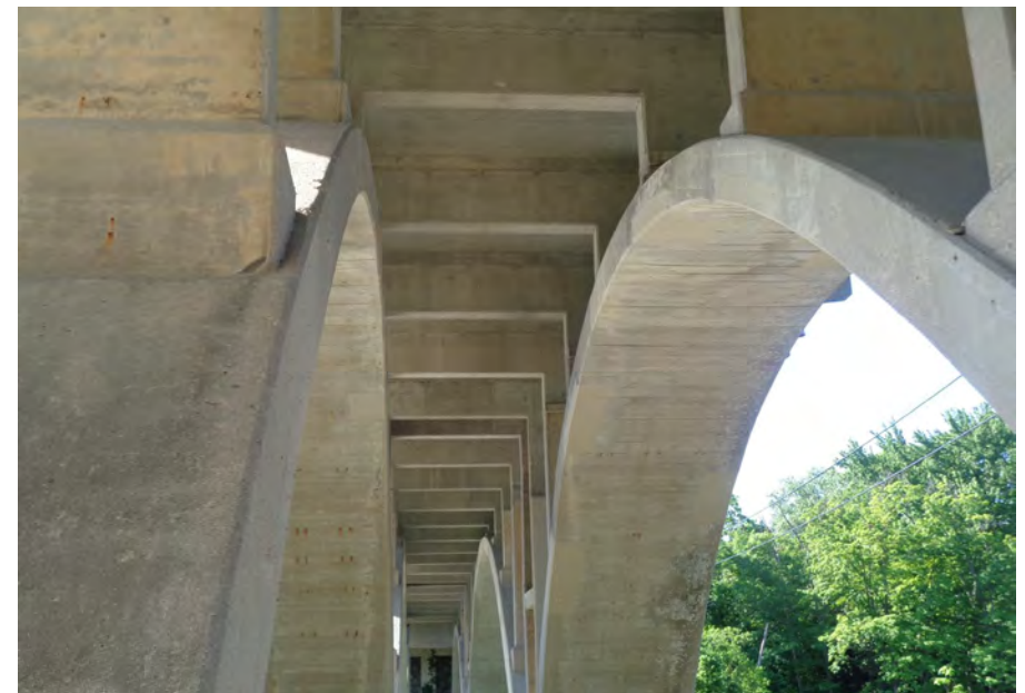
40. Looking South at Patching underneath S.N. 050-0096 West Span #4
