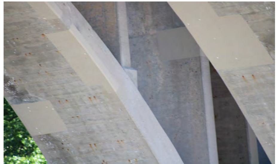
124. Looking North-West at Patching underneath S.N. 050-0096 Span #5
