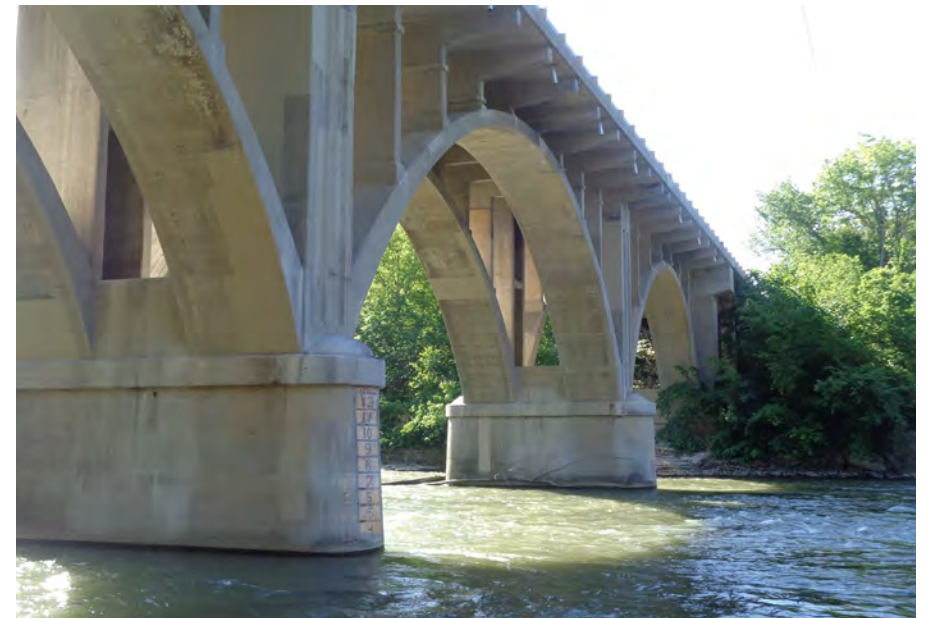
12. Looking South at Patching on the West Profile of S.N. 050-0096
