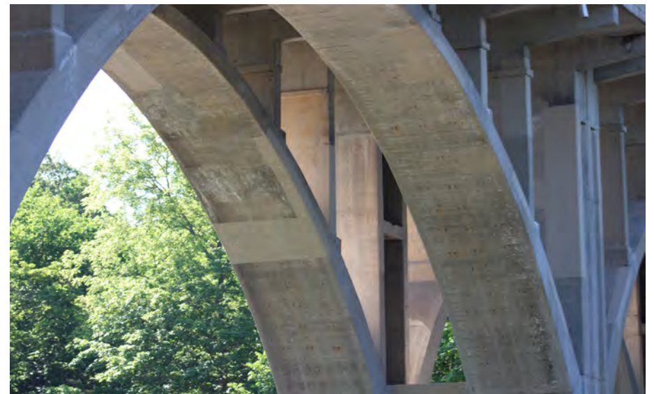
104. Looking South-East at Patching underneath S.N. 050-0096 Span #5
