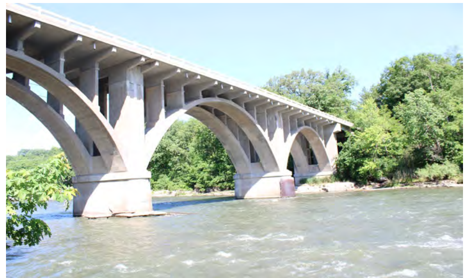
8. Looking North-West at Patching on the East Profile of S.N. 050-0096
