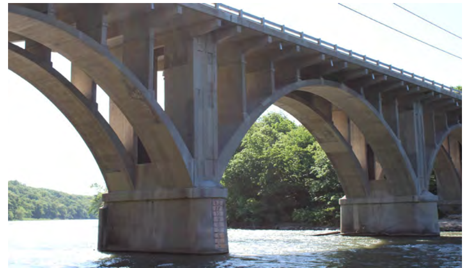
80. Looking South-East at Patching on the West Profile of S.N. 050-0096 Pier #4
