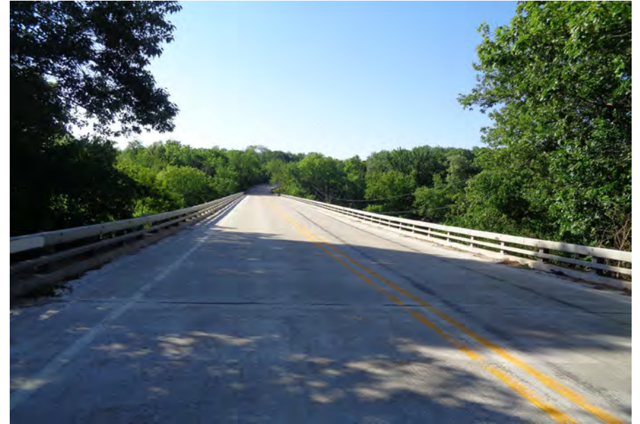
10. Looking South along IL 178 through S.N. 050-0096 at Sta. 196+85
