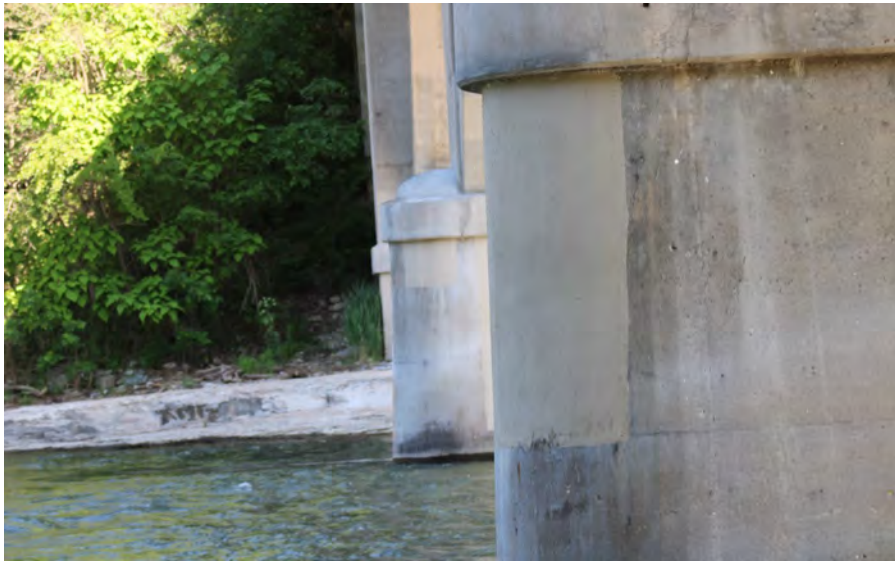
149. Looking North at Patching on the South Profile of S.N. 050-0096 Pier #5
