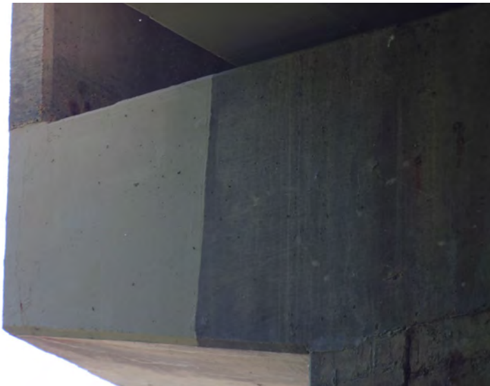
19. Looking South-East at Patching on the North Profile of S.N. 50-0096 East Pier #3
