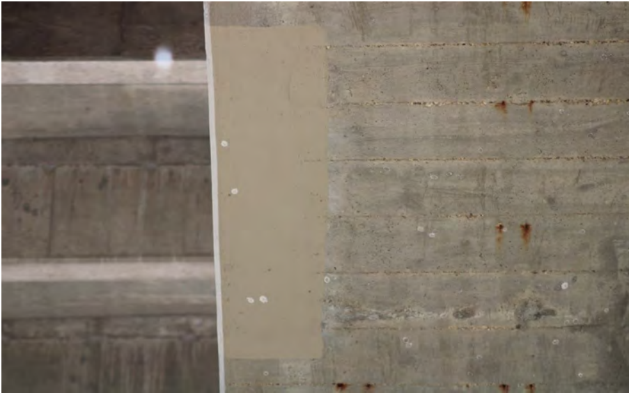
69. Looking South at Patching underneath S.N. 050-0096 West Span #4
