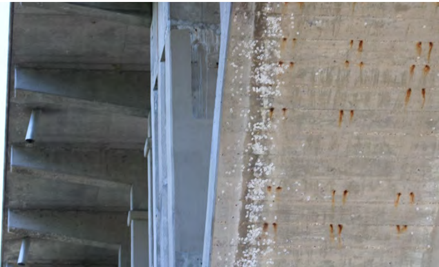
159. Looking North at Patching on the West Profile of S.N. 050-0096 Pier #5
