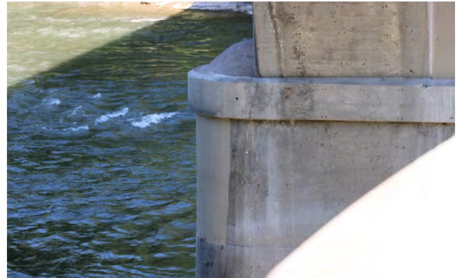
150. Looking North at Patching on the South Profile of S.N. 050-0096 Pier #5
