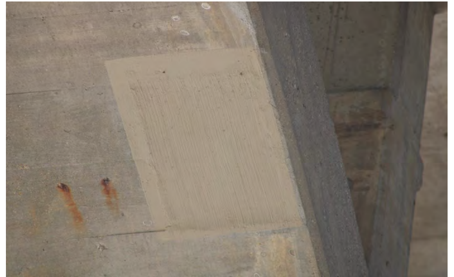
70. Looking South-East at Patching underneath S.N. 050-0096 East Span #4
