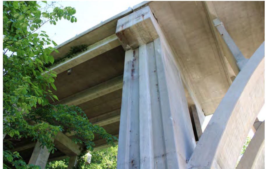
24. Looking East at Patching on the West Profile of S.N. 050-0096 West Pier #3
