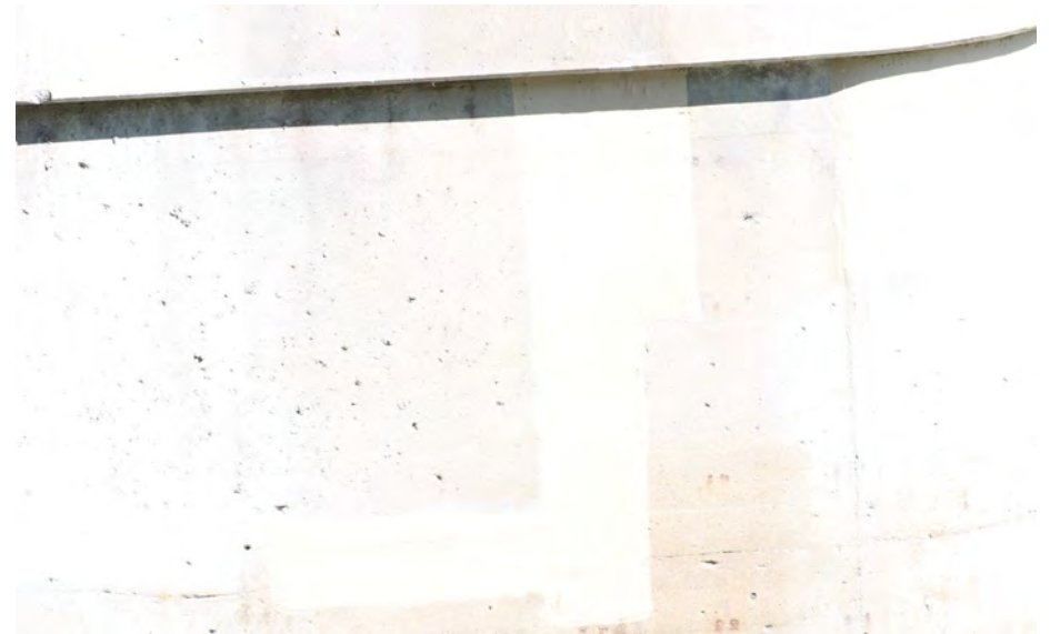
138. Looking North-West at Patching on the East Profile of S.N. 050-0096 Pier #5
