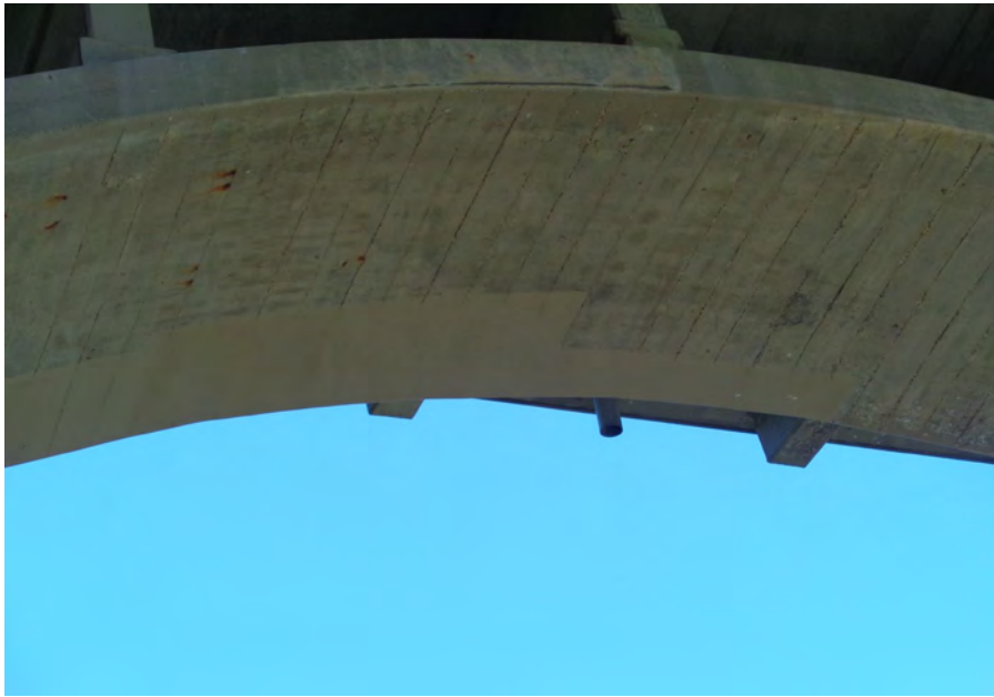
185. Looking Directly Up at Patching underneath S.N. 050-0096 West Span #6
