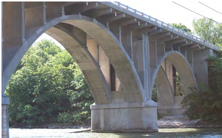
99. Looking South-East at Patching on the West Profile of S.N. 050-0096 Span #5
