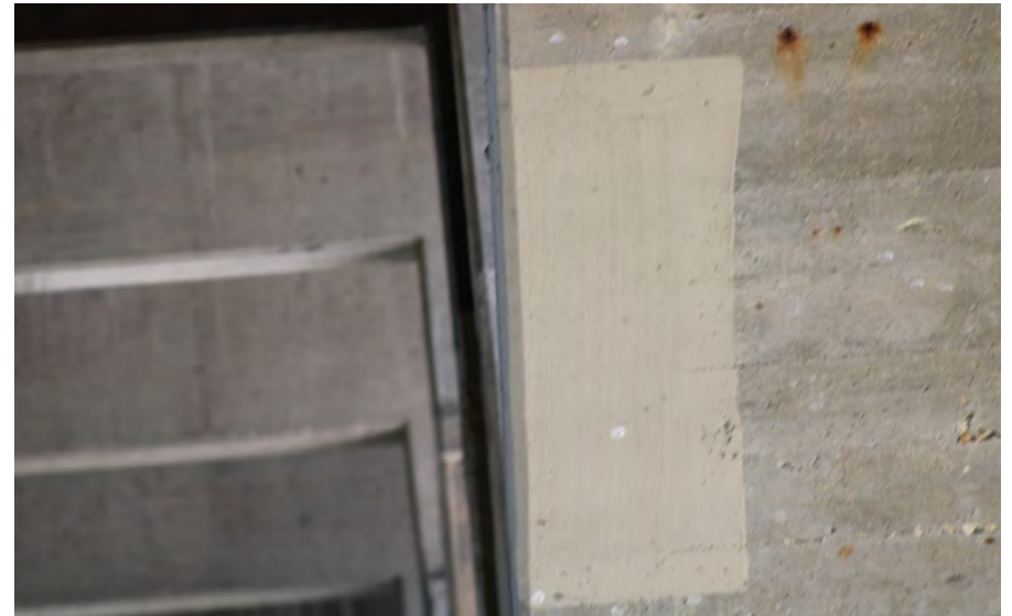
182. Looking Directly Up at Patching underneath S.N. 050-0096 East Span #6
