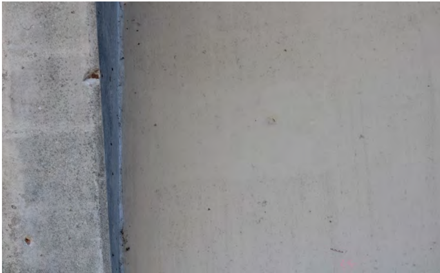
212. Looking South at Patching on the North Profile of S.N. 050-0096 Pier #6
