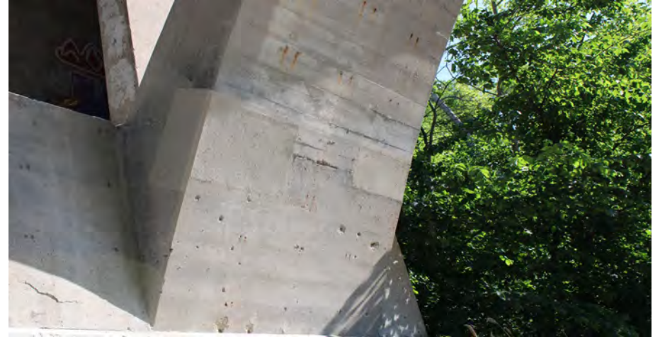
34. Looking North-East at Patching underneath S.N. 050-0096 East Span #4
