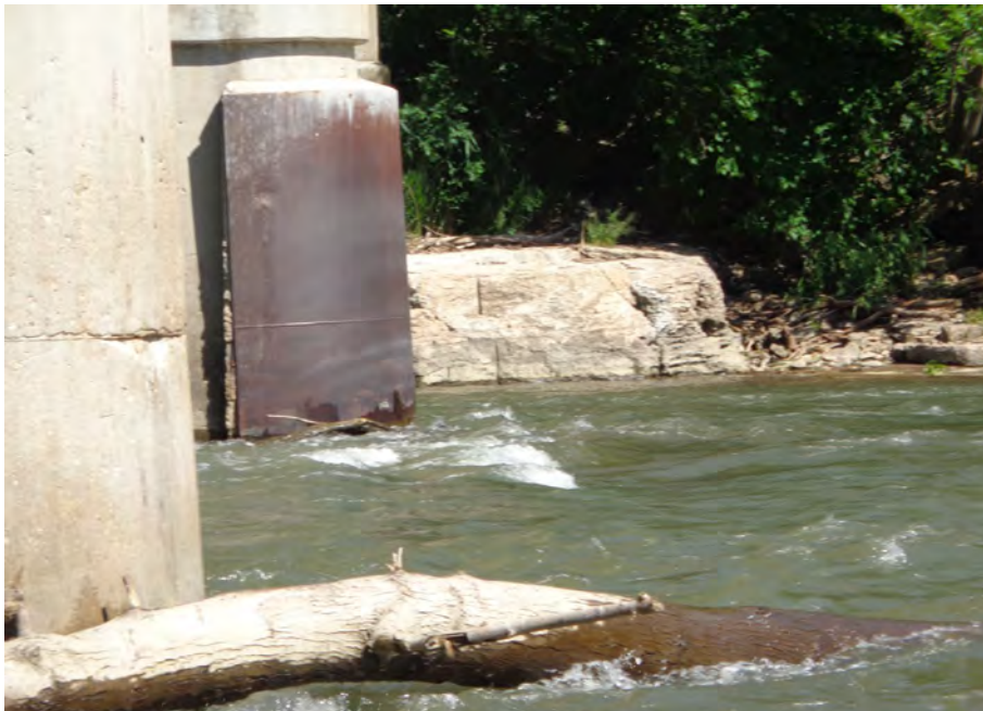
95. Looking North at the East Profile of S.N. 050-0096 Pier #4
