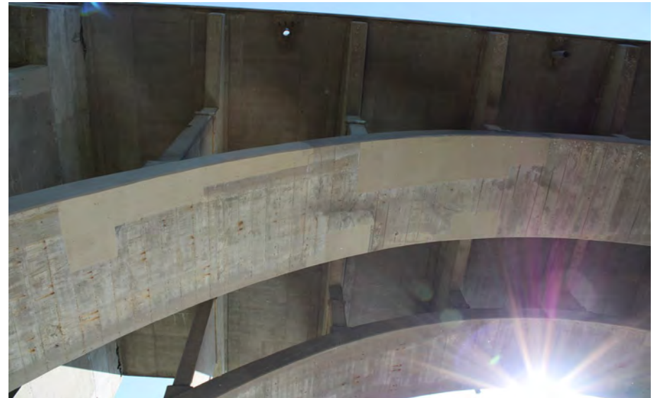
52. Looking East at Patching underneath S.N. 050-0096 West Span #4
