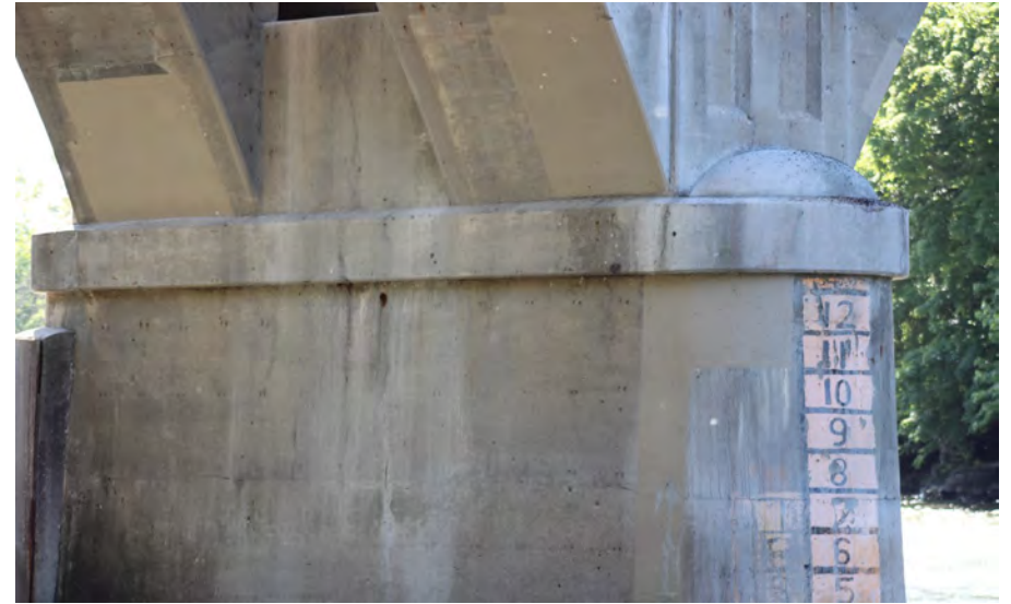
82. Looking South-East at Patching on the West Profile of S.N. 050-0096 Pier #4
