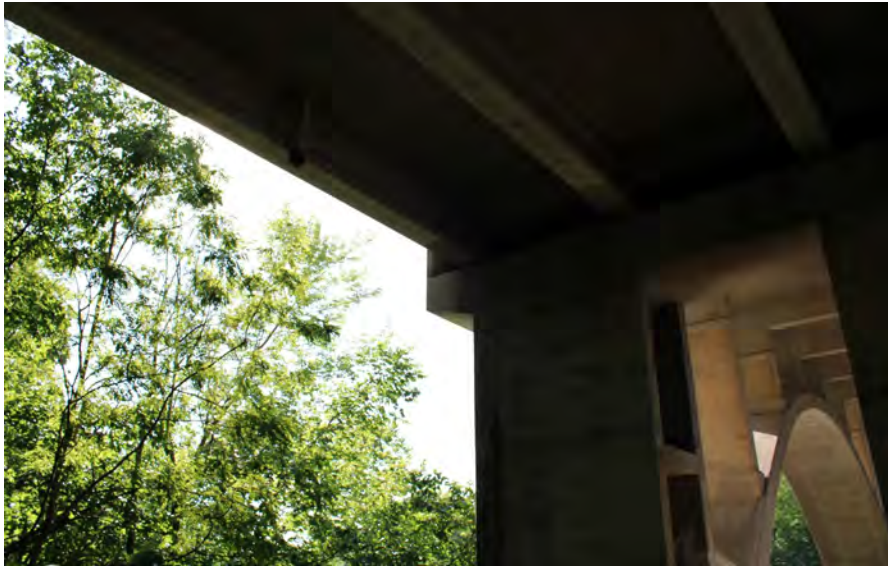
17. Looking South-East at Patching on the North Profile of S.N. 50-0096 East Pier #3
