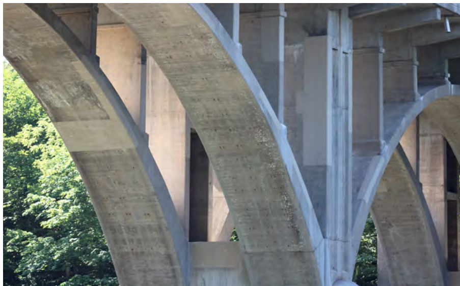
163. Looking South-East at Patching on the West Profile of S.N. 050-0096 Pier #5
