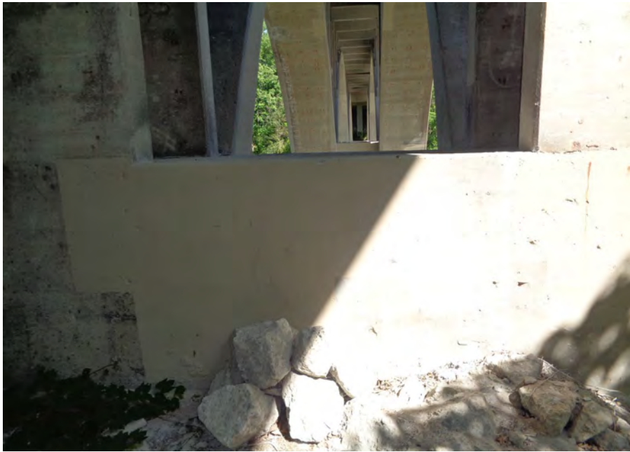
209. Looking North at Patching on the South Profile of S.N. 050-0096 Pier #6
