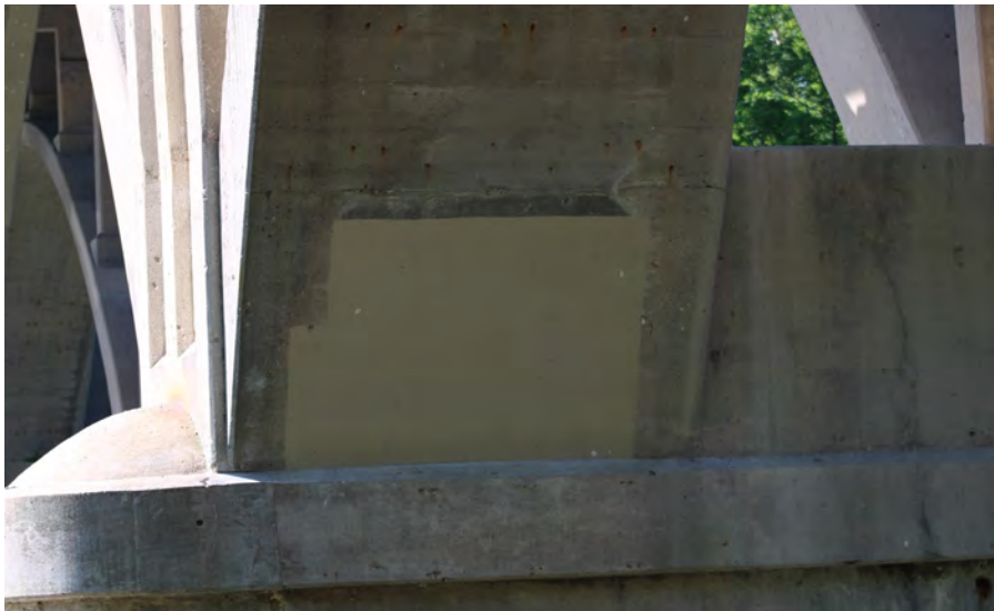
43. Looking South at Patching underneath S.N. 050-0096 East Span #4
