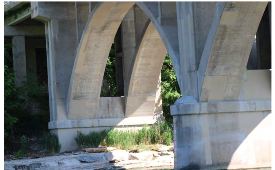
92. Looking North at Patching on the West Profile of S.N. 050-0096 Pier #4
