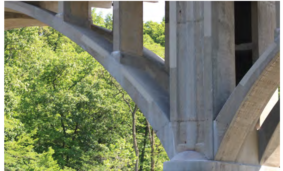
122. Looking East at Patching on the West Profile of S.N. 050-0096 Span #5
