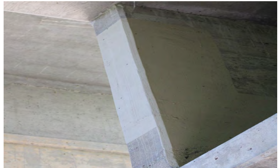
188. Looking North-East at Patching on the inside of S.N. 050-0096 Pier #6
