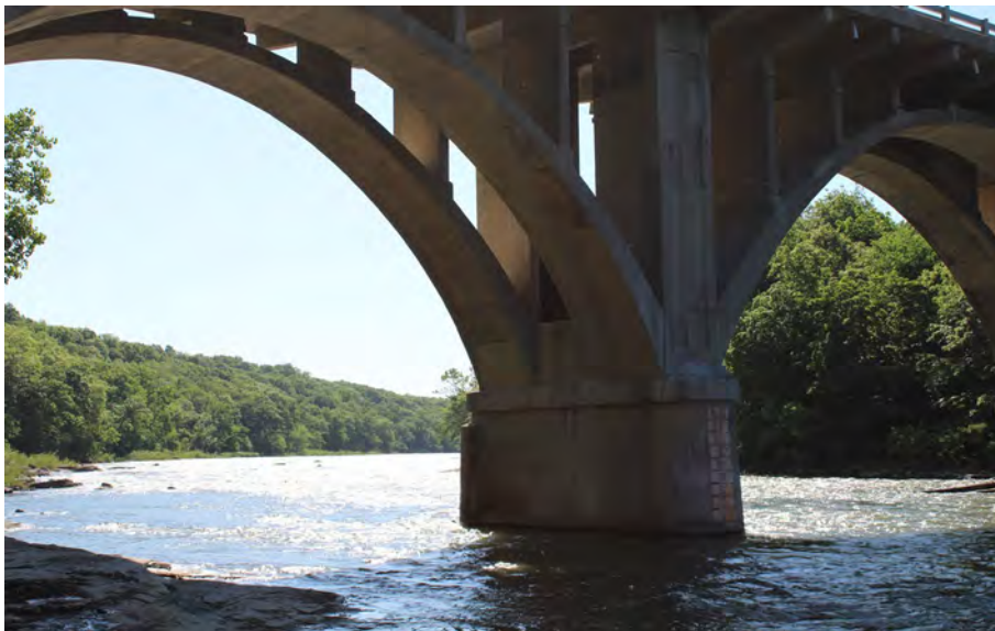
83. Looking South-East at Patching on the West Profile of S.N. 050-0096 Pier #4
