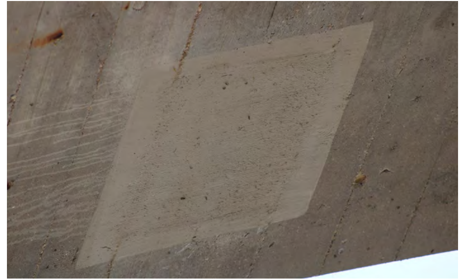
66. Looking East at Patching underneath S.N. 050-0096 East Span #4
