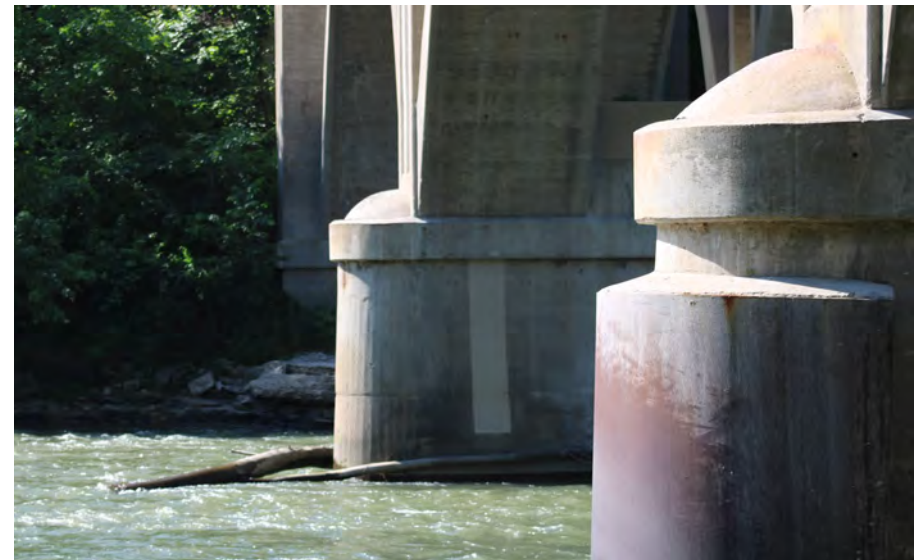
88. Looking South at the East Profile of S.N. 050-0096 Pier #4
