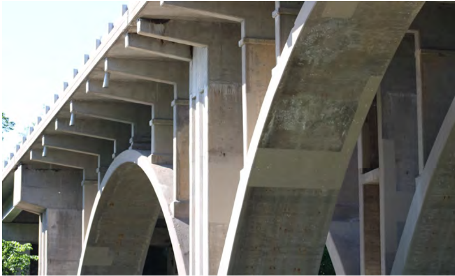
101. Looking South at Patching underneath S.N. 050-0096 East Span #5
