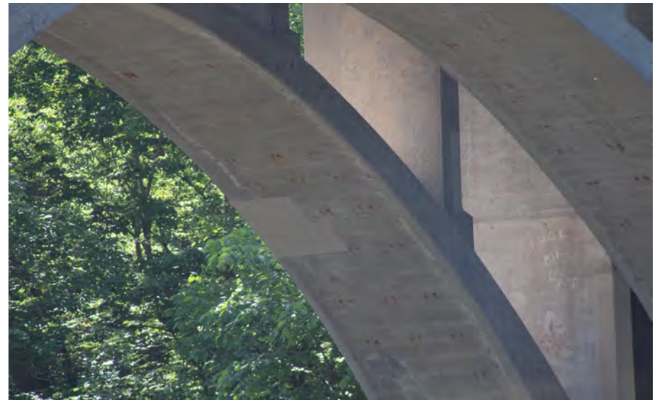
184. Looking South-East at Patching underneath S.N. 050-0096 East Span #6
