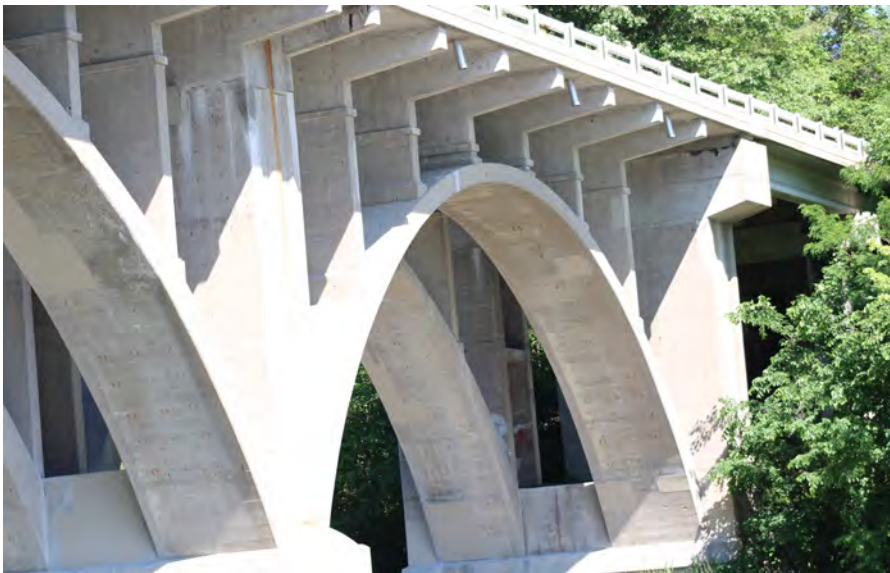
75. Looking North-West at Patching on & under S.N. 050-0096 Span #4
