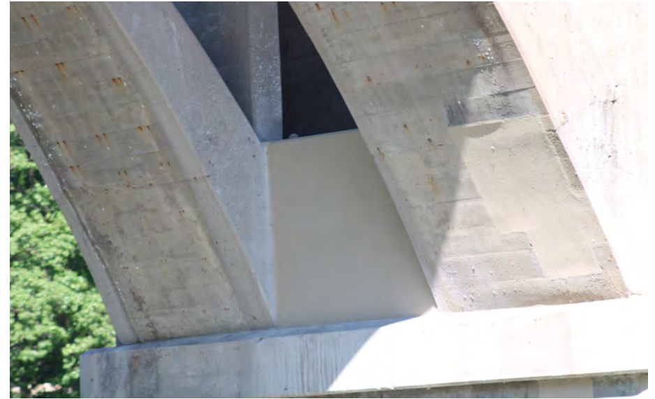
162. Looking North-West at Patching on the South Profile of S.N. 050-0096 Pier #5
