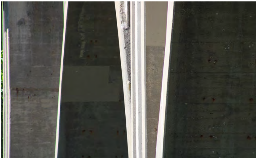
183. Looking South-West at Patching underneath S.N. 050-0096 East Span #6
