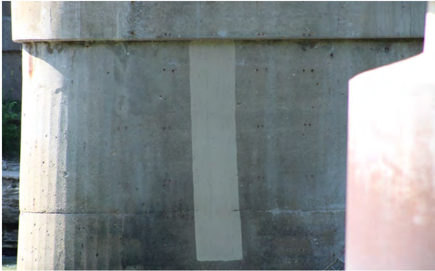
129. Looking South at Patching on the North Profile of S.N. 050-0096 Pier #5
