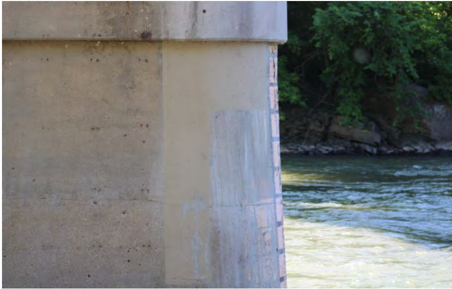
81. Looking South at Patching on the North Profile of S.N. 050-0096 Pier #4
