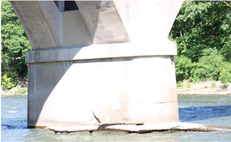
141. Looking West at Patching on the South Profile of S.N. 050-0096 Pier #5
