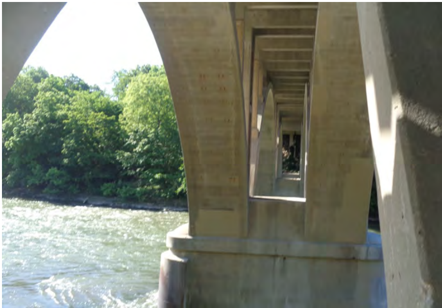
39. Looking South at Patching underneath S.N. 050-0096 Span #4
