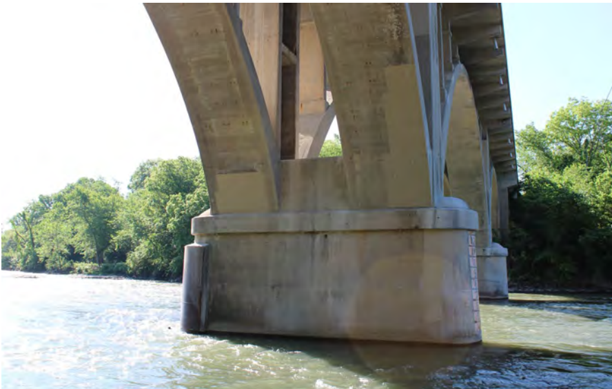
71. Looking South at Patching underneath S.N. 050-0096 Span #4
