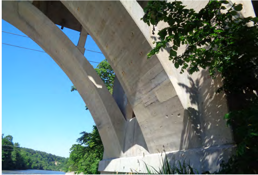
35. Looking West at Patching underneath S.N. 050-0096 West Span #4
