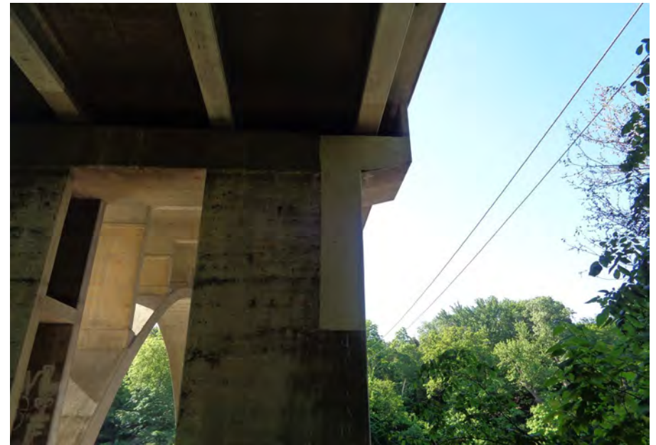
16. Looking South at Patching on the North Profile of S.N. 050-0096 West Pier #3
