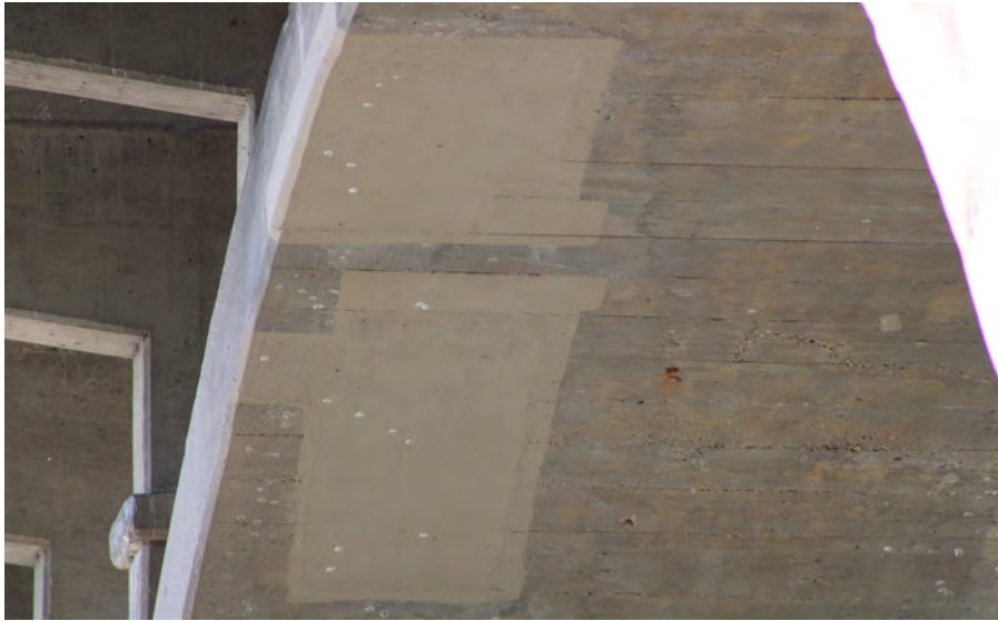
125. Looking South at Patching underneath S.N. 050-0096 East Span #5
