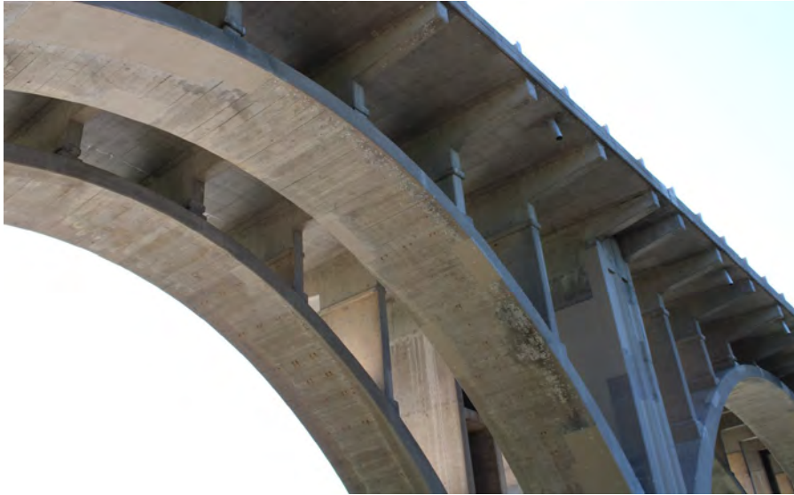
53. Looking East at Patching underneath S.N. 050-0096 West Span #4
