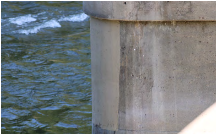
143. Looking North at Patching on the South Profile of S.N. 050-0096 Pier #5
