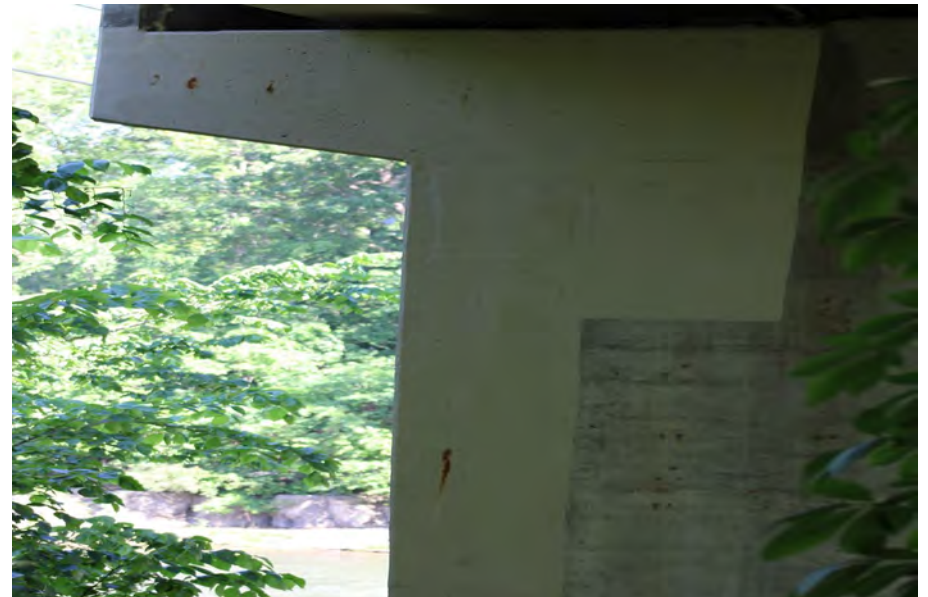
214. Looking North at Patching on the South Profile of S.N. 050-0096 West Pier #7
