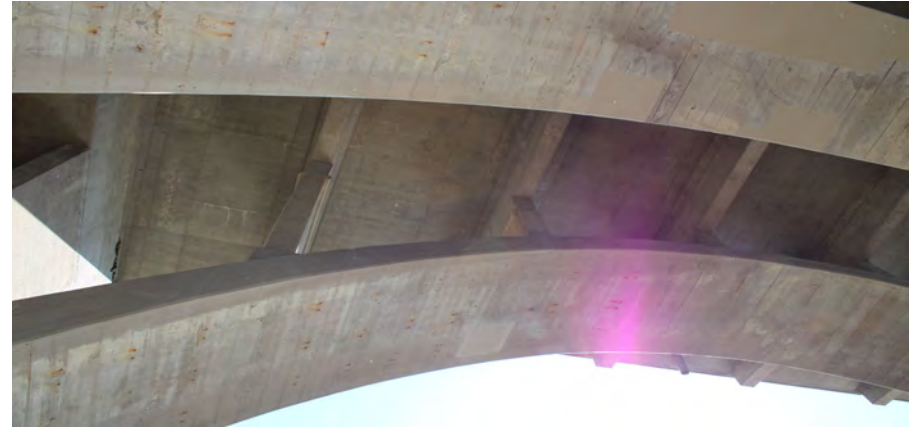
58. Looking East at Patching underneath S.N. 050-0096 East Span #4
