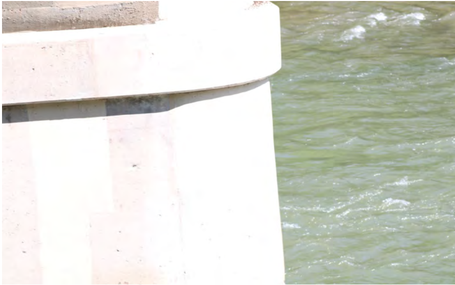
137. Looking North at Patching on the South Profile of S.N. 050-0096 Pier #5
