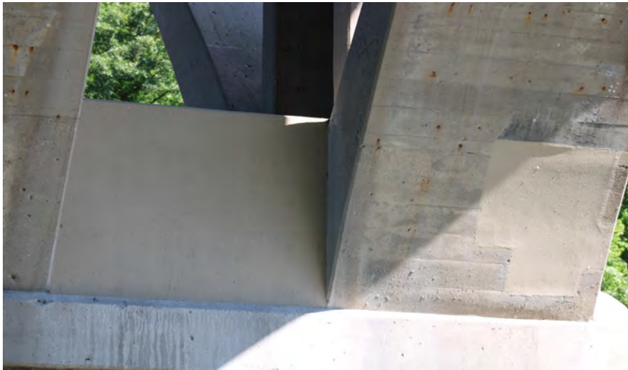
195. Looking North at Patching on the South Profile of S.N. 050-0096 Pier #5
