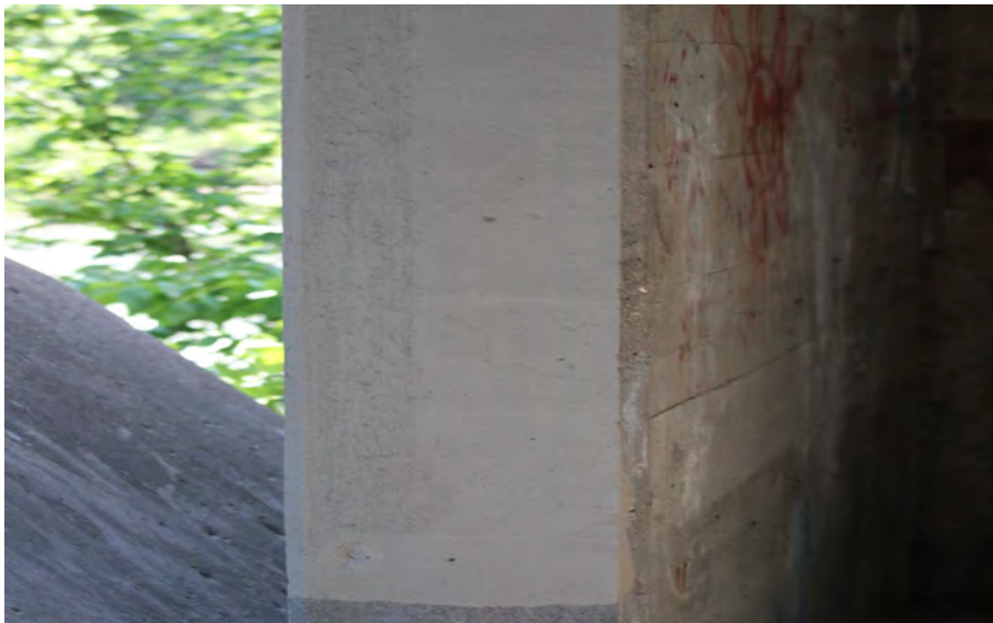
207. Looking East at Patching on the inside of S.N. 050-0096 Pier #6
