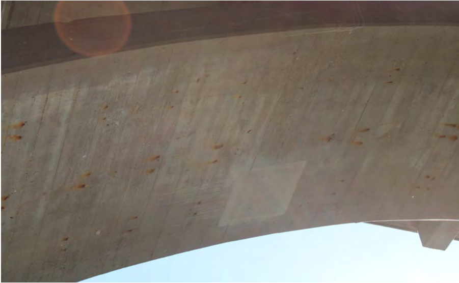
57. Looking East at Patching underneath S.N. 050-0096 East Span #4
