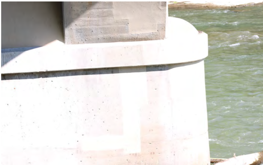
139. Looking North at Patching on the South Profile of S.N. 050-0096 Pier #5
