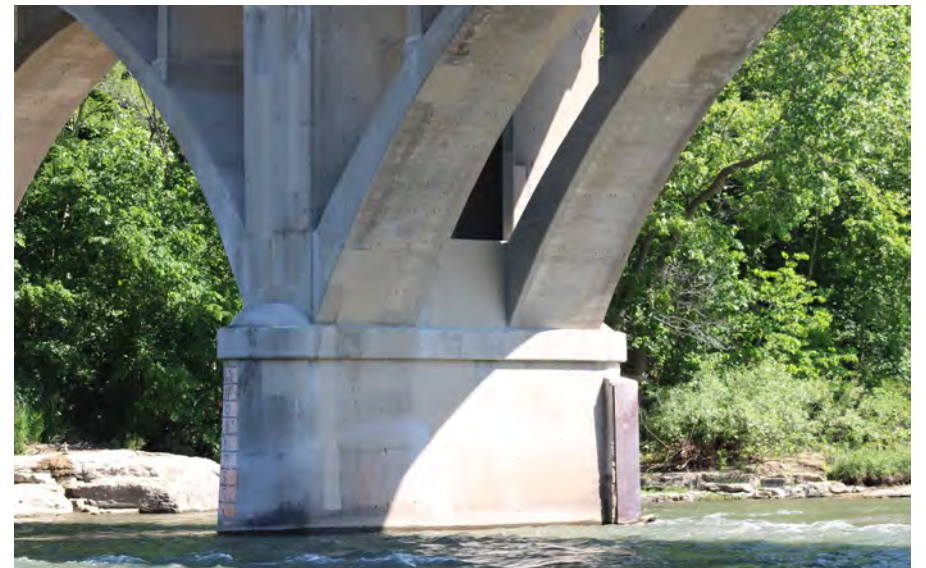
84. Looking North-East at Patching on the South Profile of S.N. 050-0096 Pier #4
