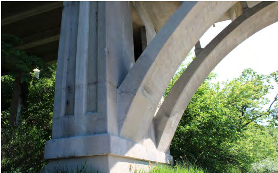
27. Looking East at Patching underneath S.N. 050-0096 Span #4
