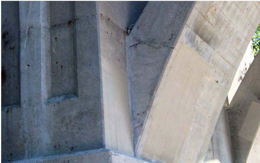
37. Looking North-East at Patching underneath S.N. 050-0096 West Span #4
