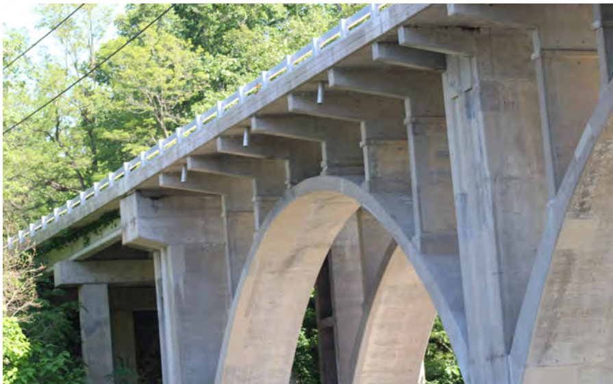
87. Looking North at Patching on the West Profile of S.N. 050-0096 Pier #4
