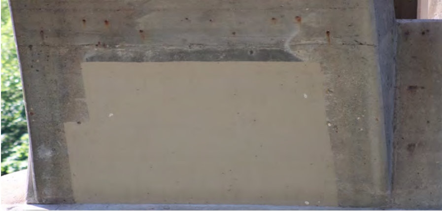
73. Looking South at Patching underneath S.N. 050-0096 East Span #4
