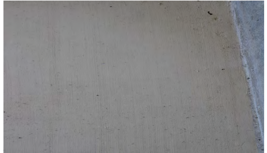
213. Looking South at Patching on the North Profile of S.N. 050-0096 Pier #6
