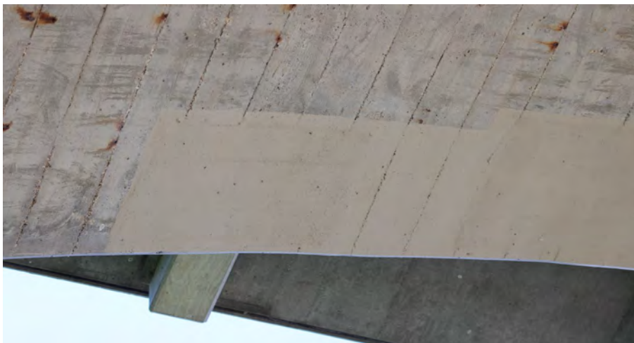
191. Looking Directly Up at Patching underneath S.N. 050-0096 West Span #6
