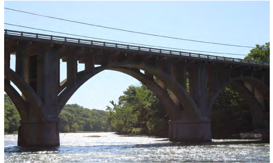
2. Looking East at Patching on the West Profile of S.N. 050-0096
