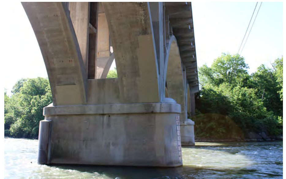
68. Looking South at Patching underneath S.N. 050-0096 Span #4
