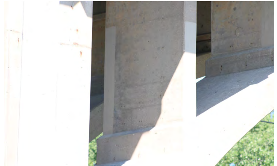
126. Looking North-West at Patching on S.N. 050-0096 East Span #5
