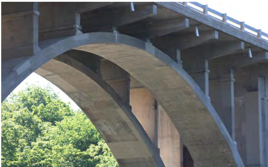
103. Looking South-East at Patching on the West profile of S.N. 050-0096 Span #5
