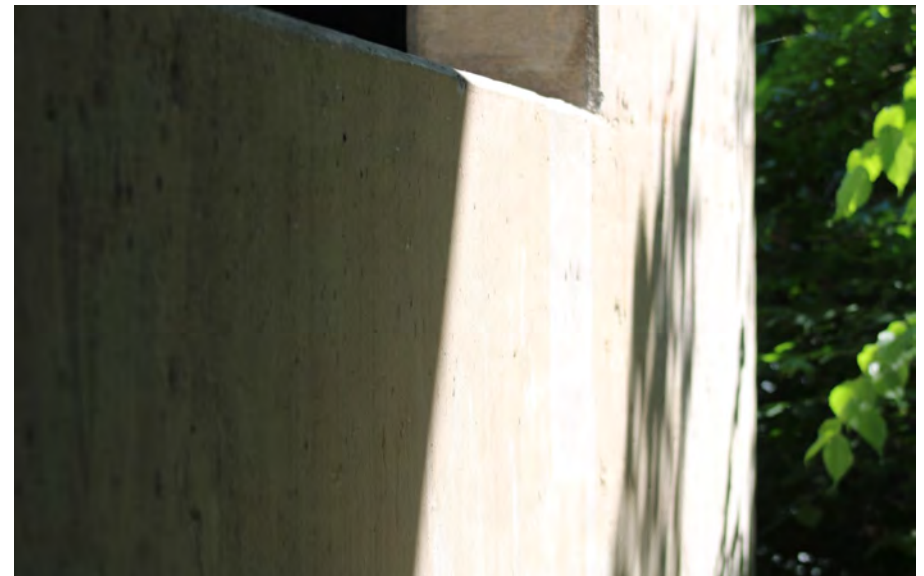
211. Looking East at Patching on the South Profile of S.N. 050-0096 Pier #6
