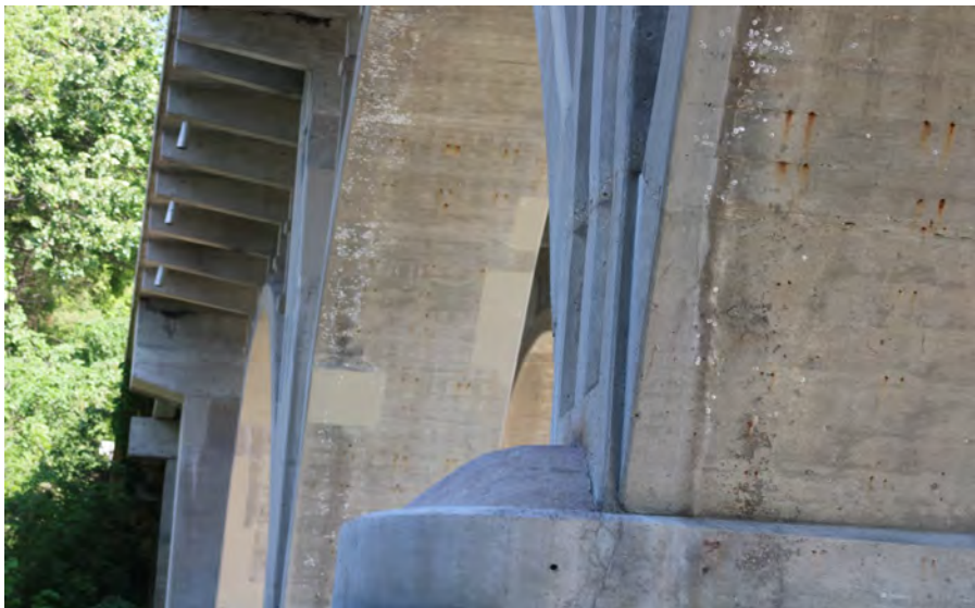
123. Looking North at Patching underneath S.N. 050-0096 West Span #5
