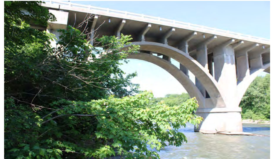
170. Looking West at Patching on the East Profile of S.N. 050-0096 Span #6
