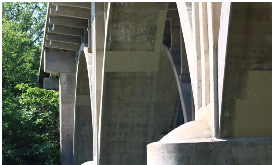
107. Looking South at Patching underneath S.N. 050-0096 East Span #5
