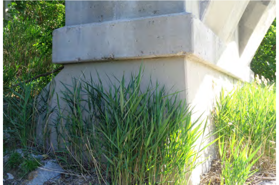
32. Looking East at Patching on the South Profile of S.N. 050-0096 West Pier #3
