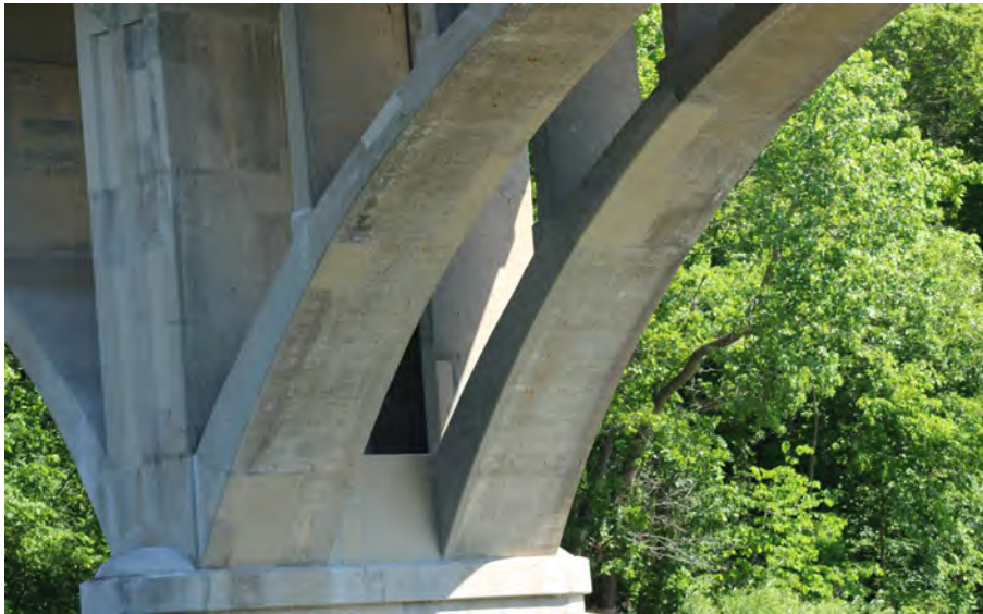
167. Looking North-East at Patching underneath S.N. 050-0096 Span #5
