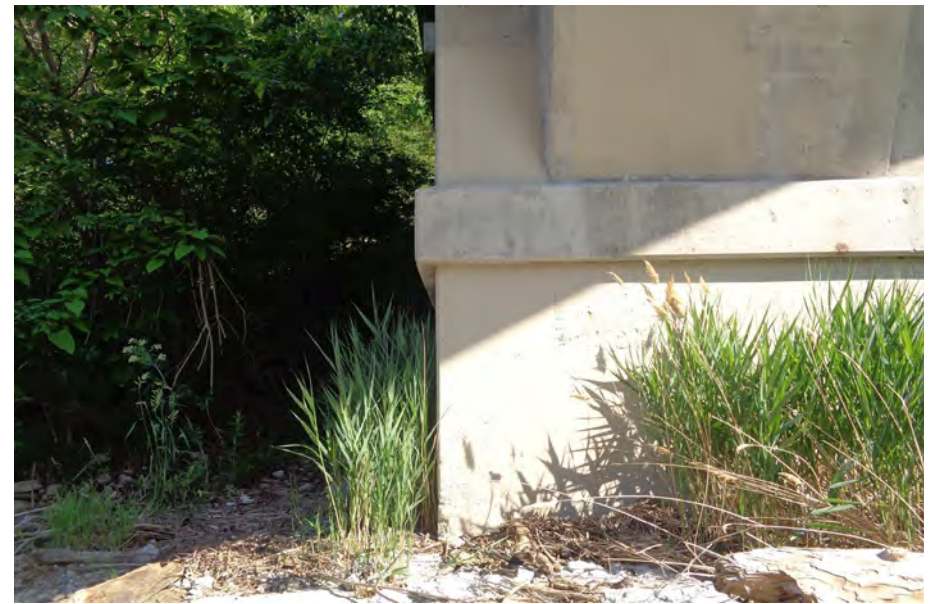
30. Looking North at Patching on the South Profile of S.N. 050-0096 West Pier #3
