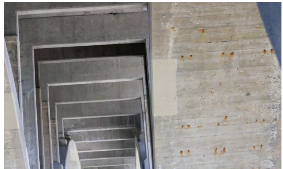
192. Looking North at Patching underneath S.N. 050-0096 East Span #6
