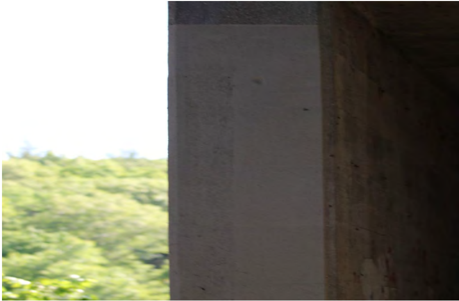
205. Looking East at Patching on the inside of S.N. 050-0096 Pier #6
