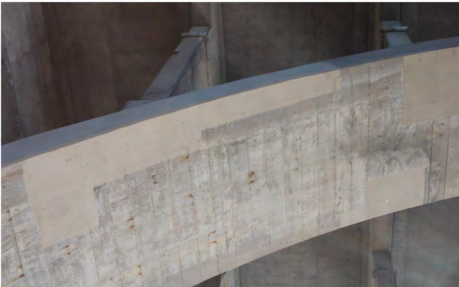
51. Looking East at Patching underneath S.N. 050-0096 West Span #4
