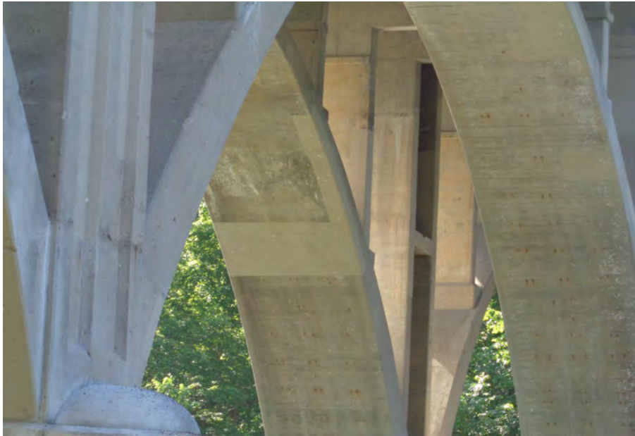
105. Looking South-East at Patching underneath S.N. 050-0096 East Span #5
