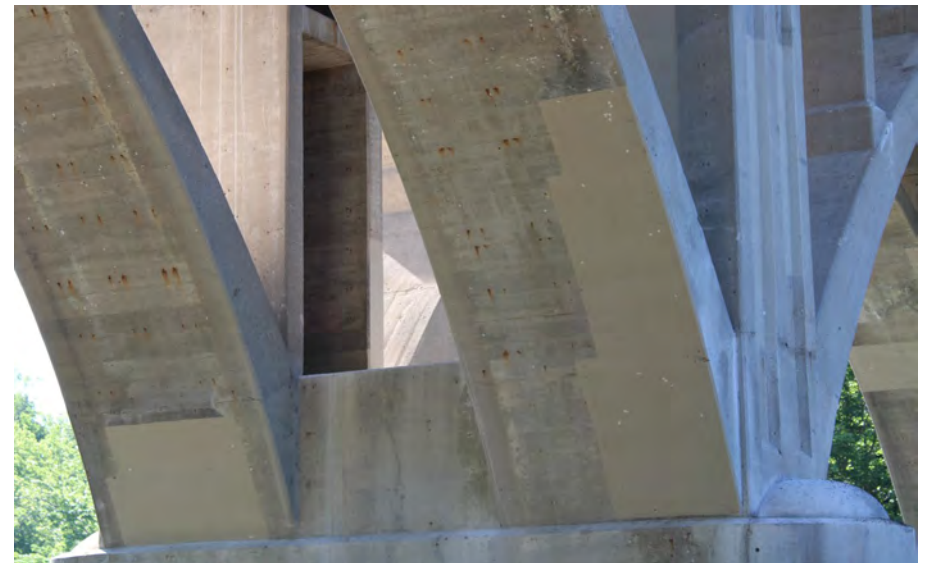
56. Looking South-East at Patching underneath S.N. 050-0096 Span #4
