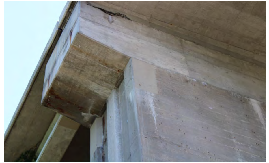
26. Looking North at Patching on the South Profile of S.N. 050-0096 West Pier #3
