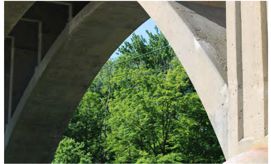
102. Looking South-West at Patching underneath S.N. 050-0096 West Span #5
