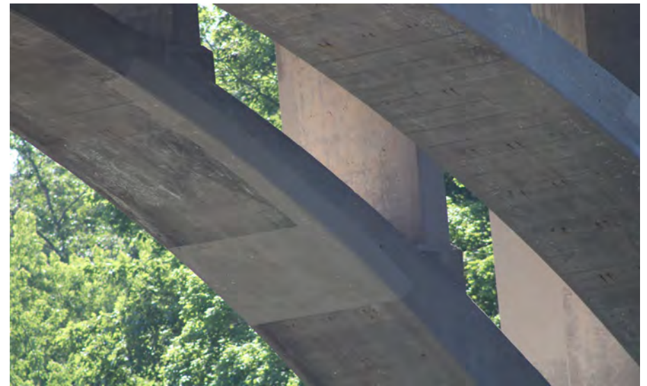
114. Looking South-East at Patching underneath S.N. 050-0096 East Span #5
