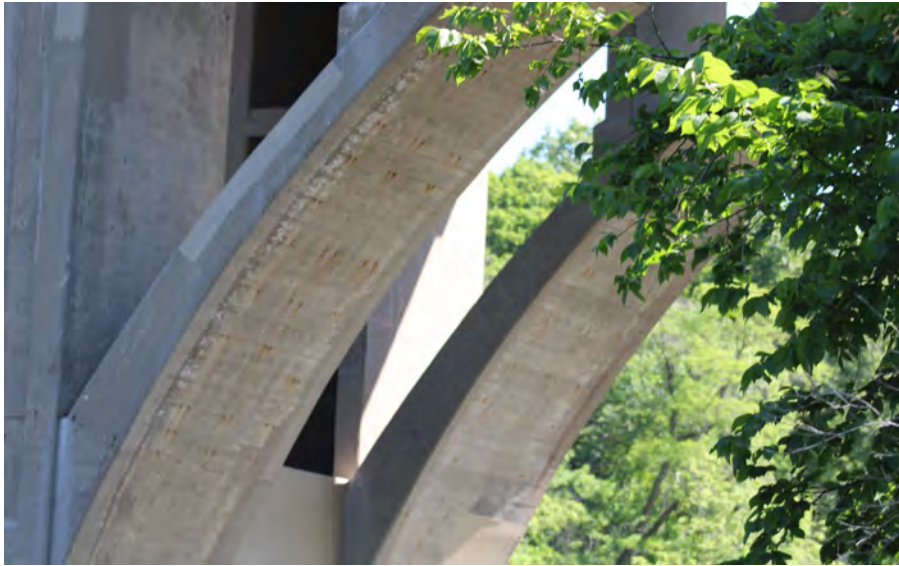
165. Looking North-East at Patching on the South Profile of S.N. 050-0096 Pier #5
