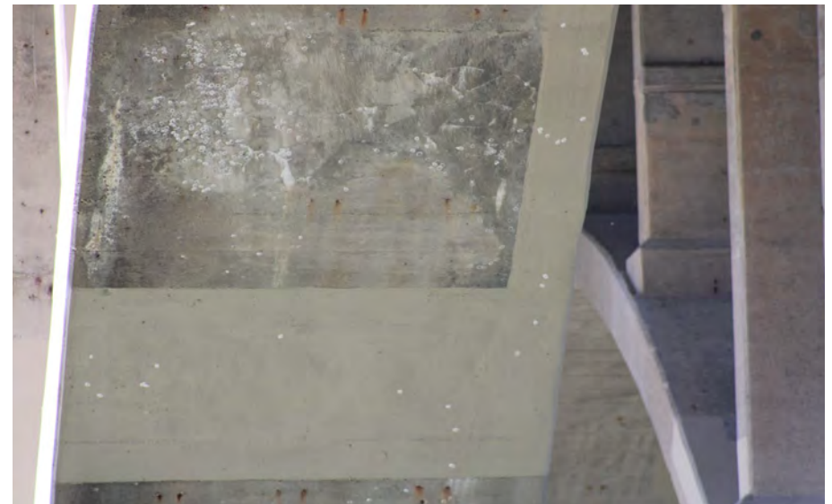
108. Looking South at Patching underneath S.N. 050-0096 East Span #5
