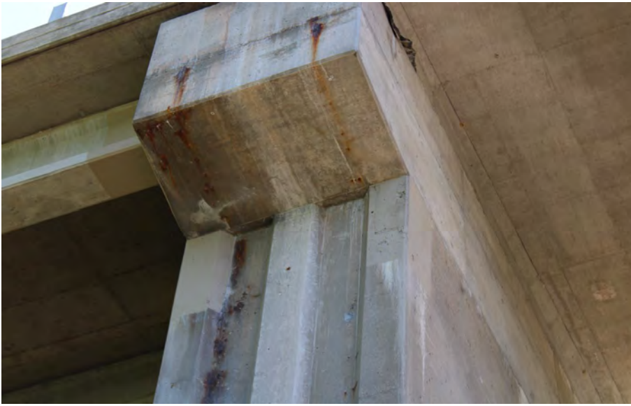
25. Looking East at Patching on the West Profile of S.N. 050-0096 West Pier #3
