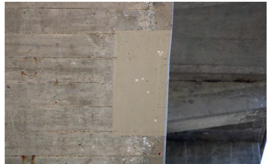
64. Looking South at Patching underneath S.N. 050-0096 West Span #4
