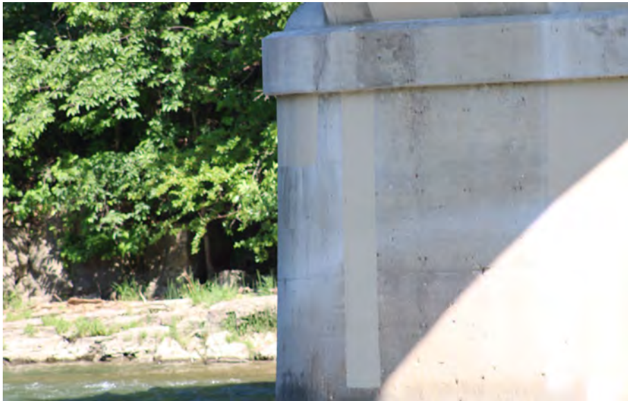
91. Looking North at Patching on the South Profile of S.N. 050-0096 Pier #4
