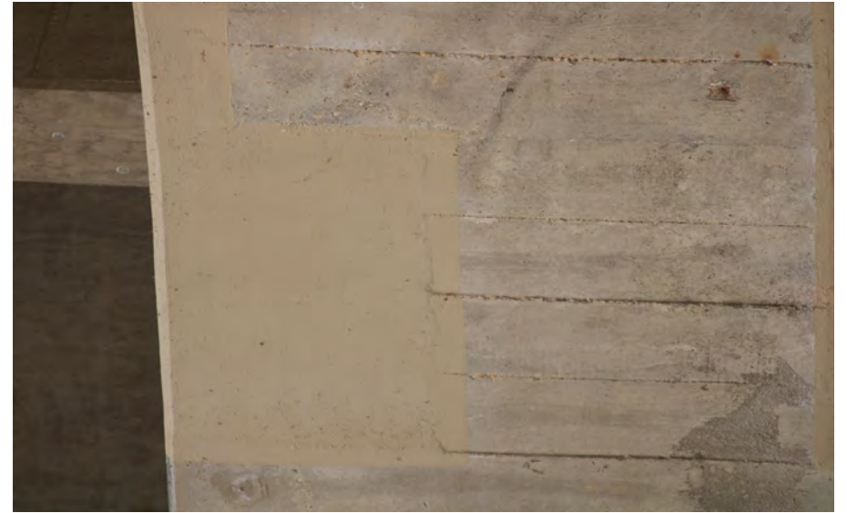
74. Looking South at Patching underneath S.N. 050-0096 West Span #4
