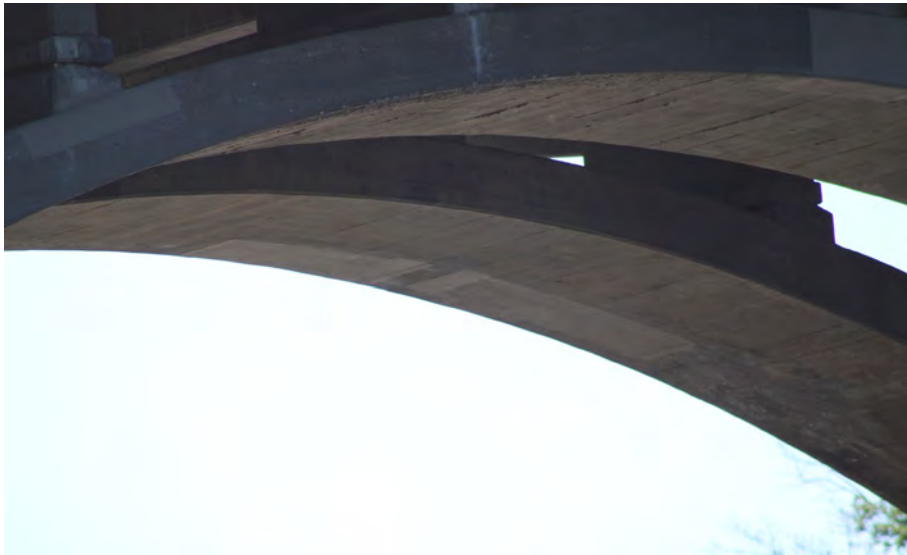
113. Looking South-East at Patching underneath S.N. 050-0096 East Span #5
