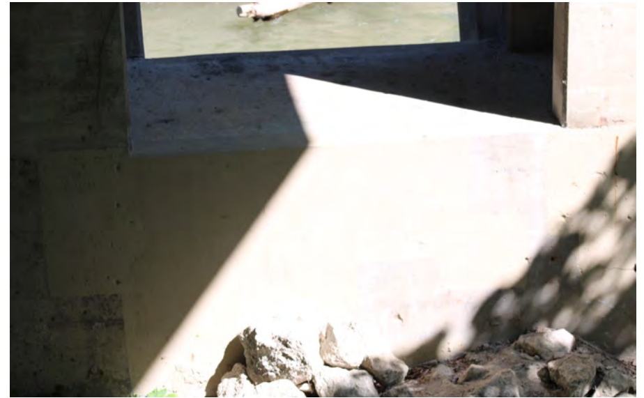
210. Looking North at Patching on the South Profile of S.N. 050-0096 Pier #6
