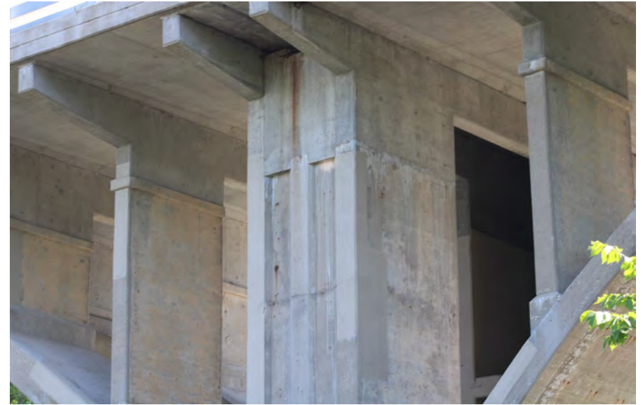
142. Looking North-East at Patching on the West Profile of S.N. 050-0096 Pier #5
