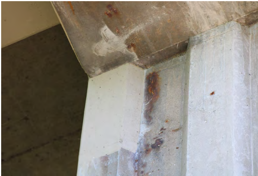
23. Looking East at Patching on the West Profile of S.N. 050-0096 West Pier #3
