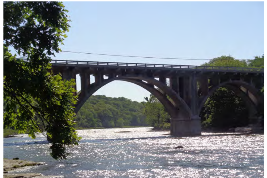
4. Looking East at Patching on the West Profile of S.N. 050-0096
