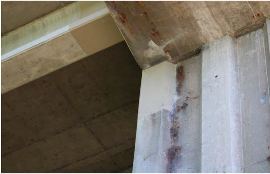
21. Looking East at Patching on the West Profile of S.N. 050-0096 West Pier #3
