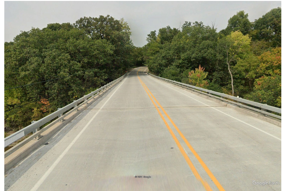
Looking North along IL 178 from S.N. 050-0096 at Sta. 197+40
