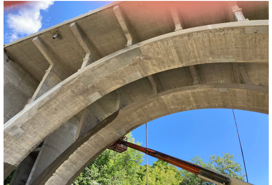
Looking straight up at patching underneath S.N. 050-0096 Span #4
