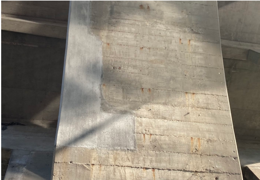
Looking North at patching underneath S.N. 050-0096 Span #4
