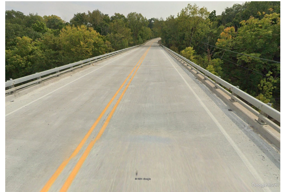
Looking South along IL 178 from S.N. 050-0096 at Sta. 197+40
