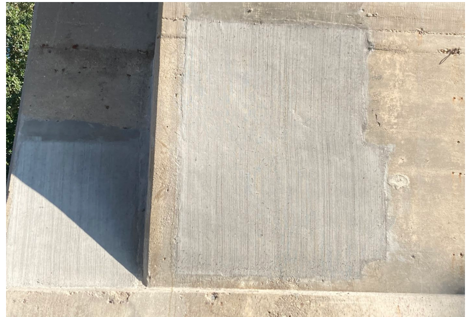
Looking North at patching on the South profile of S.N. 050-0096 Pier #3
