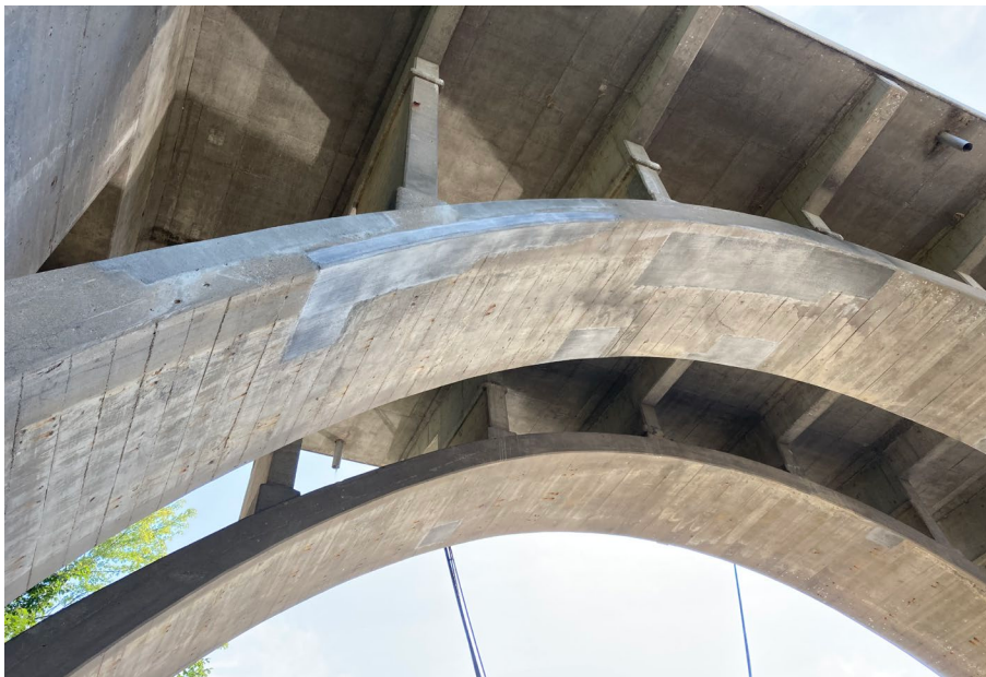
Looking East at patching on the West profile of S.N. 050-0096 Span #4
