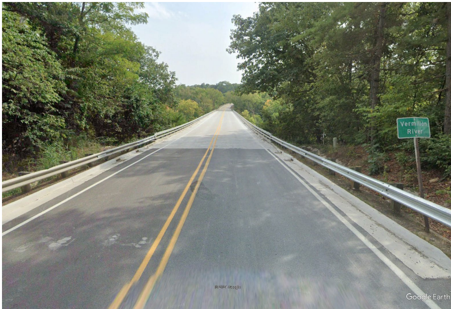
Looking South along IL 178 through S.N. 050-0096
