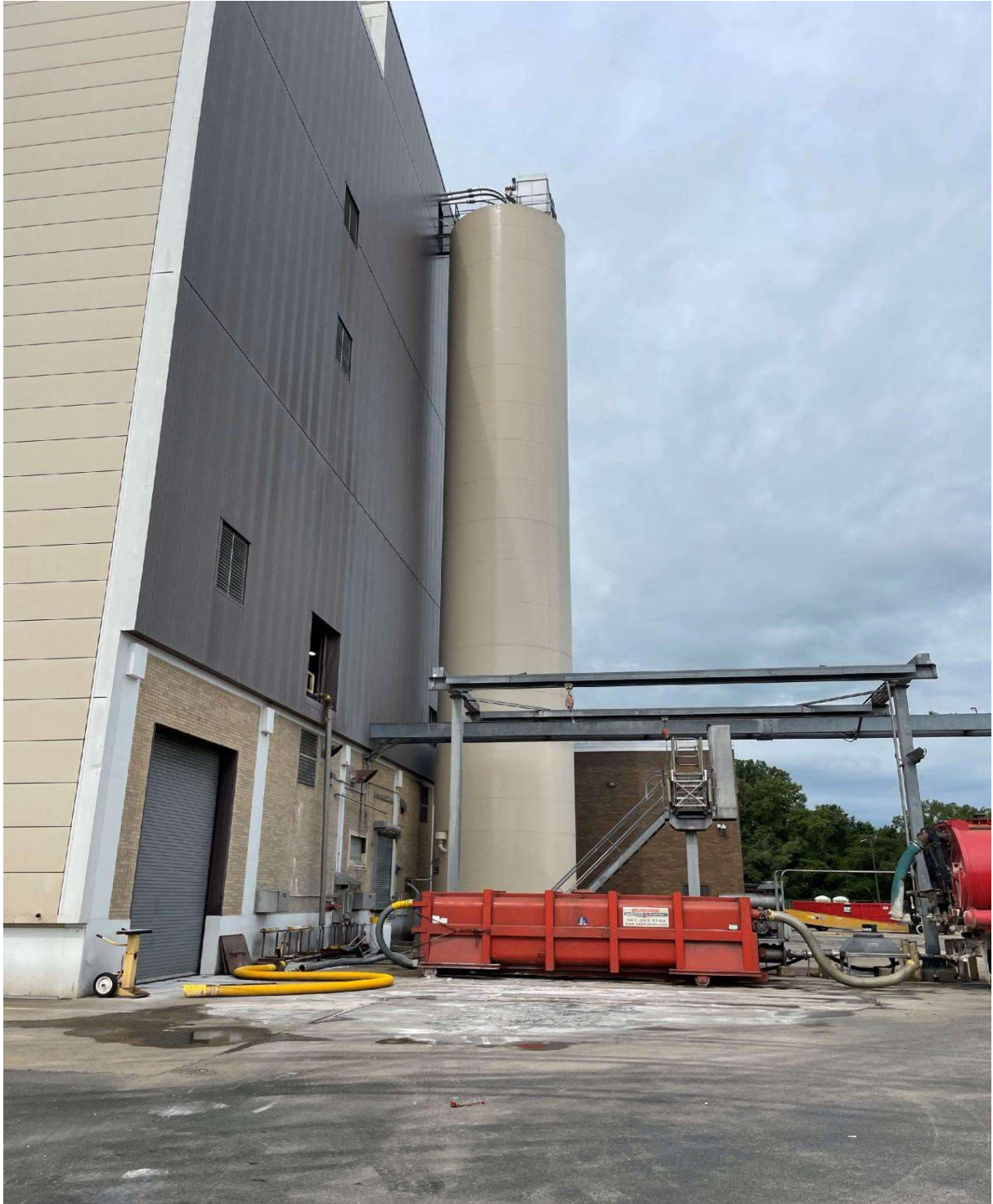
South side of the building looking west
