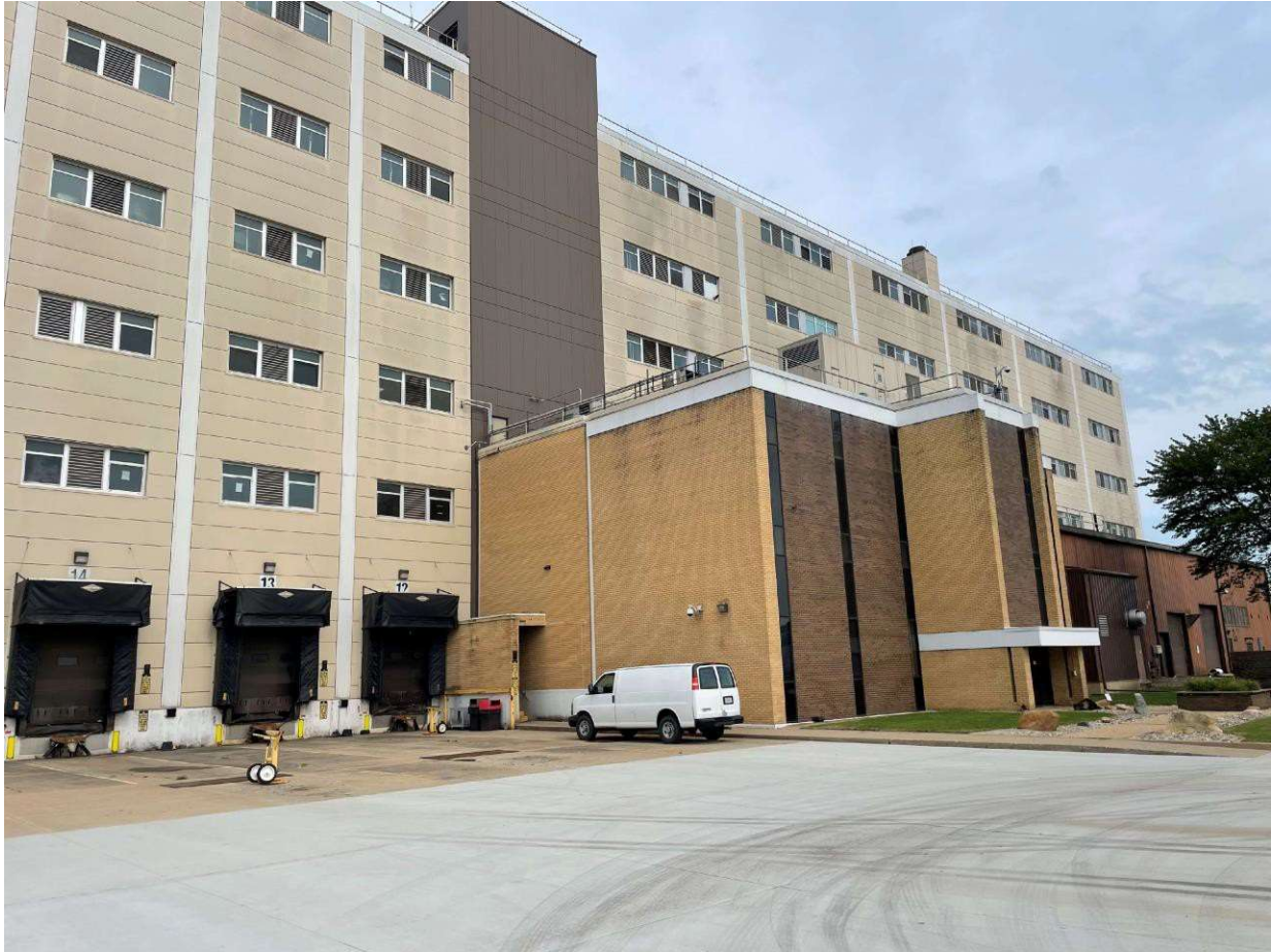
East side of the building looking west
