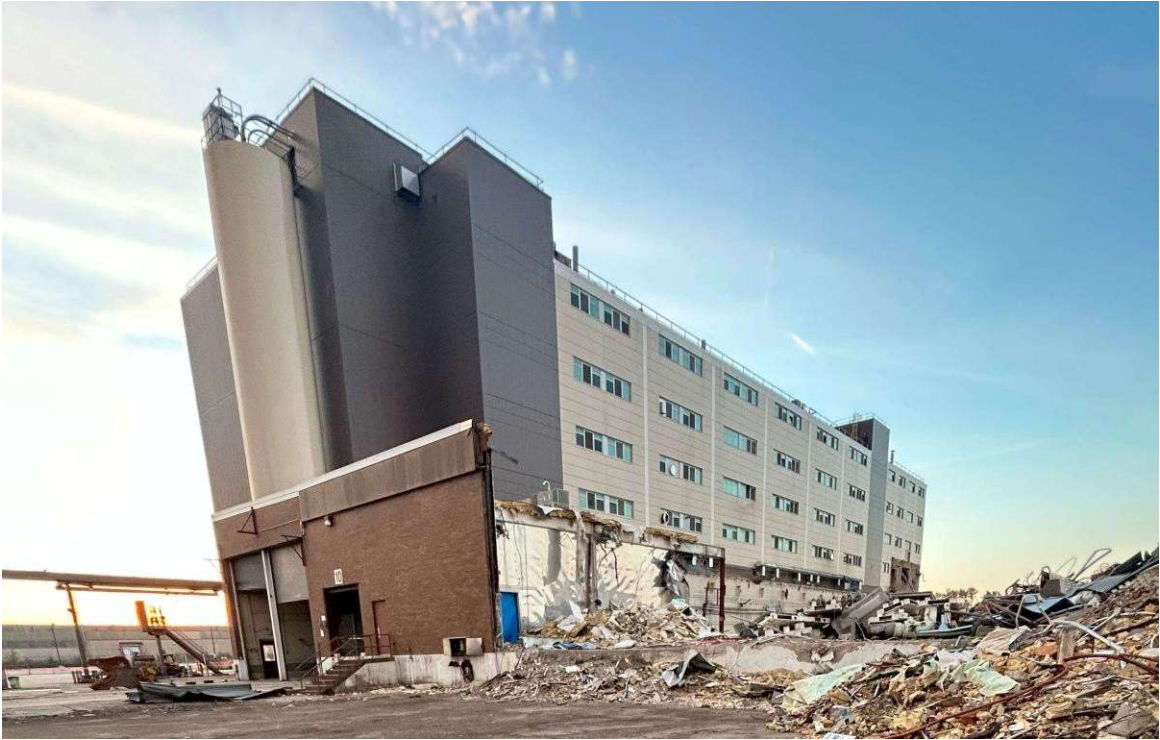
West side of building:
