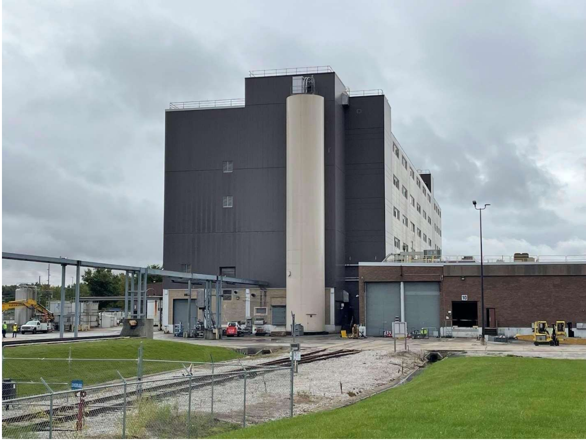
South side of the building looking north
