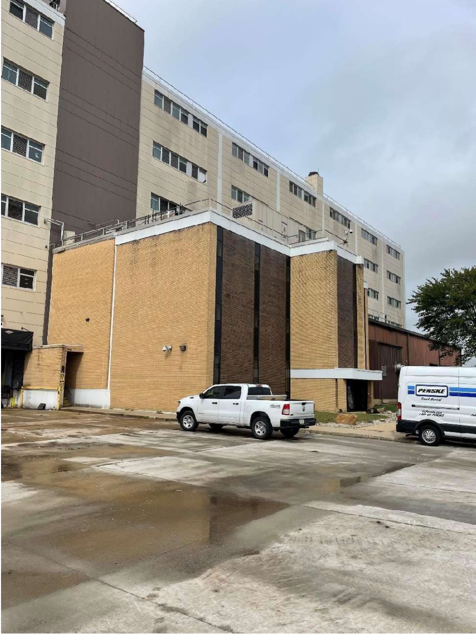
East side of the building looking northeast
