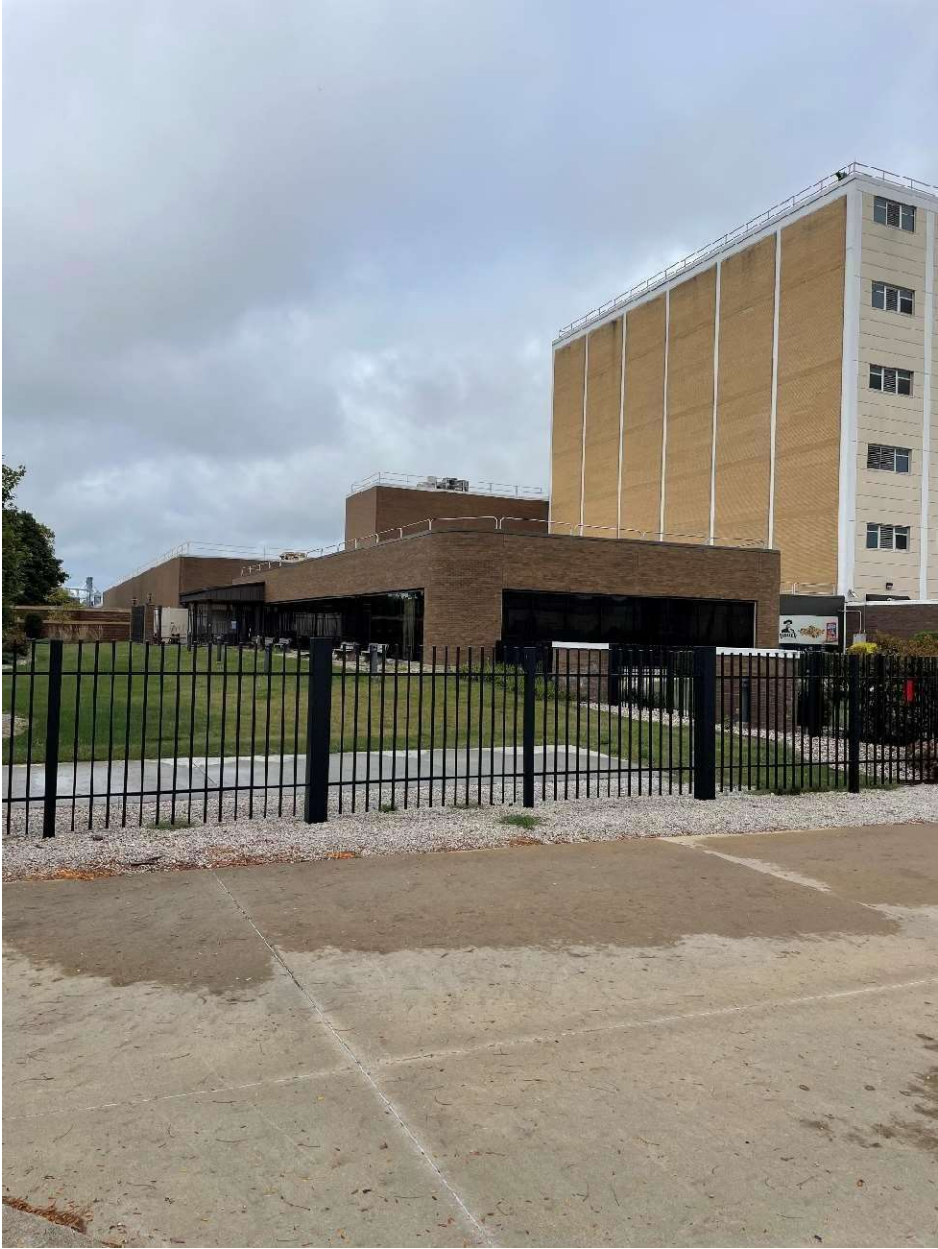
Front of the building from the east side
