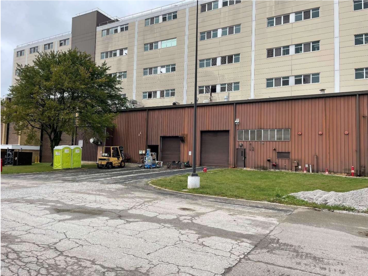
East side of the building:
