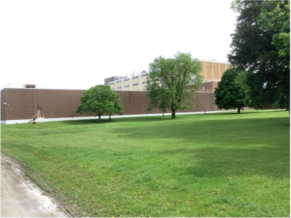
Subject Property from the southwest corner
