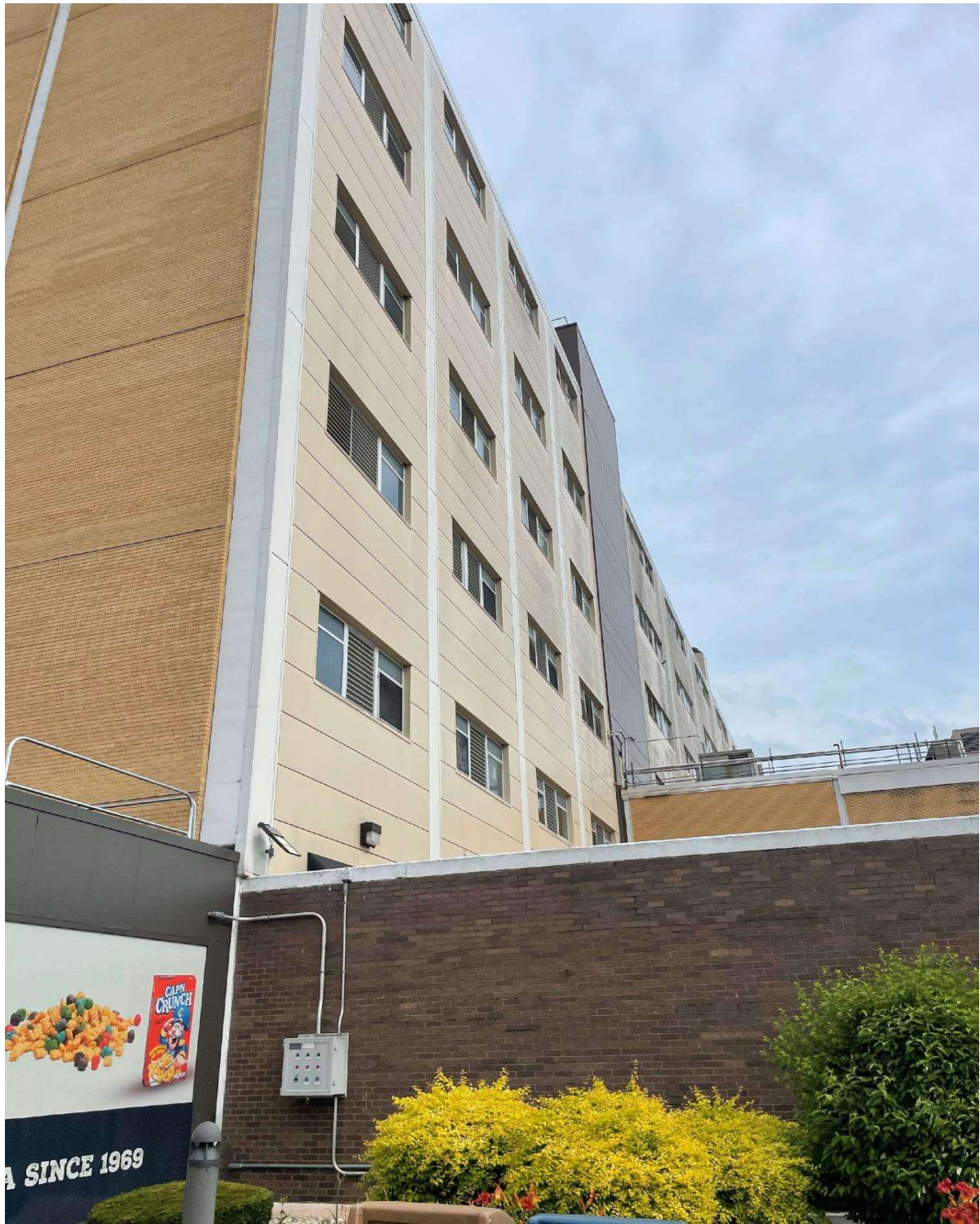
Front and east side of the building
