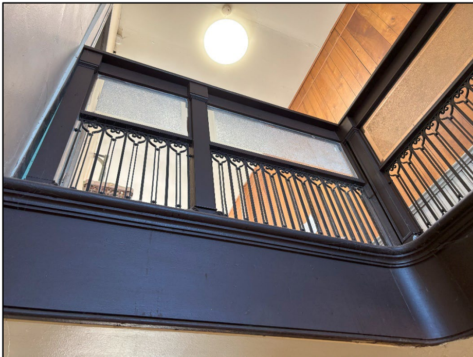
Plate 13. Detail of surviving Art Deco Opera House railing and wooden paneling
