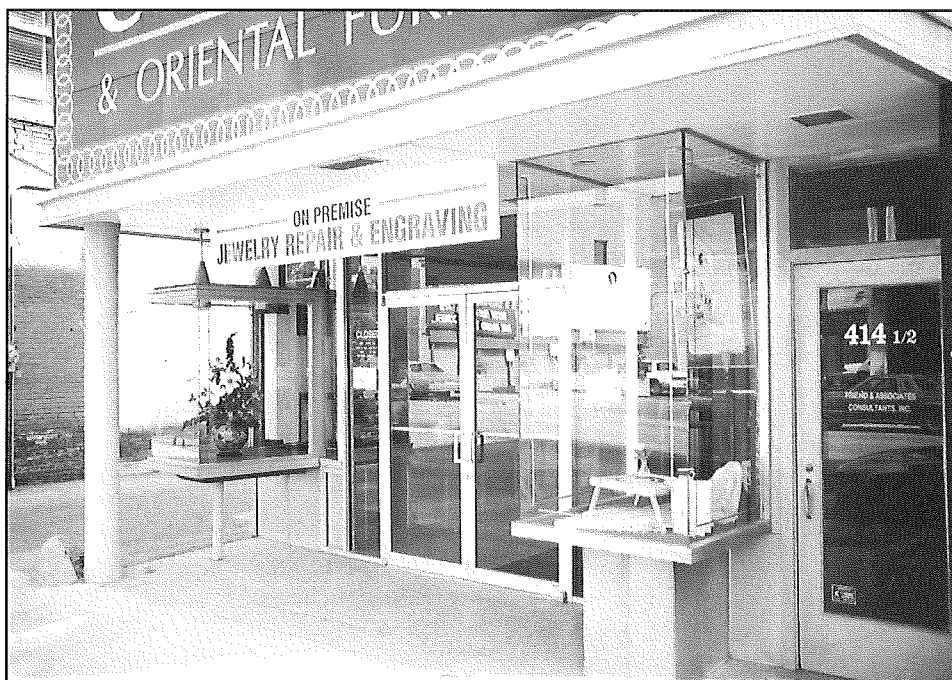
Figure 4. Springfield, Illinois. Corso Jewelry, circa 1960. This small shopfront is a well-preserved example of the “open front” with “floating” display window boxes that project so far out they required supporting columns. The display windows are framed with a mullionless system of clips to maximize the display window viewing. Photograph by the author.
