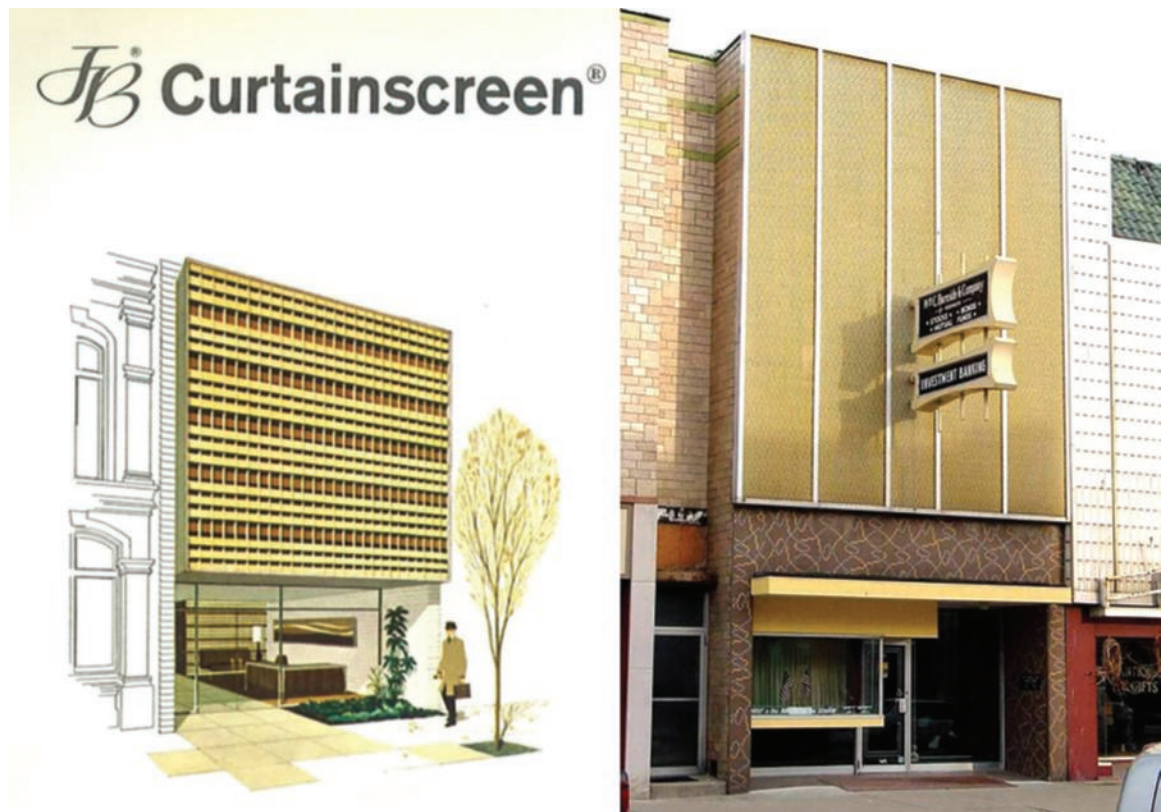
Figure 6: On the left is “The Art of Refacing the New Art in Architecture” Julius Blum & Co.’s JB Curtainscreen, 1965. On the right, Burnside and Co., in Danville, Illinois, is an excellent example of an unusually intact design with gold anodized aluminum slipcover, cantilevered display case, decoratively tiled storefront, and period signage and deserves preservation.
