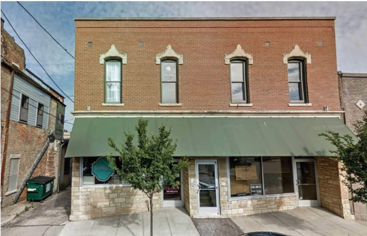
Figure 8: For purposes of the federal historic tax credit project the SHPO explained that the mid-century storefront was historic and required its retention. The owner kept the mid-century storefront and installed a compatible clear-view door, restored the white metal window framing and added a canvas awning.
