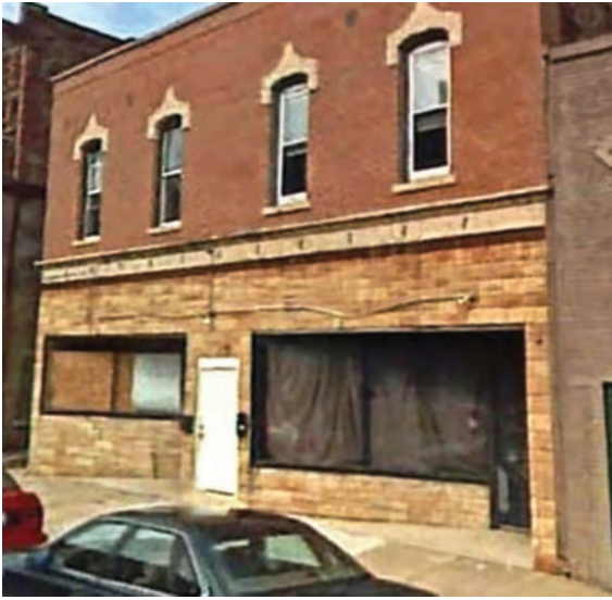
Figure 6: This ca. 1890 building in Rockford, Illinois received a number of alterations during the period of significance of the historic district, including the installation of an angled mid-century stone veneer storefront. Sometime after the period of significance the mid-century storefront window frames were painted dark and a later door installed.
