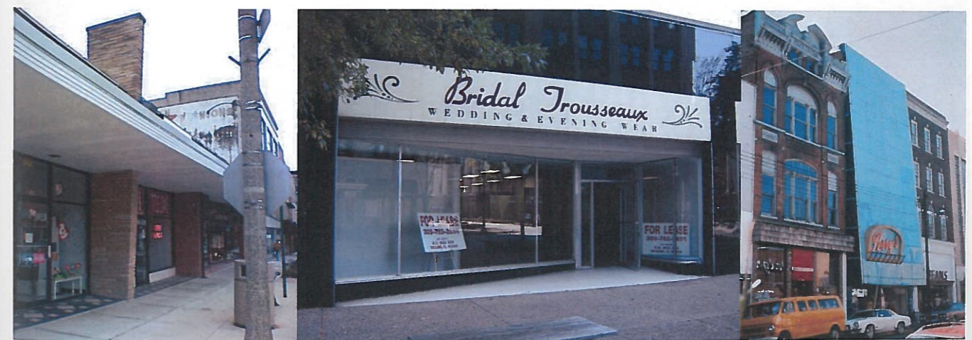
Figure 4: Left, a Freeport, Illinois, angled stone pylon. Center, a Moline, Illinois example of the common post-war angled open storefront, shown here in structural glass. Right, a much more unusual design angles the entire porcelain enamel facade out from top to base. Left photo: author, center and right photos: IHPA archives
