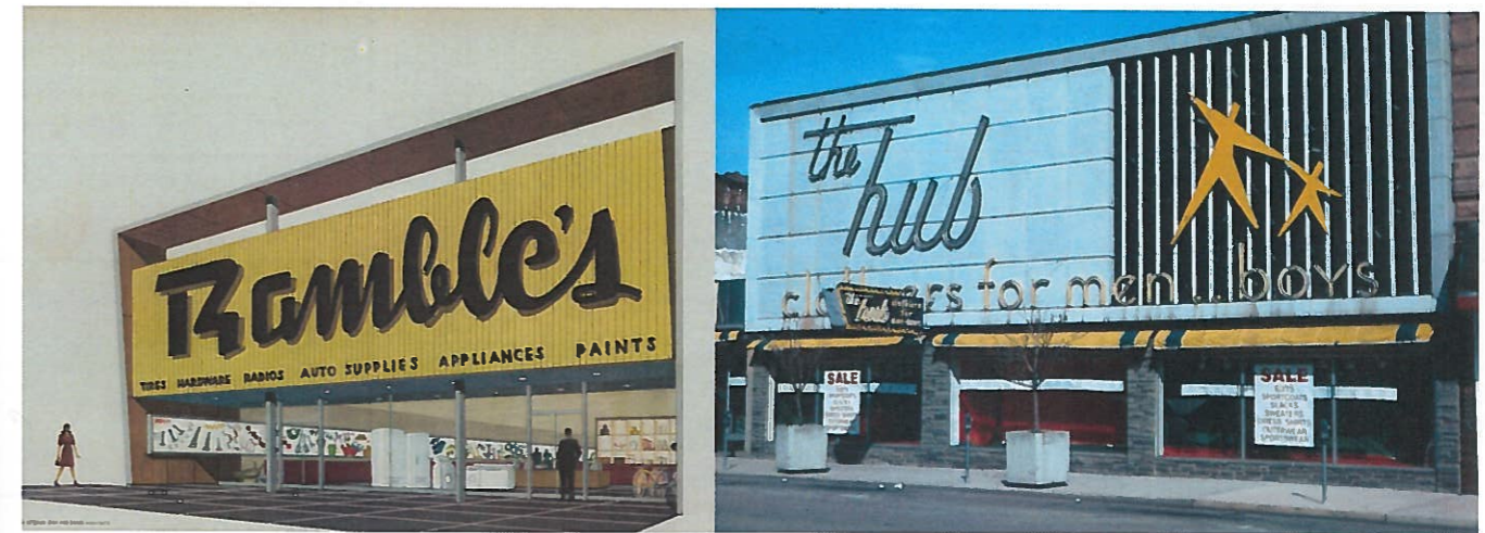
Figure 3: Left, The Rambles hardware store design by Ketchum, Gina and Sharp combines dramatic signage with linear display boxes that run from the exterior plywood and aluminum frame through the open front and on into the store. The sign and slat backing are porcelain enamel and the exposed columns are polished aluminum. From Machines for Selling , Kawner, Niles Michigan, 1946. Right, the Hub Clothiers, formerly in Springfield, Illinois, displayed dramatic porcelain enamel signage on a granite textured porcelain enamel backdrop above the stone veneer and plate glass lower floor, photo: author
