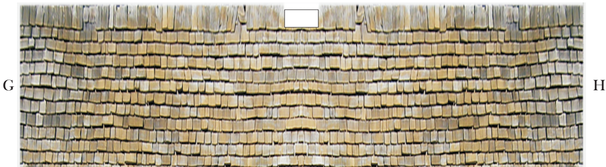
Bottom edge of Front Roof
