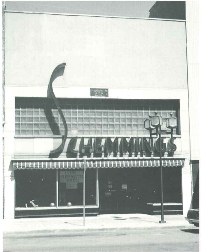
Limestone, structural glass, and glass block are combined in this modern open-front design. The sinuous S of the neon lettering unites the facade.
