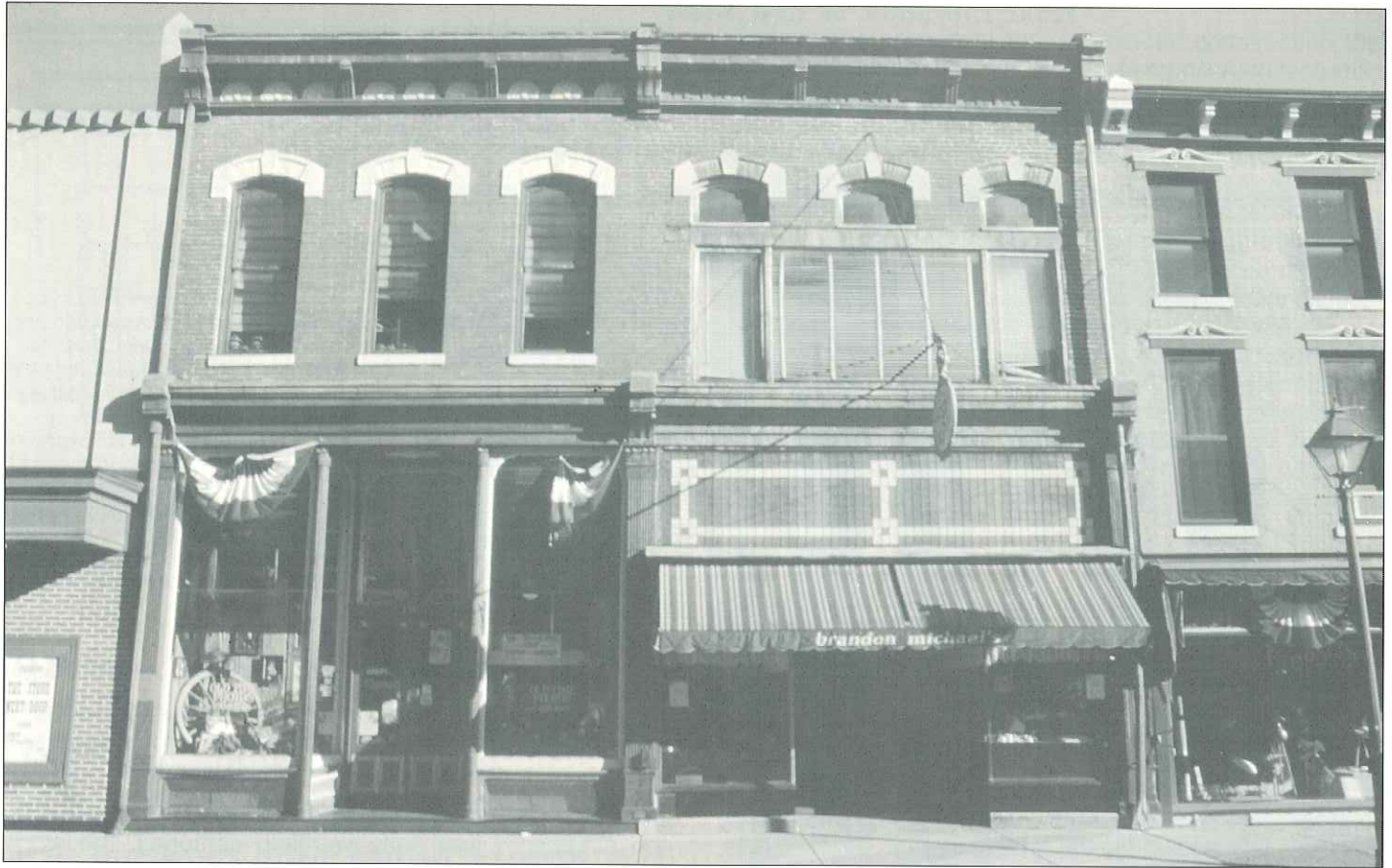
The two buildings in the center were architectural twins when constructed in the mid-nineteenth century, but the facade on the right has been altered several times over the years. The prism-glass transom and second-story windows on the right date from the early-twentieth century. The original storefront survives on the left, while the modernization on the right dates to the 1940s.
