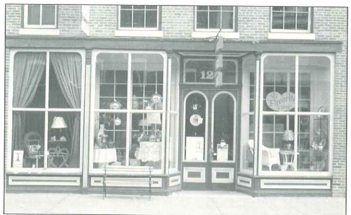
The cast-iron columns supporting the front of this Galena building, constructed ca. 1856, are extremely slender and almost indistinguishable from the millwork. The most distinctive parts of this storefront are the arched-glass doors and the multi-light sash.
