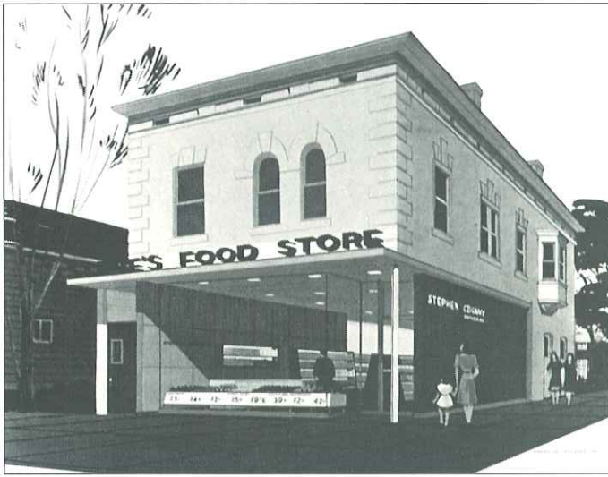
Kawneer Co. published this drawing in its folio Shopfronts of Tomorrow (1946), which promoted the open-front storefront design that would dominate storefront architecture for two decades. The aluminum framing system allowed maximum window display area.
