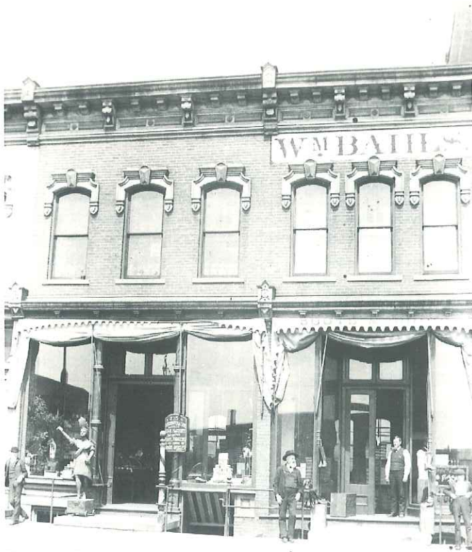
The decorative cast-iron columns on this building in Danville are one of its most distinctive features. The architectural ornament of the upper facade is stamped sheet metal. Note the large size of the plate glass.
