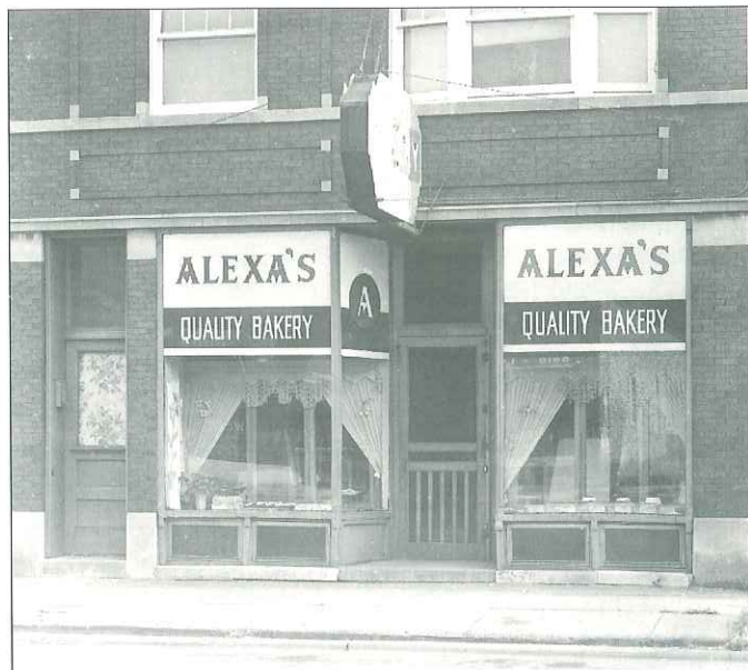
Alexa's Quality Bakery, location unknown, was located behind this simple wood storefront, which included a number of innovative features such as screens on the bulkhead windows (which allowed light into the basement) and stamped decorative metal at the corners of the sash. Contrast this ca. 1910 view of the building with the ca. 1935 view on page 12.
