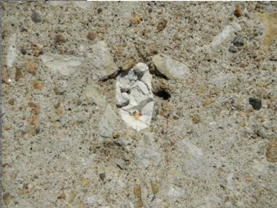
FIG. 25 Weathered surface finish differs throughout roadway segments. (Left) crushed limestone coarse aggregate and sand is exposed and (Right) rounded pea gravel and sand is exposed.
