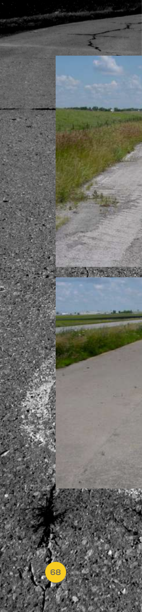
FIG. 109 Litchfield, IL. Rt. 66 bypass segments. Most of this section is covered with multiple layers of rock and oil. Camera facing north. Photograph by Travis Ratermann, 30 June 2008.
