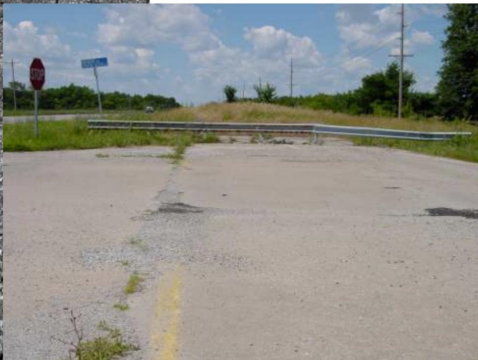
FIG. 115 Litchfield, IL. Segment on east side of bypass just north of the old RR bridge. Large embankment to the right has rolled over on to the roadway. Camera facing north. Photograph by Emilie Eggemeyer, 9 July 2008.
