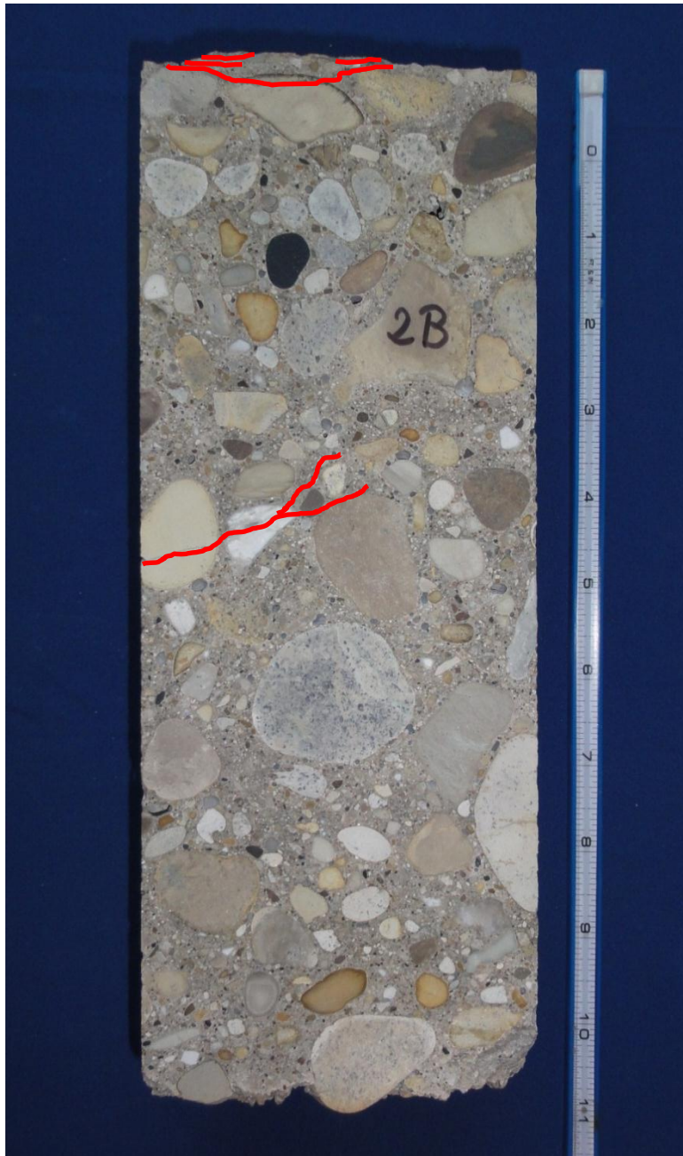
Figure 14. Lapped section of Core 2B. Crack locations are marked in red.
