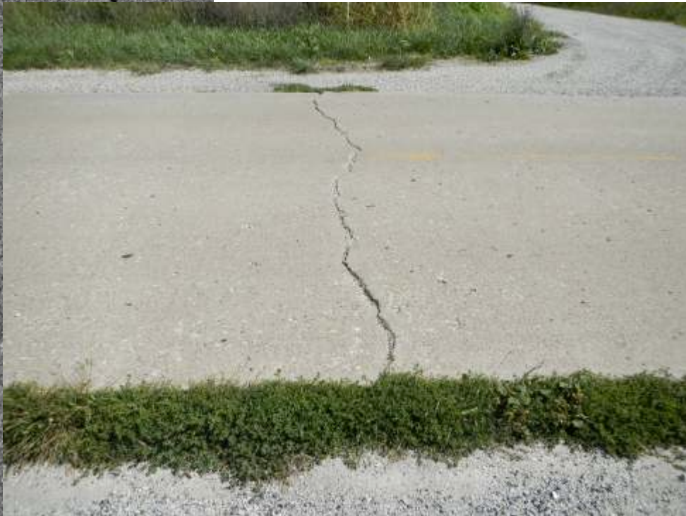
FIG. 1 Concrete in "good" condition (Girard, IL).
