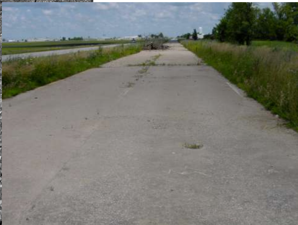
FIG. 109 Litchfield, IL. Rt. 66 bypass segments. Most of this section is covered with multiple layers of rock and oil. Camera facing north. Photograph by Travis Ratermann, 30 June 2008.
