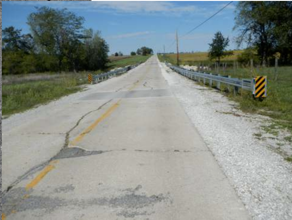
FIG. 3 Small spall previously patched with asphalt (Girard, IL).
