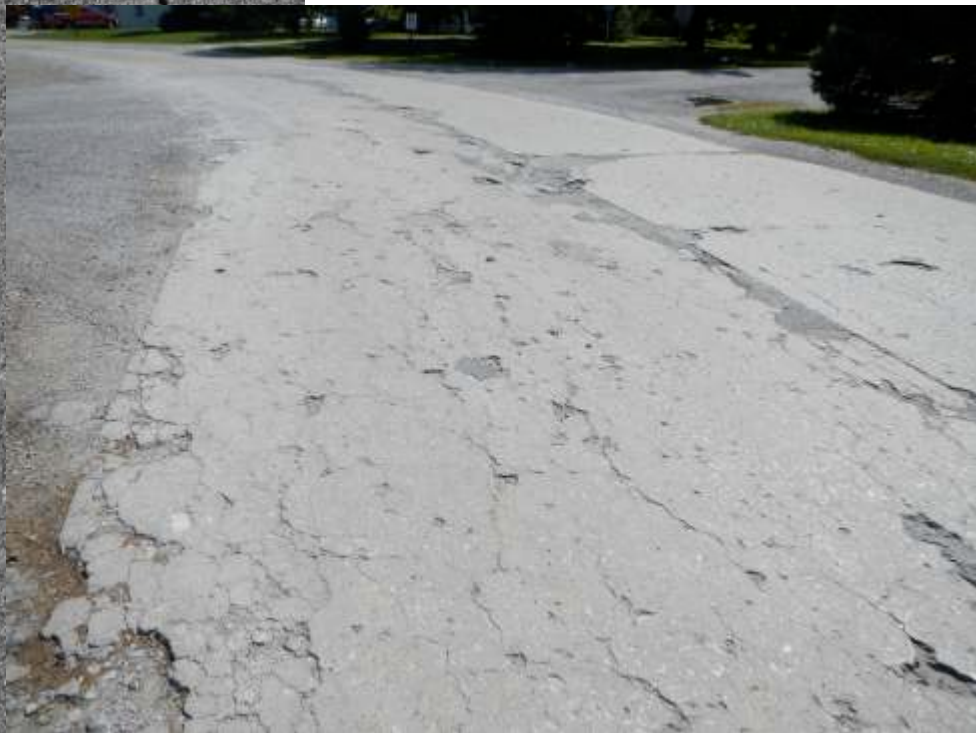
FIG. 9 Concrete in "poor" condition with multi-directional cracking and previous asphalt patches with multi-directional cracking (Nilwood, IL).
