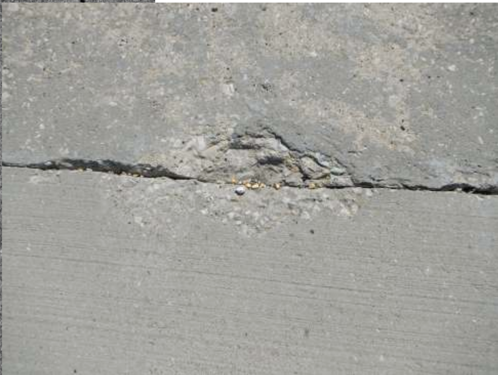
FIG. 7 Large previous patch that does not match existing concrete (south of Girard, IL).
