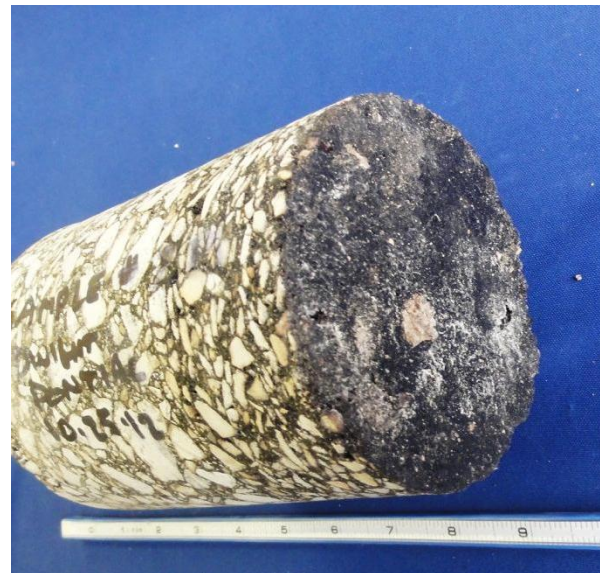
Figure 9. Bottom surface of the asphaltic core.
