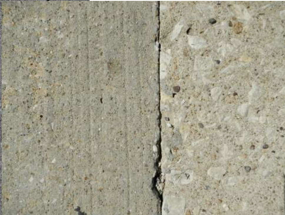
FIG. 31 Blends of cements and pozzolans to create a 'light grey buff tone' cementitious color.
