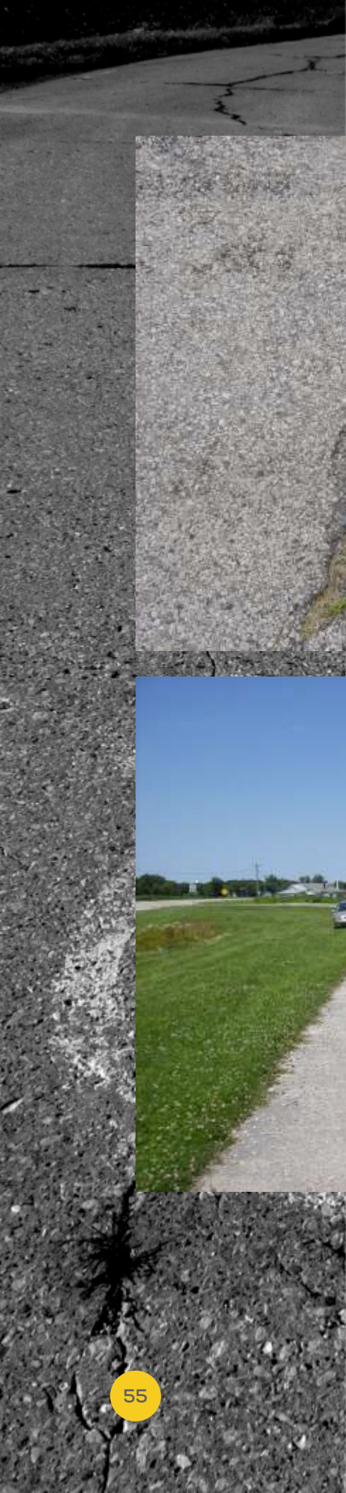
FIG. 83 Carlinville, IL. Rt. 66 segment on Deerfield Dr. Portland is covered by rock and chip that is crumbling. Camera facing south and down. Photograph by Travis Ratermann, 24 June 2008.
