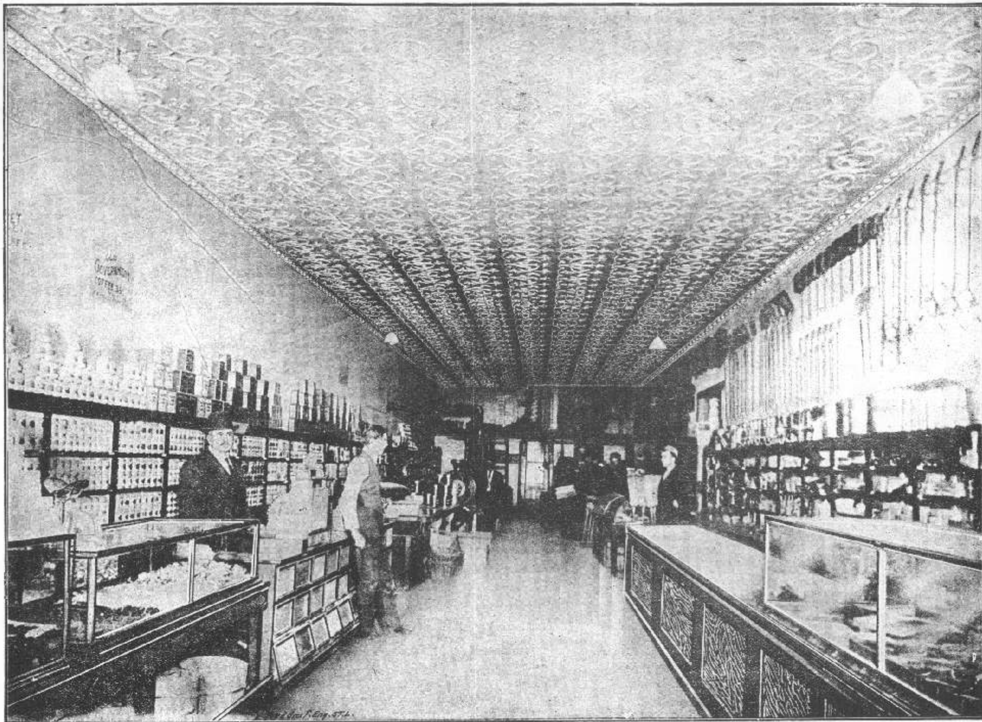
This illustration shows the interior of one of two 25x100 foot store rooms, owned and operated by Mr. G. A. Pulley, Cody, Wyo., for which we supplied the Embossed Steel Ceilings, our Design No. 1.
