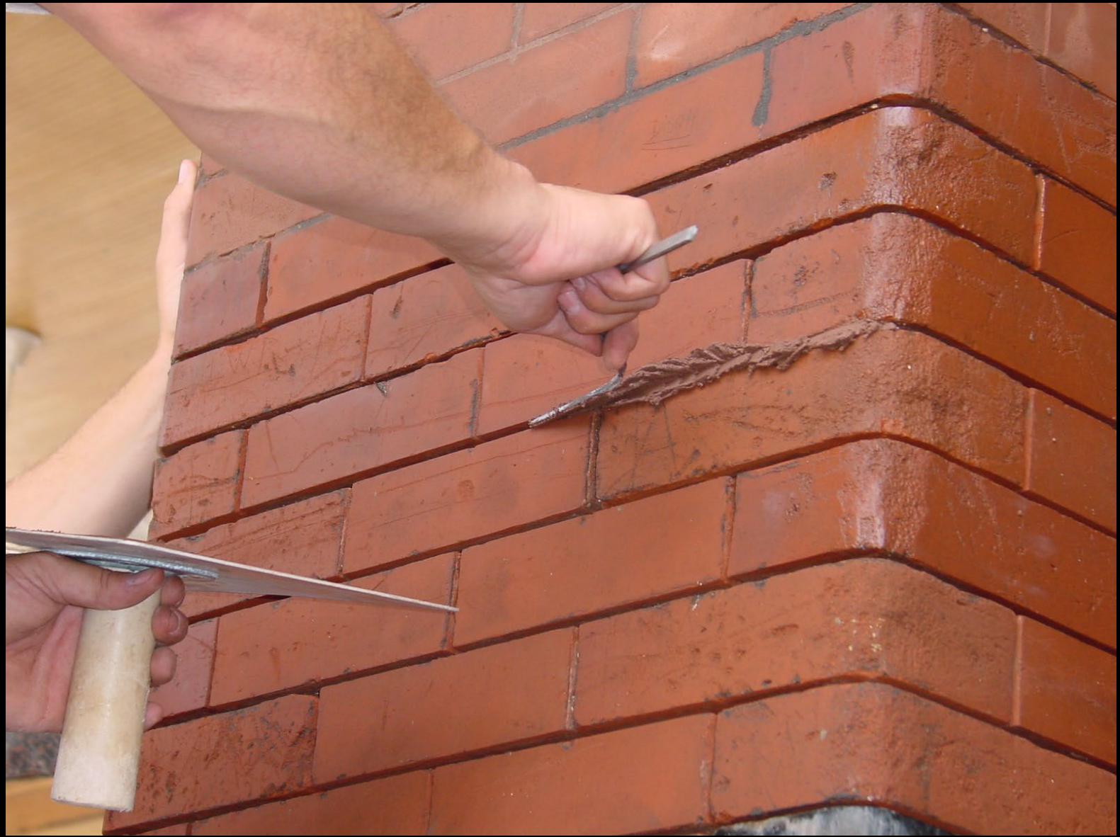
Packing the new “old” mortar
