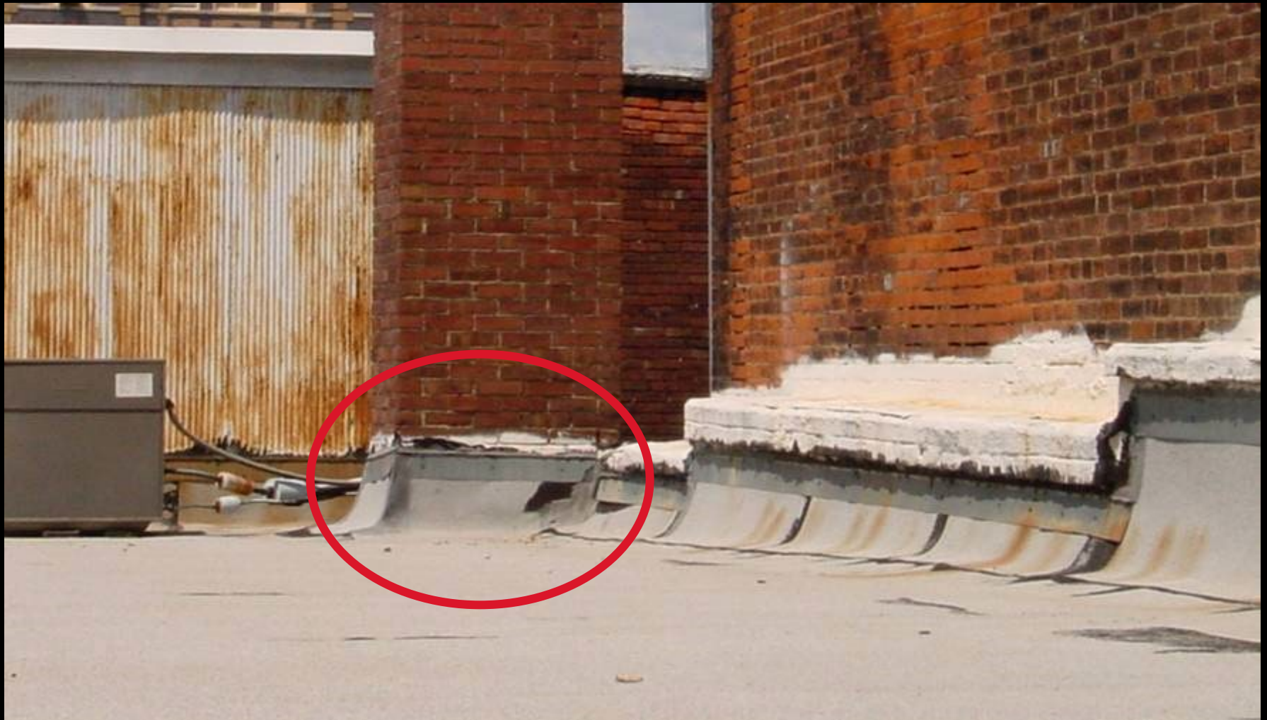
Flashing covering the connection of the roof and chimney
