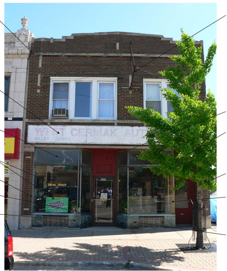
The existing sign armature may be kept if it is to be used to hang a sign. Prior to reuse, its connections should be inspected and the armature painted. Otherwise, it should be removed. All holes should be patched with mortar that matches the composition and visual characteristics of the original.
