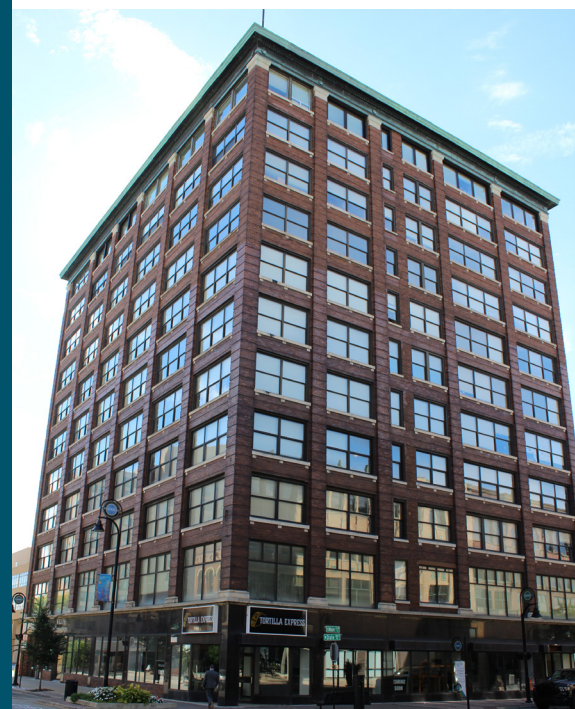
Burnham Lofts (Rockford Trust Building)
