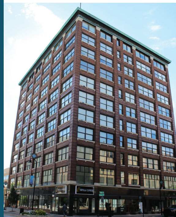
Burnham Lofts (Rockford Trust Building)
