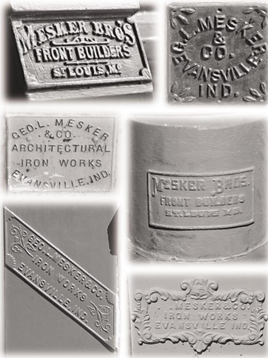
Mesker company nameplates were either molded into the bases of columns or bolted on as a plate.
