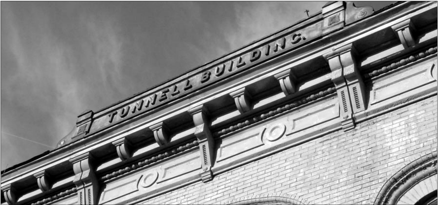
The elaborate cornice on the Tunnell Building in Edwardsville is a product of Mesker Brothers Iron Works in St. Louis.
