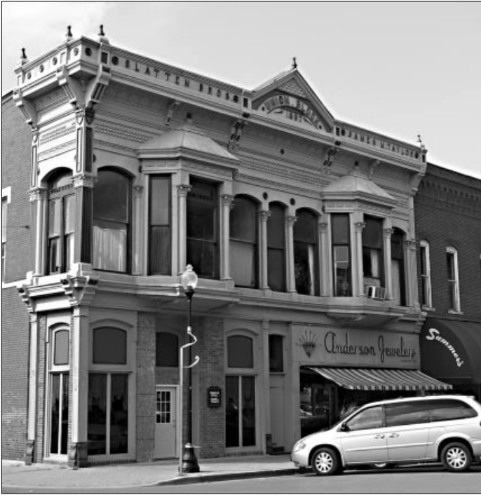
The facade of the Union Block Building in Taylorville, which dates to 1887, was manufactured by Mesker Brothers Iron Works.
