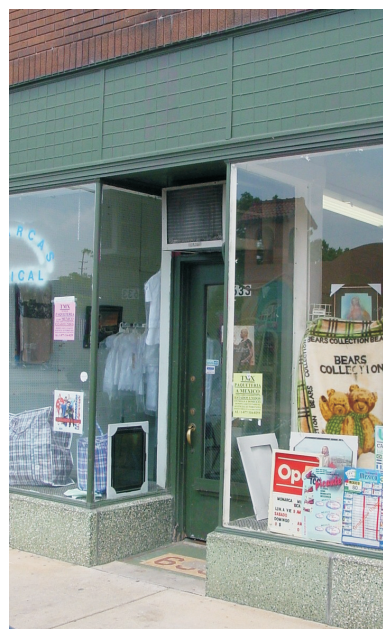
EXISTING HISTORIC DOOR
