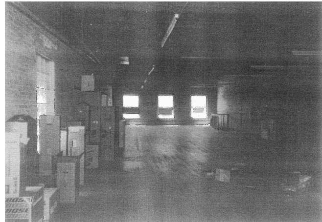
"Before" photo of second floor space
