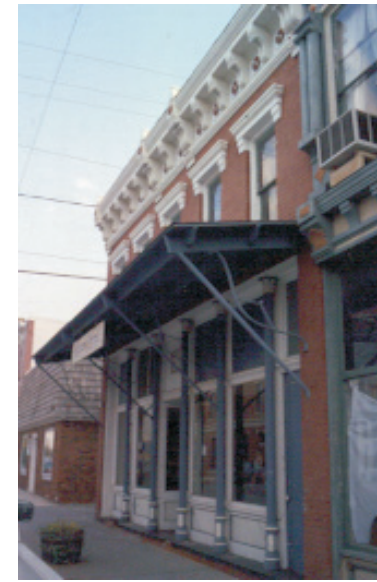
WOOD SHEATHING WITH STANDING-SEAM PANELS ON TOP
