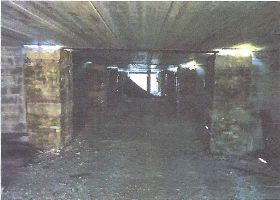
Basement - Historic Piers with 1990-era CMU walls supporting concrete plank flooring
