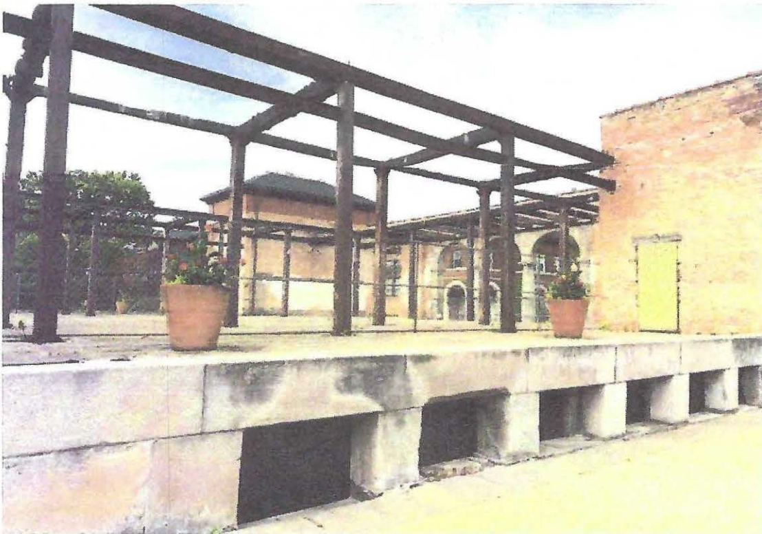
North Façade Basement Window Openings and Extant Steel and Wood Framing Remnants
