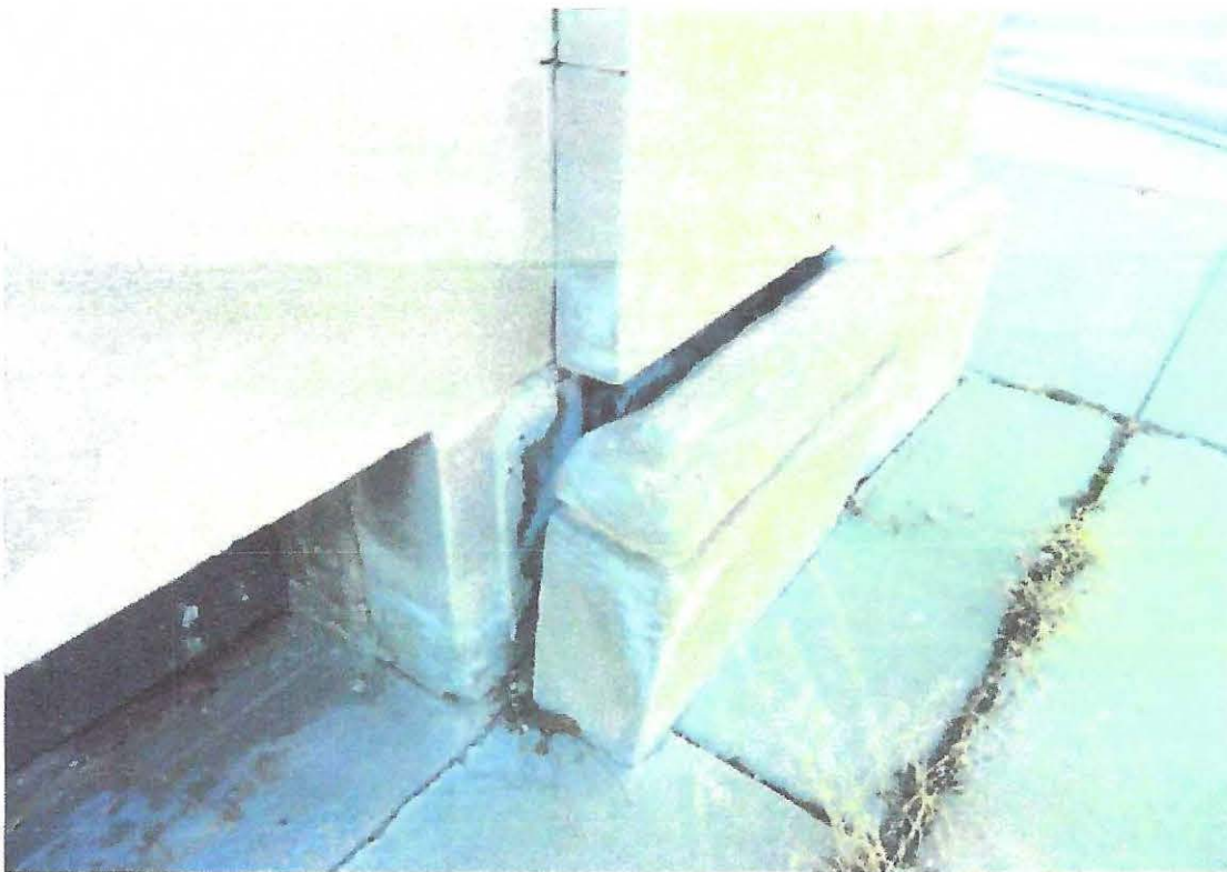
Failing Stone on All Facades
