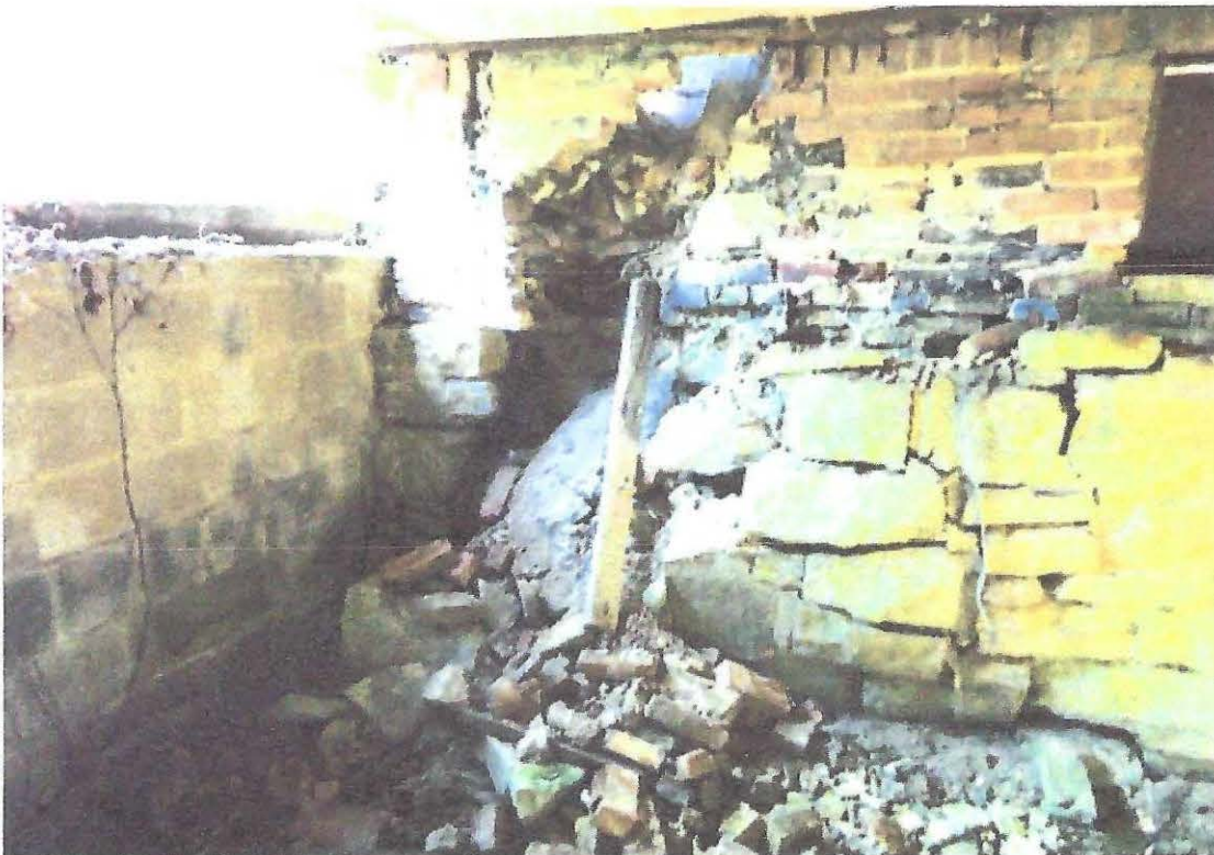
Chimney Foundation Failure at West Wall
